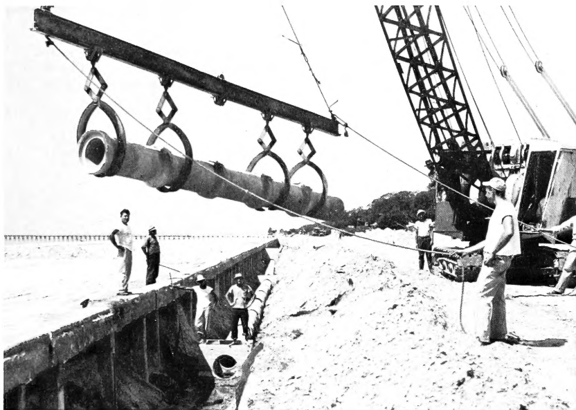
FIGURE 3. LAYING COLLECTING DRAIN BEHIND SEAWALL
