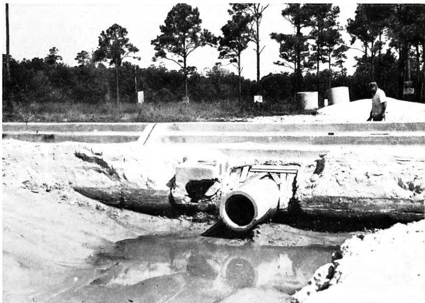
FIGURE 4. DRAIN OUTFALL THROUGH SEAWALL (Old outfall at left.)
