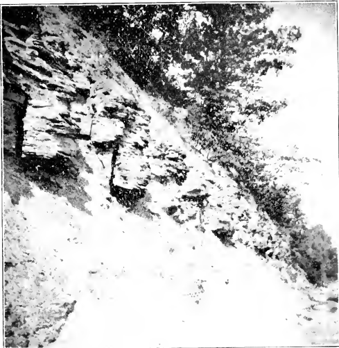
(b).—View of the Genesee shales of Section 4, showing the characteristic jointage of the black shales. —Photographed by A. W. GRABAU.
