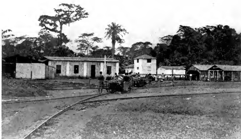
Fig. 1.—Electric switch station, carpenter's workshop and mono rail.
