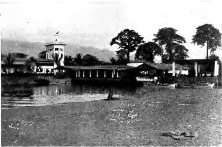
Fig. 1.—Bibundi Estate. Manager's house, showing landing jetty and beach stores.
