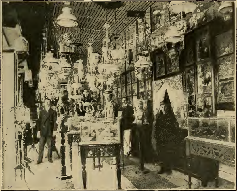
INTERIOR OF A RETAIL STORE IN BARRANQUILLA, COLOMBIA.
