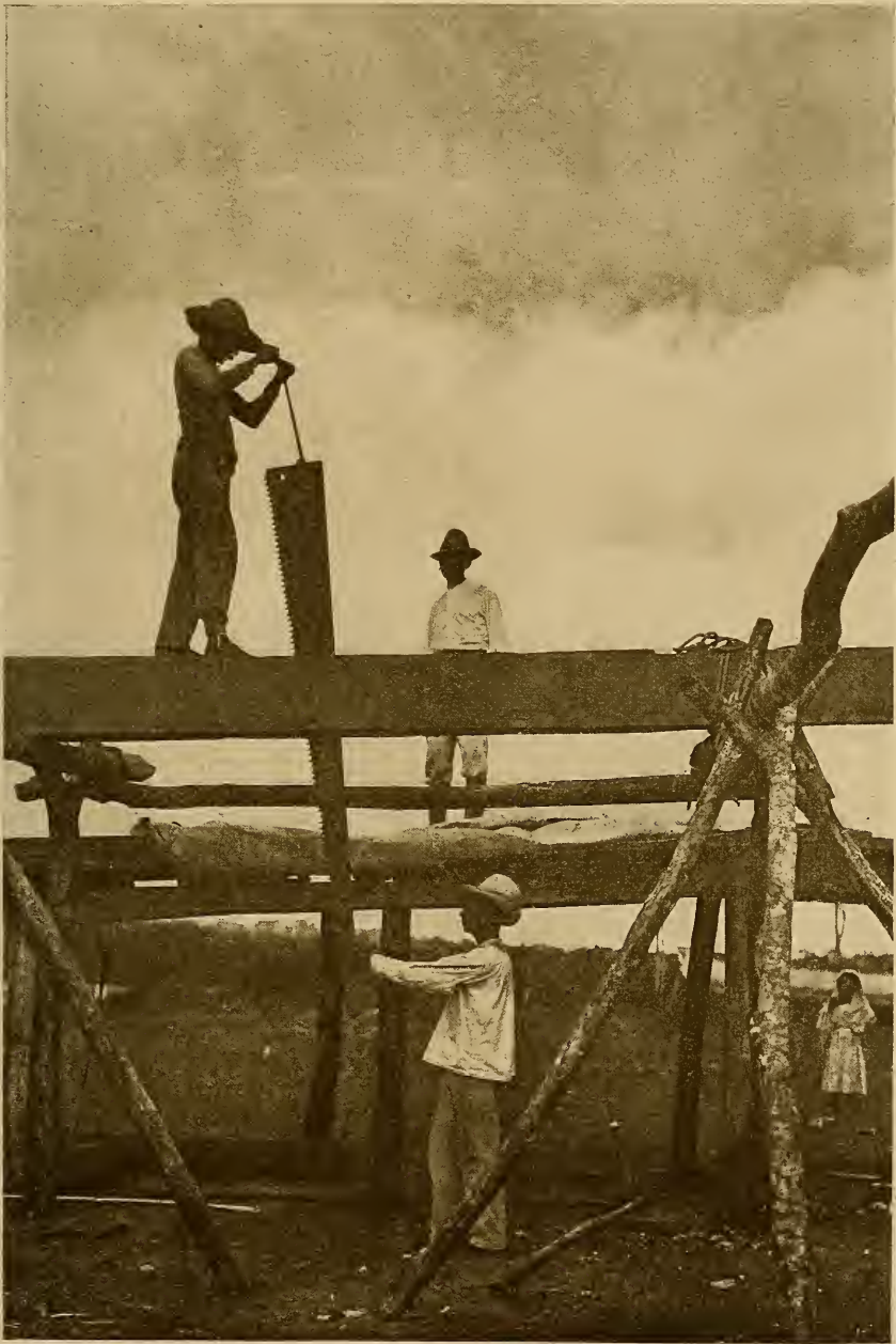
SAWING THE LOG INTO LUMBER.
