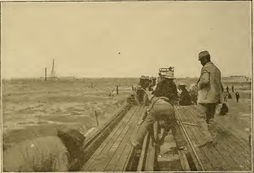
TRACK LAYING NEAR ORURO.
