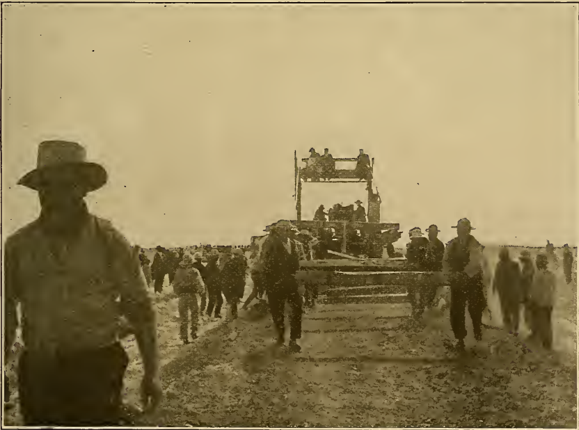
TRACK LAYING INTO ORURO.
