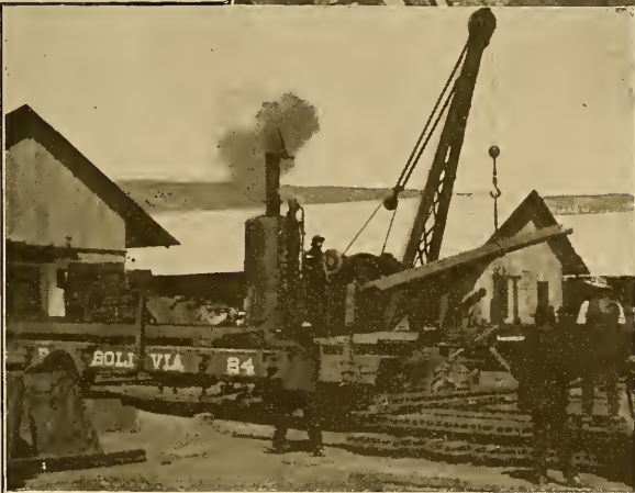
UNLOADING TIES AND RAILS AT GUAQUI, BOLIVIA.
