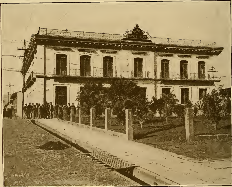
THE MERCANTILE BANK OF COSTA RICA, SAN JOSE.
