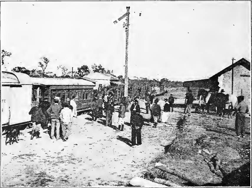
A RAILWAY STATION IN THE QUEBRACHO WOODS.
