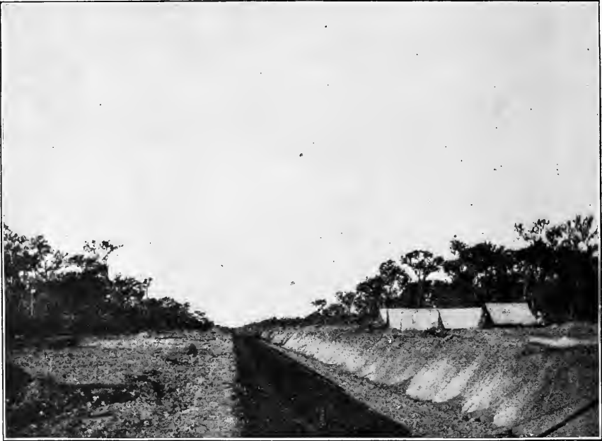
A RAILWAY RECENTLY CONSTRUCTED IN "THE CHACO."
