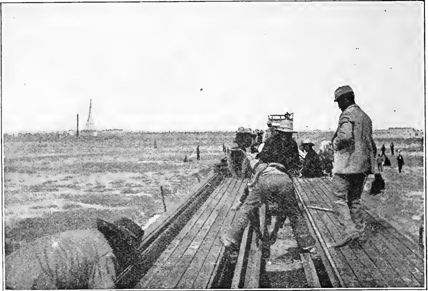
TRACK LAYING NEAR ORURO.
