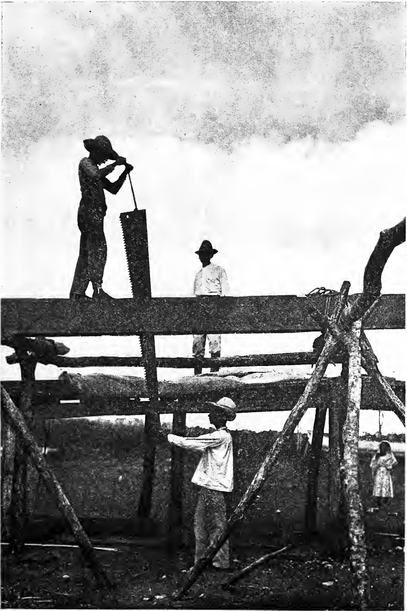
SAWING THE LOG INTO LUMBER.
