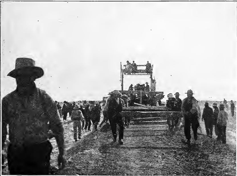
TRACK LAYING INTO ORURO.
