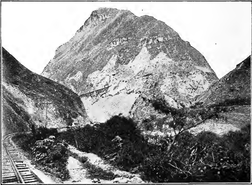
DOUBLE ZIGZAG TRACK FROM THE DEVIL'S NOSE NEAR ALAUSI ON THE GUAYAQUIL AND QUITO RAILWAY.
