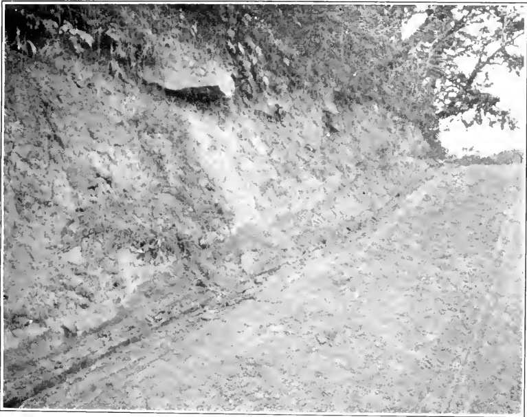
Fig. 9. A highway-cut, about 65 feet below the highest point of Claggett's Hill, in residual soil: in upper part of Section is a block which has crept down from above.
