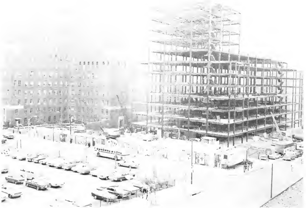
GROWS NEARER COMPLETION —A maze of steel fabrication forms the North Hospital building in mid-December as it approaches completion. University Hospital can be seen adjacent to the construction which has a decorative fence painted by local artists to enhance the beauty of the construction area.
