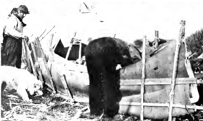
Assembling bark over on building site.
