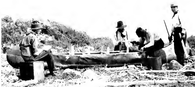
Setting ribs inside bark cover with a mallet.
