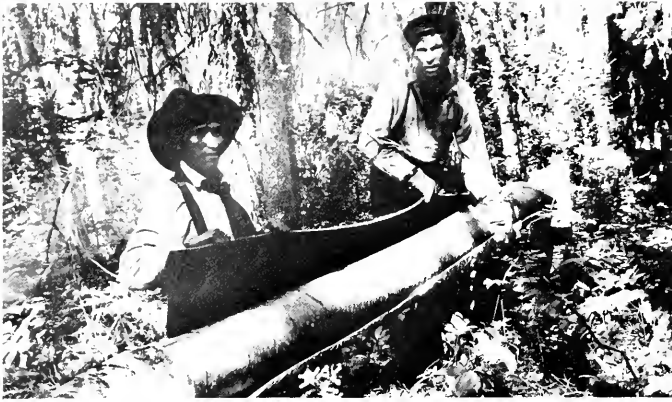
Figure 155 OJIBWAY CANOE CONSTRUCTION. (See pp. 122-131.)
