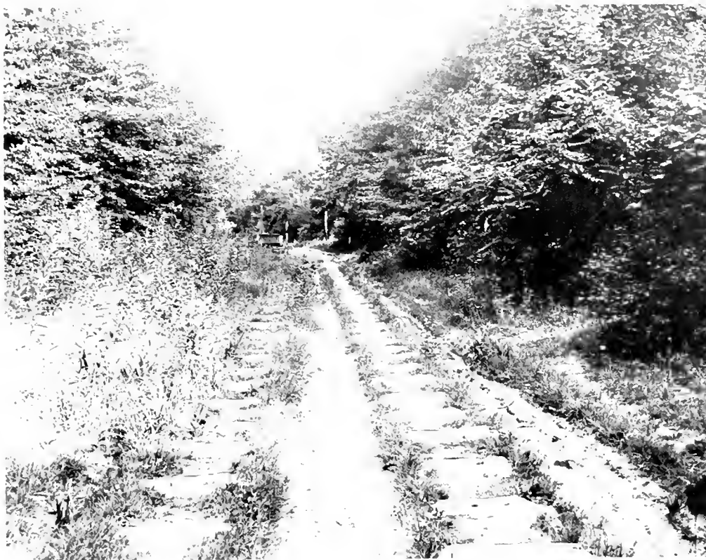
FIGURE 63.—Roadbed of abandoned Portage Railroad. Note the closely spaced granite blocks. From an original photograph in division of transportation, Smithsonian Institution.
