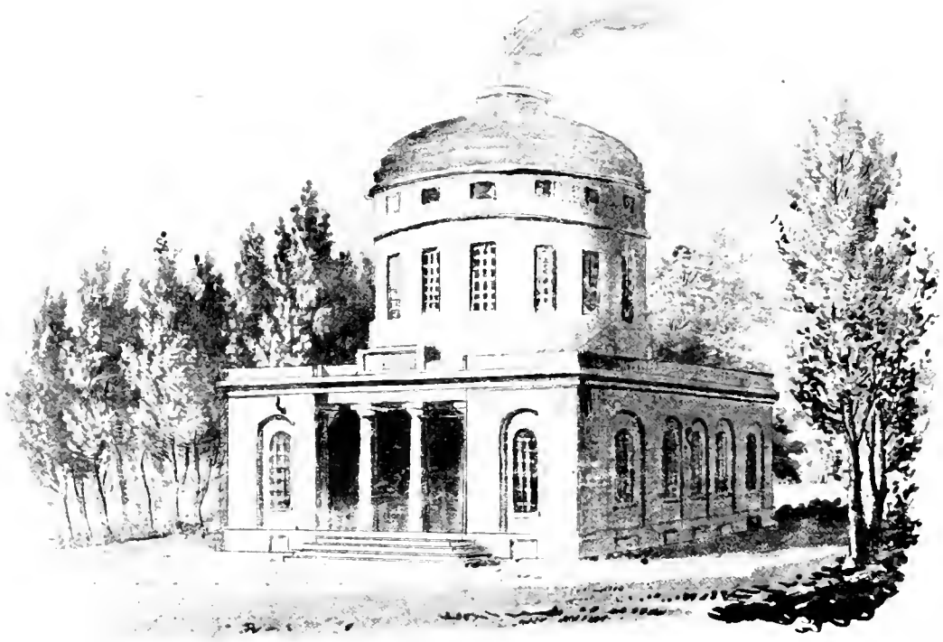
FIGURE 21.—Center Square Water Works, Philadelphia. From Charles W. Janson, Stranger in America (London, 1807). Library of Congress photo.
