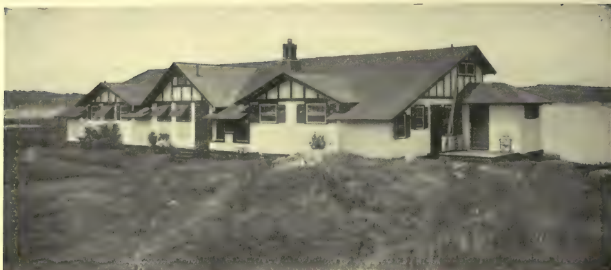
A particularly good example of the seacoast bungalow—where the plan is extremely long, following the line of the shore and giving almost all the rooms the water view
