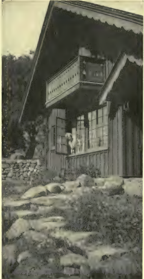
See also Frontispiece and pp. 46, 61 Myron Hunt & Elmer Grey, architects The characteristic ornament of the Swiss chalet type—sawed-out eaves boards and balcony railing
