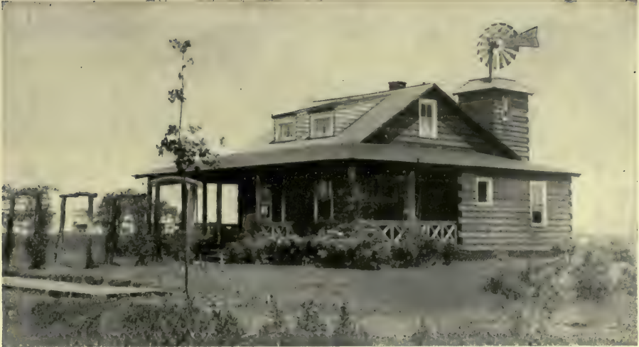
The windmill is usually passed over as a possibility for water supply on account of its unsightliness. In this example, however, the designer has incorporated it rather ingeniously with the design of the whole building
