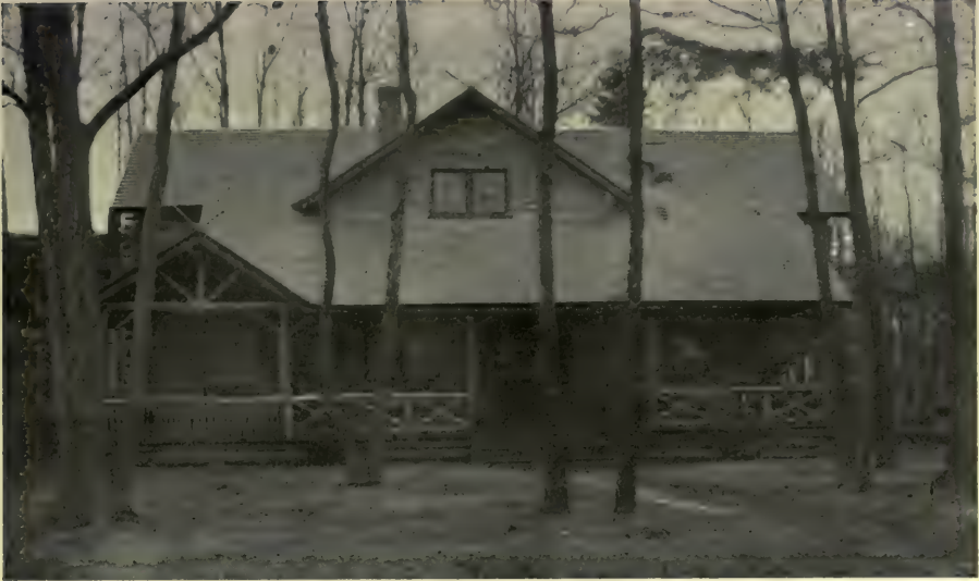
In this log structure the logs project one over another at the right-hand end to form a support for a balcony
