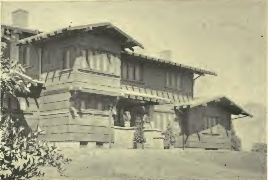
Other exteriors on pages 57, 115; interiors on pages 145, 151 — Gco. A. Clark & L. du P. Millar, architects The roof of the Childs California home is covered with one of the prepared roofings that comes in a dull lead color
