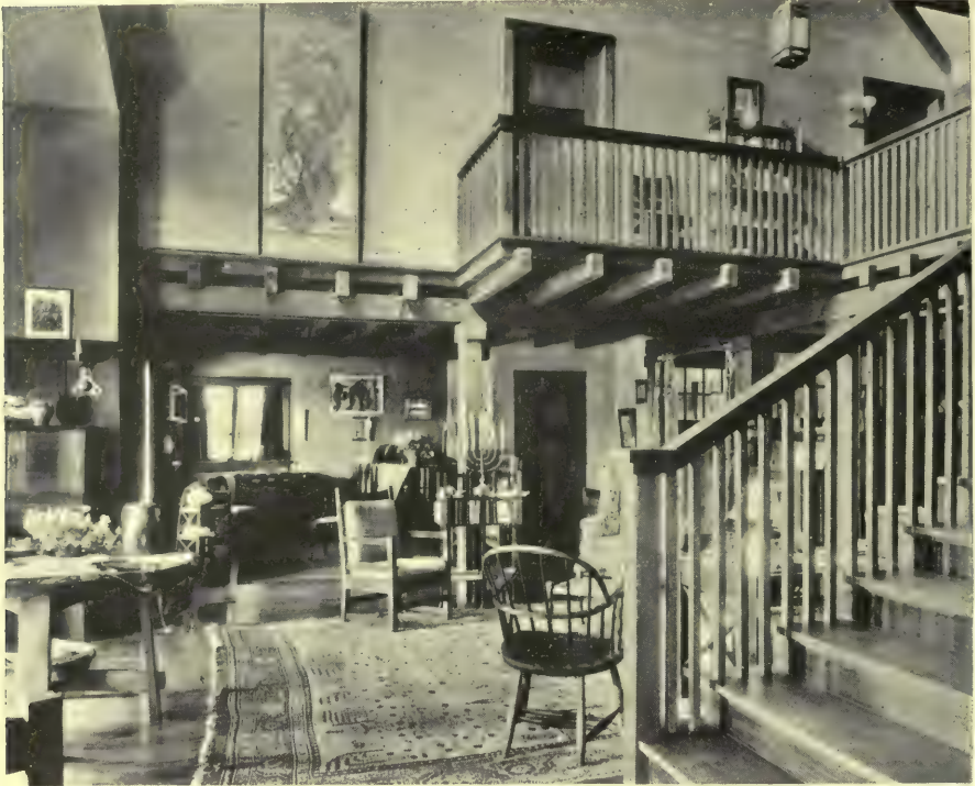
An interesting effect has been secured by leaving the floor joists uncovered to form the ceiling of the first story. The balcony is supported on these floor joists as cantilevers
