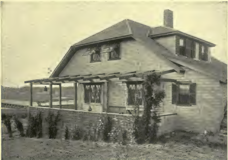
There is an excellent suggestion here in the Haynes house for a method of building porches that will not cut off light from the most important rooms of the house. The framework may be covered by a roll awning when desired
