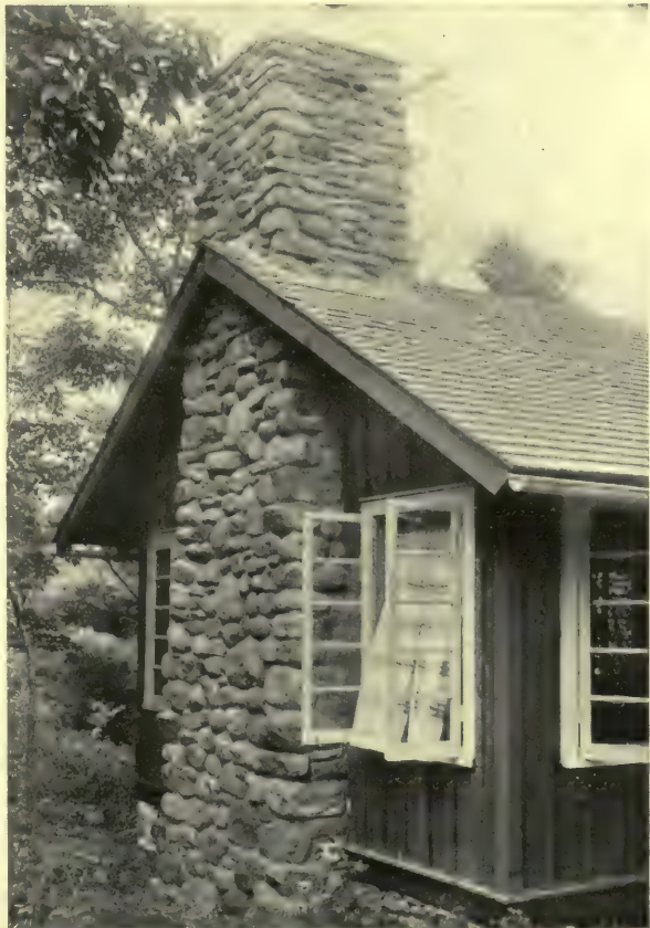
The chimney of rough stonework seems in many ways to be more appropriate for use with a rough wooden building than a chimney of brick or cement
