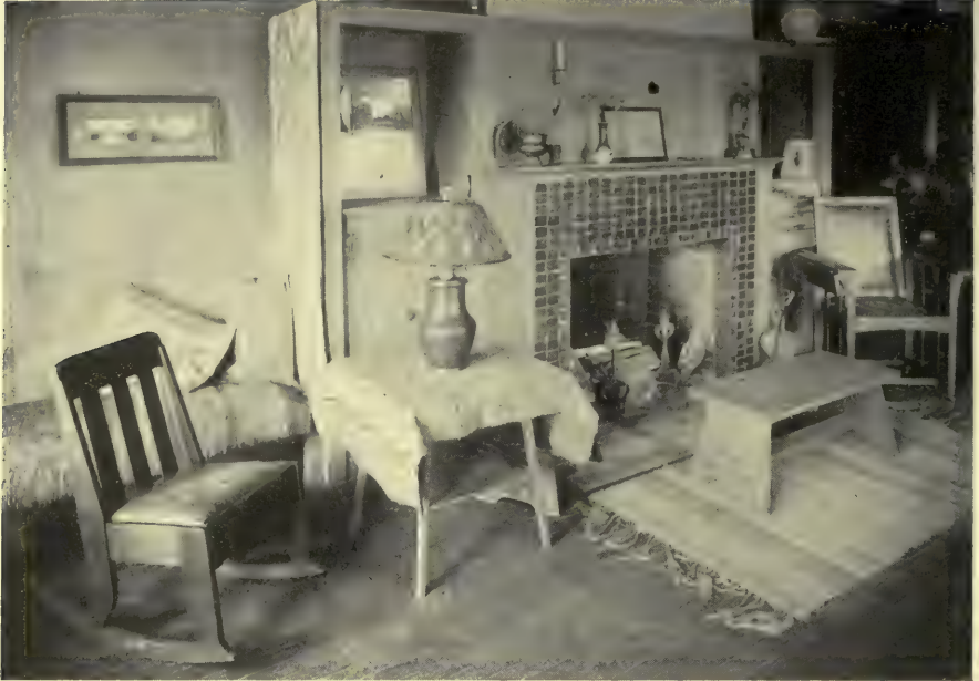
The facing of dark red hand-made tile has been applied over the facing of rough brickwork. The best way to get and keep these tiles most attractive is to rub them occasionally with linseed oil
