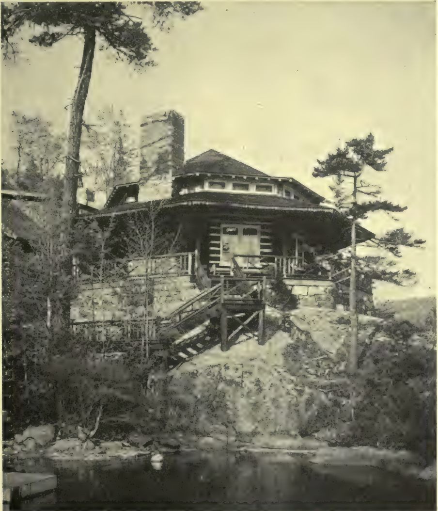
Exteriors pp. 30, 94, 100, 111, 153; interiors pp. 118, 148, 150, 152. Davis, McGrath & Shepard, architects The typical Adirondack lodge, this particular example being on Lake Wilbert, Franklin County, N. Y. The structure is of smooth logs with plastered chinks
