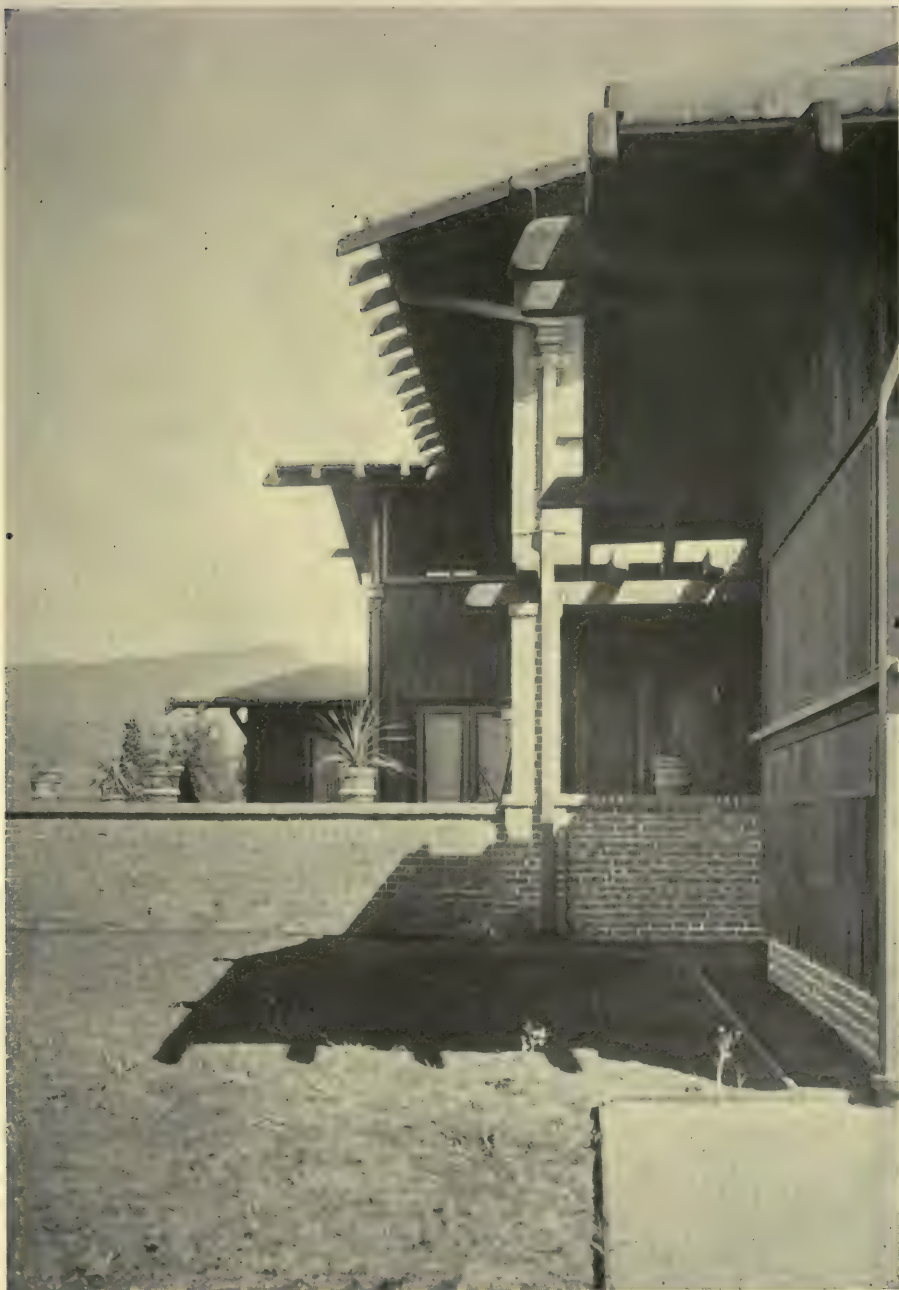
Other exteriors on pages 57, 114; interiors on pages 145, 151 Geo. A. Clark & L. du P. Millar, architects The roofing is turned over a rounded edge at the eaves in a way that gives it the appearance of a solid lead roof. The roof rafters inside are sheathed, the spaces between them being filled with sawdust to keep out the heat
