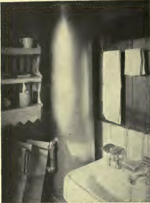
The kitchen boiler in this little bungalow was placed on the other side of the kitchen partition, bringing it into the bathroom, which room it serves to heat
