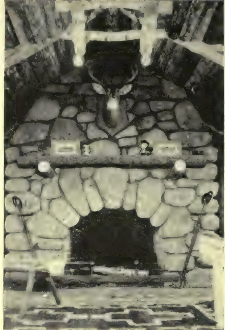
A very good piece of arch work with large stones and raked-out joints. Notice the shelf of a half-log supported on log pins
