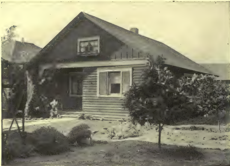
Clapboards differ but slightly in appearance from the overlapped boards, but they are narrower. The cost was $700
