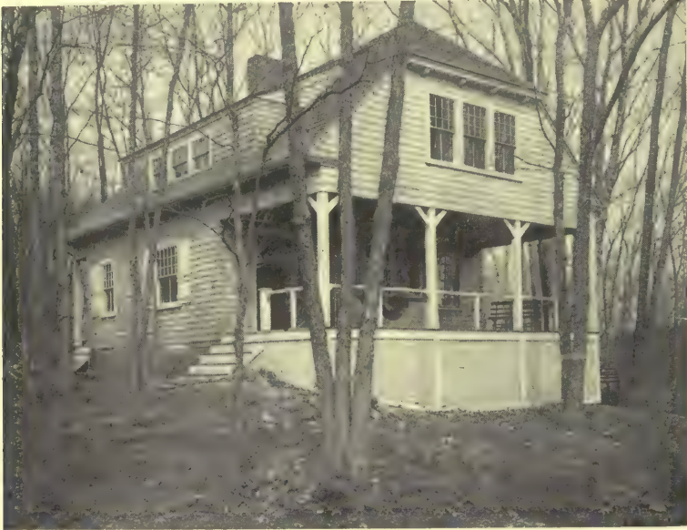
Plan on page 57; interiors on pages 80, 81, 130 William P. Hubon, architect Mr. Hubon's camp near Salem, is said to have been built at a cost of $1100, of shingles that have been allowed to weather
