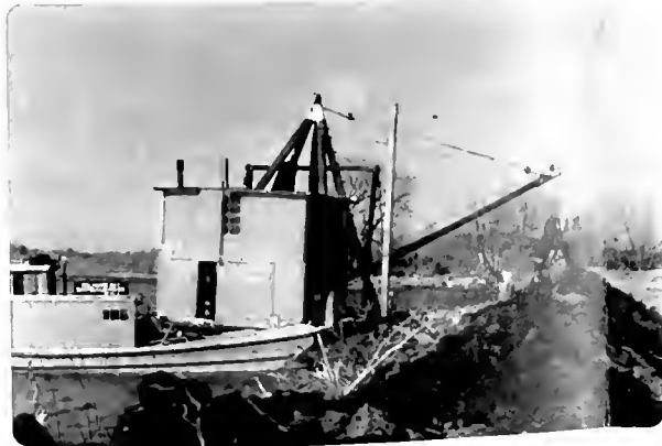
Old "Muddigger" used to repair dykes in 1960's
