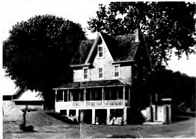
East face before Re-stuccoing in 1984.
