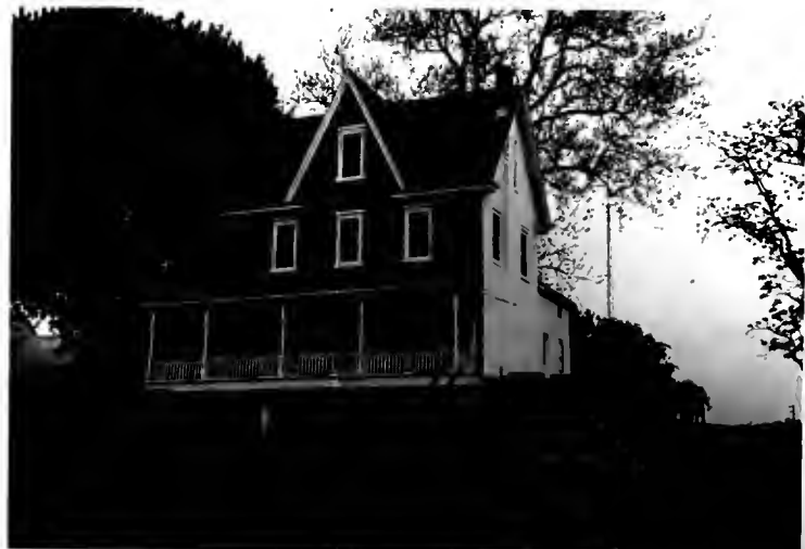
1995 Southeast corner after stuccoing.
