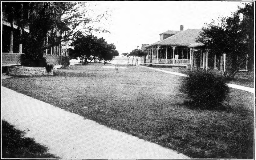
Laboratory on the left, mess house and pump house on the right.
