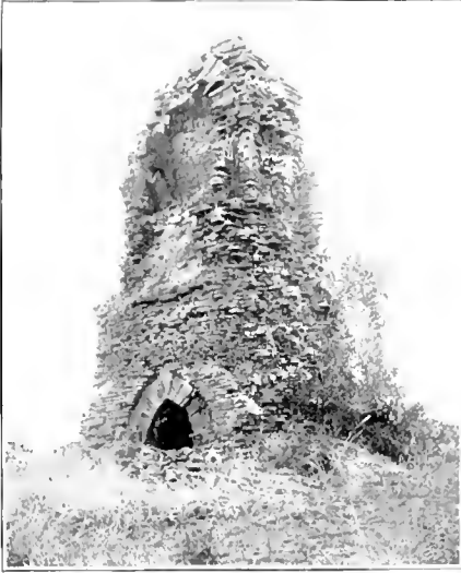
75. EXAMPLE OF KEYED VAULT AT PAGAN
