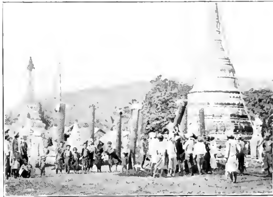
123. REARING THE POSTS OF THE WUT.
