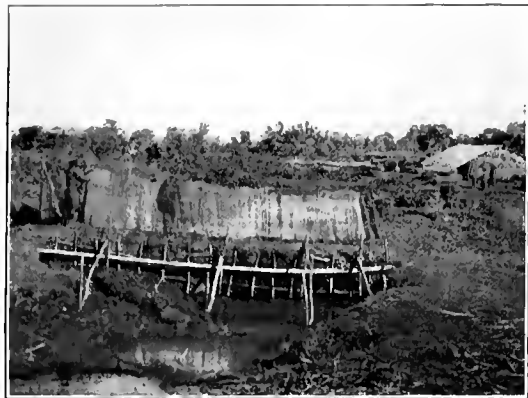
198. SLUICE OF LAGOON FISHERY (IN)
