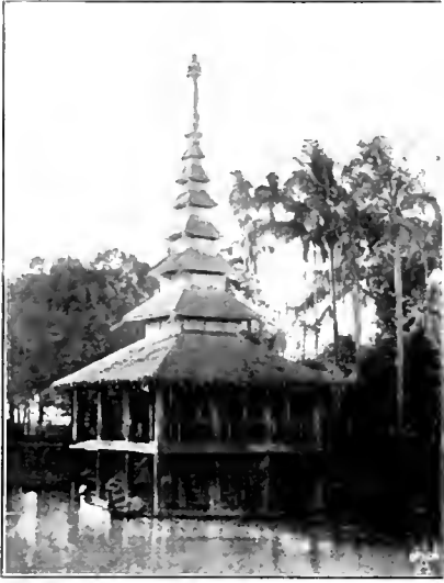
5. LANDING-STAGE IN THE TIDAL REGION
