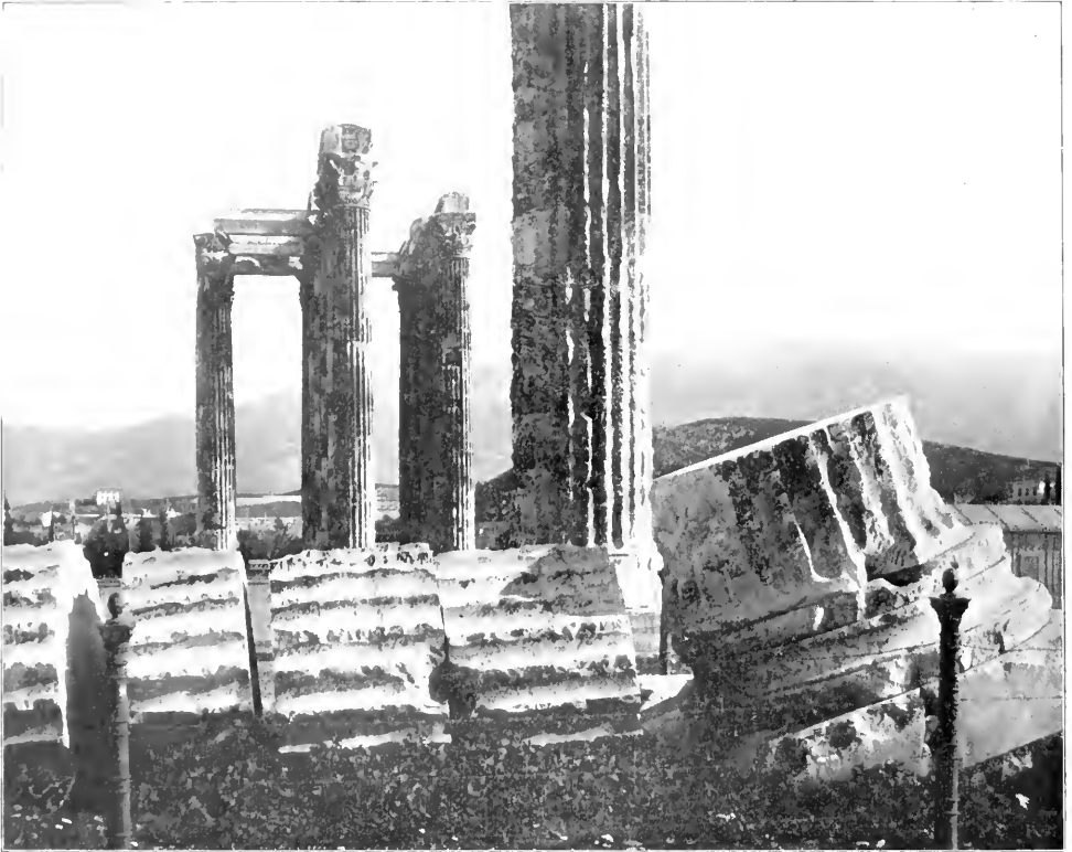
A FALLEN COLUMN
