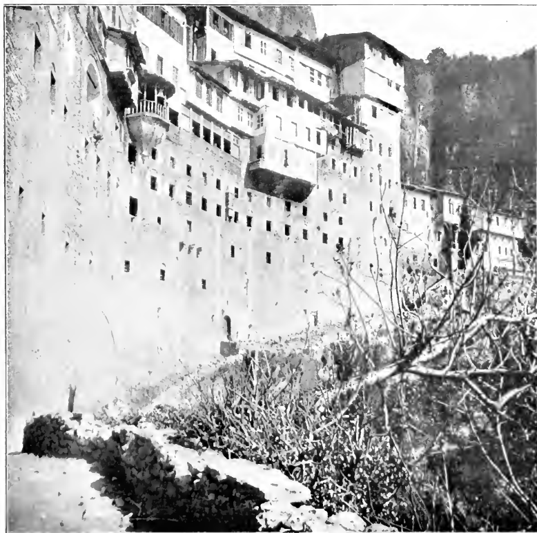
THE CELLAR WALLS
