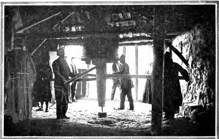
THE HOISTING "MACHINERY"
