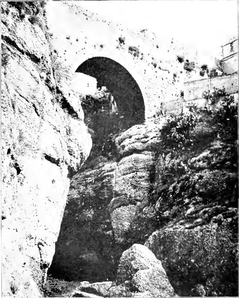
A ROMAN BRIDGE
