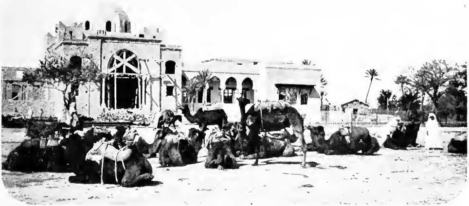
THE CASINO IN CONSTRUCTION
