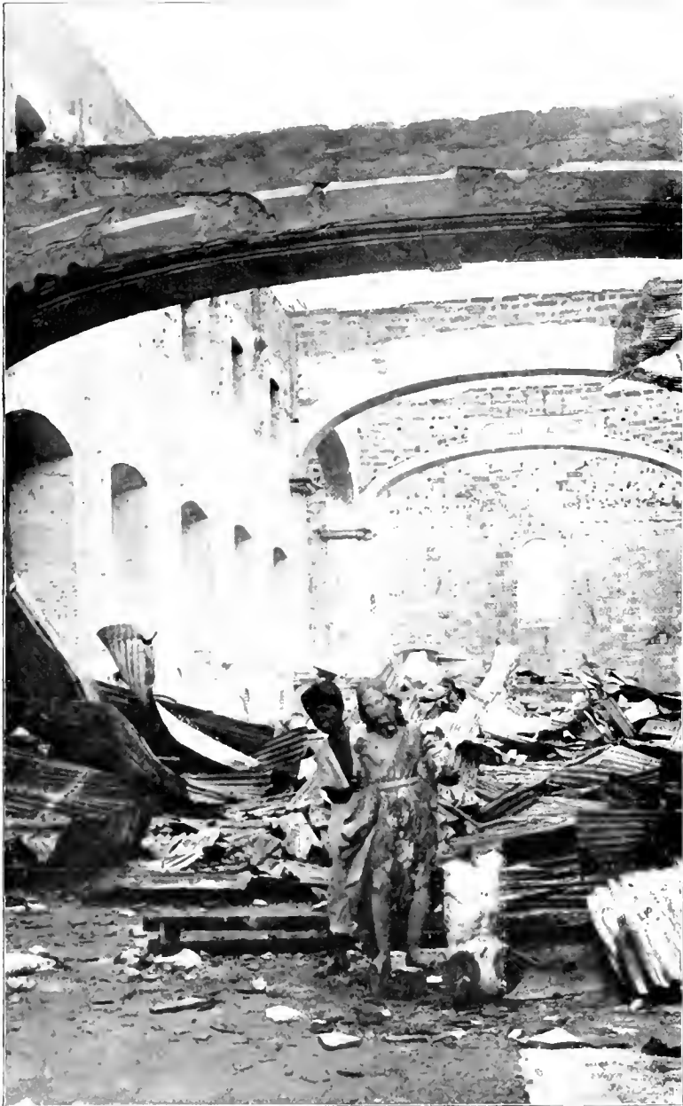
FILIPINO WORK AT SAN FERNANDO
