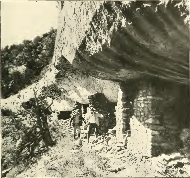
ABANDONED CLIFF DWELLINGS IN WALNUT CAÑON
