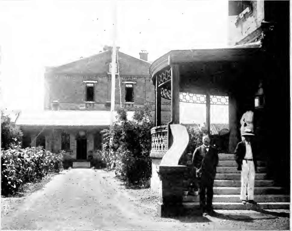
THE AMERICAN CONSULATE AT TIEN-TSIN
