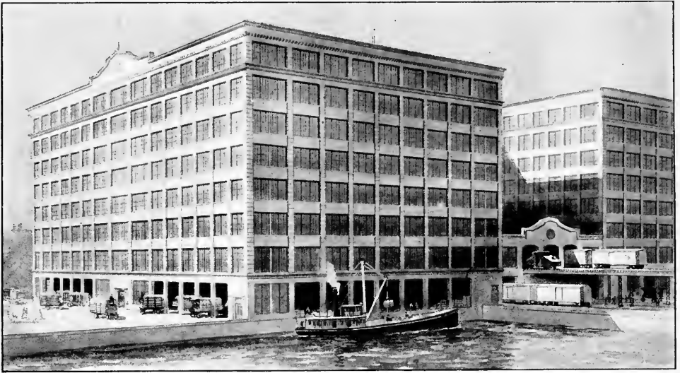
View of new Bush Terminal Service Building
