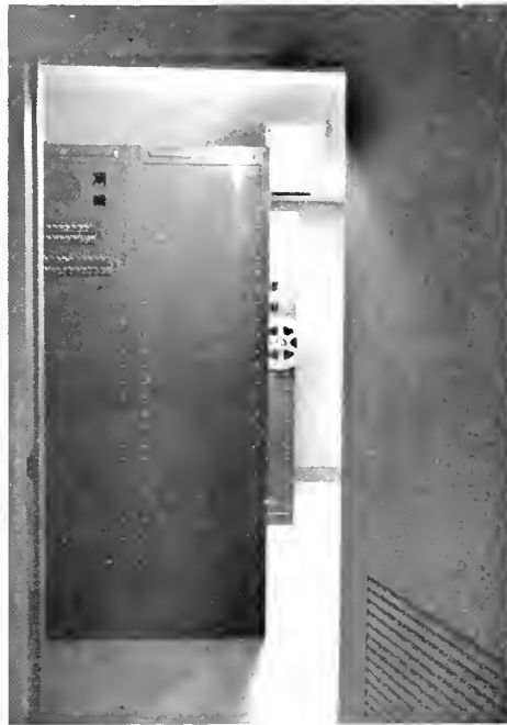
Above: control room of the Socony-Mobil sound system. Serving 650 speakers throughout the building are 19 RCA amplifiers in these racks, one for each floor of Socony offices. Tape reproducer is a Magnecorder 814. Music is controlled by IBM clocks, delivered for 15-minute and half-hour periods daily.
