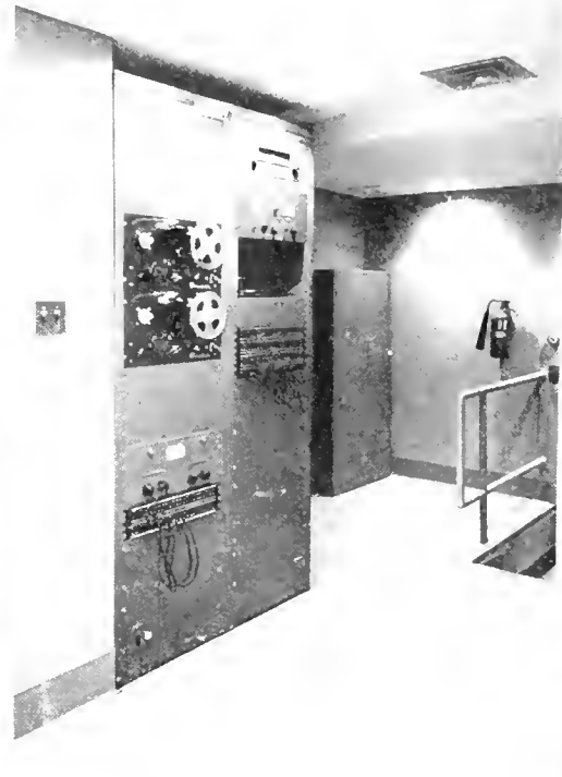
Above: control room of the Socony-Mobil sound system. Serving 650 speakers throughout the building are 19 RCA amplifiers in these racks, one for each floor of Socony offices. Tape reproducer is a Magnecorder 814. Music is controlled by IBM clocks, delivered for 15-minute and half-hour periods daily.
