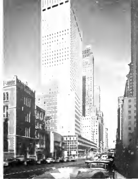
This 45-story stainless steel-sheathed tower houses the new headquarters offices of the Socony Mobil Oil Company in New York.
