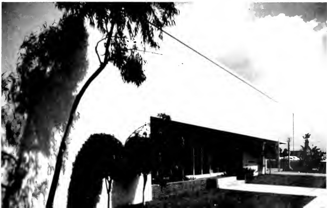
Functional design which expresses its purpose is exemplified in front facade view of the Audio-Visual Center.
