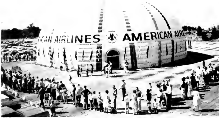
The Astrosphere: said to be largest dual-walled air-inflated unit built.
