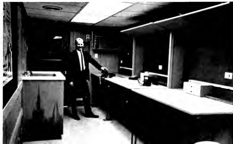
Below: workshop section at rear of van has bench space for actual demonstrations and for student participation; unit has own power, a/c conditioning, heating and water system.
