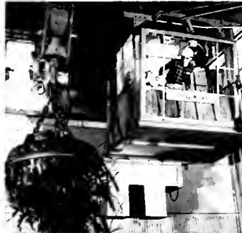
The Craneman guides magnet-lift of scrap, watchful of men on floor.
