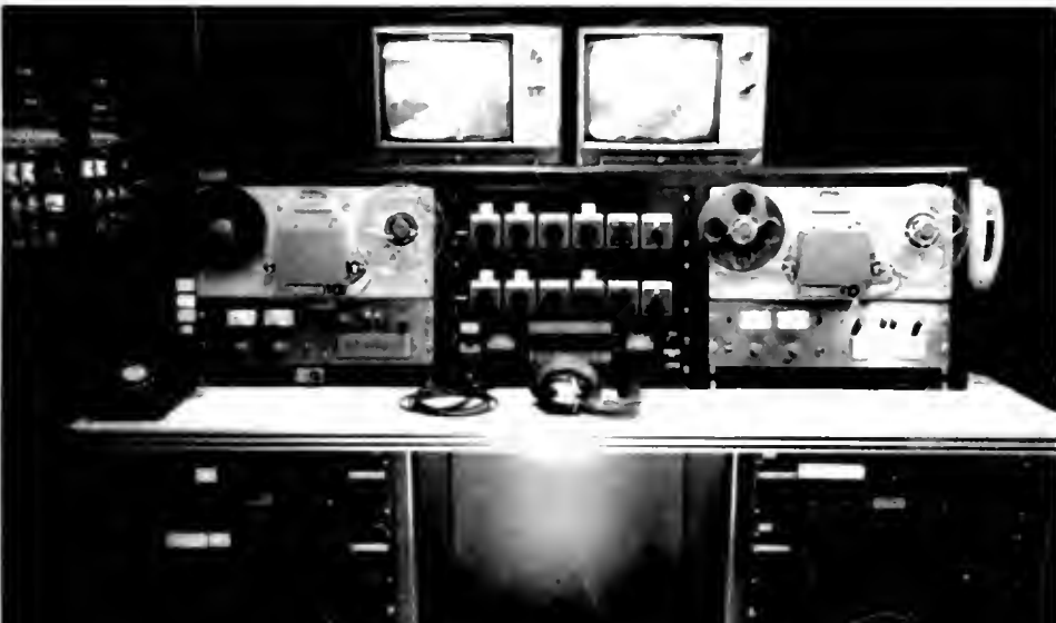
Master sound console with duplicate set of podium controls for Rooms 1 and 2 at the left
