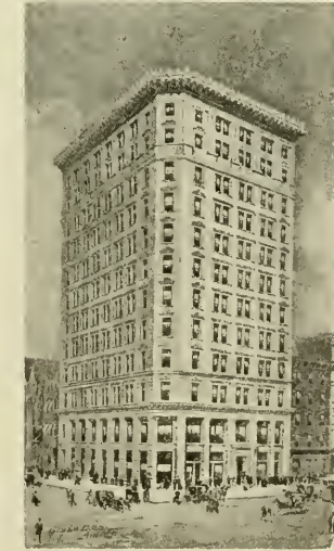
Townsend Building, N. Y. City, where the Eastern office of the Gregg Publishing Co. is located.
