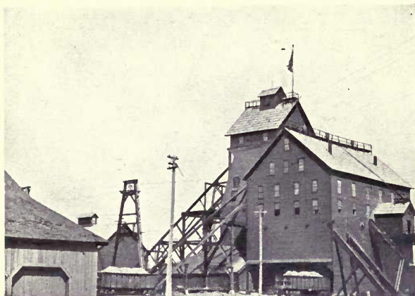
Shaft No. 3, TAMARACK MINING COMPANY, CALUMET, MICHIGAN.
