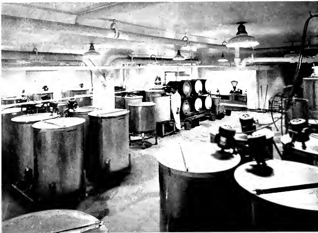
Chemical mixing room: here's where the basic ingredients must be blended for their journey to the developing machines on the floor below. All tanks are stainless steel, equipped with Eastern mixers.
