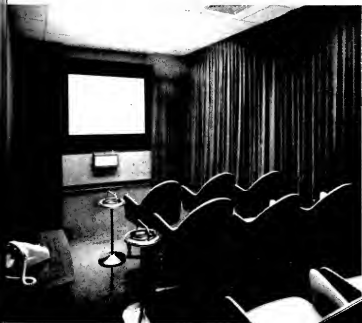
At the left: this comfortable smaller projection room on first floor is conveniently located for customers to check answer prints. Below: on the second floor, this sound-mixing studio (see pp. 14,15) features an eight-position Westrex sound mixing console; electronic counter below screen is for both 16 35mm footages. Altec Lansing speakers assure the quality of sound.
