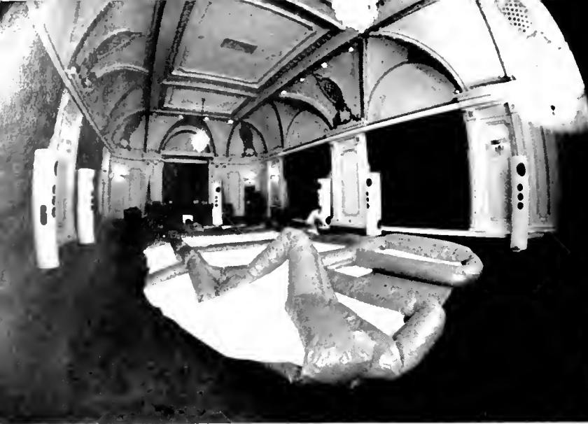
Plastic theatre in the process of being inflated (left) rises to full size (right). Pillars around the outside house the projectors and sound equipment
