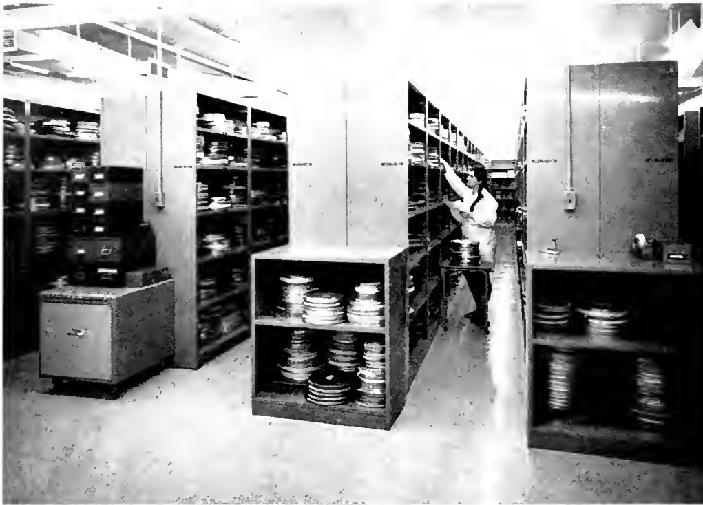
A section of the laboratory's active, humidity-controlled film vault. Note cans stored on sides.
