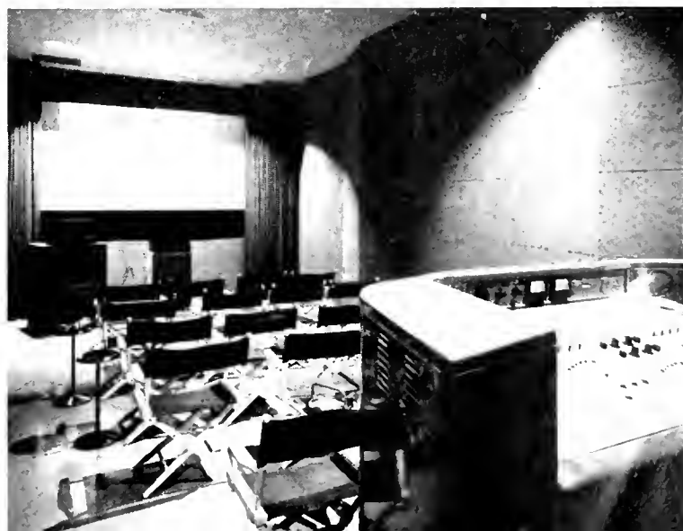
At the left: this comfortable smaller projection room on first floor is conveniently located for customers to check answer prints. Below: on the second floor, this sound-mixing studio (see pp. 14,15) features an eight-position Westrex sound mixing console; electronic counter below screen is for both 16 35mm footages. Altec Lansing speakers assure the quality of sound.
