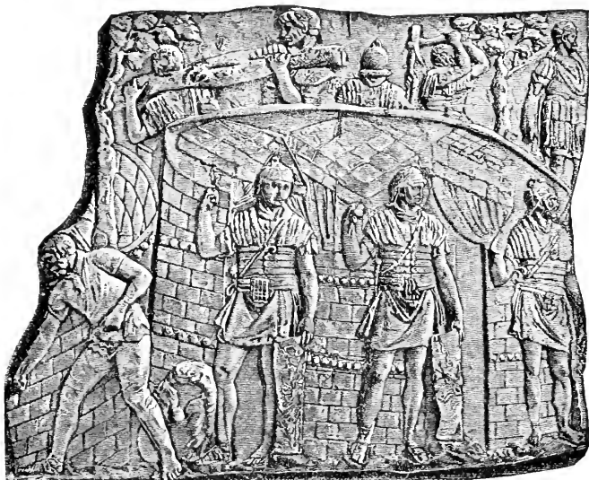
FIG. 69. — SOLDIERS BUILDING CAMP, WITH GUARDS.
