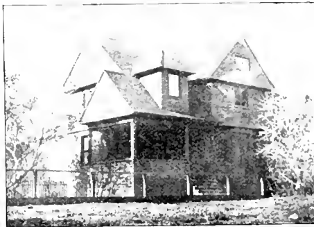
House of A. W. Pooley, Millwood, Cal., H. A. Klyce, Architect, Eastland.
