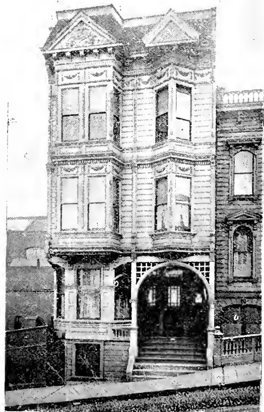
Three Flats, Six and Seven Rooms, Jackson Street, near Mason. Owner, George H. Jacobs, Esq. Architect, Chas. M. Rousseau.
