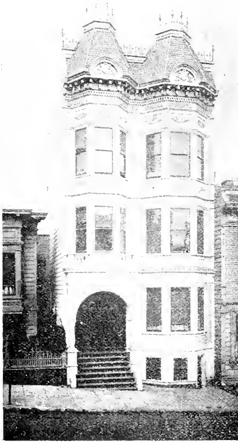
Three Flats, Six and Seven Rooms, Pine Street, near Lyon. Owner, V. C. Clark. Architect, Chas. M. Rousseau.
