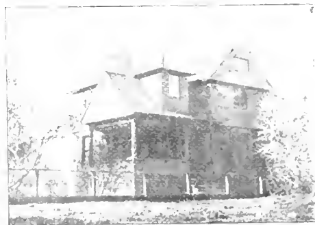
House of A. W. Pooley, Millwood, Cal., H. A. Klyce, Architect, Eastland.
