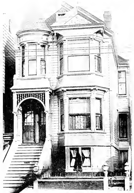
Two Flats, Six and Seven Rooms, 510 Devisadero St., P. ROTHERMEL, Esq., Owner.
