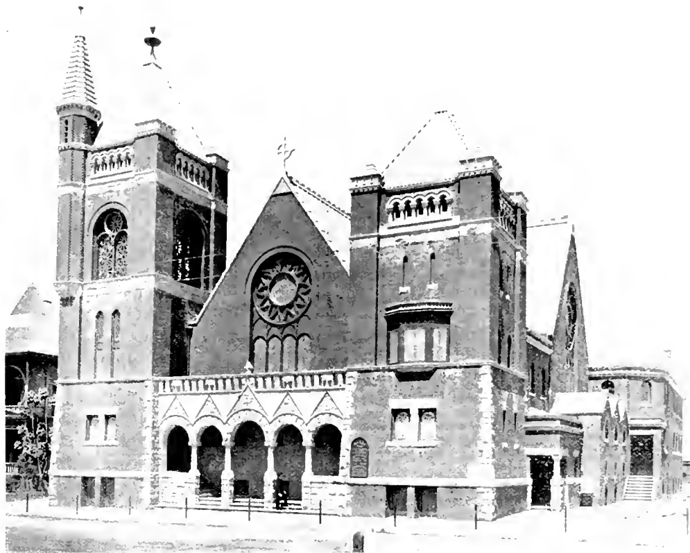
FIRST BAPTIST CHURCH, LOS ANGELES—HEATED BY THE MORGAN HEATING COMPANY
