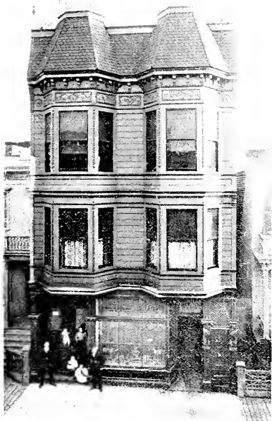
Store and Two Flats, Five and Six Rooms, Silver Street, between Third and Fourth. Chas. M. Rousseau, Architect. Owner, Mrs. Emilie Festu.
