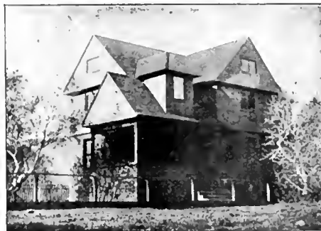
House of A. W. Pooley, Millwood, Cal., H. A. Klyce, Architect, Eastland.
