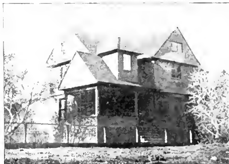
House of A. W. Pooley, Millwood, Cal., H. A. Klyce, Architect, Eastland.
