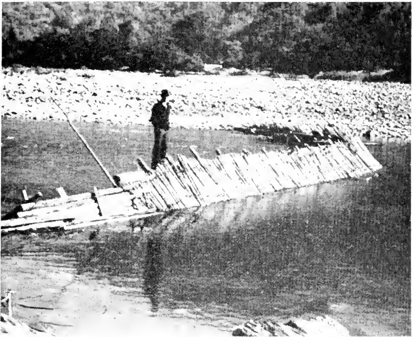
Fig. 27. Indian Weir at Hoopah on the Trinity River. While in operation, until taken out by the first heavy rains, this weir is an effective block to the early fall salmon.
