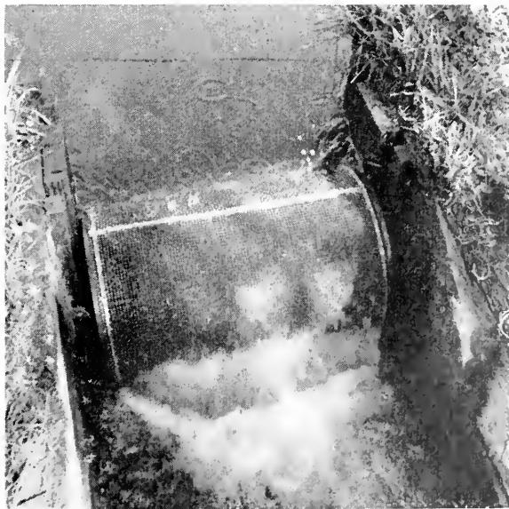
FIG. 48. The Murray fish screen in operation.
