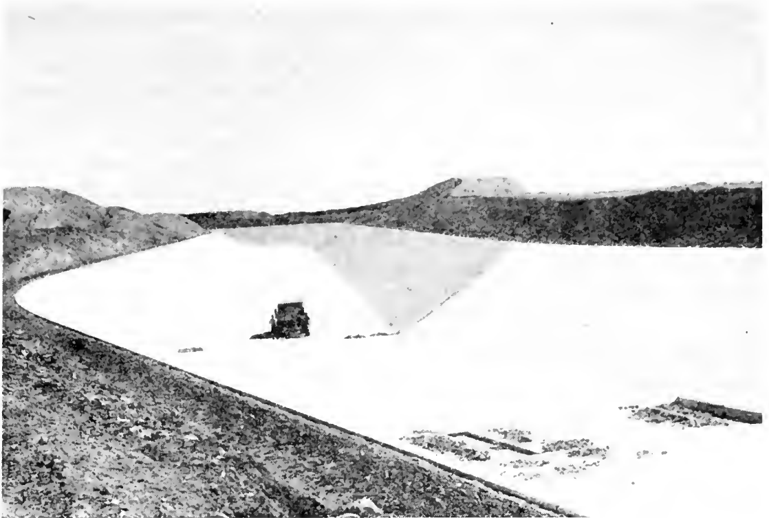
FIGURE 74. Completed section of the Delta-Mendota Canal near its intersection with Highway 50
