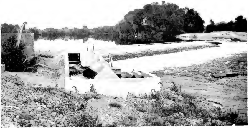
FIGURE 4. The new fishway at Sutter Butte dam on the Feather River. Photograph by J. A. Aplin, July, 1952.
