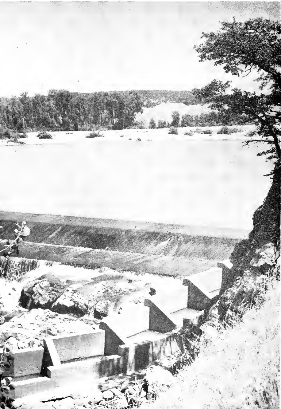
FIGURE 3. Fishway at the north end of the Daguerre Point dam. Photograph by J. A. Aplin, July, 1952.
