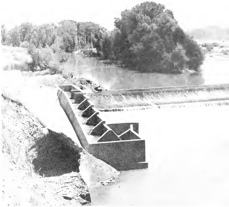
FIGURE 2. The new ladder at the south end of the Daguerre Point dam
