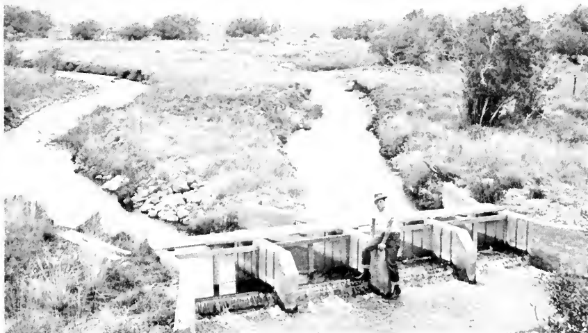
FIGURE 4. Lower water control and screen structure, showing terminal portions of Sections 3 and 4 and discharge of flow into the main stream. Photograph by E. Philip Pister, September, 1950.
