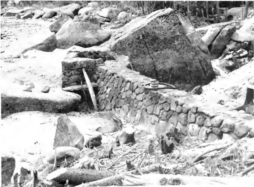
FIGURE 17. Right wing of flow maintenance dam at Stony Ridge Lake, El Dorado County. Note outlet box in left center of photograph, at end of dam, to regulate flow in stream below dam.
