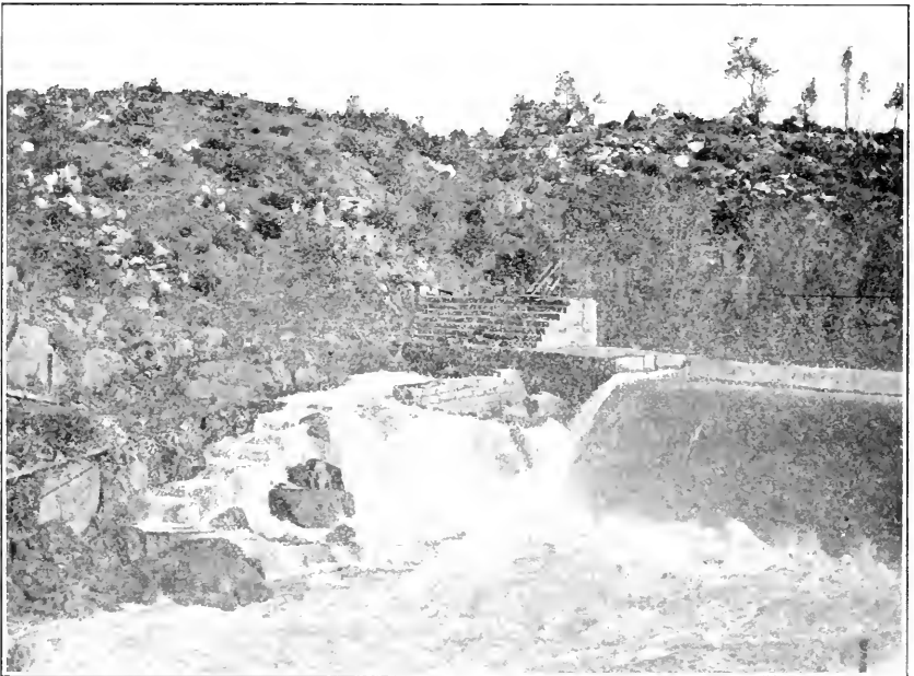
FISHWAY AT FOLSOM DAM, AMERICAN RIVER.
