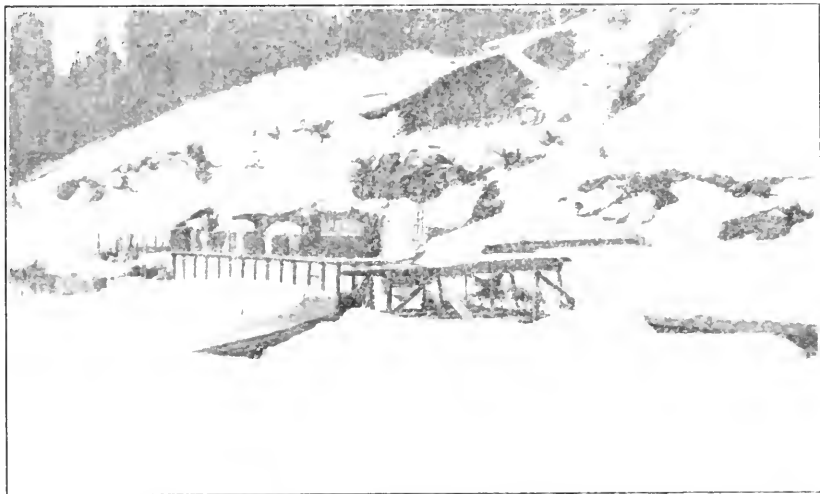
FIG. 10. Eyeing house and tank at Canyon Dam, Lake Almanor, Plumas County, April, 1919. Spawning operations must be begun under such conditions as these. Photograph by S. Campbell.
