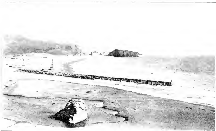
Russian river jetty—August 9, 1930. Looking south from county road, showing entire jetty, railroad and quarry.
