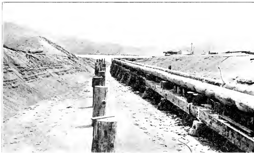
Russian river jetty—August 30, 1929. Core wall and railroad timber construction through bar.
