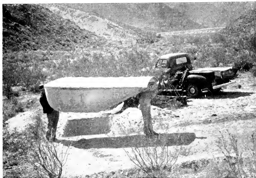
FIGURE 4. Installing one of the new type plastic gallinaceous guzzlers
