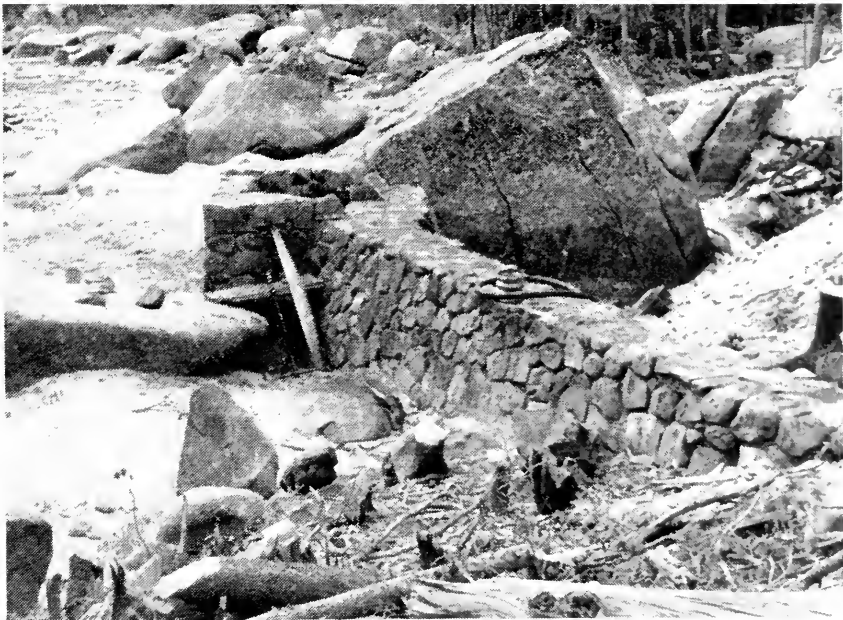
FIGURE 17. Right wing of flow maintenance dam at Stony Ridge Lake, El Dorado County. Note outlet box in left center of photograph, at end of dam, to regulate flow in stream below dam.
