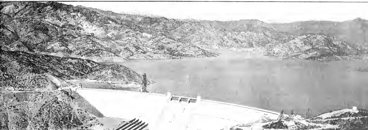
Shasta Dam, which backs up the headwaters of the Sacramento River.
