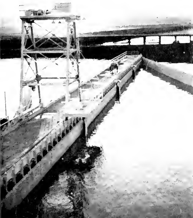
Fish screen at Tracy Pumping Plant of Delta Mendota Canal on San Joaquin River.
