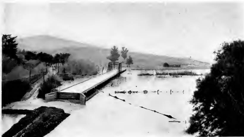
State Highway bridge near San Luis Obispo, showing flood during construction.
