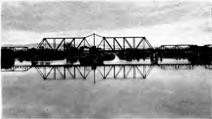
Middle River bridge on Borden Highway west of Stockton.
