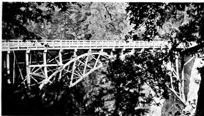
Rock Creek Bridge in Mendocino County.
