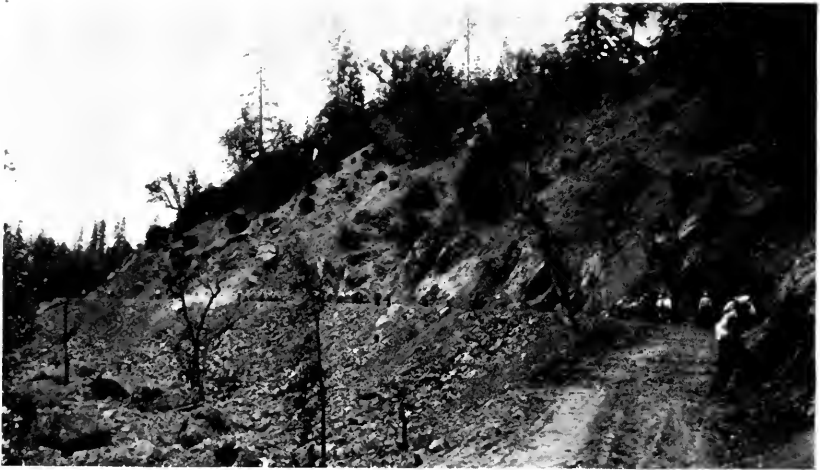
A typical convict labor scene on the California Highway system.
