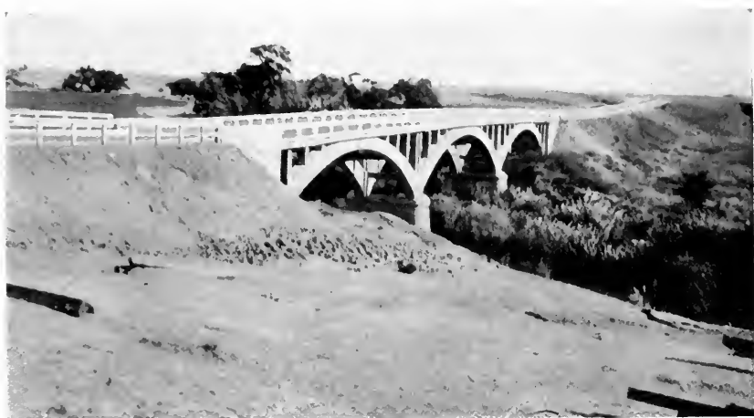
Dry Creek bridge on Stanislaus County highway system.
