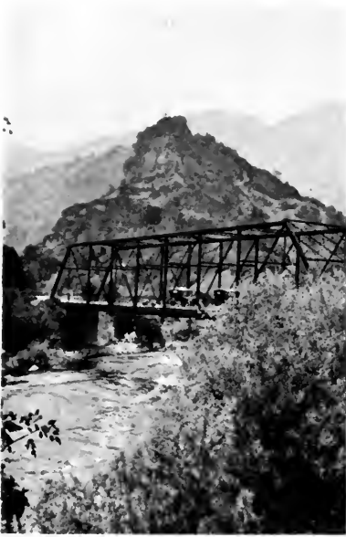
Klamath River bridge.
