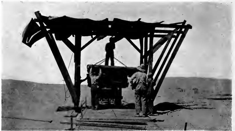
Unloading sections of plank road. Canopy protects workmen from sun.
