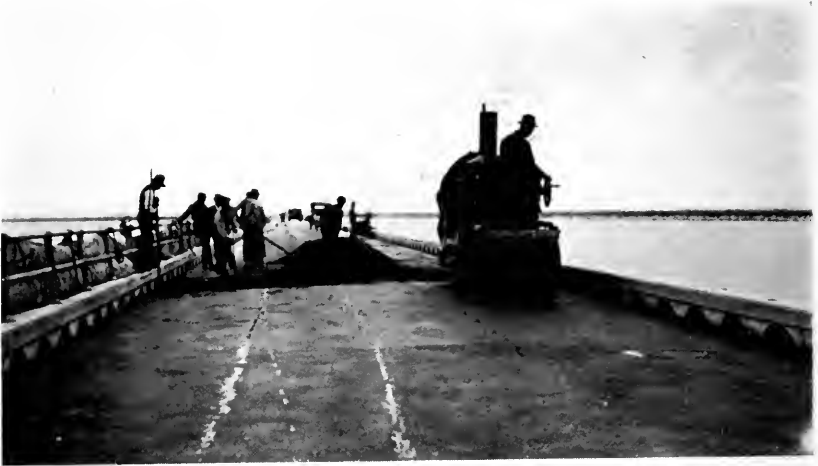
Surfacing the Yolo Causeway.
