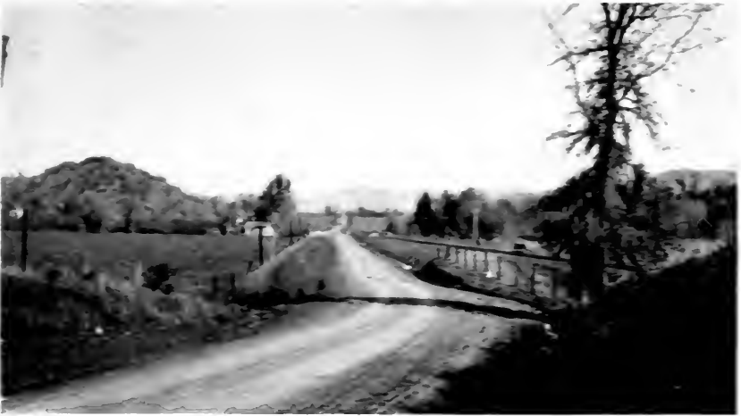
A rerouting of this State Highway line eliminated two grade crossings. Old road to right.
