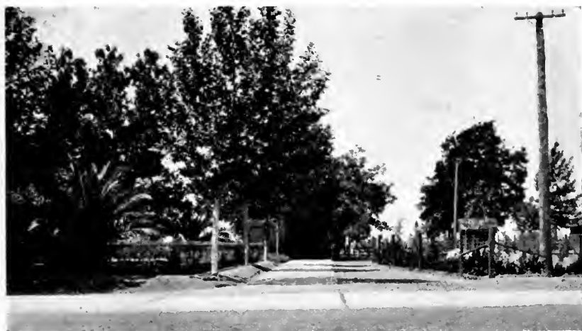
Concrete runway from county highway to a ranch garage.
