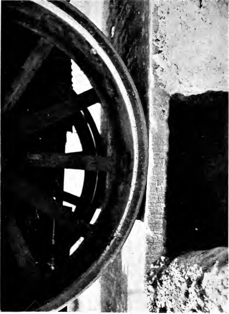
One of the early concrete road tests of the State Highway Engineers. Sixteen hundred and sixty-six pounds weight to the inch on an unsupported four inch concrete slab.
