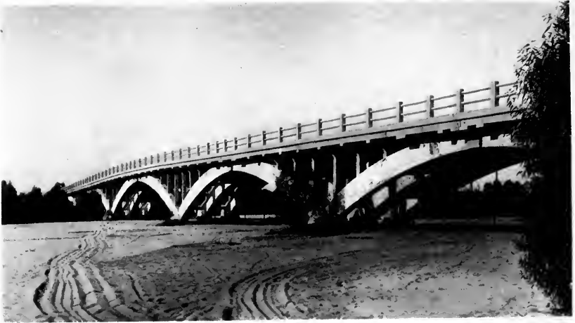
Type of bridge built by County cooperation on the State Highway in the San Joaquin Valley.
