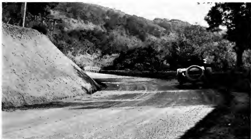
Stone wall and guard rail on Half Moon Bay Road.
