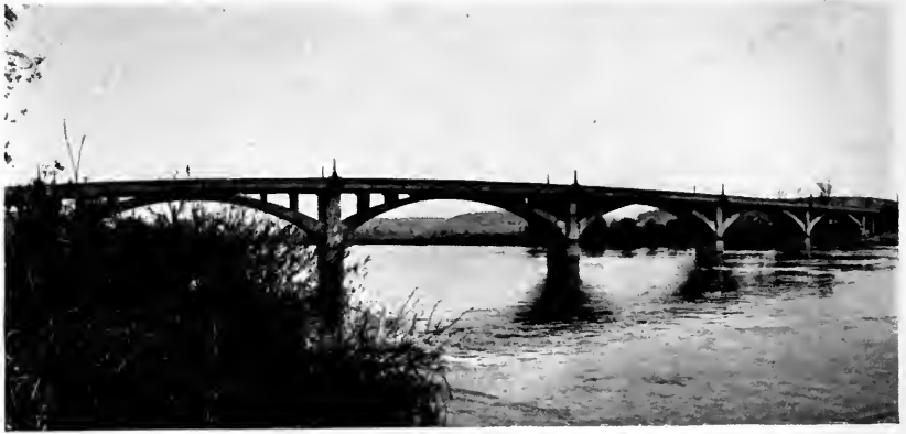
Bridge across Sacramento River at Redding.
