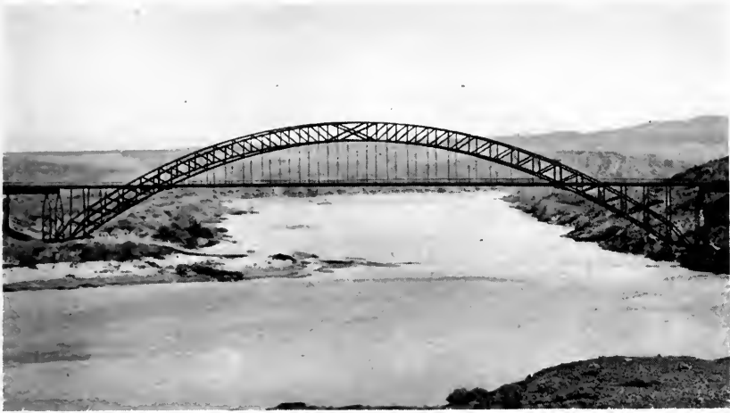
Looking down river at Colorado River bridge at Topoc, Arizona.
