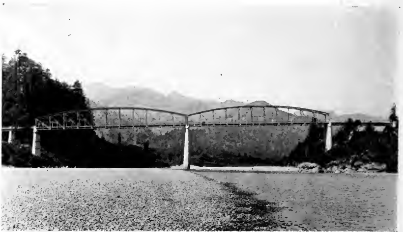
Another view of Scotia bridge. Note the automobile on right span and angler below.
