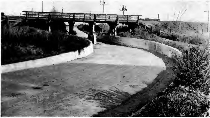
San Joaquin County's highways are built for safety. Subway on Borden Highway protected from seepage by concrete walls.
