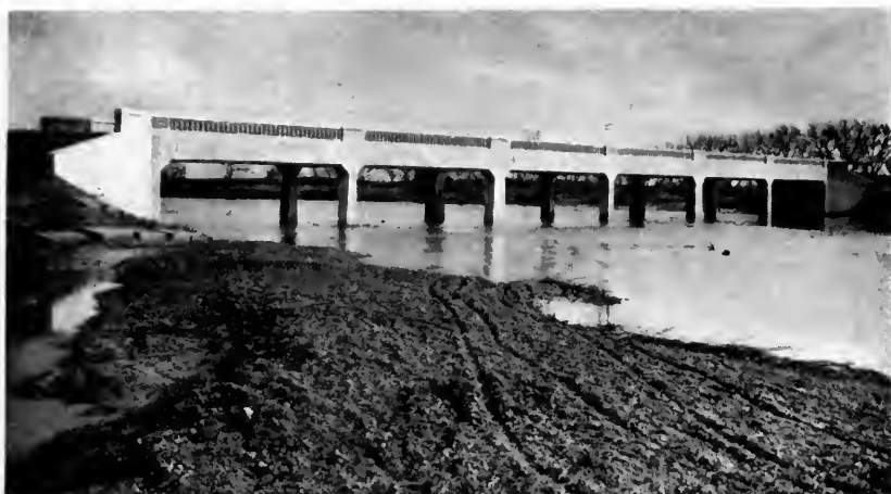
Type of concrete trestle built by Yolo County Board of Supervisors and County Engineer.
