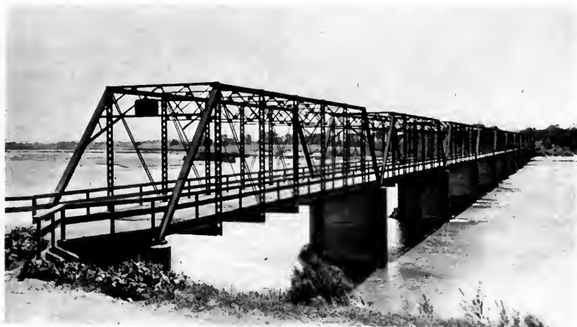
Salinas River Bridge on State Highway near Soledad, Monterey County.
