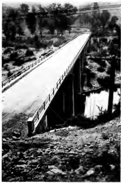
Bridge over Sacramento River.
