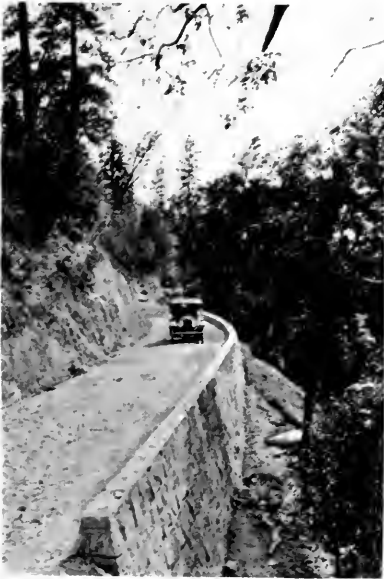
Rock wall protection on Pit River.
