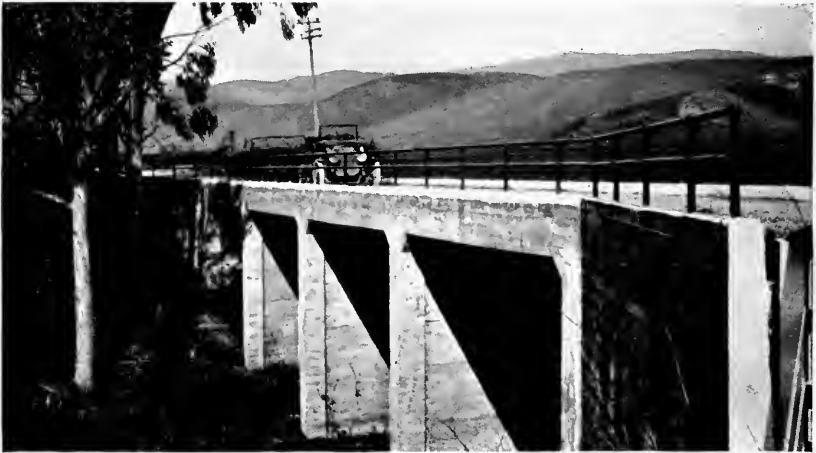
Near Half Moon Bay, showing type of guard rail used on bridges.
