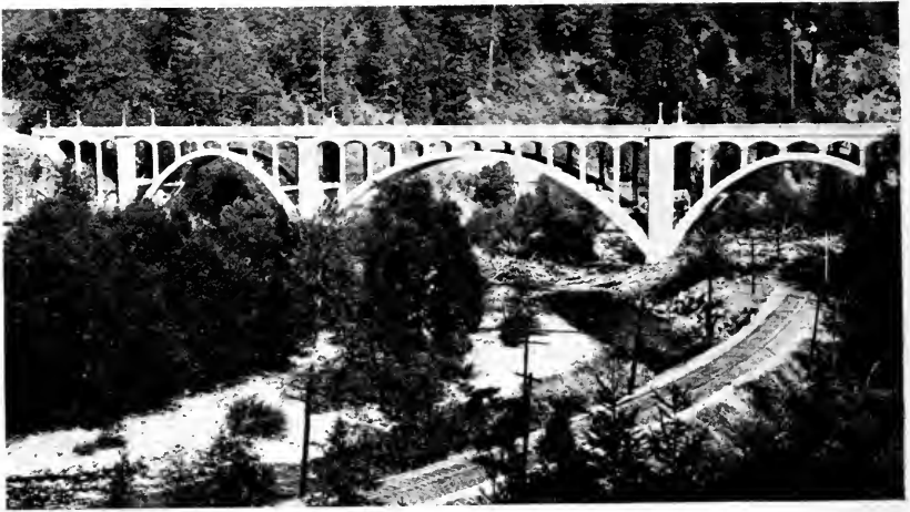
Bridge across Sacramento River at Dunsmuir.
