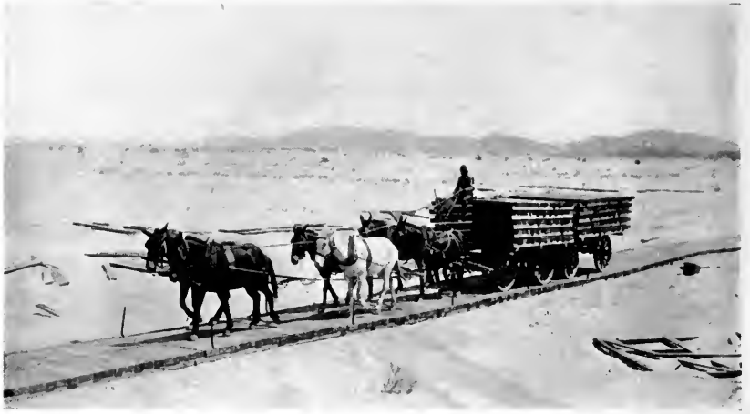
Hauling sections of plank road out into the desert on the El Centro-Yuma Highway.
