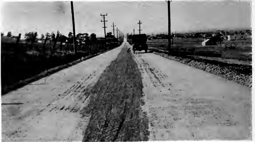
Two eight-foot slabs of concrete with four feet of oil macadam between. An experiment being tried out in Contra Costa County.
