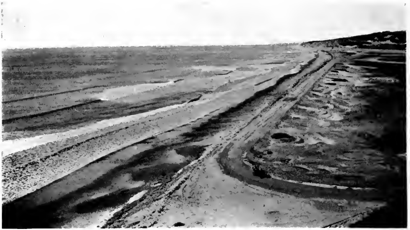
Before construction—a sandy, unkempt stretch of road.
