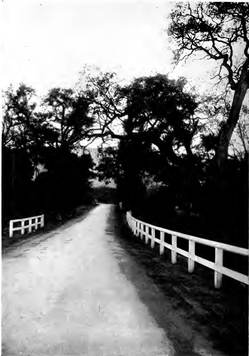
This stretch of State Highway was paved by Santa Barbara County and presented to the State.
