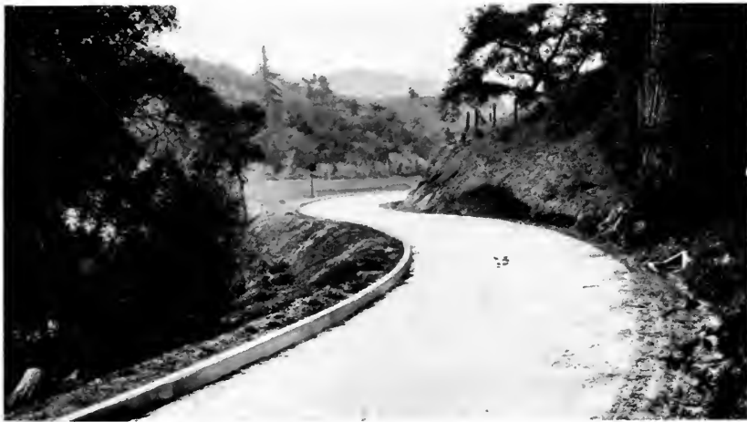
Concrete curb, in addition to preventing roadside wash, supplies a measure of safety.
