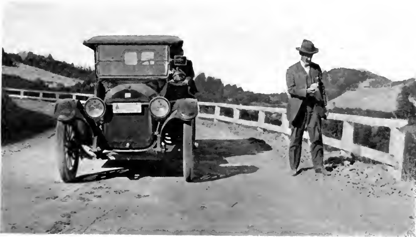
Guard rails in Division IV, and Division Engineer W. Lewis Clark.
