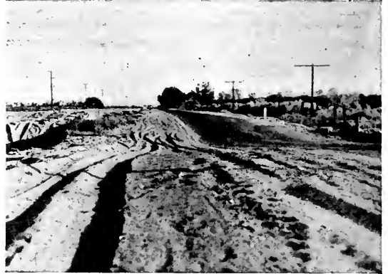
SAND SHOULDERS along the old fifteen-foot highway through Coachella Valley and dip being replaced by modern pavement.
