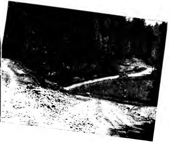
IN TALL TIMBER , this part of new mountain route involves long hauls from cuts to fills.
