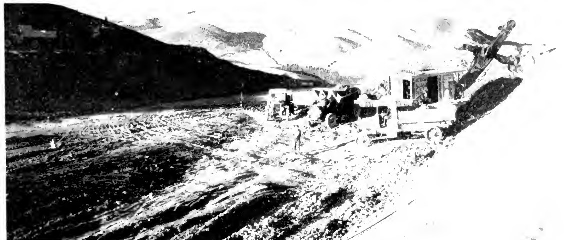
TERRACING OPERATIONS in the "Big Cut" are shown in this picture. A shovel and truck are making a 12-foot terrace along the left slope. Fills will also be terraced.
