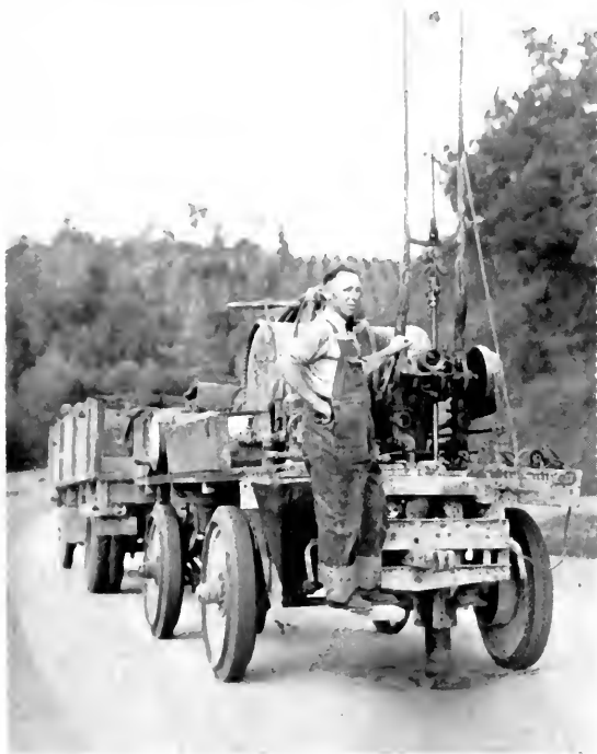
SAMPLING HIGHWAYS is the job of Art Savage. With this truck and trailer equipped with a power drill he takes pavement cores five inches in diameter for tests by State engineers.
