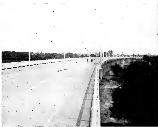
New Tuolumne River Bridge
