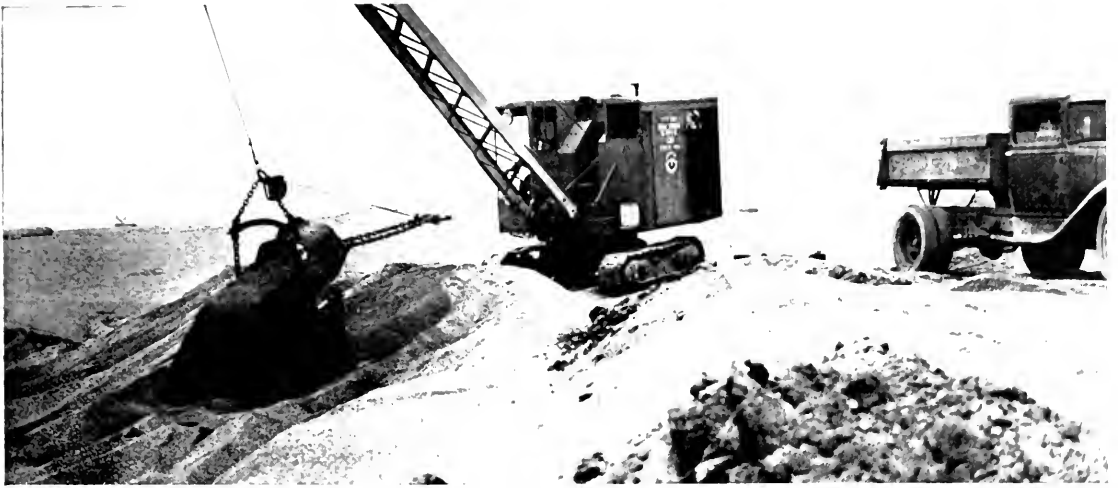
BEACH GOLD MINE this proved to be for the highway builders in Humboldt County. With no supply of aggregate available they tried beach sand for asphalt paving and it worked.
