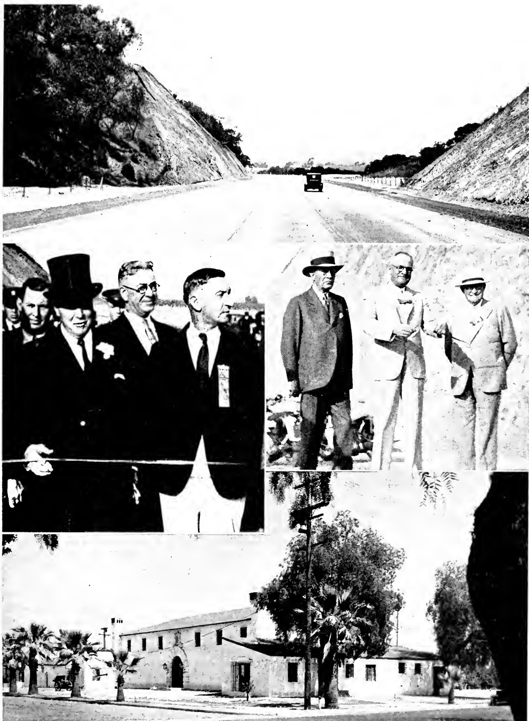
"THE TIDE HAS TURNED and these new highways are evidence of progress," declared Governor James Rolph, Jr., in dedicating two recently completed projects and an armory at Pomona July 15th. He referred to the extensions of Holt Avenue and Fifth Avenue westward from the city. At top—One of many big cuts on the Fifth Avenue extension, a link of State Highway 19. Left center—Governor Rolph cutting the Holt Avenue barrier surrounded by city and county officials. Right center—State Highway Commissioners Phillip A. Stanton at left and Frank A. Tetley at right assisting Senator Nelson T. Edwards in the official ceremony on the Fifth Avenue link. At bottom—New State Armory for Company F, California National Guard.
