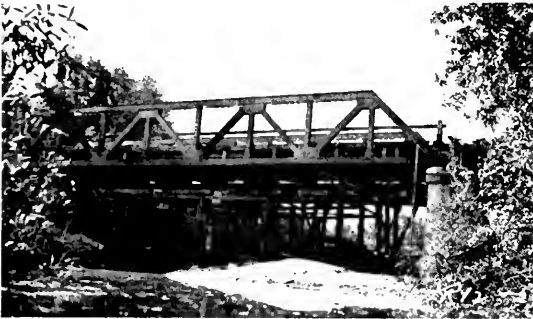
THE ICEMAN'S BRIDGE over the Russian River on Tahoe-Ukiah cut-off after being properly iced into place.
