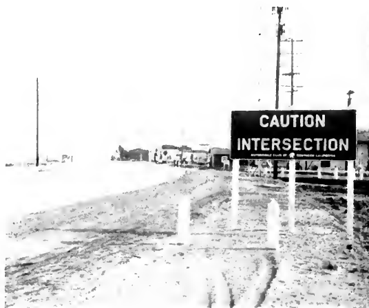
DAYLIGHT appearance of reflectorized warning sign showing method of erection.
