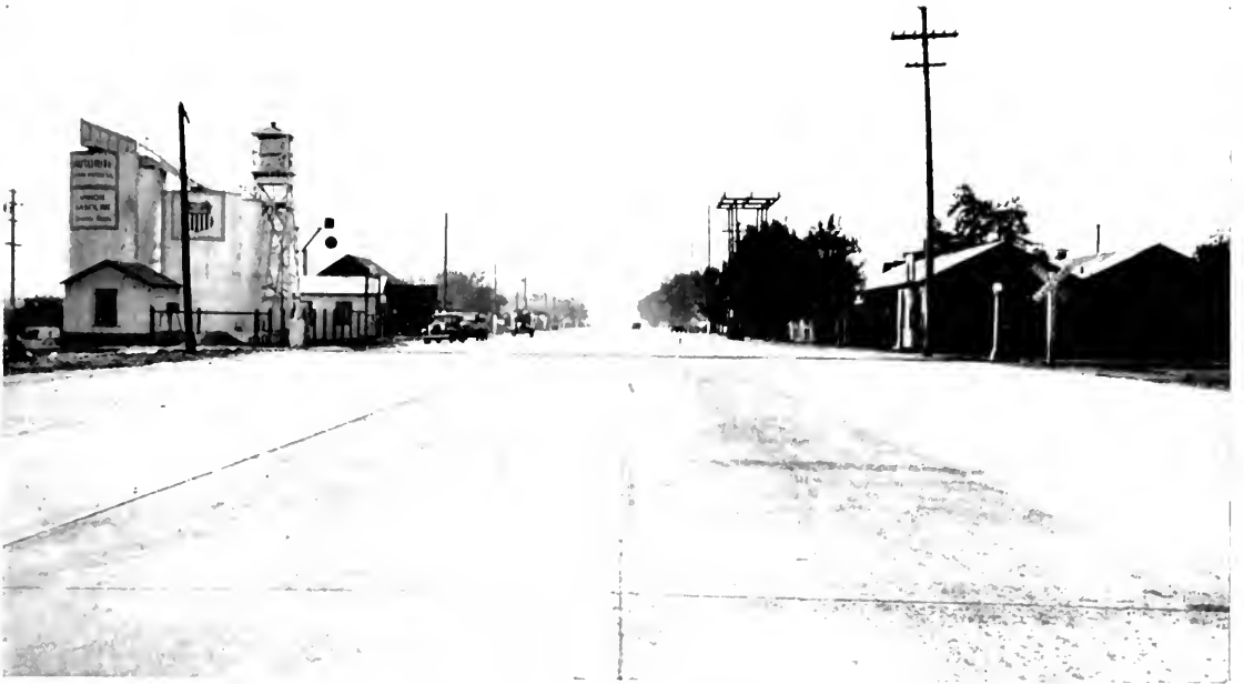
PORTLAND CEMENT CONCRETE pavement on Golden State Highway through Lodi in San Joaquin County.
