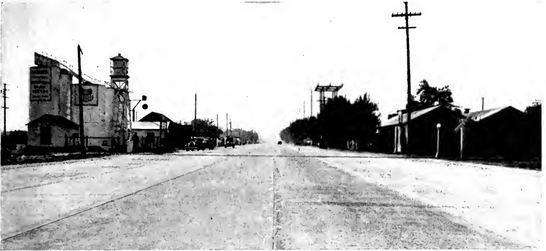
SEVENTY-SIX FEET WIDE , the new concrete pavement of the Stockton-Sacramento arterial through the city of Lodi renders traffic congestion practically impossible on this busy highway. The State paid for 40 feet of this cooperative project.
