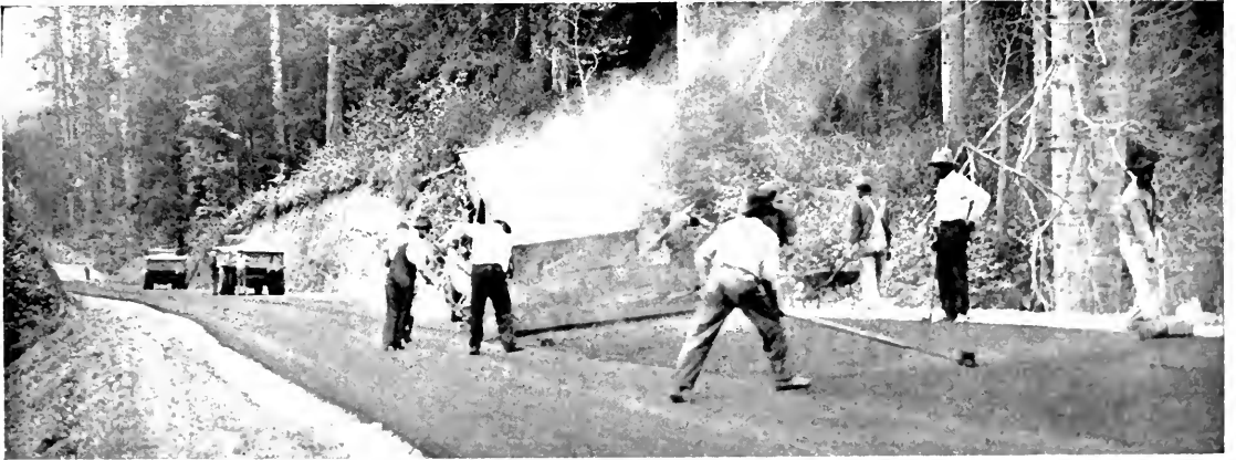
QUICK ACTION was obtained with the new mixture. A few rakers were used but the roller was able to follow close to the spreader instead of three to five hours behind as with regular mixes.
