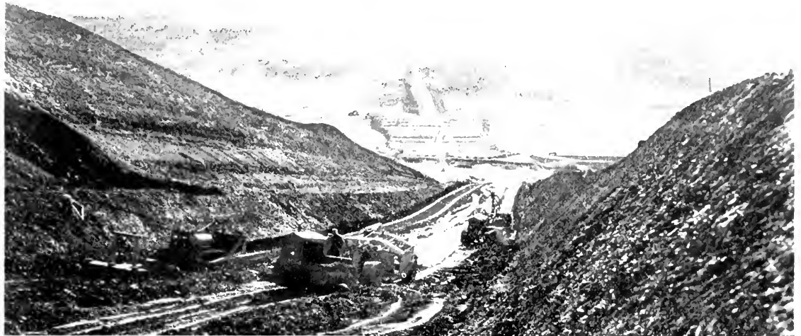
"BIG FILL," adjacent to the "Big Cut," is 2500 feet long, with a maximum height of 75 feet, requiring 605,600 cubic yards of material.
