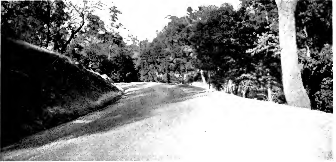
ONE HUNDRED PER CENT right is this "California Type" highway—hard, smooth and durable with low initial cost. The picture shows a primary road of proper oil mix construction in Tehama County.
