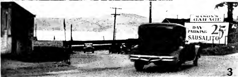
Nos. 3-4—The terminal stretch of the Redwood Highway approaching the ferries in Sausalito is a narrow two-lane way abounding in right angle turns, each a danger point because of greatly restricted vision. Two of these are shown in picture No. 3 while No. 4 shows how a truck and trailer can hold up the whole parade.
