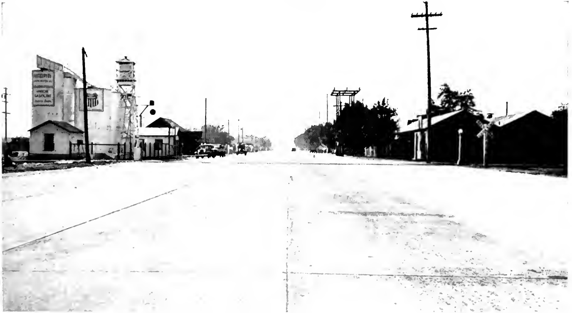
AFTER the cooperative improvement was finished, this view, taken in September, 1931, at the same point, looking south from the north end of the project, shows the broad new concrete pavement, 76 feet wide over which traffic flows through the city without congestion.
