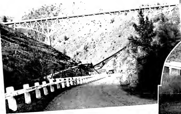
Viaduc Crossing or Shasta Bridge No. 2 300 feet above canyon floor - 200 feet long - 6 miles north of Yreka.
