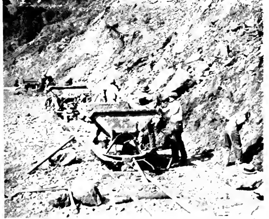
HEAVY ROCK WORK was also done by the men of the Needles camp on southern California roads.
