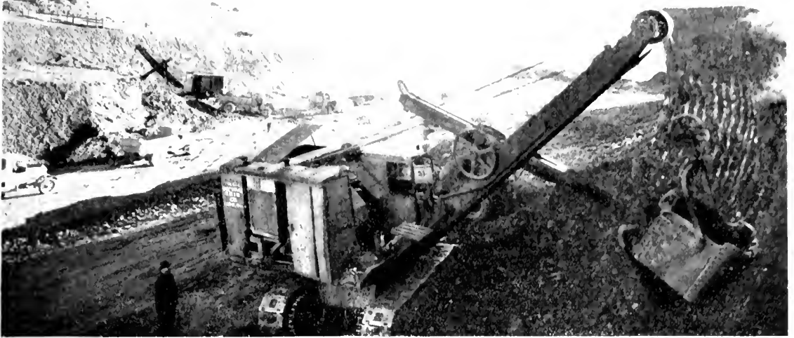
"BIG CUT" of the American Canyon cut-off project where a total of 520,500 cubic yards will be moved. The cut is 2400 feet long with 130-foot maximum depth.
