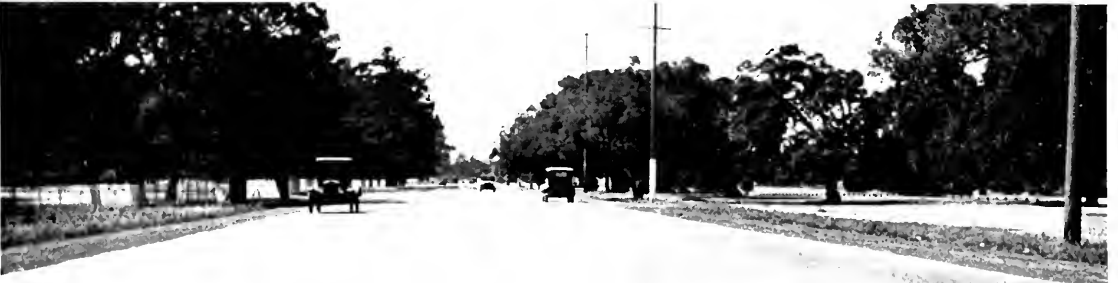
NO WRINKLES or rough places are to be found in this fine forty-foot asphalt concrete pavement laid in Santa Clara County under superior mix formulas and finishing methods developed in the Public Works laboratory.
