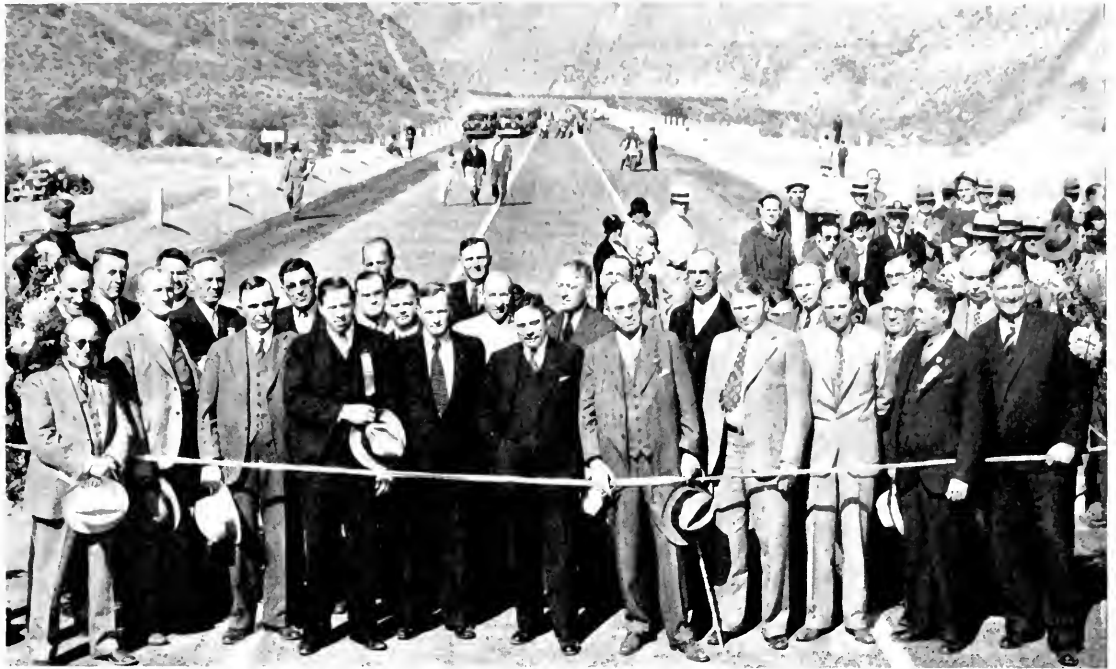
OFFICIAL GROUP at Ridge Alternate ceremonies: (left to right) Secretary Howe, Highway Commission; Asst. State Highway Engineer McCoy; Acting Dist. Engineer Gillis; Dist. Engineer Cortelyou; Asst. Resident Engineer Telford; Chief Engineer East Auto Club of So. Calif.; Supervisors Mitchell, Orange and Brito of Kern; Asst. Dep. Director Public Works Keaton; Contractor N. F. Jahn; Secretary Nourse, Kern Chamber of Commerce; Resident Engineer Templeton; Assemblyman Rogers, Los Angeles; Wm. Shoemaker, Orange; Col. A. Marks, Taft; Chairman Hopkins; C. C. Carlton, State Rights of Way Chief; Acting Dist. Const'n Engineer George; Highway Commissioner Stanton; Nat Neff, Orange County Engineer; President Loudon, Economic Council, So. Calif.; Secretary Brashear, L. A. Chamber of Commerce; Carl Mock, Santa Ana Chamber; City Manager Nighbert, Bakersfield; Editor McCracken, Anaheim; Supervisor Wimmer, Kern County; President Simpson, L. A. Chamber of Commerce; Supervisor Quinn, Los Angeles County.
