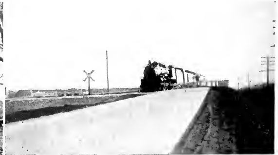
BAD SPOT , this was, where highway crossed the tracks at a severe skew, impairing visibility, augmenting danger.
