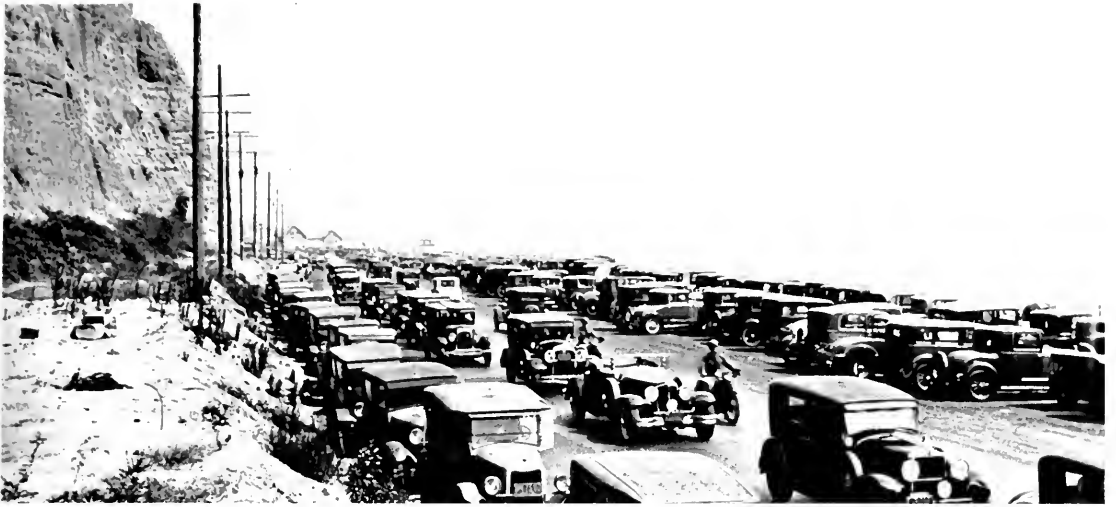
GREATEST TRAFFIC DENSITY in the State is recorded for this section of the Coast Highway west of Santa Monica Canyon where 53,303 vehicles passed in a 16-hour period. The roadway will be graded to a width of 80 feet.
