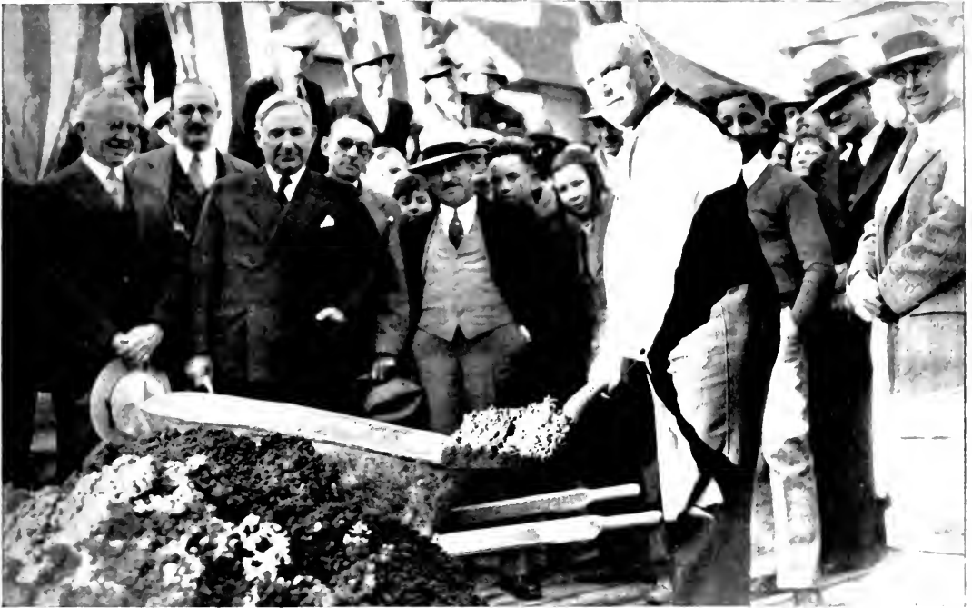
WIELDS A WICKED SHOVEL. —Governor Rolph is becoming an expert in dirt digging through officiating at ground-breaking ceremonies. During the past month he participated in four such events in various parts of the State where the Architectural Division of the Department of Public Works has building projects under way. The above picture shows the Governor turning up the earth for an annex to the State Printing Plant at Sacramento. The bareheaded man in the center of the group is Director of Public Works Colonel Walter E. Garrison. Deputy Director James I. Herz is on the right and on the left is Superintendent J. M. Welsh of the Printing Plant.
