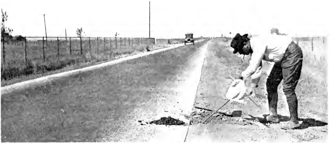
TAKING SAMPLES of soil from beneath existing pavement with a soil auger in 1923. The sample was taken in the white bag to the laboratory. Improved methods now prevail.
