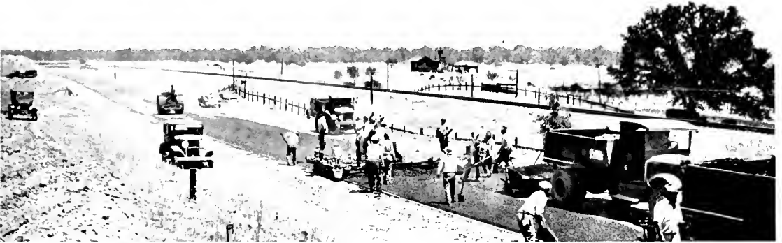
LIKE A CARPET this big gang laid a broad strip of asphalt concrete pavement in San Luis Obispo County in record time by employing more efficient methods developed by State experts.
