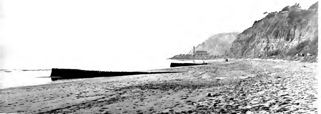
HARNESSING OLD OCEAN , compelling it to work in building up beach by use of groynes or bulkheads, this view shows results obtained on Santa Monica coast. Note tops of groynes nearly submerged by newly deposited sand.
