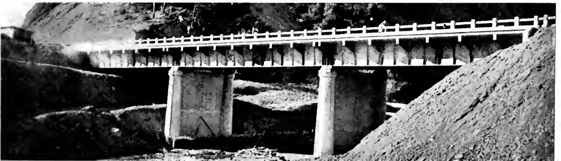
OLD GIRDERS TURNED UPSIDE DOWN AT LOS ALAMOS CREEK WITH NEW WIDE ROADWAY
