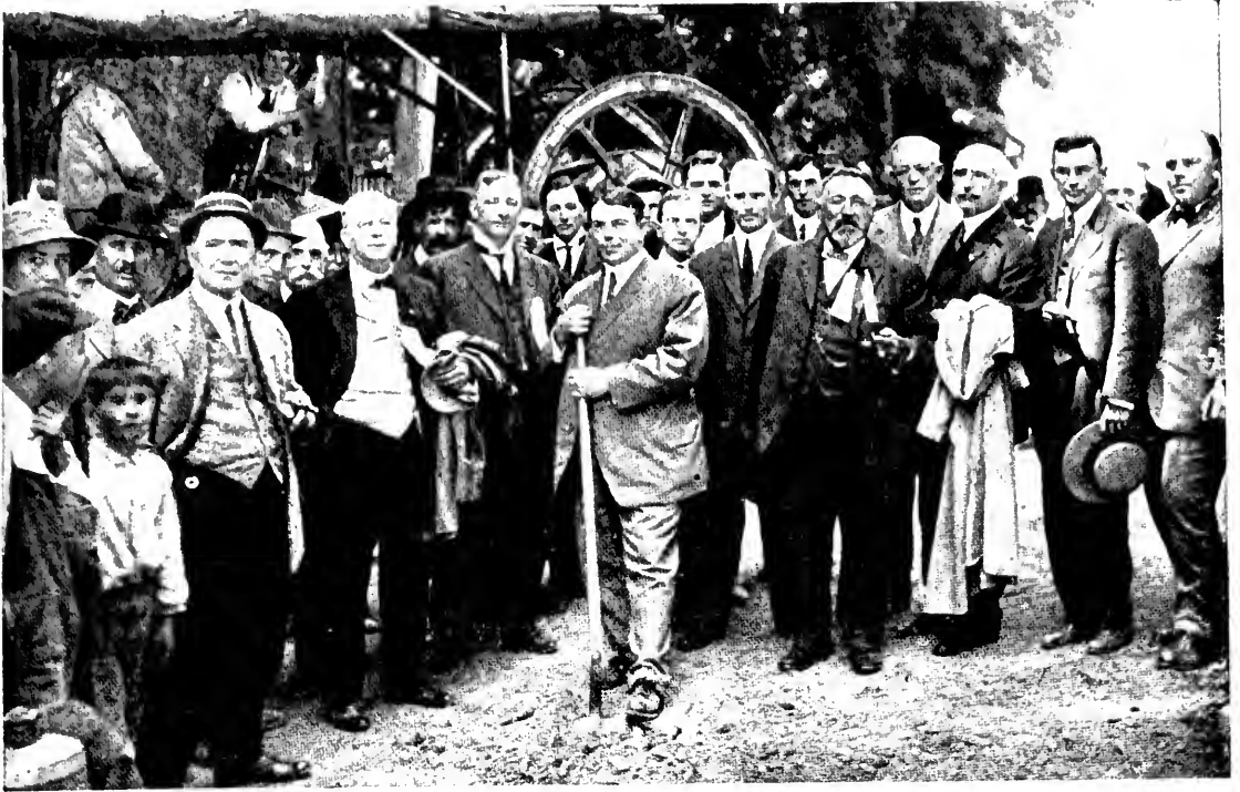
TWENTY YEARS AGO on August 7, 1912. Chairman Burton A. Towne of the first California Highway Commission turned the first shovelful of earth on the first State highway contract. The scene is reproduced from the book "California Highways" by Ben Blow, field secretary of the National Automobile Club.
