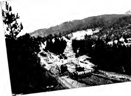
SPEEDY WORK being done in moving vast quantities of earth on highway relocation near Gold Run hydraulic diggings.
