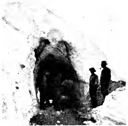
VOLUNTEER WORKERS at mouth of tunnel.
