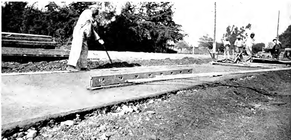
Sixteen foot one-man finishing float on P. C. C. pavement.
