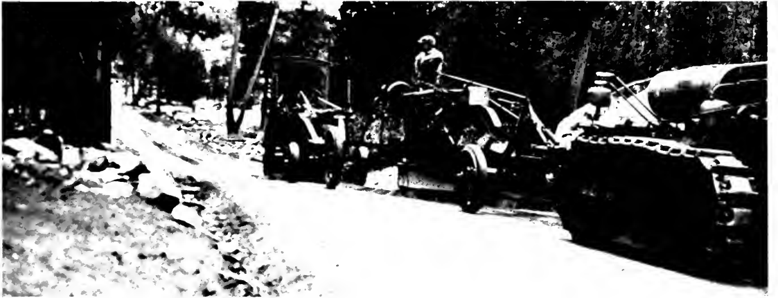
MODERN OUTFITS of the Division of Highways composed of tractor and grader team up in the preparatory work of leveling the road for the oil treatment and covering and mixing the oiled surface material.
