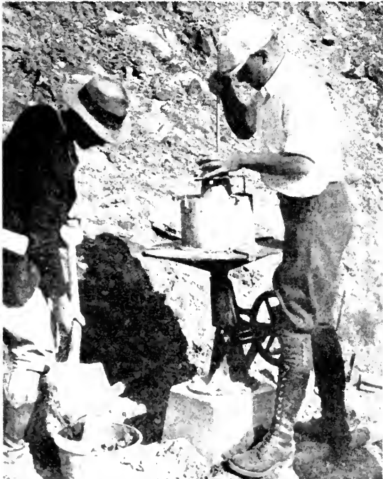
Making workability tests during construction
