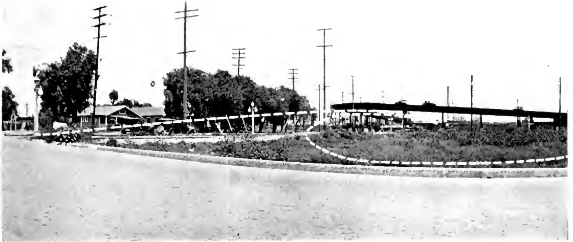
A DANGEROUS KINK or right angle turn in the narrow old viaduct carrying the State Highway over the Santa Fe yards at Mount Vernon Avenue in the city of San Bernardino has been the cause of traffic fatalities. The above view shows the existing crooked viaduct which will be replaced by a wider modern structure on an alignment indicated by the white dotted line.
