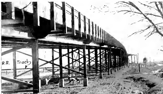
A LONG JUMP is made by this unique, welded steel viaduct carrying the highway over the railroad tracks east of Merced.
