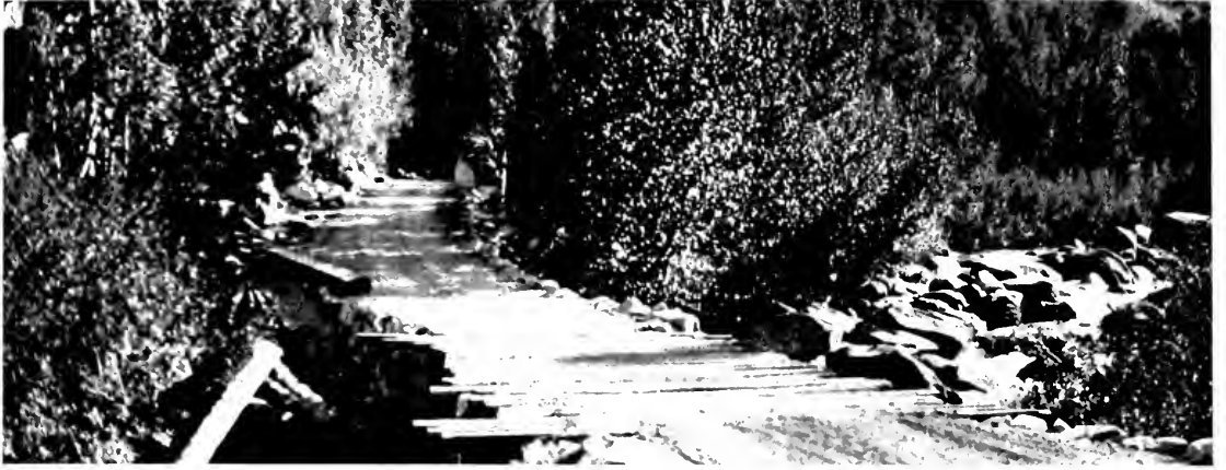
HISTORIC COUNTRY is traversed by the Kit Carson Trail, famous old route over the Sierra. Eighty miles of it will be oil surfaced through scenic countryside like this along the Carson River in Alpine County.
