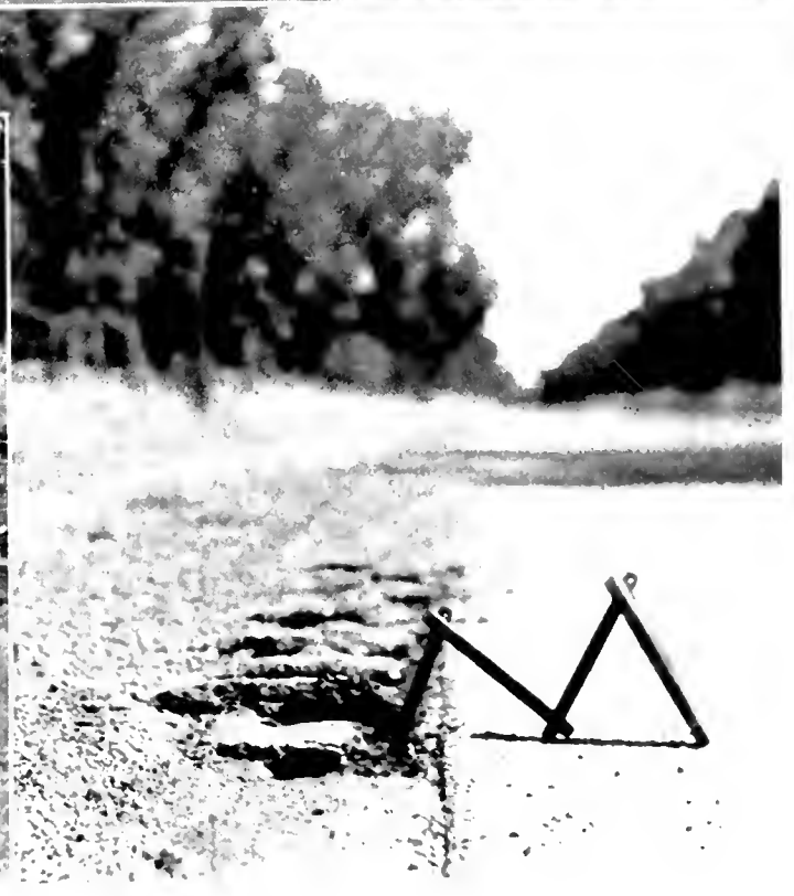
RAVAGES OF A TRACTOR. Upper left—Route 50 between Madison and Brooks, Yolo County. Caterpillar tractor and flanged heavy wheels have torn out and loosened edge of oil mixed pavement. Upper right—Route 50, between Madison and Brooks showing deep cut caused by flange of heavy wheel in bituminous macadam pavement. Lower left—Route 50, between Madison and Brooks where tractor and harvester pulled diagonally across at railroad crossing West of Capay leaving ravelled out track about 14 inches wide. Lower right—Route 50, Yolo County, armor type or bituminous pavement between Brooks and Codannassa approximately 1\frac{1}{2} inches thick where sharp flange of harvester wheel cut off edge of pavement.
