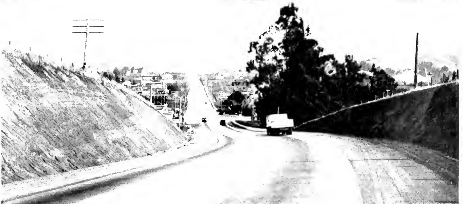
STRAIGHT THROUGH THE HILLS runs the new, shorter Dublin Canyon Boulevard on a high standard of alignment with a minimum of curves and a maximum of sight distance and 6 per cent grade. No. 1—General view of three-lane highway through central part of canyon showing elimination of many curves. Nos. 2 and 3—Comparative views of new and old highway taken at same location. Below—The broad curve on Castro Hill with three lanes widening to four-lane 40-foot pavement.
