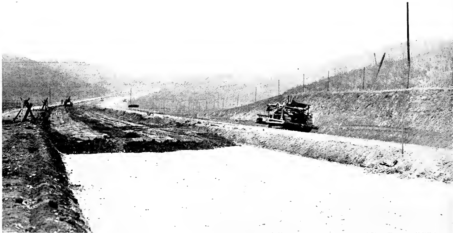
PLACING SELECT MATERIAL over oiled subgrade in Los Angeles County.
