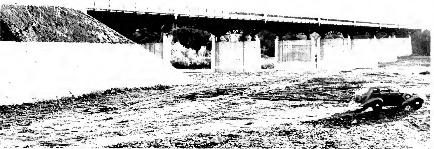
RIVER VIEW of the new steel girder type bridge consisting of six 108-foot continuous plate girder spans and two 45-foot cantilever end spans on concrete piers.
