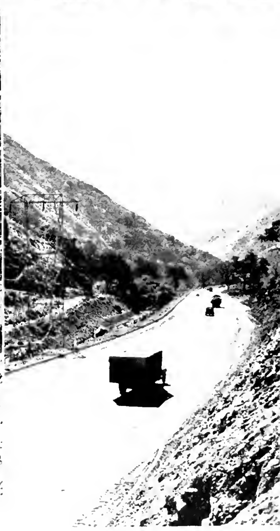
NO "DEATH CURVES" HERE. Views of the completed 3½ mile improvement of the northern section of the famous Ridge Route show that the former dangerous curves and narrow roadway have been replaced by a fine, safe three-lane modern highway. This canyon, which is the main pass between Los Angeles and the San Joaquin Valley, carries not only the State Highway, but also transmission lines of two power companies, three gas pipelines from Kettleman Hills to Los Angeles and pipelines of two large oil companies. All these utilities had to be constructed and rearranged to avoid interference with the new highway.
