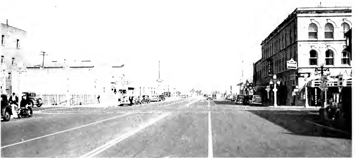
THROUGH CITY OF COLTON , the State Highway follows I street, which has recently been widened to provide four traffic lanes in addition to an ample strip for parallel parking.
