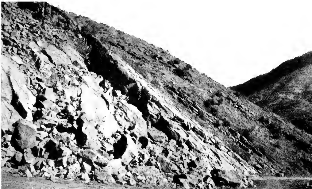
2000 YARD ROCK SLIDE on State Route 138 in Ventura County.
