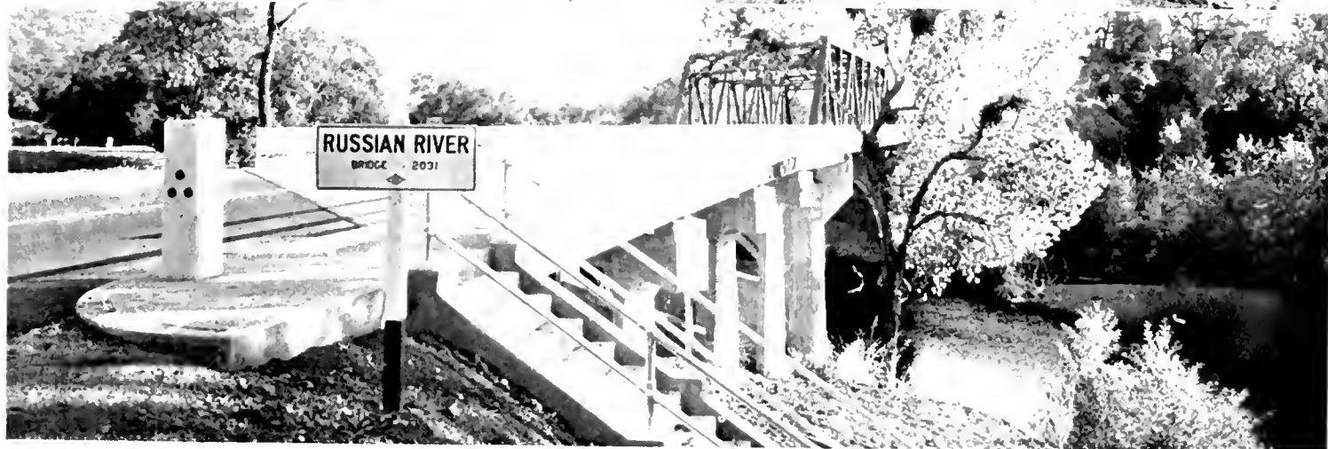
SOME BRIDGES BUILT IN BIENNIUM —At top, 500-foot bridge with 150-foot concrete arch across west branch of Feather River on State Highway 21. Below, 2050-foot steel girder and concrete head, a concrete rigid frame structure on State Route 26. At bottom, a 150-foot steel truss structure across the Russian River on the Redwood Highway near Preston in Sonoma County.
