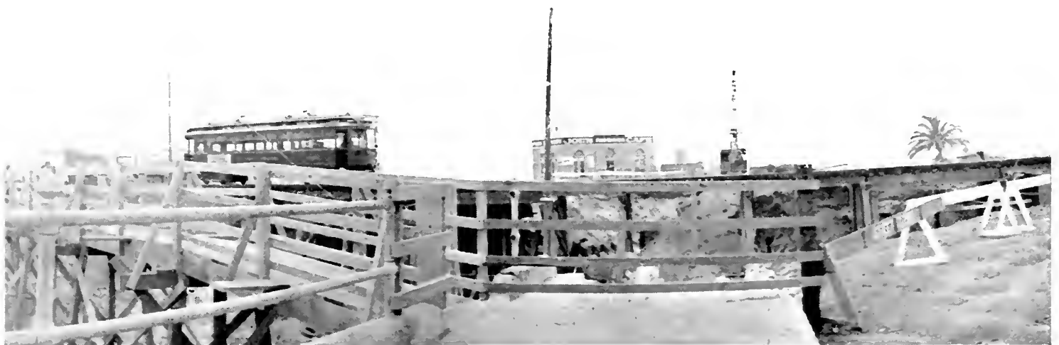
TEMPORARY TRESTLES for pedestrians and trolley cars are provided for the traffic on Ocean Avenue and to numerous beach resorts, especially heavy on weekends and holidays.
