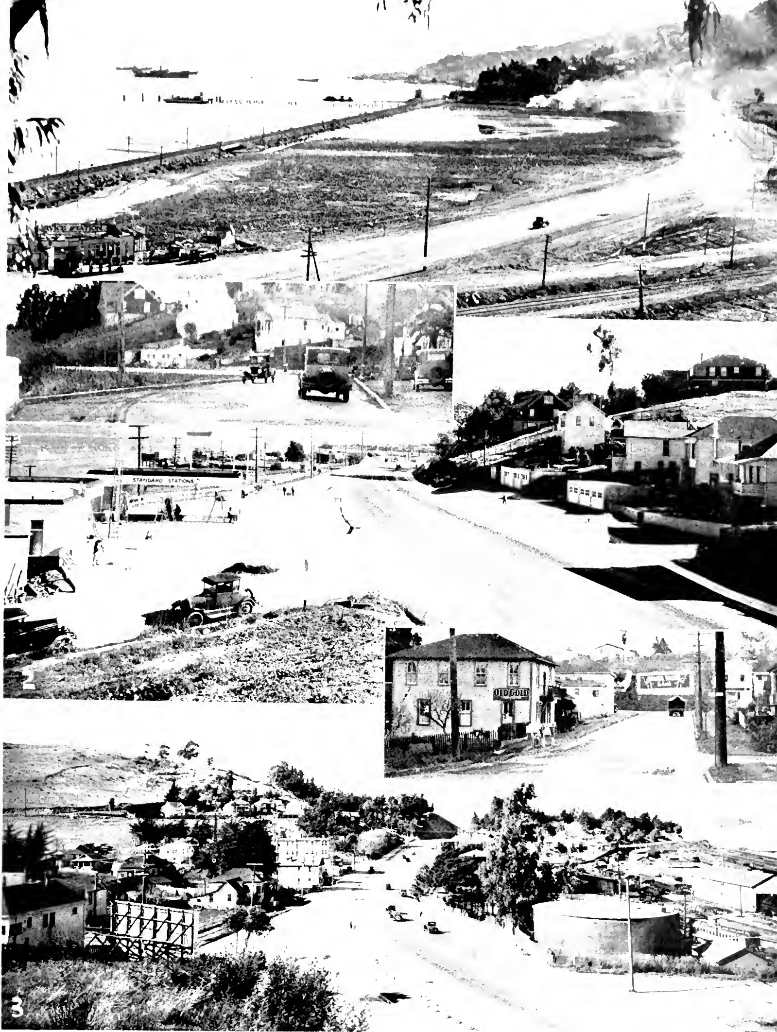
THE SAUSALITO BOTTLENECK terminal of the Redwood highway is just a bad memory. Four-lane modern roadways have replaced narrow winding streets. No. 1—New construction across tidal flats of Richardson Bay near Waldo Point. No. 2—Typical improvement on Bolinas Street. Inset shows former condition. No. 3—Reconstruction at junction of Bonita and Filbert streets. All buildings on left side of road were removed and highway was cut through hills.
