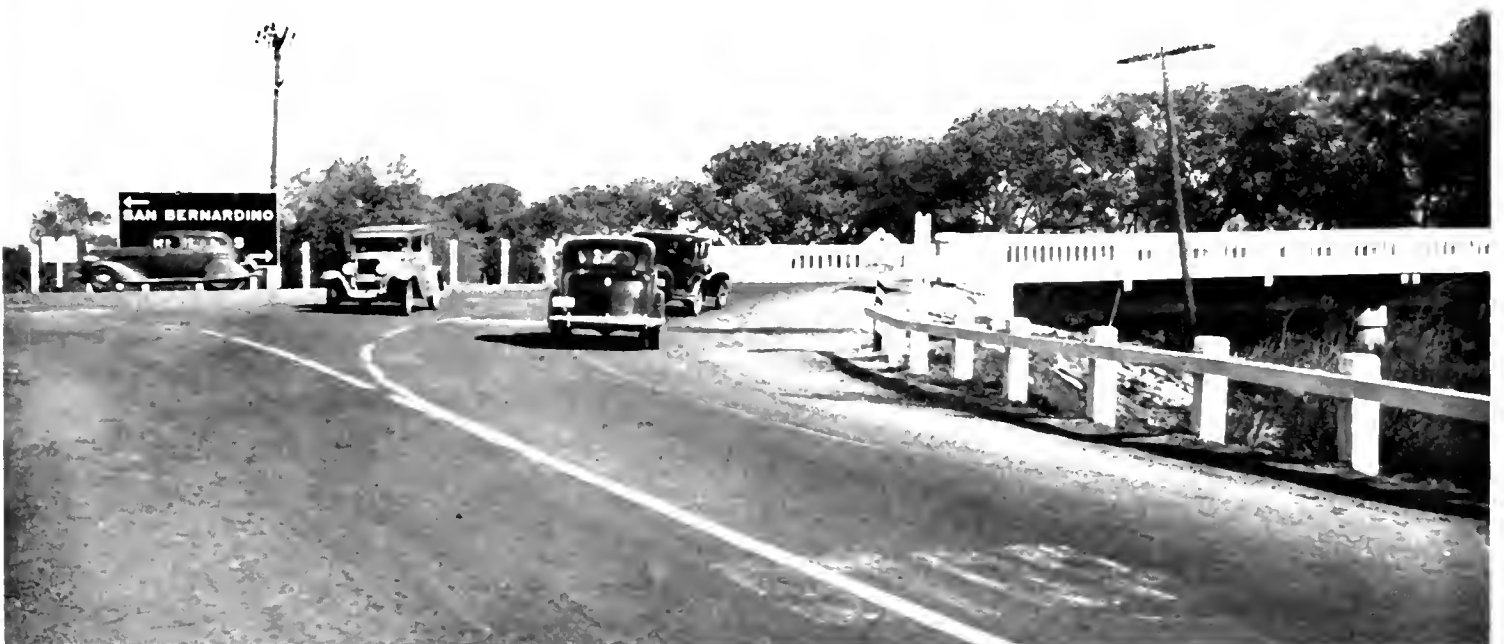
ANOTHER SAFETY FEATURE of the Redlands-Colton relocation will be elimination of this sharp turn at the north end of Santa Ana River bridge, leaving a straight approach for traffic from San Bernardino.
