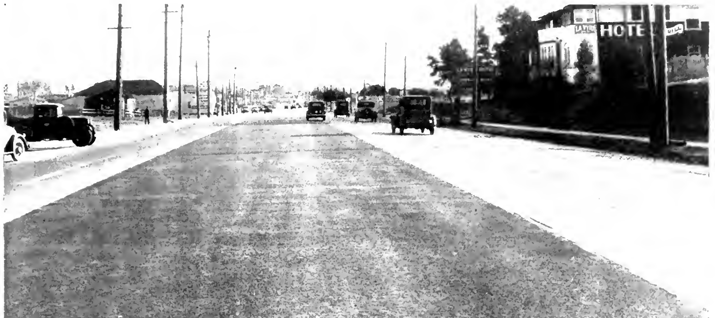
FINISHED PRODUCT presents a 74-foot pavement adding two broad lanes for motor vehicle traffic.
