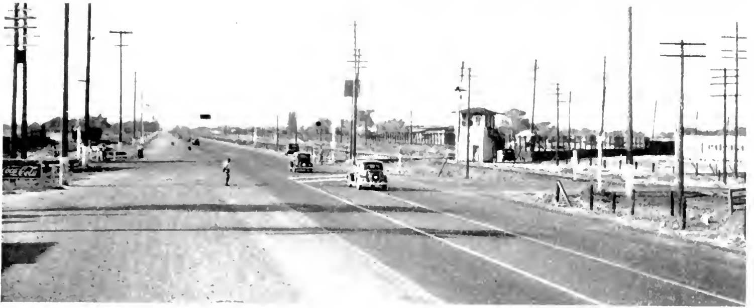
A DOUBLE DANGER is encountered at Calwa where the Santa Fe railroad crosses the Golden State highway and the Southern Pacific tracks at grade. An overhead structure will be provided for motor vehicles.
