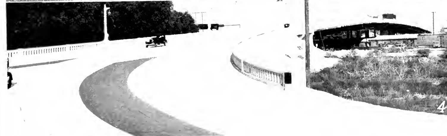
SOME STATE BRIDGES BUILT IN LAST BIENNIUM. No. 1. Prize winning Eel River bridge at Smith Point on Redwood Highway. No. 2. Dolan Creek Timber Arch structure on Carmel-San Simeon Highway. No. 3. Eureka Way overhead in Redding. No. 4. Vernon Avenue overhead in San Bernardino.
