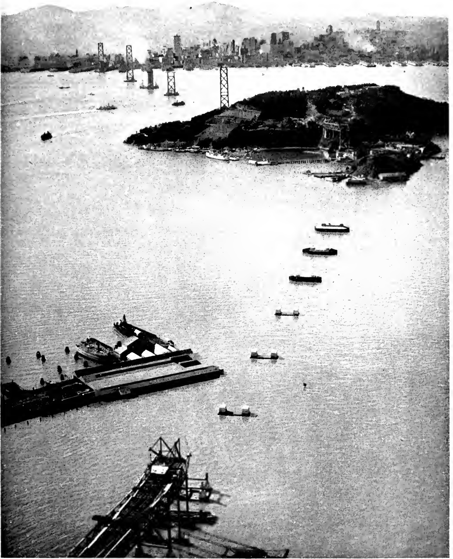
"STEPPING STONES" for the World's greatest bridge. In the foreground are seen the pier foundations for the East Bay crossing extending to Yerba Buena Island with a view of a traveling derrick erecting the last of the 288 foot spans of the Oakland shore superstructure. Erection of span YB-1 on Yerba Buena Island is in progress and beyond the island is seen the entire West Bay Crossing, with Tower W-5 under construction and the city of San Francisco in the background.
