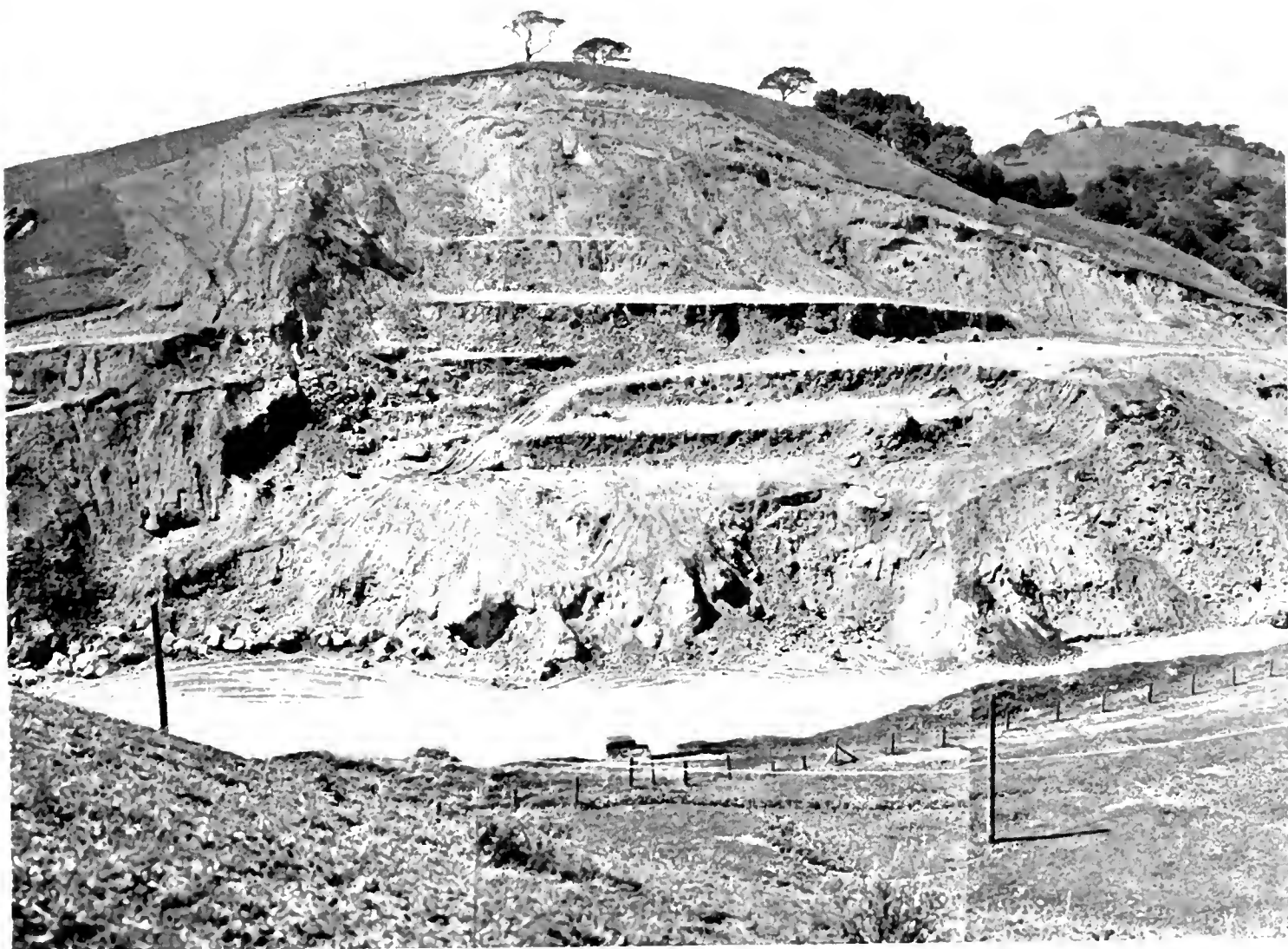
GIANT BENCHES WERE CUT for the removal of the slide material but the movements destroyed them almost as soon as they were graded. A total of 200,000 cubic yards of material was moved and the highway kept open at all times. Height of slide can be judged by comparison with size of the automobile on the highway in foreground.
