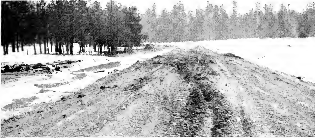
SURFACE BREAK west of Donner Summit caused by thawing and heavy trucking.
