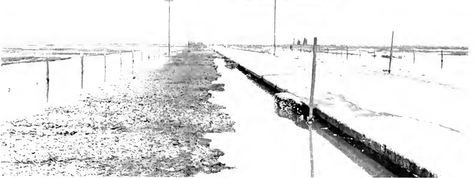
STORM DAMAGED HIGHWAYS. At top—Typical surface failure at mud slide on Coast Highway in Mendocino County. Center—Mountain stream diverted by blocked culvert wrecking highway. Bottom—Shoulder of Golden State Highway washed out by flood near Merced.
