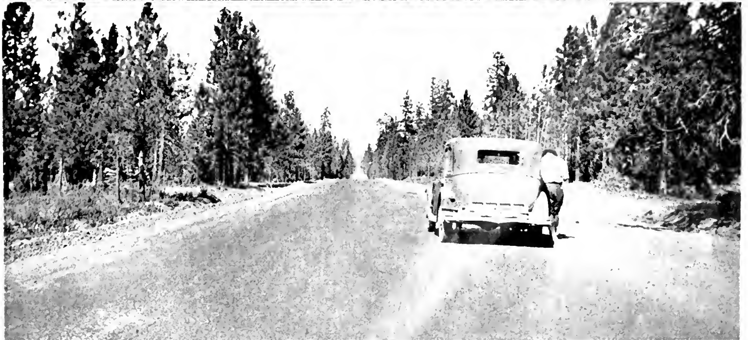
LAVA BEDS, CURVES AND MILEAGE are eliminated by realignment of the Redding-Alturas lateral between Burney and Fall River Mills. At top, narrow, winding old road through lava beds. Left center, new highway through chalk cliffs near Hat Creek Bridge. Right, construction scene in Pit River Canyon. At bottom, completed road east of Burney with only one curve in 7.5 miles.
