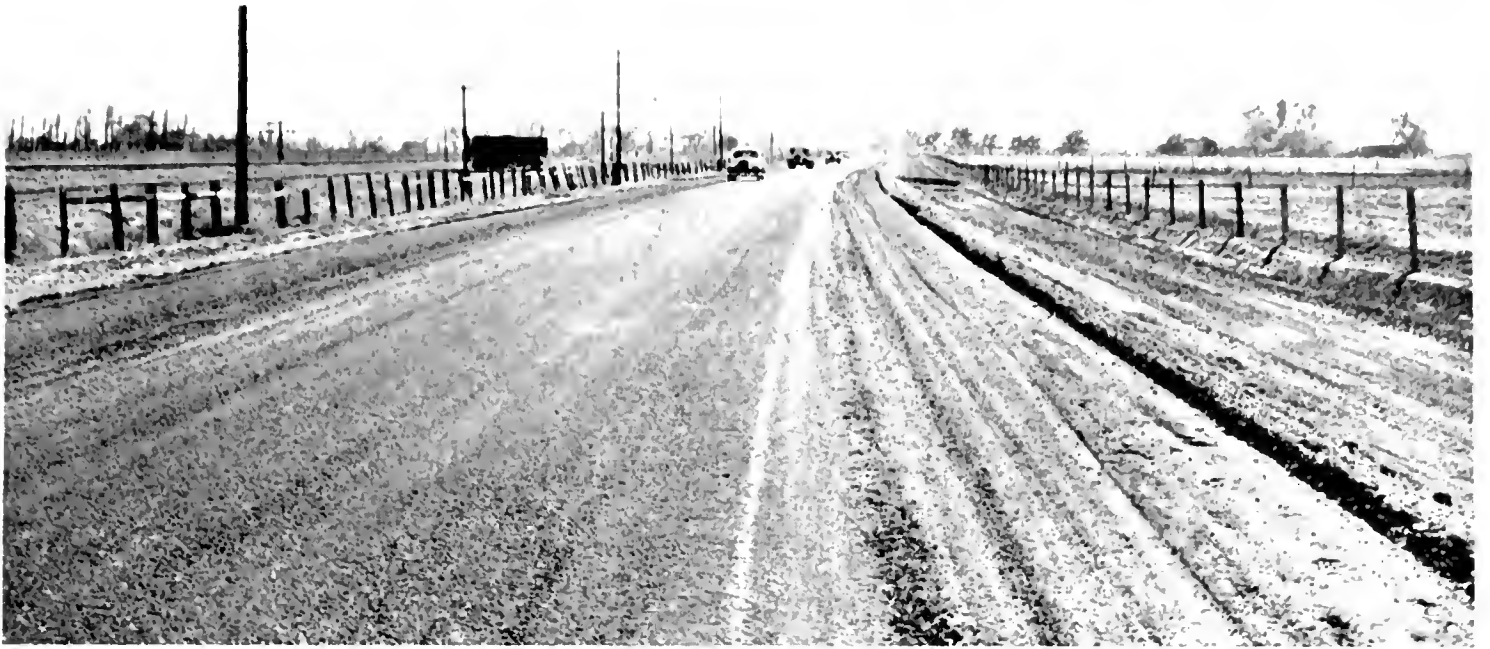
STRAIGHT AND WIDE runs the new highway for 4.54 miles between Newman and Crows Landing on State Route No. 41, cutting out many dangerous curves on the narrow old county route.
