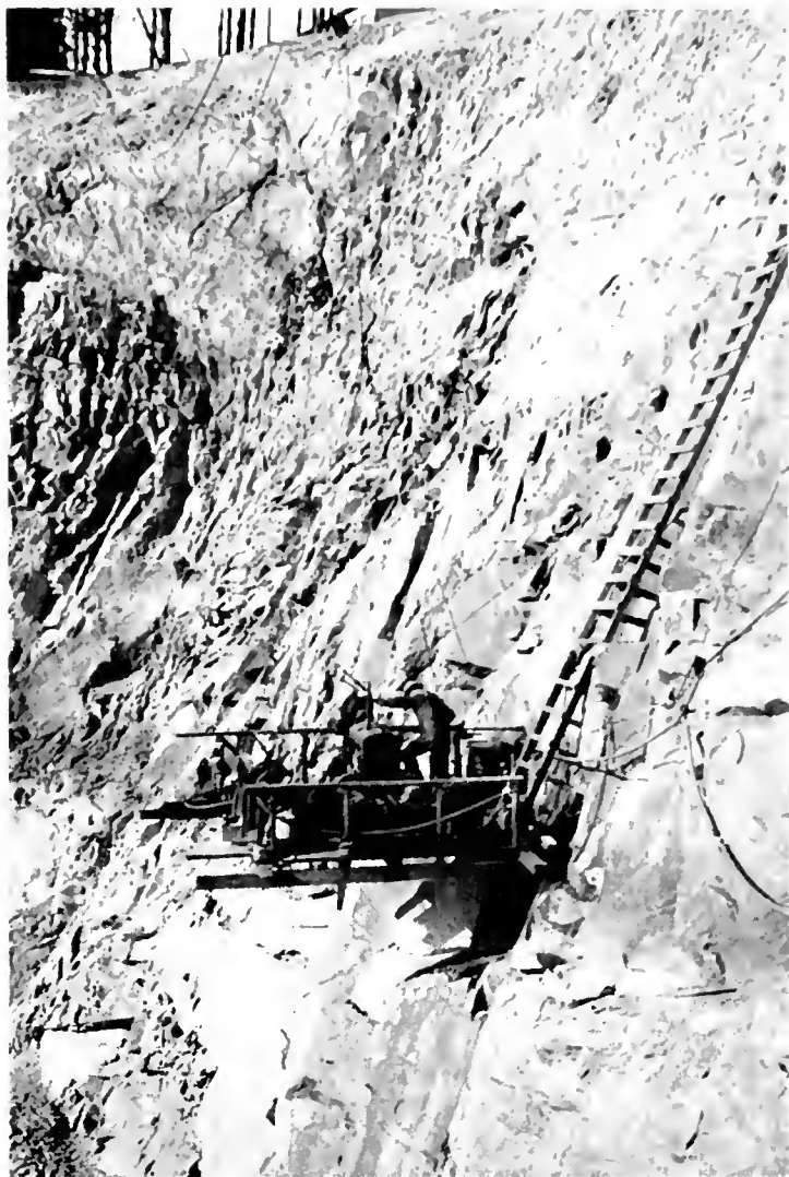
AN AIRY PERCH is provided for this equipment on the face of the west portal of the Yerba Buena Island tunnel where a 200-foot grout hole is being drilled.
