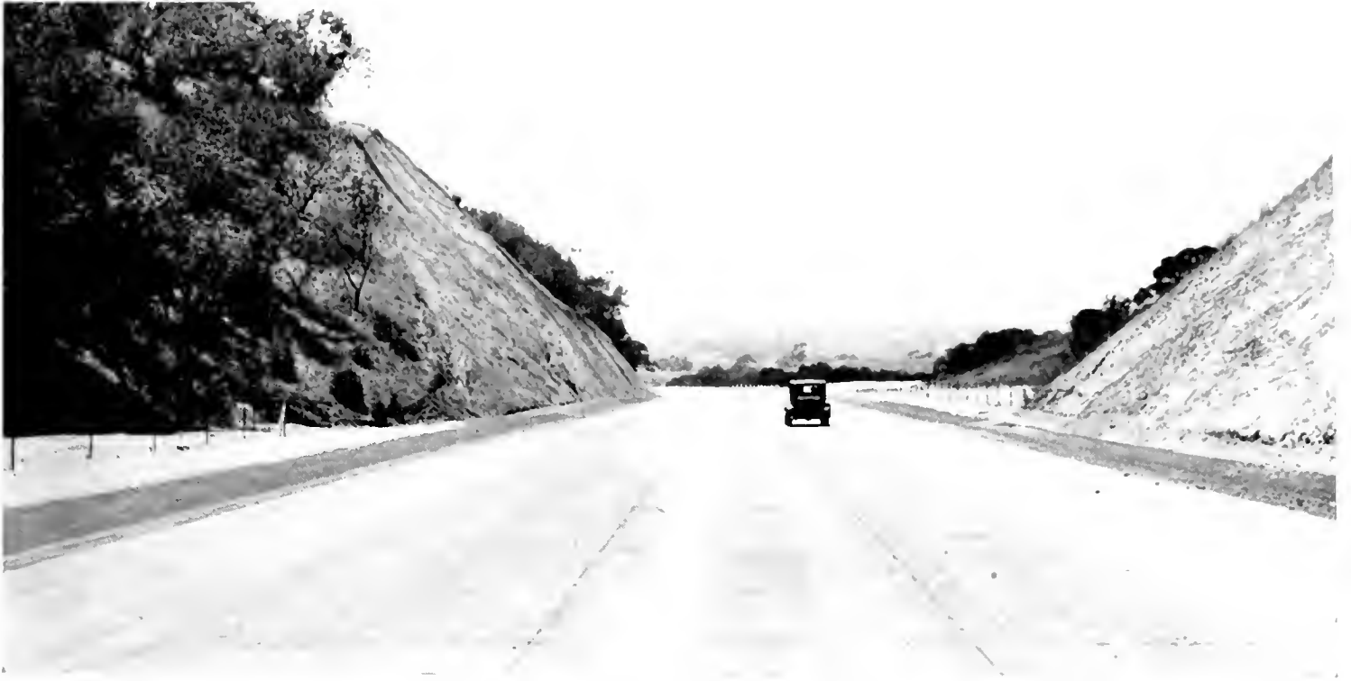
MANY BIG CUTS on Los Angeles-Pomona Highway permit a direct route through hills and wide oiled shoulders give additional width to broad traffic lanes.
