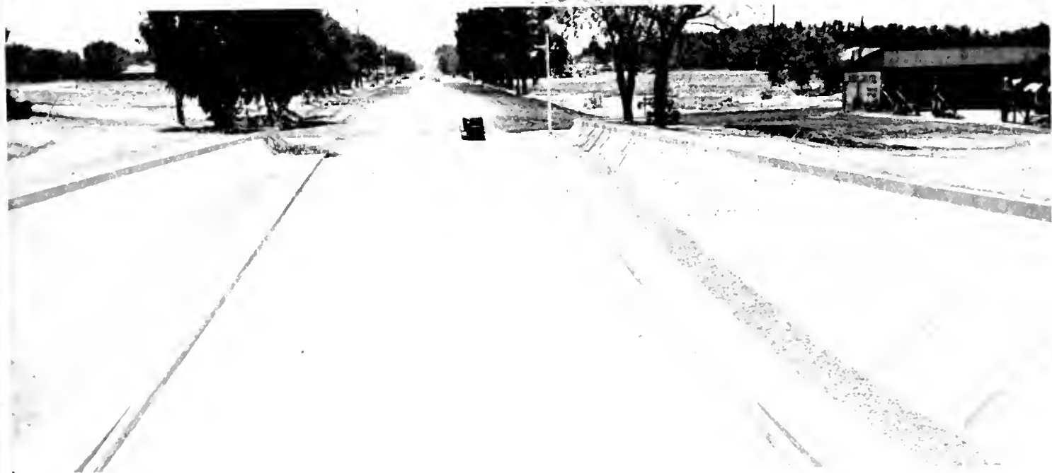
GRADE SEPARATION recently completed at Union Avenue on the Ridge Route in the city of Bakersfield with State gasoline tax funds. At top is shown the heavy girder span carrying four railroad tracks, the four lane subway with pedestrian walks and concrete slopes. Center pictures show the old structure and narrow road compared with the new wide approach and highway shown below.
