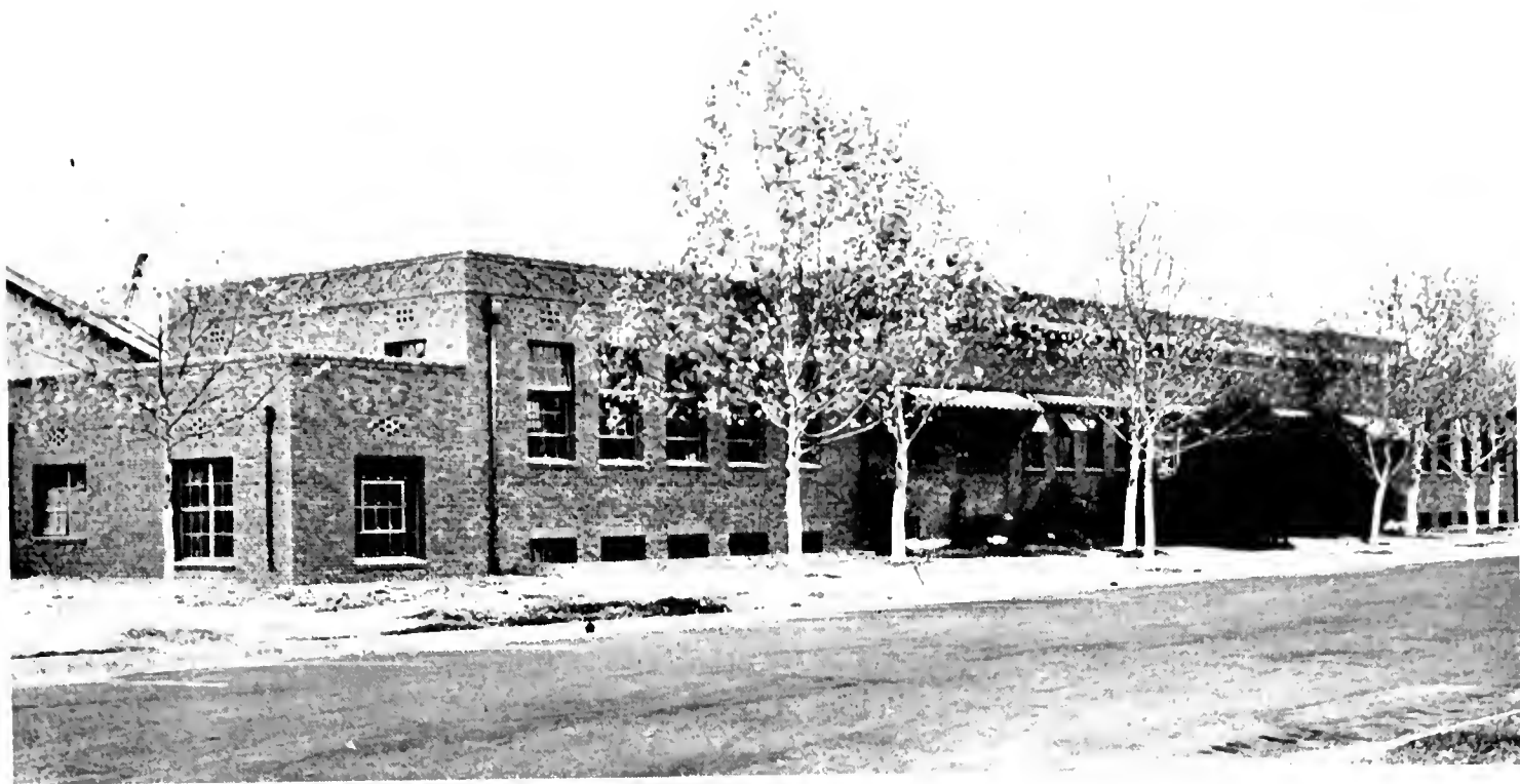
GROWING WINGS the Testing and Research Laboratory of the Division of Highways at 34th and Serra Way is expanding to take care of increased work. The wings add 5000 square feet of floor space.
