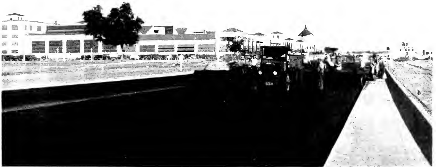
EXTENDING THE IMPROVEMENT for 600 feet east of Alameda street the original thin bituminous mixture surfacing, too light for the increased heavy traffic, is being paved to bring it up to the standards of pavement on either side of that short section.
