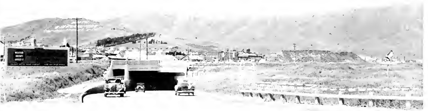
TRAFFIC DEMANDS MORE ROOM in the South San Francisco underpass on Bayshore Highway. Dotted lines on photo of Southern approach show proposed widening operation on structure, hillside and roadway.
