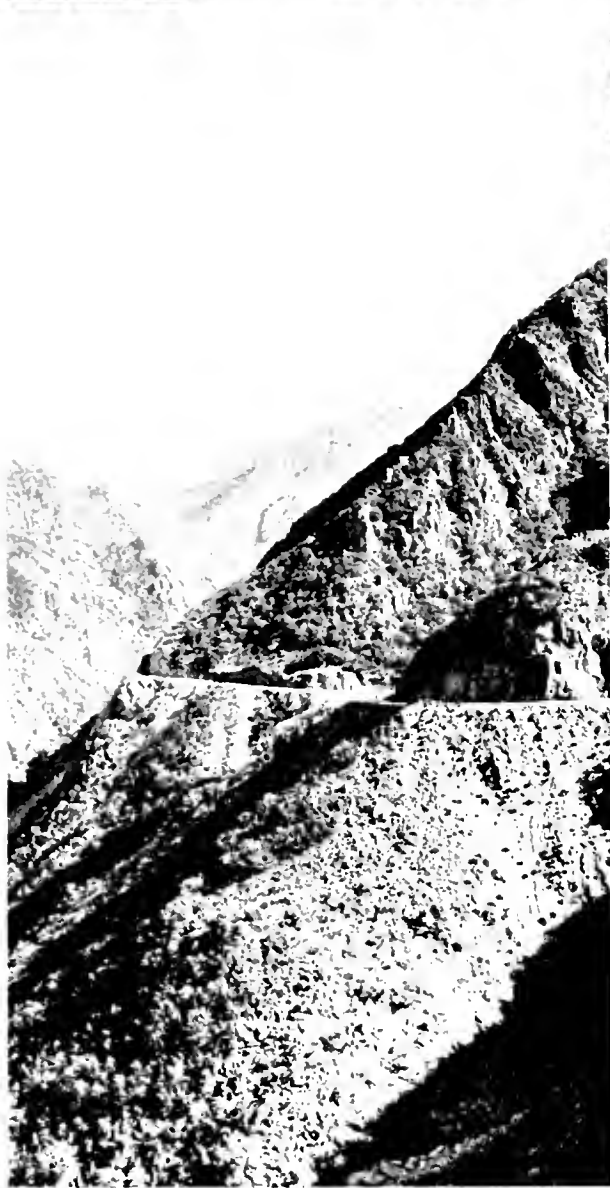
A MOUNTAIN RENT ASUNDER by the explosion of 75,450 pounds of dynamite was the spectacle beheld by a party of engineers in the Kings River canyon when the big blast moved 50,000 cubic yards of rock barring the progress of the Kings River Highway. Left upper photo shows the mountain spur and pioneer road before the blast and at right is seen the result of the blast. Below are shown a portion of the completed highway and the billowing smoke clouds that filled the canyon.
