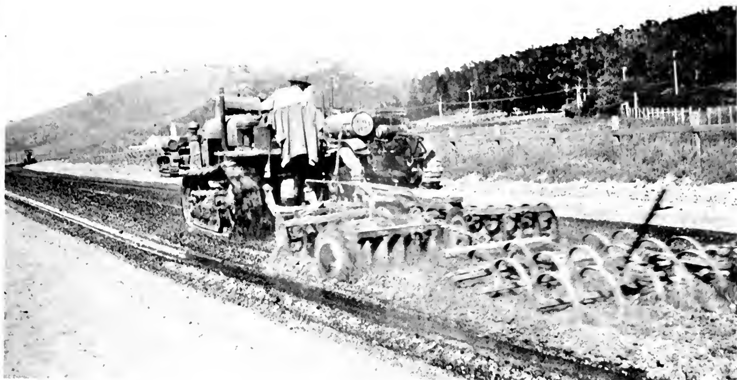
DISCING AND HARROWING road mix oiling project in Monterey County.
