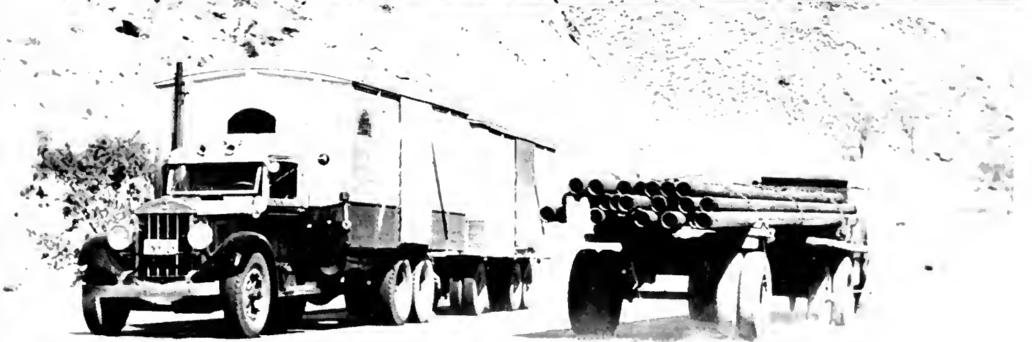
SPEED DIFFERENTIAL AN ACCIDENT FACTOR —The above pictures illustrate how slow moving trucks force faster moving autos into the lane of approaching traffic. At top, a scene on U. S. 99 near Banning showing automobiles trying to pass a line of 5 hay trucks from Imperial Valley. In center, autos are held up by a slow truck passing another in Altamont Pass. Bottom picture shows heavy trucking monopolizing the highway in Grapevine Canyon, Kern County.
