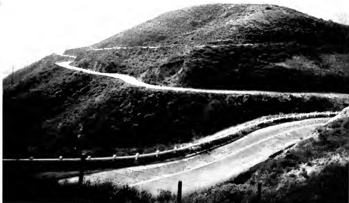
THROUGH THE HILLS to Half Moon Bay goes the new State highway instead of around the sides of steep gorges on stiff grades. The two upper pictures show the new highway and glimpses of the old line. At bottom is a view of the winding dangerous old road of many curves.
