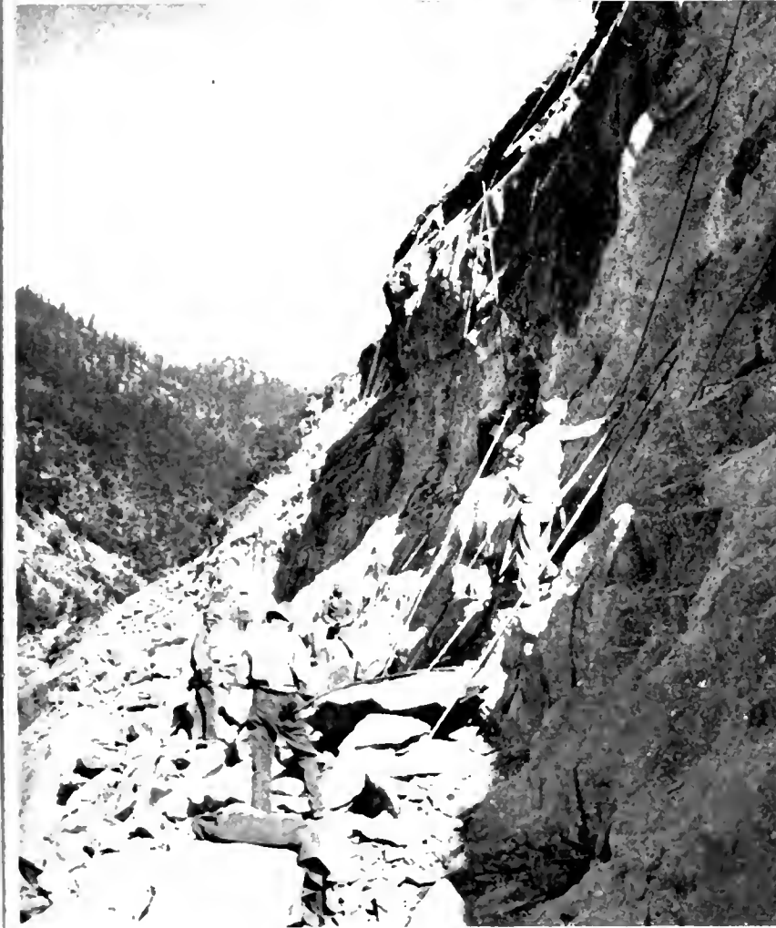
GRIZZLY DOME HIGHWAY OPERATIONS in Feather River Canyon involve much heavy rock work. At top drillers are widening the 400 foot bore. Lower views show crew widening the highway bench beyond tunnel and, at right, the entrance to the bore. The tractor is on grade.
