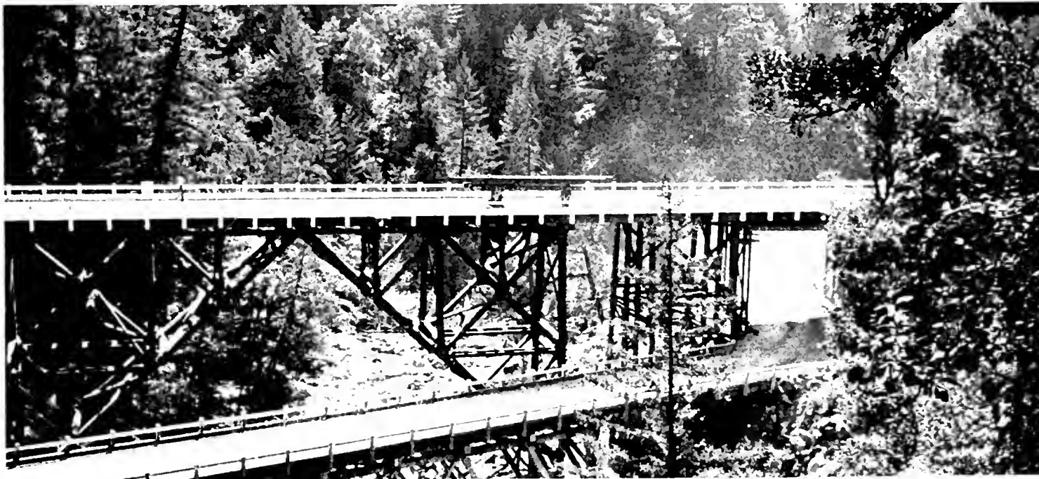
THE NEW AND OLD bridges are shown in this picture. The new crosses the creek 75 feet above stream-bed carrying the highway on a better grade and alignment and eliminating a vertical curve where the old road climbed out of the gorge.
