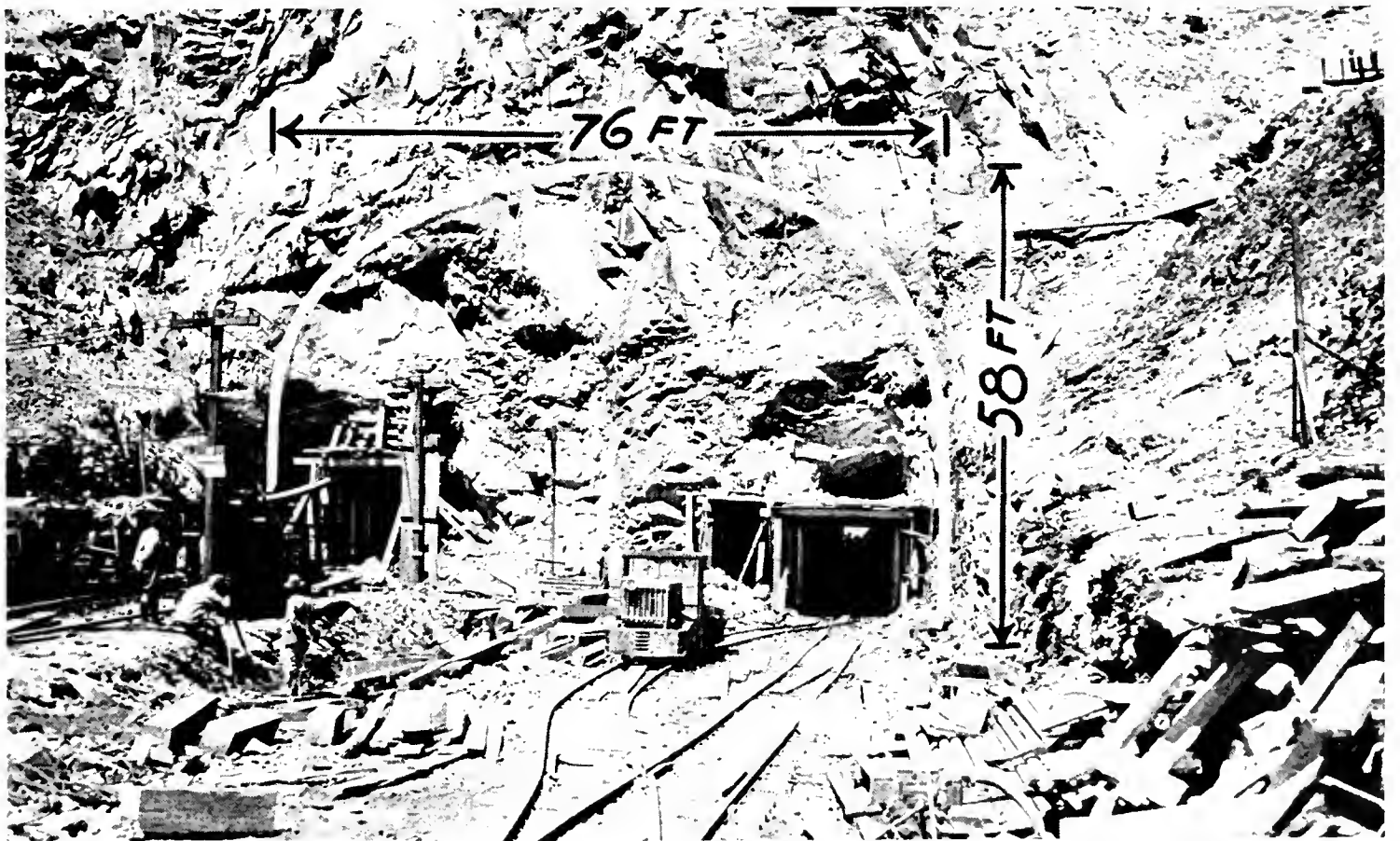
TWO PILOT TUNNELS each 12 by 12 feet have been bored through Yerba Buena Island, the first of which was completed on July 24th when Governor Merriam led a party through it. Three more small bores will be driven and all broken into one large 58 by 76 foot tunnel.— Photo courtesy San Francisco Examiner.
