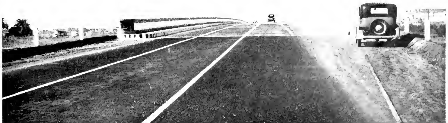
OVER THE SAN DIEGO RIVER, a noble steel and concrete bridge carries the new highway on a 40-foot roadway. It has a total length of 641 feet.
