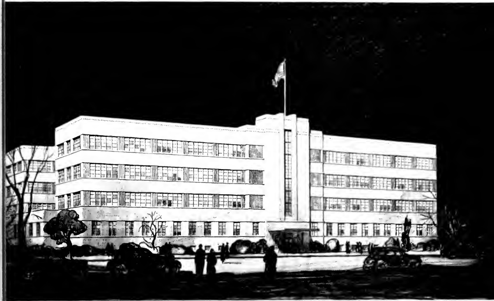
DIGNITY AND BEAUTY characterize the simple modern design of the new Public Works Building under construction in Sacramento, a 4-story reinforced concrete structure with provision for a fifth story.
