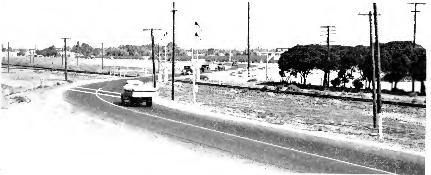
GRADE CROSSING on "S" curve at Delano on the Golden State highway. This bad situation is being corrected with a realignment of the highway and construction of an underpass.
