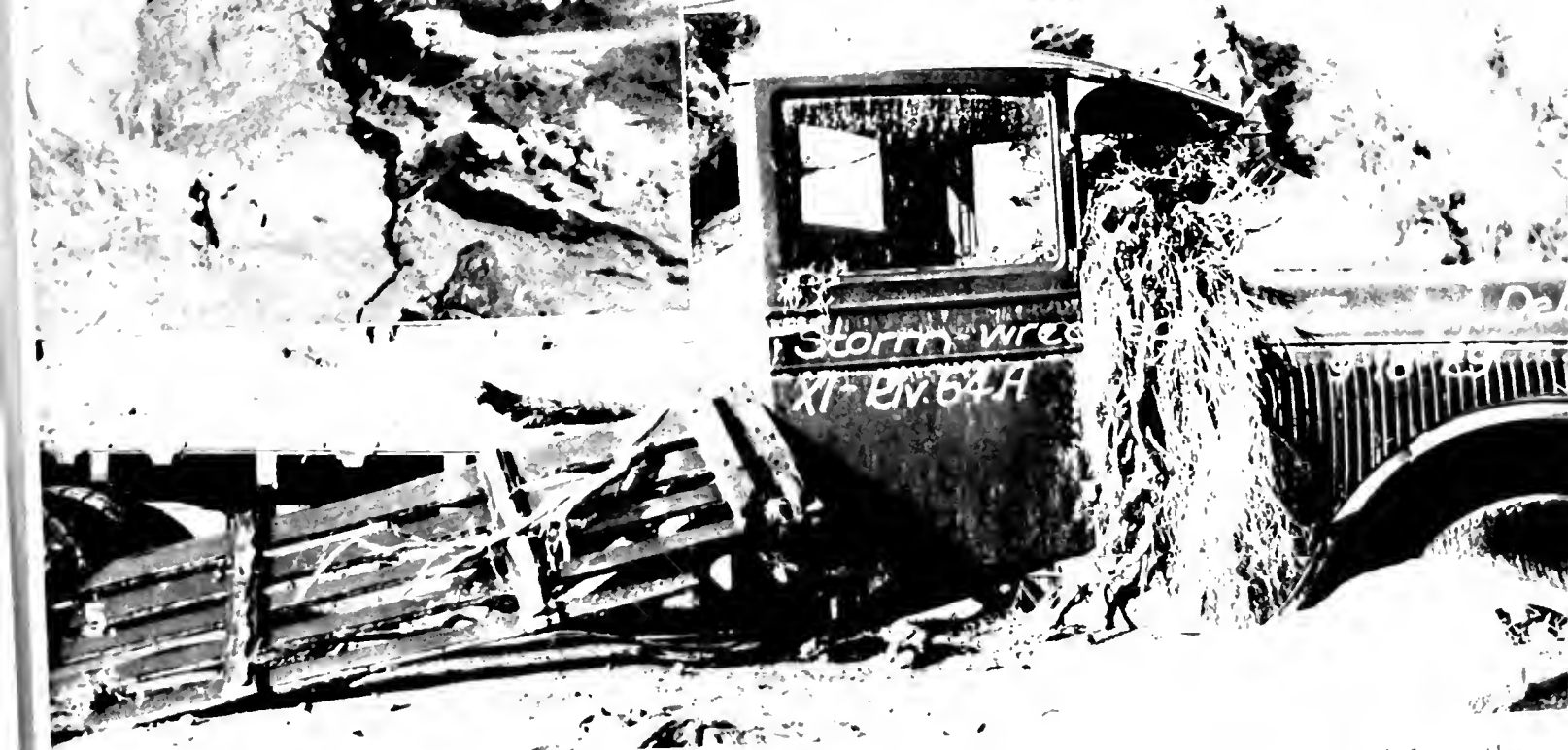
INDIO CUTOFF COMPLETED and opened to traffic removes U. S. 60 on State Route 64 from the storm damage and hazards of travel on old Box Canyon route. Nos. 1 and 2 show sections of the new cutoff. No. 3. Old winding road between precipitous rock walls in bottom of Box Canyon. No. 4. Example of storm damage on old route. No. 5. Truck caught and wrecked in Box Canyon flood.
