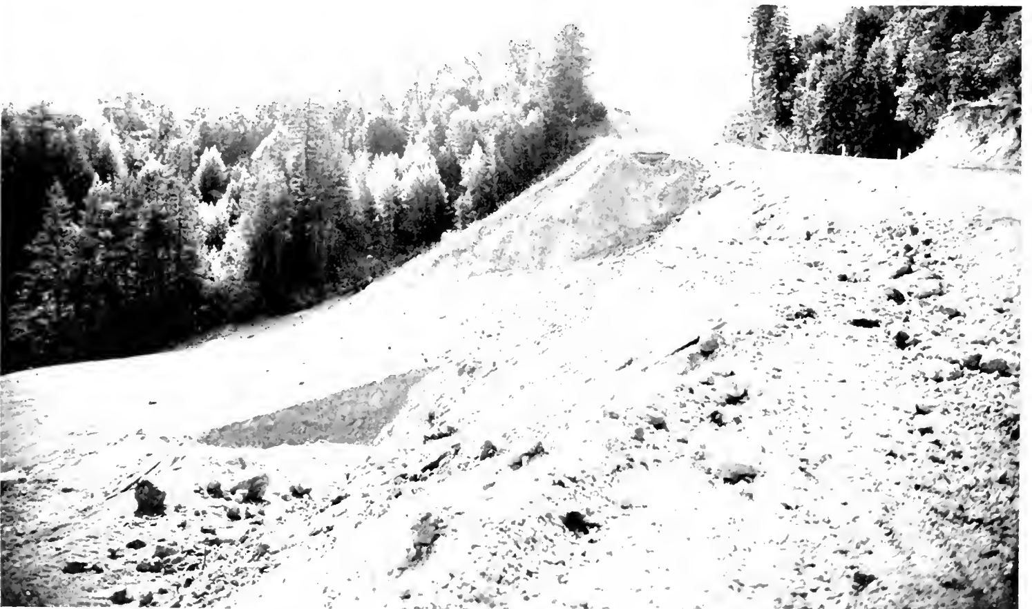
LOWER SLIDE AREA where 50 per cent of the fill slipped a distance of 300 feet down the mountain side and was stopped by trenching and backfilling with rock.
