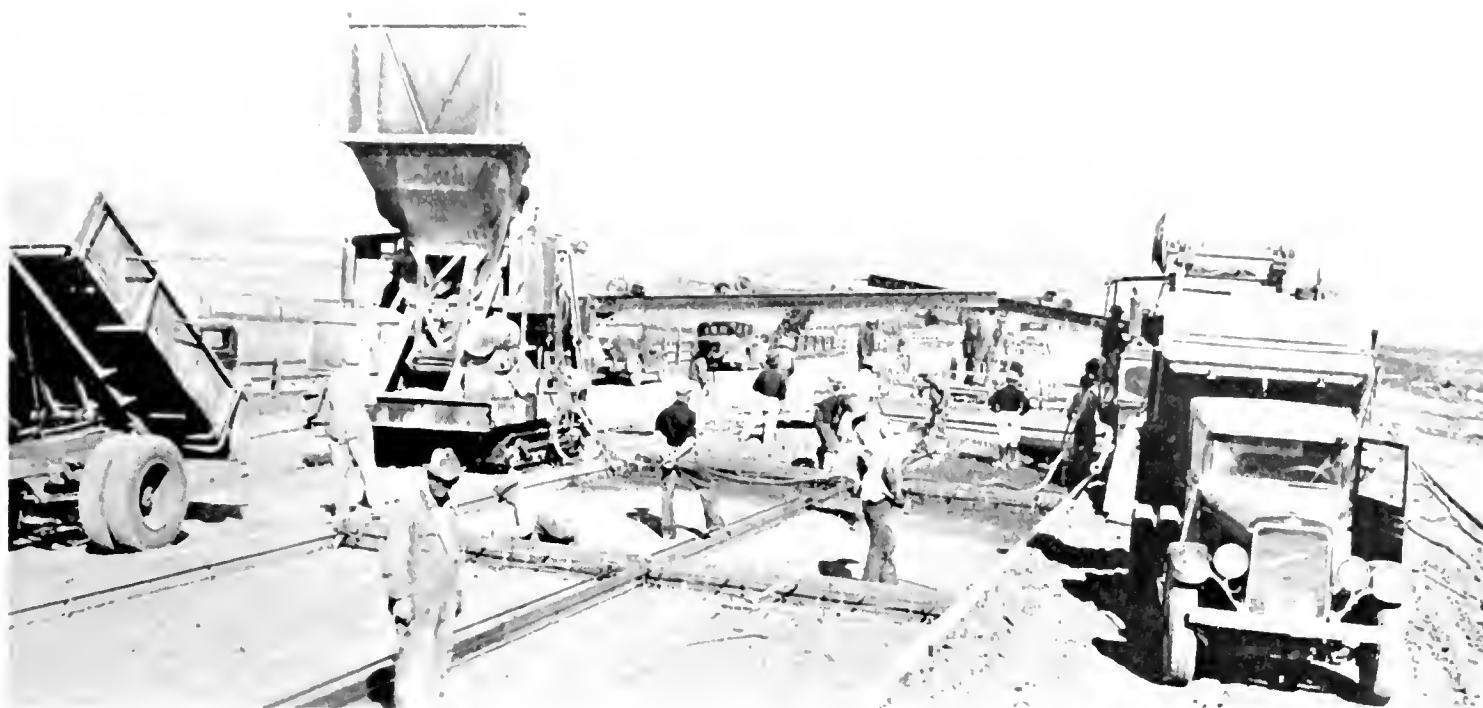
TWO PAVERS working on 40-foot portland cement project on Bayshore Highway in Santa Clara County
