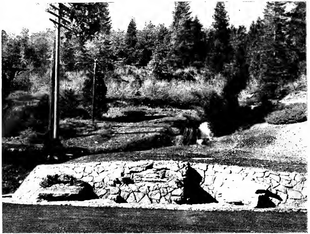
ROCKWORK SEAT and drinking fountain on new realignment
