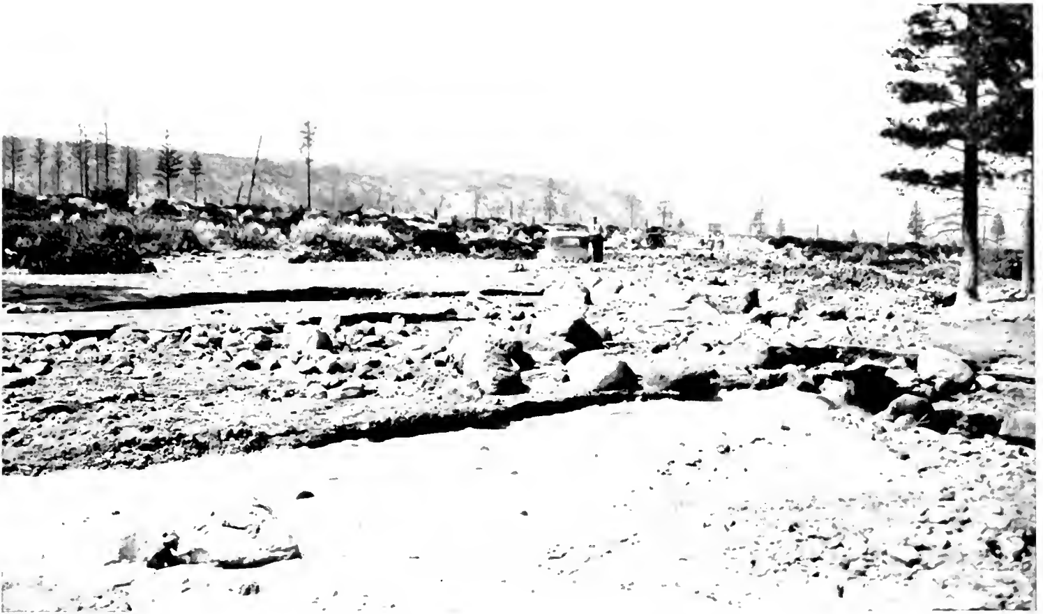
DEBRIS FROM SHASTA GLACIER flood waters covered State Highway 72 in storm of August 28 to a depth of four feet as shown in pictures on this page and page 29.
