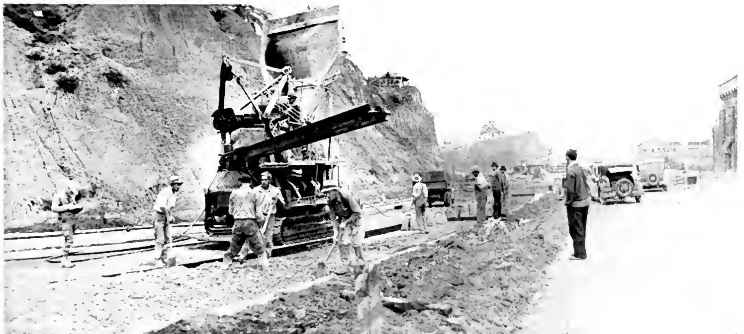
CONCRETE PAVER AT WORK on the widened Coast Highway along the Palisades in the Santa Monica beach recreational area in Los Angeles County. This contract provides a 76-foot pavement at a point of heavy traffic where the highway swings from the beach toward the portal of the Colorado Street tunnel now under construction.
