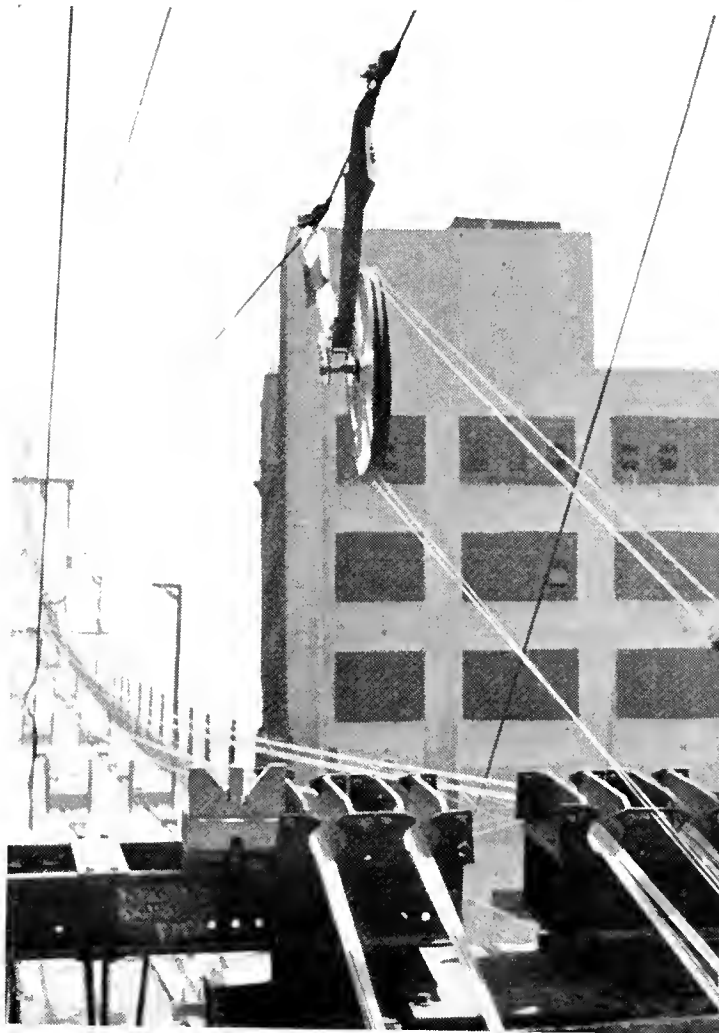
THE SPINNING WHEEL is 5 feet in diameter and carries two loops of the pencil size cable wire on each trip traveling 7 miles an hour.
