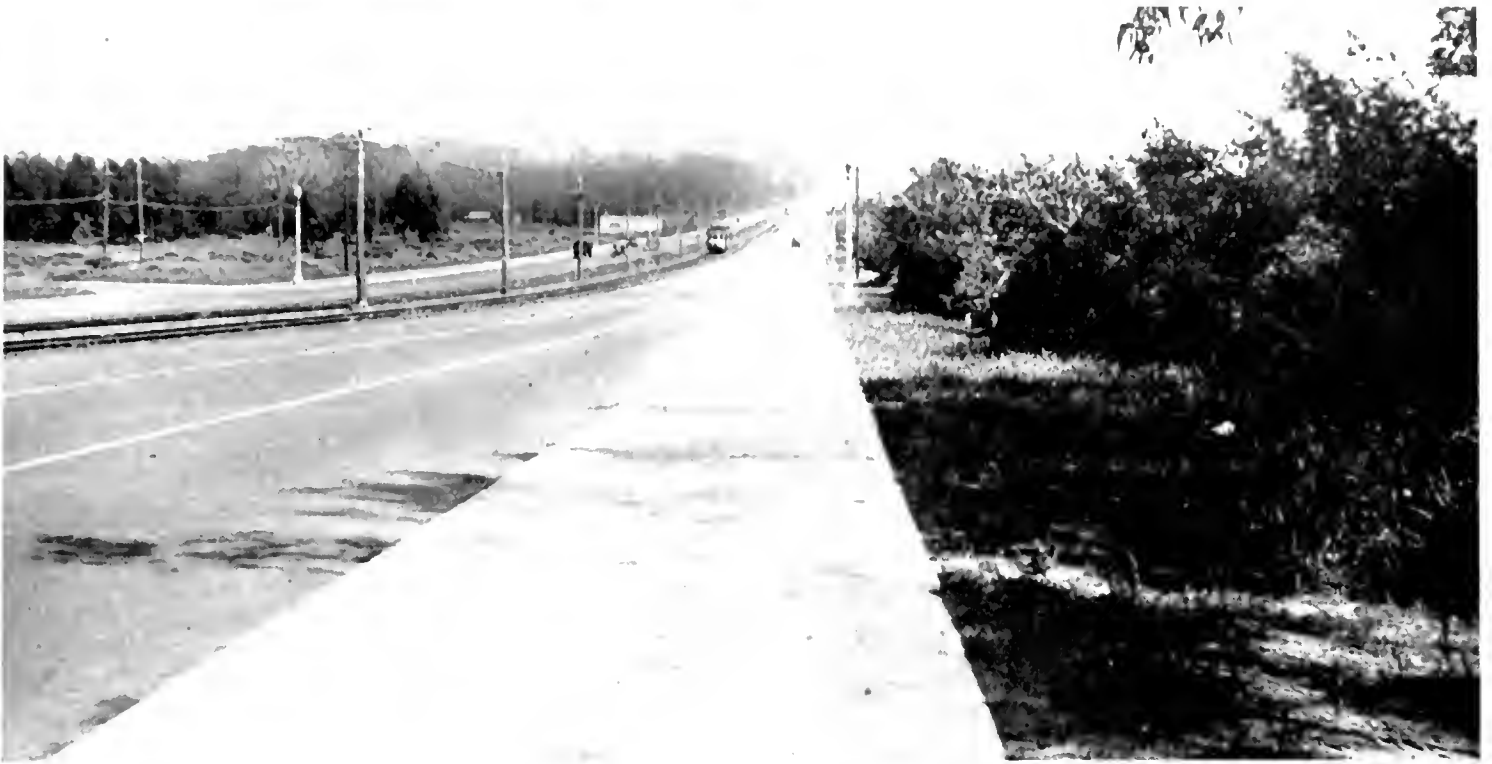
SLOAT BOULEVARD, San Francisco County, with 40-foot asphalt concrete pavement and 16-foot portland cement concrete widening.
