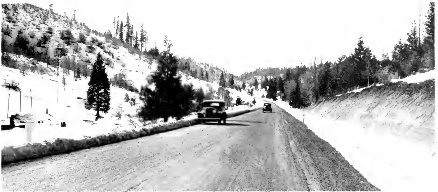
SPEEDY, SAFE TRAVELING for motorists is provided by the 11.5 miles of new highway on the Donner Summit route affording the only year-round trunk road leading out of northern California.
