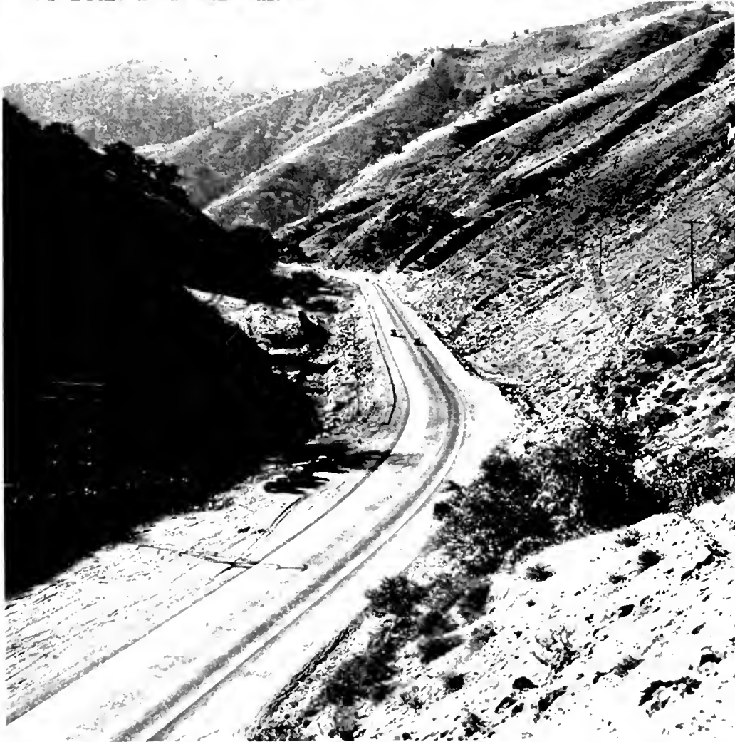
NO "DEATH CURVES" HERE. Views of the completed 3½ mile improvement of the northern section of the famous Ridge Route show that the former dangerous curves and narrow roadway have been replaced by a fine, safe three-lane modern highway. This canyon, which is the main pass between Los Angeles and the San Joaquin Valley, carries not only the State Highway, but also transmission lines of two power companies, three gas pipelines from Kettleman Hills to Los Angeles and pipelines of two large oil companies. All these utilities had to be constructed and rearranged to avoid interference with the new highway.
