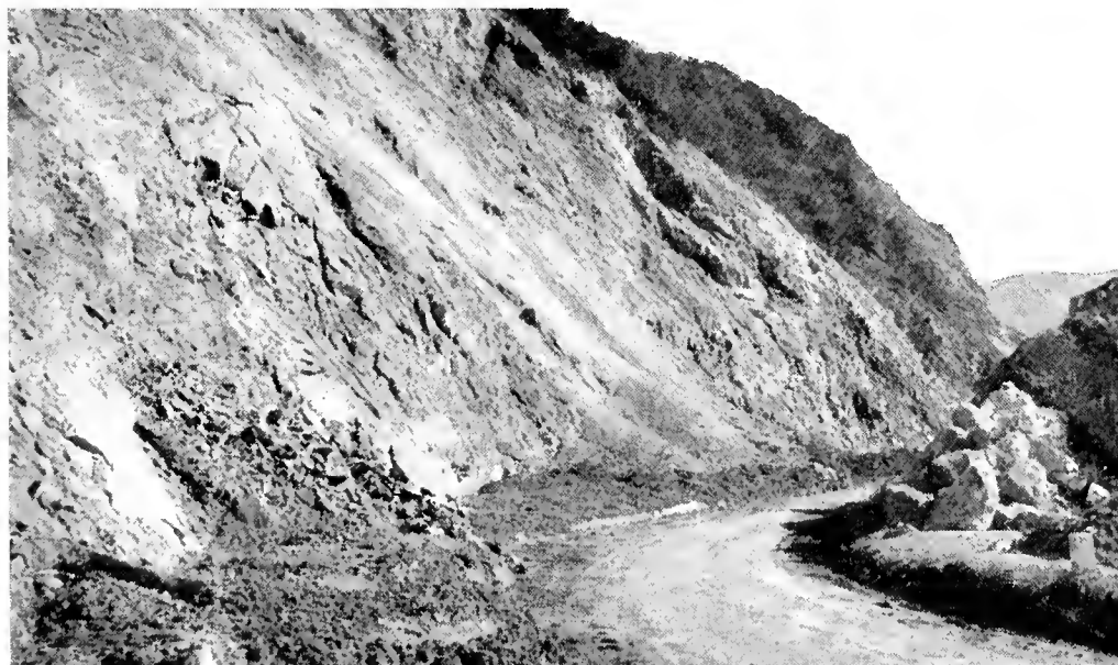
STORM SLIDES AND MUD blocked Route 162, San Gabriel Canyon.
