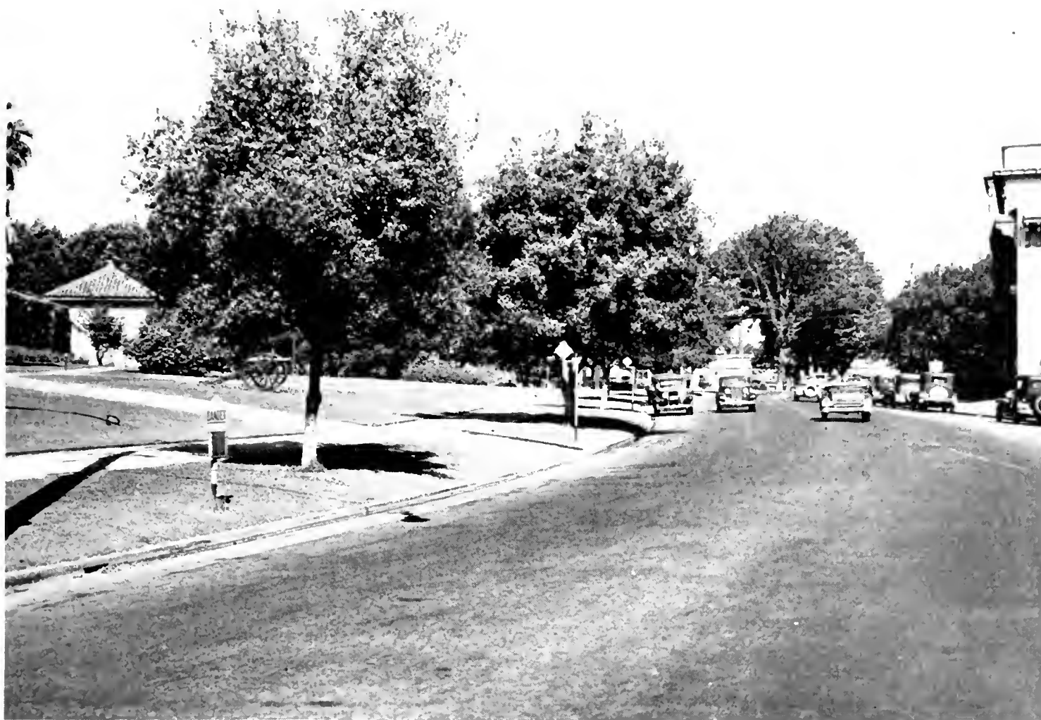
GAS TAX PAVEMENT recently completed on "L" Street in the city of Sacramento where State Highway Route No. 4 passes the historic Fort Sutter situated in Sutter Park.
