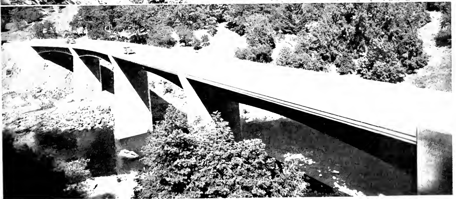
BEAUTY AWARD WINNER in a bridge contest and not a card game, is this State designed structure on the Redwood Highway where it crosses the South Fork of the Eel River just south of Garberville. It is the first continuous steel girder bridge built on a curve in America and was awarded honorable mention in a national competition for the most beautiful steel bridge built last year.
