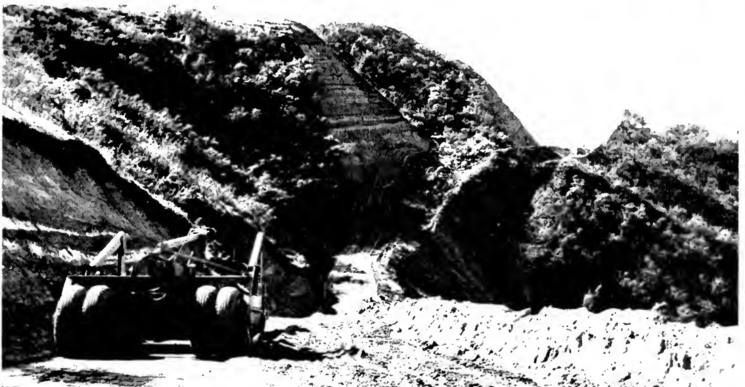
CONSTRUCTION SCENE showing character of heavy grading work on fill leading to two 100 foot cuts.
