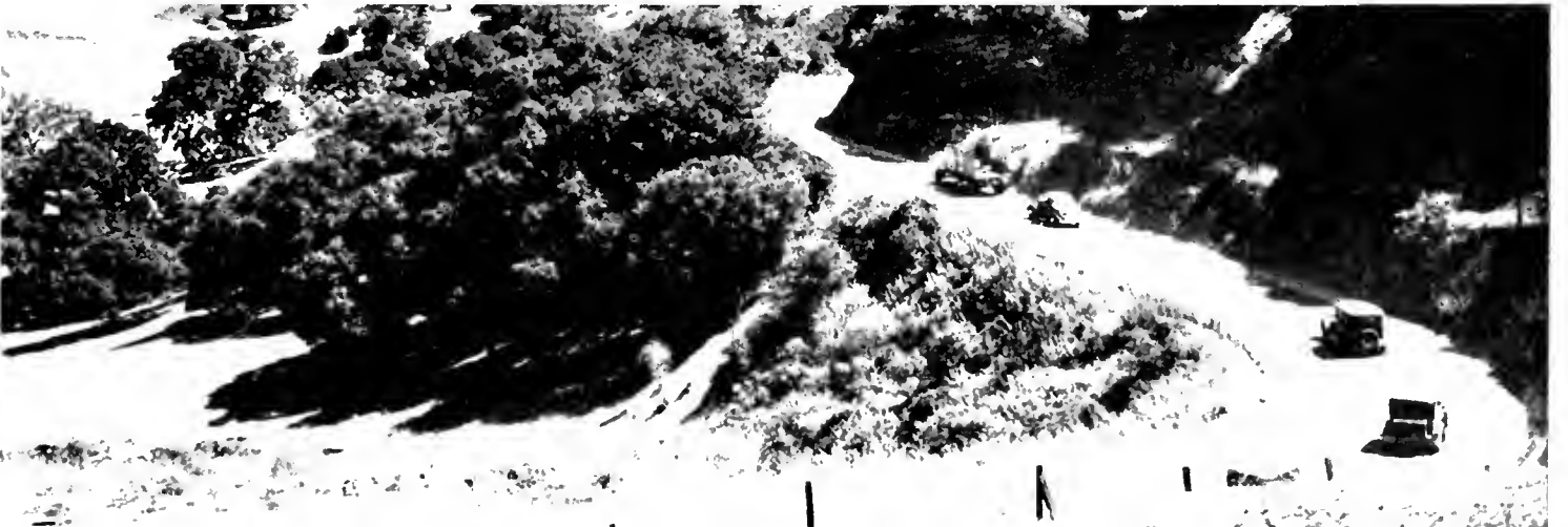
OLD ROUTE abounded in hairpin turns such as the two shown in the above picture taken before the improvement when traffic was compelled to loiter along behind heavily laden trucks.
