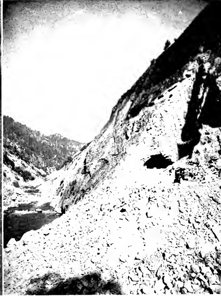
GRIZZLY DOME HIGHWAY OPERATIONS in Feather River Canyon involve much heavy rock work. At top drillers are widening the 400 foot bore. Lower views show crew widening the highway bench beyond tunnel and, at right, the entrance to the bore. The tractor is on grade.
