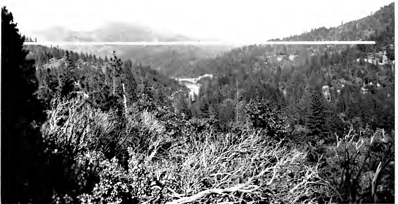
NEW BRIDGE SITE across the Pit River for the proposed joint highway and railroad bridge made necessary by the Kennett Dam project is indicated by the white line, 325 feet higher than present bridge shown in background.
