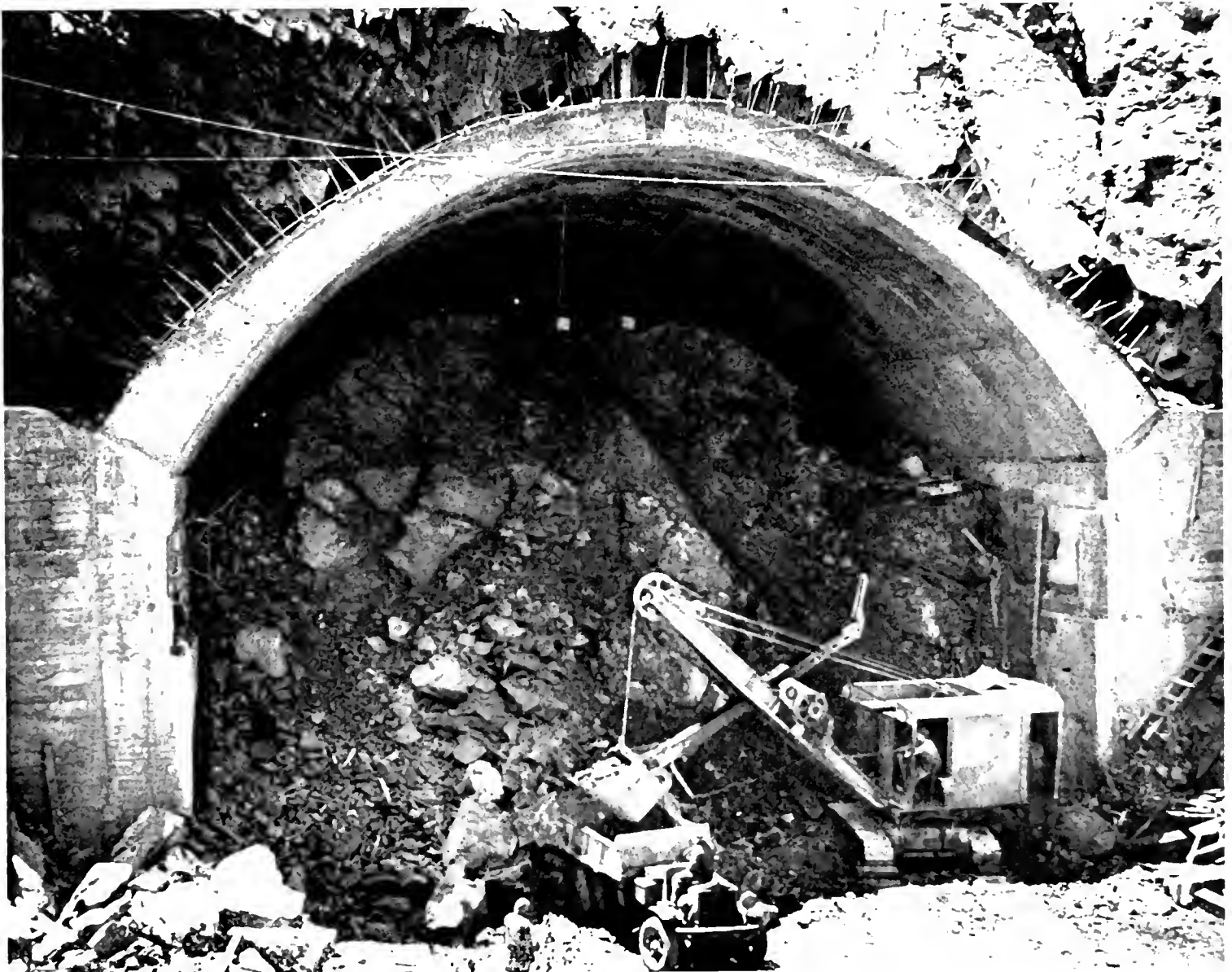
DOWN TO THE CORE. With the tunnel completely concreted and steel lined by novel construction methods a steam shovel begins removal of thousands of cubic yards of rock from 58 by 76-foot bore.
