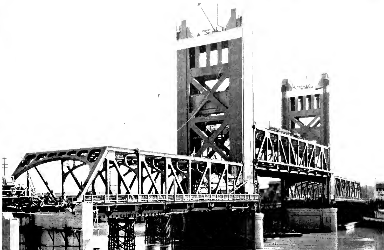
NEARING COMPLETION, the M Street bridge over the Sacramento River at the State capital is pictured with the 202-foot steel truss lift span in raised position still partially supported by false work.
