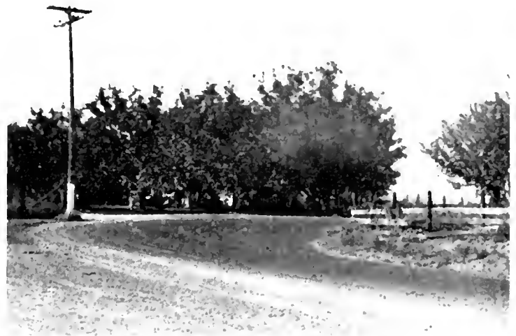
RIGHT ANGLE TURNS were responsible for a bad accident record on the six mile stretch of old highway, one in particular being the scene of several fatalities. Two of these turns are pictured.
