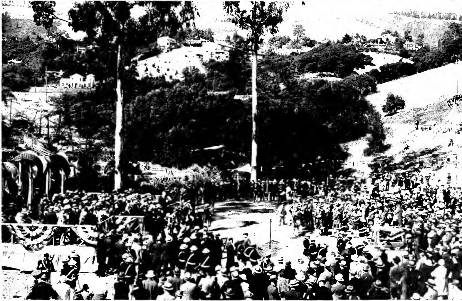
STARTING WORK ON A GREAT PROJECT. Governor Merriam and Director Earl Lee Kelly participated on June 17 in ground breaking ceremonies at Oakland for the Broadway low level tunnel to connect Alameda and Contra Costa counties. In the upper picture Governor Merriam is seen turning the first shovelful of earth assisted by Director Kelly; Supervisor T. E. Caldecott, chairman of Joint Highway District No. 13; Dudley W. Frost (kneeling), chairman of Oakland and Berkeley Junior Chamber of Commerce Committee, and a group of young women representing participating communities. A beautiful eucalyptus grove at Broadway and Chabot Road, Oakland, was the scene of the formal exercises, which included speechmaking, music of massed bands, pageantry and fireworks.
