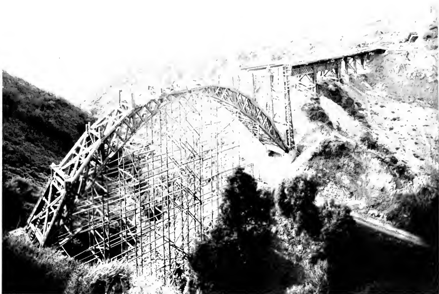
DOLAN CREEK TIMBER ARCH —This 180-foot span on Carmel-San Simeon highway involved some pioneering construction for a timber span of such length. Metal ring connectors were used to increase the strength of the timber joints.
