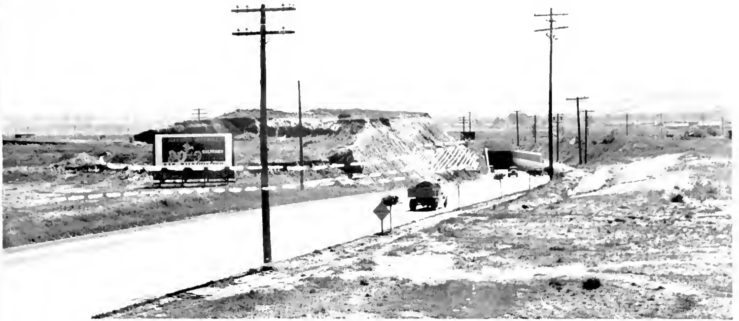
TRAFFIC DEMANDS MORE ROOM in the South San Francisco underpass on Bayshore Highway. Dotted lines on photo of Southern approach show proposed widening operation on structure, hillside and roadway.
