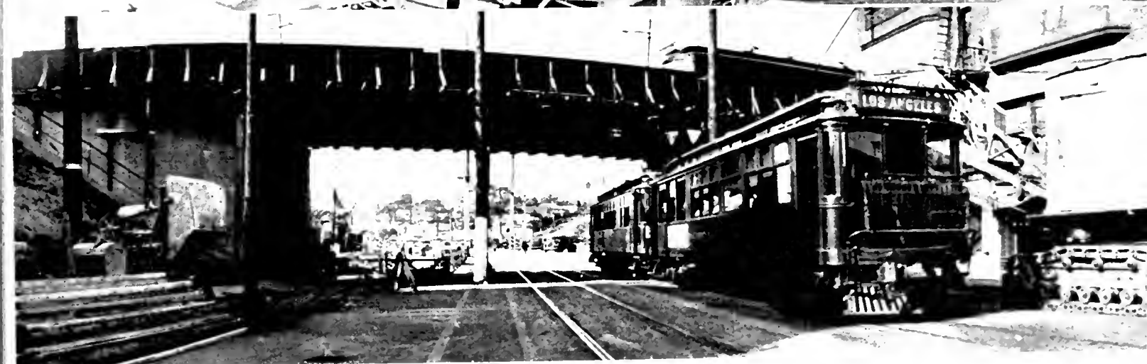
BUSY SCENE IN CITY'S HEART. Activities attendant upon the construction by the State of the $130,000 viaduct now being built over Glendale Boulevard at the intersection with Sunset Boulevard in the city of Los Angeles is shown in the top sketch by Artist Charles Owens of the "Los Angeles Times." The lower photographs show how the excavation and building work is being carried on without interrupting traffic of the two street railway lines on both levels of the grade separation.
