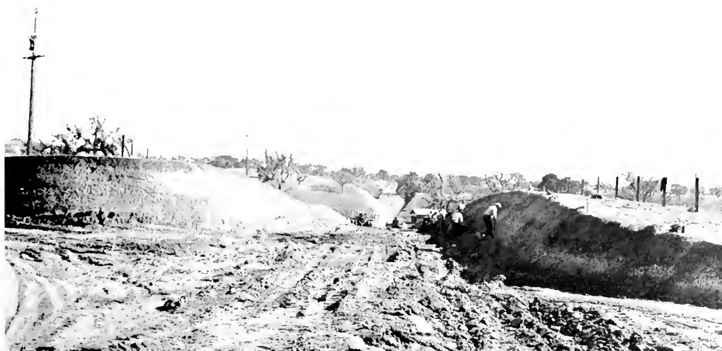
DIRECT LINE RECONSTRUCTION is typified in the realignment of 5.6 miles of San Marcos Pass route through Santa Ynez and Los Olivos in Santa Barbara County. The existing route zigzags back and forth, following section lines, resulting in many right angled turns with their accompanying dangers and inconvenience to modern traffic. The new line on which grading operations are under way goes straight across country with a resulting saving of 2 miles to motorists in time and distance.
