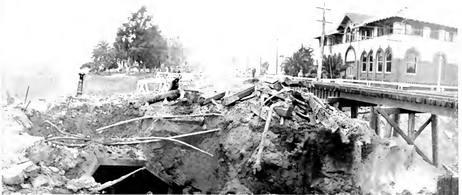
OPEN CUT CONSTRUCTION from the Beach road through Palisades Park and Ocean Avenue at Santa Monica to build tunnel for new highway. Part of old railroad tunnel shows in foreground.
