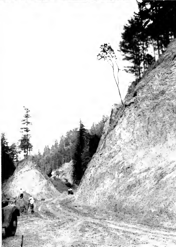
THROUGH THE REDWOODS in Humboldt County dangerous sections of the State highway are being relocated and many sharp curves eliminated. The top picture shows clearing operations preparatory to straightening the road at one of the curves. Below, at left, is a view of grading operations on the precipitous Redway Bluffs. At right is a picture of one of the redwood cribs used for fills.
