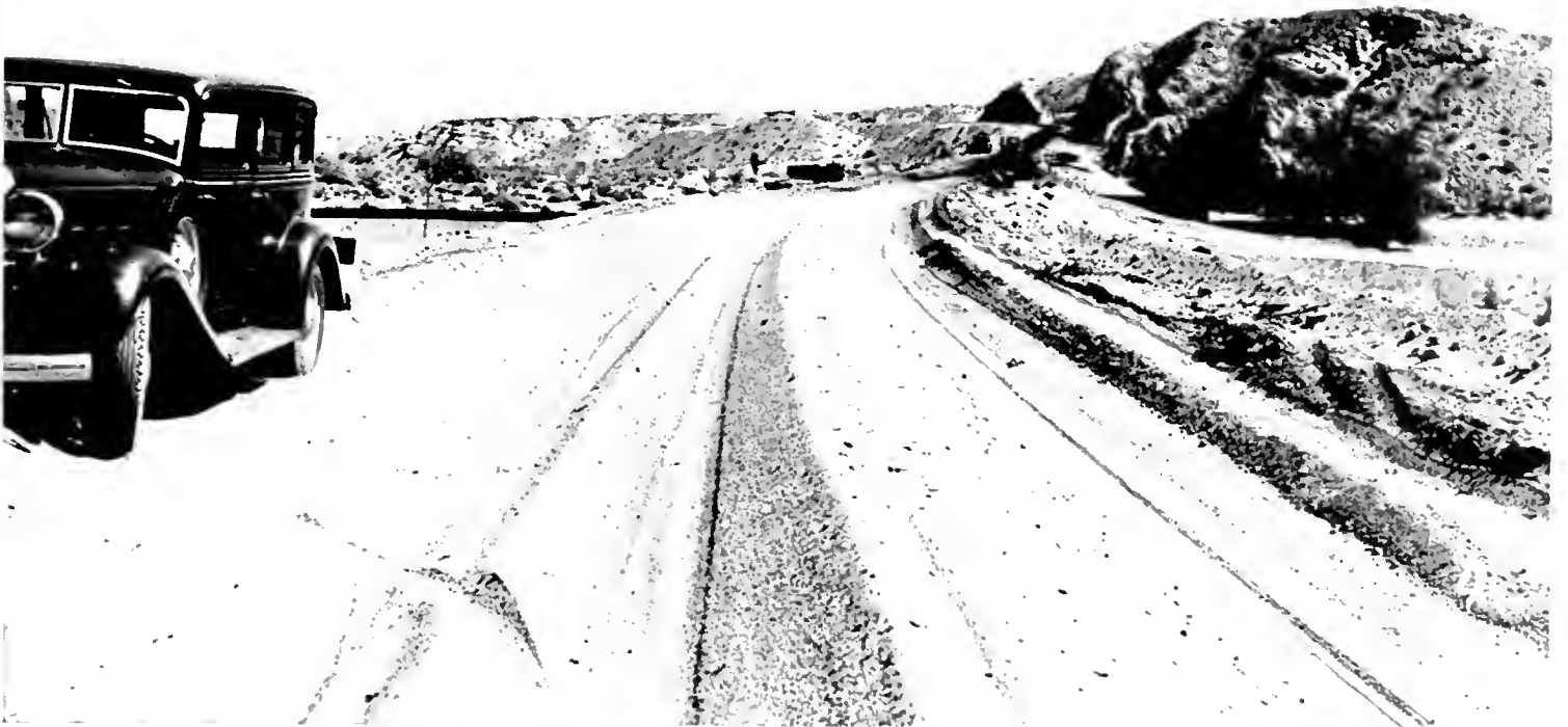
A MECHANICAL WINDROW SIZER has been invented by engineers on a State job in Riverside County. A blade grader equipped with the sizer is shown in No. 1 and a close-up of the sizer in No. 2. Note adjustable plate at top of orifice. Excess flows out wing on left. No. 3—Blocking out and weighing windrow section to determine percentage of oil. No. 4—Completed windrow showing excess on left.
