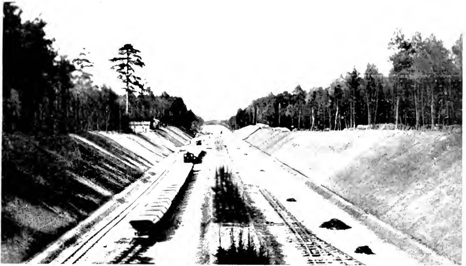
GERMAN EXPRESS HIGHWAY under construction. This typical section provides for a center lawn strip 15 feet wide, with a pavement 25 feet wide, consisting of two traffic lanes on either side bordered by shoulders. Note the planting of trees and shrubbery on center strip.
