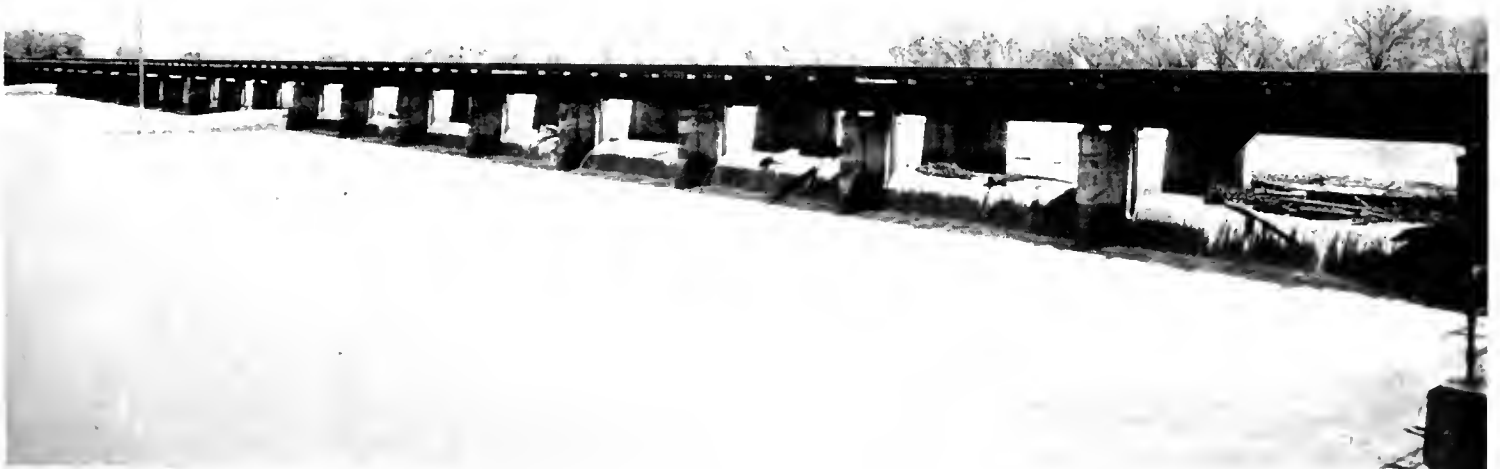
SACRAMENTO WEIR HANDLING 12,000 SECOND FEET at peak of flood is 1800 feet long and located 4 miles upstream from city. Water flowed over the weir at a depth of 1.65 feet but it was unnecessary to open the gates. Secondary State Highway Route 50 crosses on top of weir structure.
