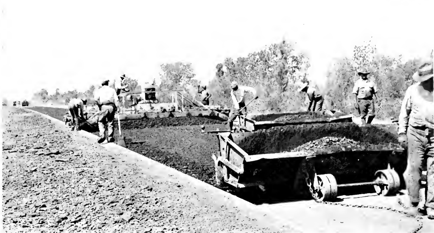
PLACING ASPHALT CONCRETE BASE COURSE on contract in Sacramento County.
