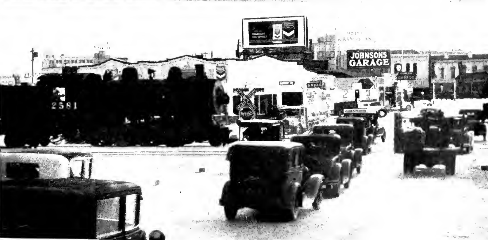
MODEL AND PHOTOGRAPHS picture the safety and traffic aspects of the proposed grade separation and subway improvement in the City of Salinas where a railroad crosses the intersection of the State highway and Main Street. The model, at top, shows the present dangerous grade intersection replaced by a wide subway with the railroad carried across on a girder bridge and a parked area separating traffic. Present conditions are shown in the photographs.
