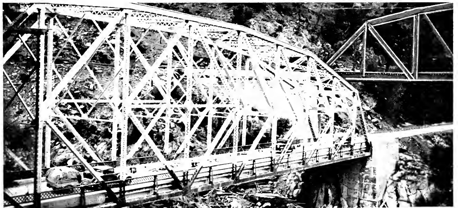
TOBIN BRIDGE, dwarfed in above picture, is larger than railroad structure, being 290 feet long, 24 feet wide.
