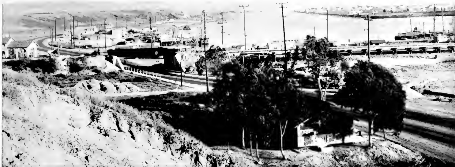
GRADE SEPARATION SITE of Newport Beach project. The Coast Highway passes building in foreground and extends southerly around Newport Bay. Santa Ana road crosses just beyond railroad overhead.
