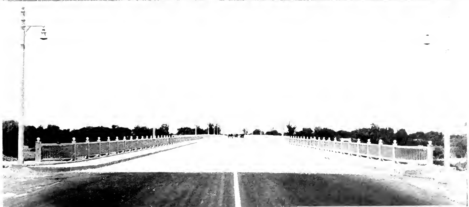
BAKERSFIELD BY-PASS UNITS examples of modern construction. At top, four-lane steel and concrete overpass spanning railroad tracks. Center, portion of 30-ft. asphaltic concrete pavement with 3-ft. shoulders. Below, steel and concrete bridge over Kern River, 2293 feet long with 40-ft. roadway.
