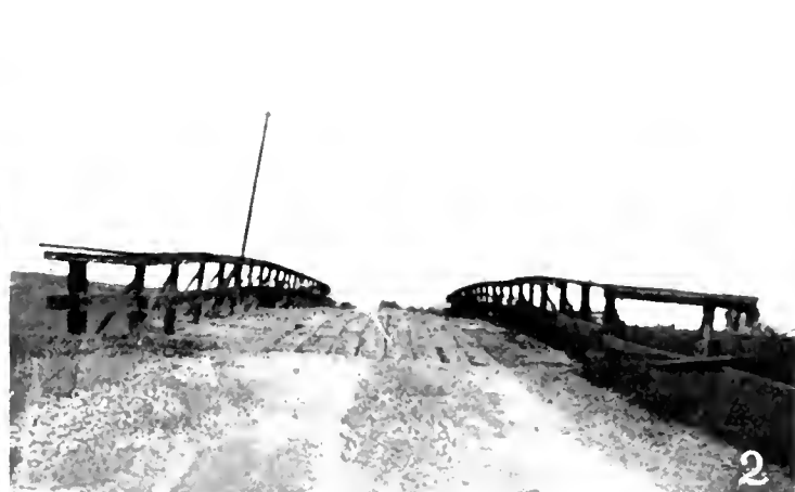
TYPICAL OF BRIDGE DETERIORATION to the danger point when taken into the secondary system was the high span across Jughandle Creek on the Mendocino shoreline coast road shown in the three top pictures. It was a combination wood and steel deck truss structure with bad approach alignment and wooden roadway shown in Nos. 4 and 5. No. 3 is a closeup of one of the lower chord joints seriously weakened by rusting of the metal. The State has made temporary repairs by adding strengthening supports. Pictures 1 and 2 show the old timber trestle on Route 101 between Dixon and the Rio Vista-Fairfield road before and after being taken over by the State.
