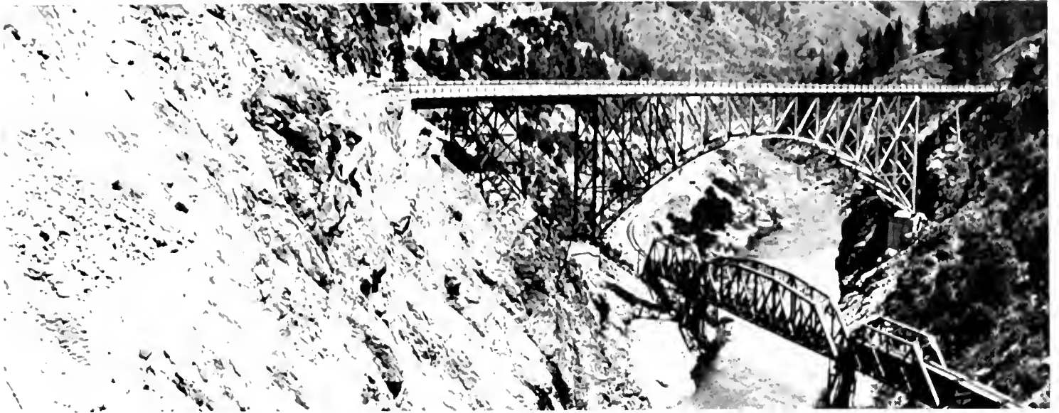
BRIDGES PLAY LEAP FROG—New State Highway crosses Feather River above railroad structure at Pulga.
