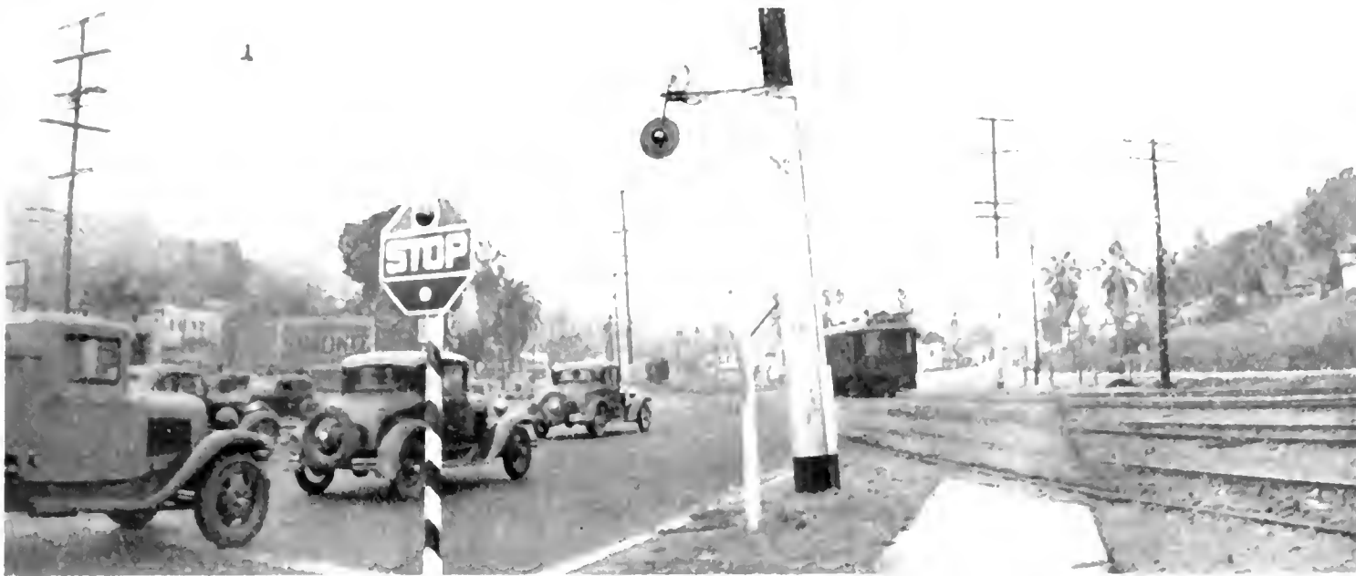
A DANGER SPOT with a high accident record in the city of Los Angeles where Mission Road crosses the Pacific Electric tracks. The tracks will be raised, permitting traffic to pass under them.
