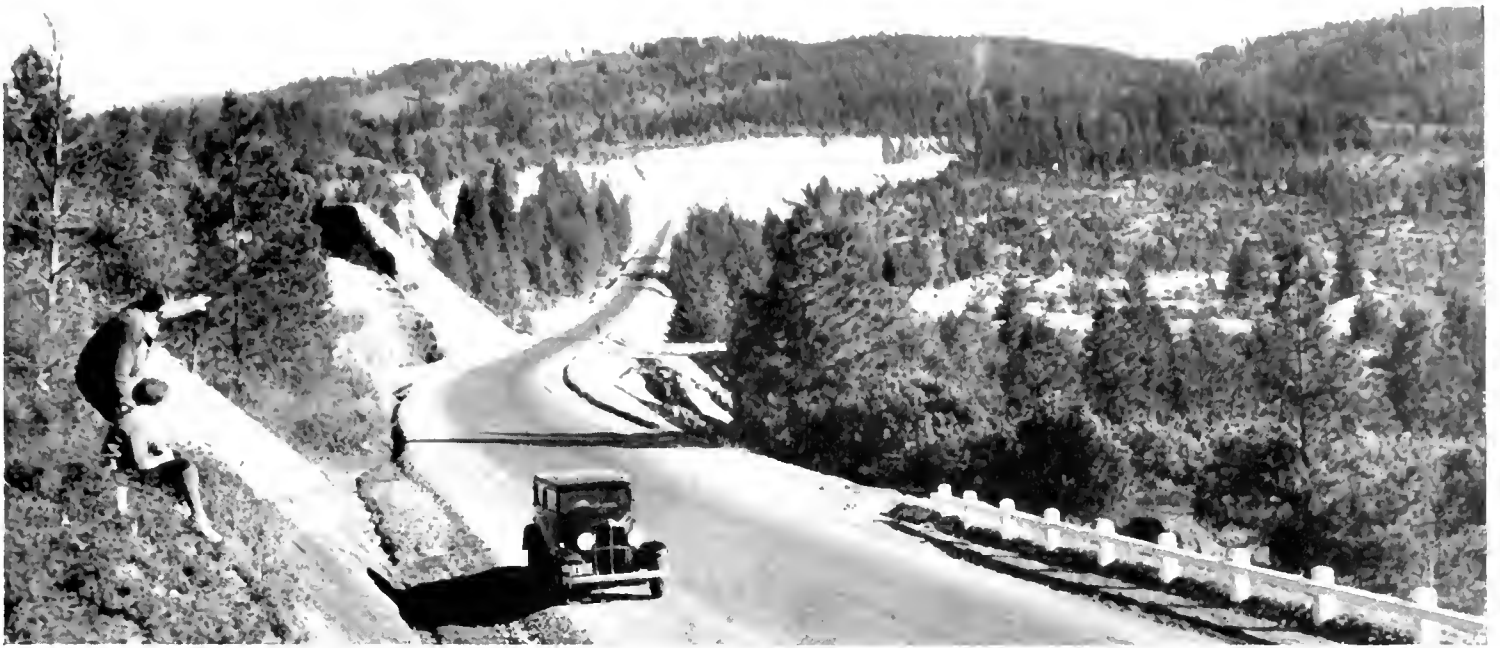
OLD GOLD DIGGINGS are traversed by this portion of the Victory Highway realignment between Gold Run and Airport where hydraulic monitors washed down thousands of dollars worth of "yellow dust."
