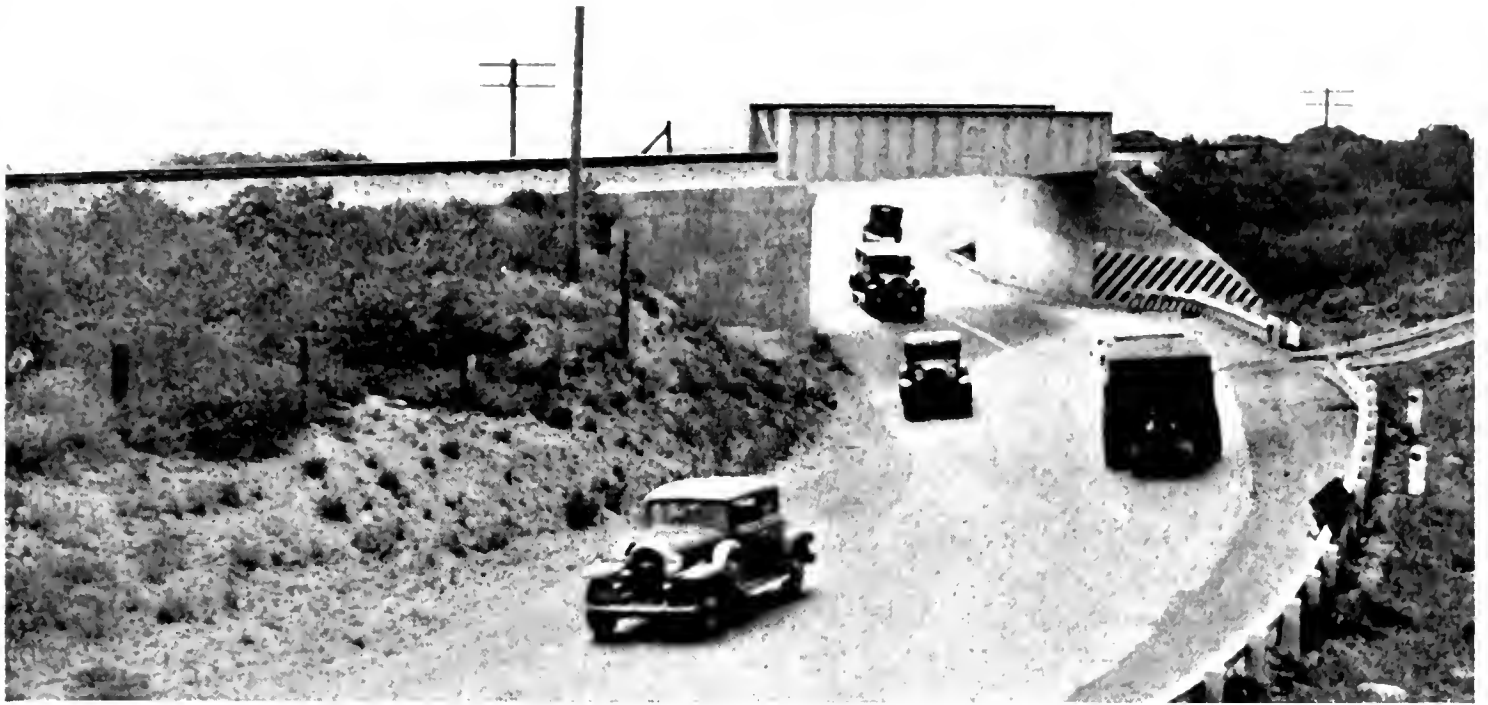
OBSOLETE UNDERPASS, of narrow width and poor visibility that will be eliminated by realignment of the Coast Route north of Ventura.
