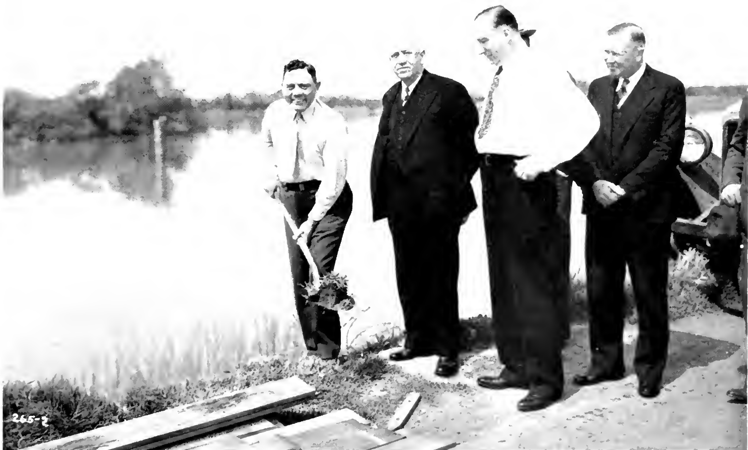
TURNING THE FIRST SHOVELFUL of earth in the groundbreaking ceremonies for the new drawbridge is Harry A. Hopkins, chairman of the California Highway Commission. Others are: Commissioner T. A. Reardon; Director of Public Works Earl Lee Kelly, who also did some shoveling, and District Engineer R. E. Pierce.
