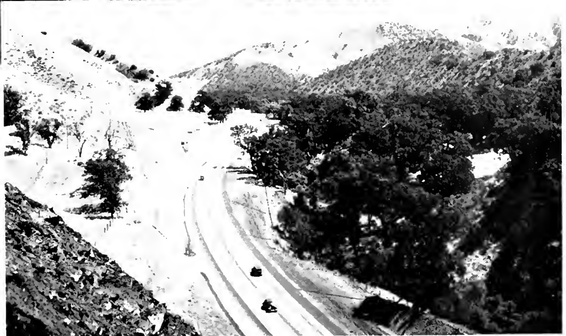
DEADMAN'S CURVE ELIMINATED —At top a picture of the dangerous curve in Grapevine Canyon on the Ridge Route and the narrow old road, a combination that produced many accidents at that point. Beneath, the same scene at the start of construction improvement showing the heavy grading work under way on the relocation project. The next lower picture affords a comparison of the old road and the new wide highway showing Deadman's Curve entirely cut off from traffic use. At bottom, a view of another part of the new, three-lane unit recently completed through this heavily traveled arterial.
