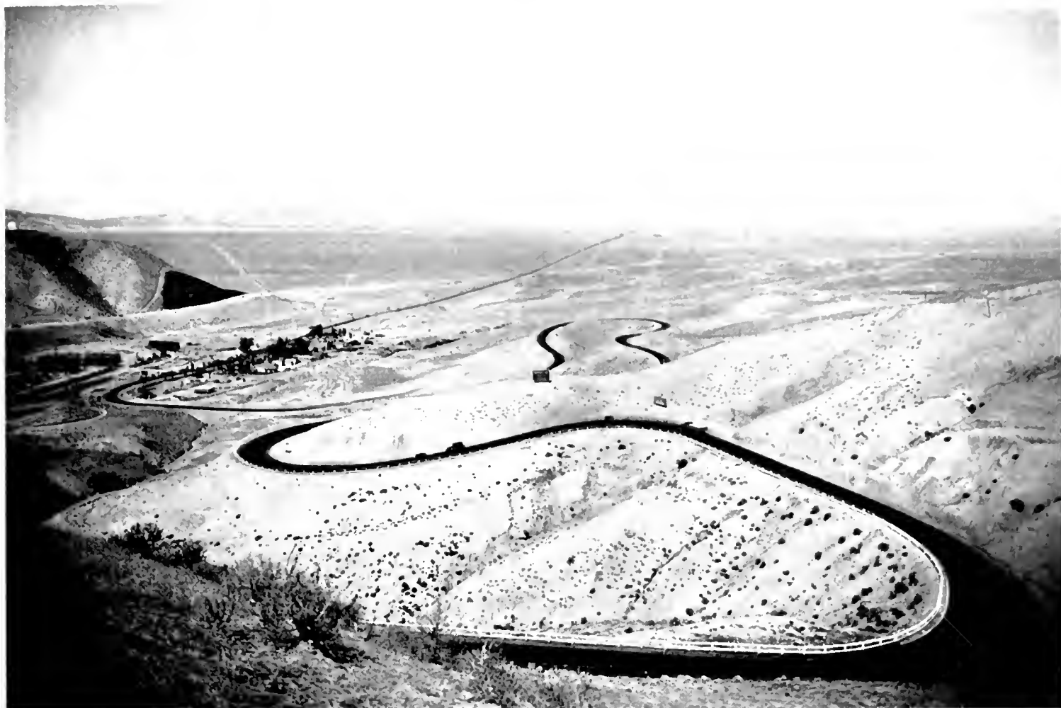
A SINUOUS COURSE with many sharp turns is followed by the existing Grapevine Grade sector of old State highway between Fort Tejon and Grapevine Station on the Los Angeles-Bakersfield arterial. The new alignment soon to be opened is shown at the extreme left center passing a huge slope cut of the high hill and joining the present straightaway to Bakersfield a mile to the north.
