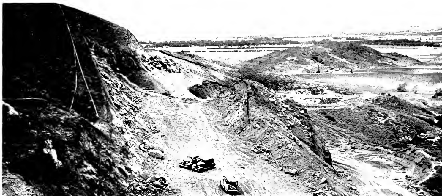
LARGE CUTS AND FILLS on new direct alignment; old winding road at right.
