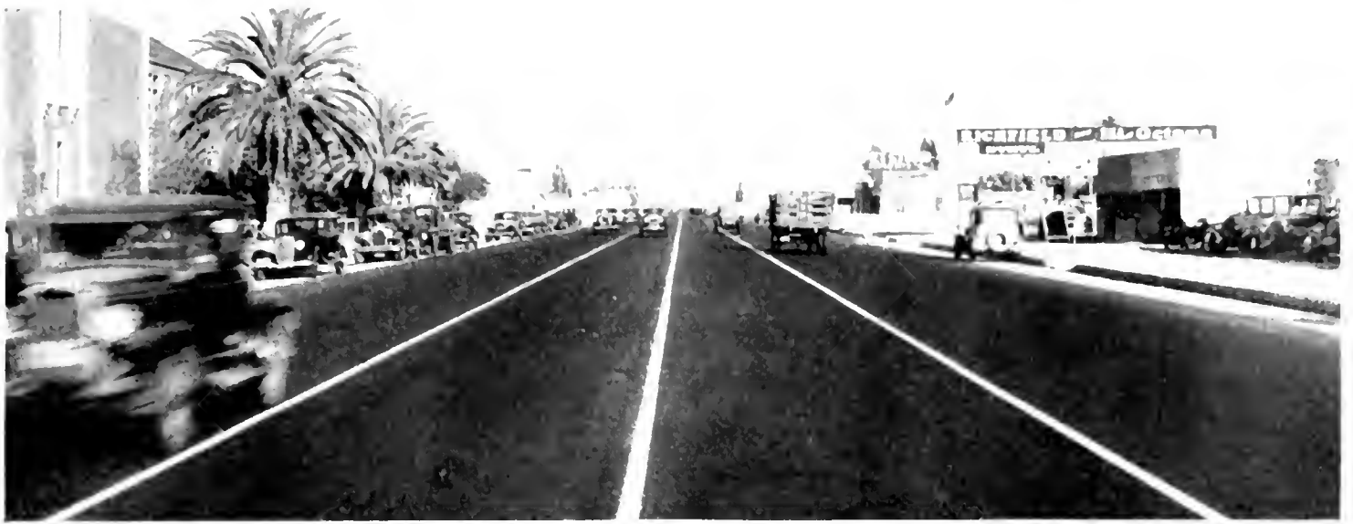
TRAFFIC CONGESTION is eliminated on Firestone Boulevard in the community of Graham, Los Angeles County, by the completion of a fine, four-lane highway, 74 feet wide between curbs.
