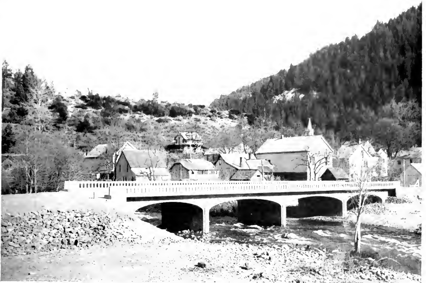
New reinforced concrete girder bridge on realigned State Highway across the North Fork of North Yuba River at Downieville.
