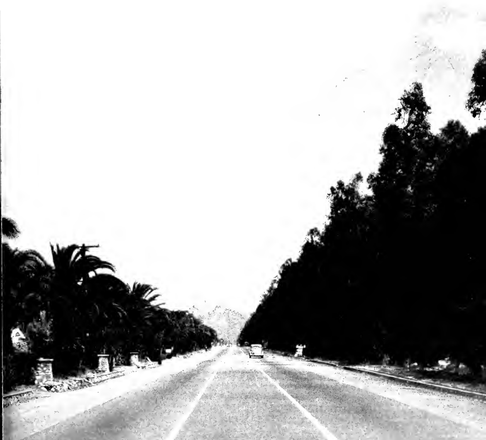
Scene on the new Boulevard, State Route 109 near Los Angeles, looking toward Pittsburg
