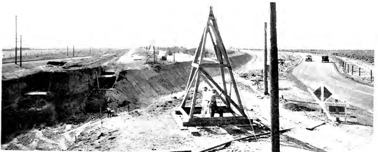
UNDER CONSTRUCTION. Both railroad and highway have been detoured to permit building of the Delano underpass. The new highway alignment, partially graded, is seen following along the cut embankment. Traffic is using the detour at right of picture.
