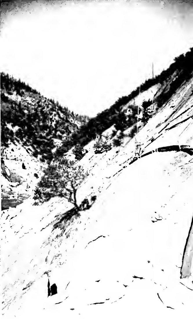
GREAT GRANITE DOMES of Feather River Canyon are being blasted and tunneled by highway engineers. The top picture shows the end of grading at Arch Rock where drilling operations begin. The upper line across the rock is a 4-inch airline for supplying the jackhammers. The other lines provide footholds for the men. Lower left photo shows 9 by 14 foot heading of tunnel No. 1. Outline for the completed tunnel is shown on face of portal. At lower right, men are loading drill holes on steep bare slope.
