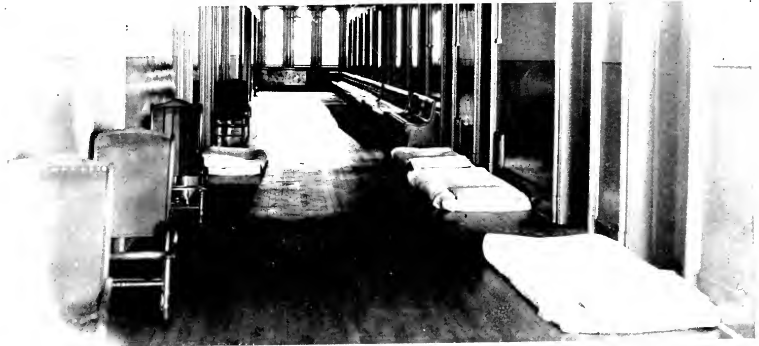
PATIENTS SLEEP ON FLOOR in H. ward, Napa State Hospital, where overcrowding of semi-violent mental cases has reached the point where beds are laid down in hallways.
