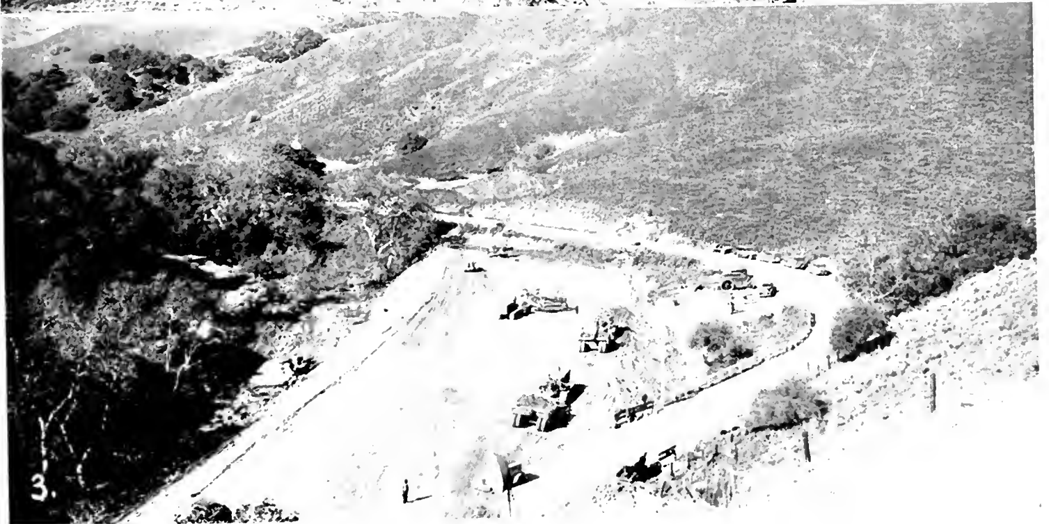
NOJOQUI GRADE REALIGNMENT of U. S. 101 through Gaviota Pass in Santa Barbara County involves some heavy grading, 581,000 cubic yards as shown in pictures 1 and 2 and elimination of 33 curves as in No. 3.
