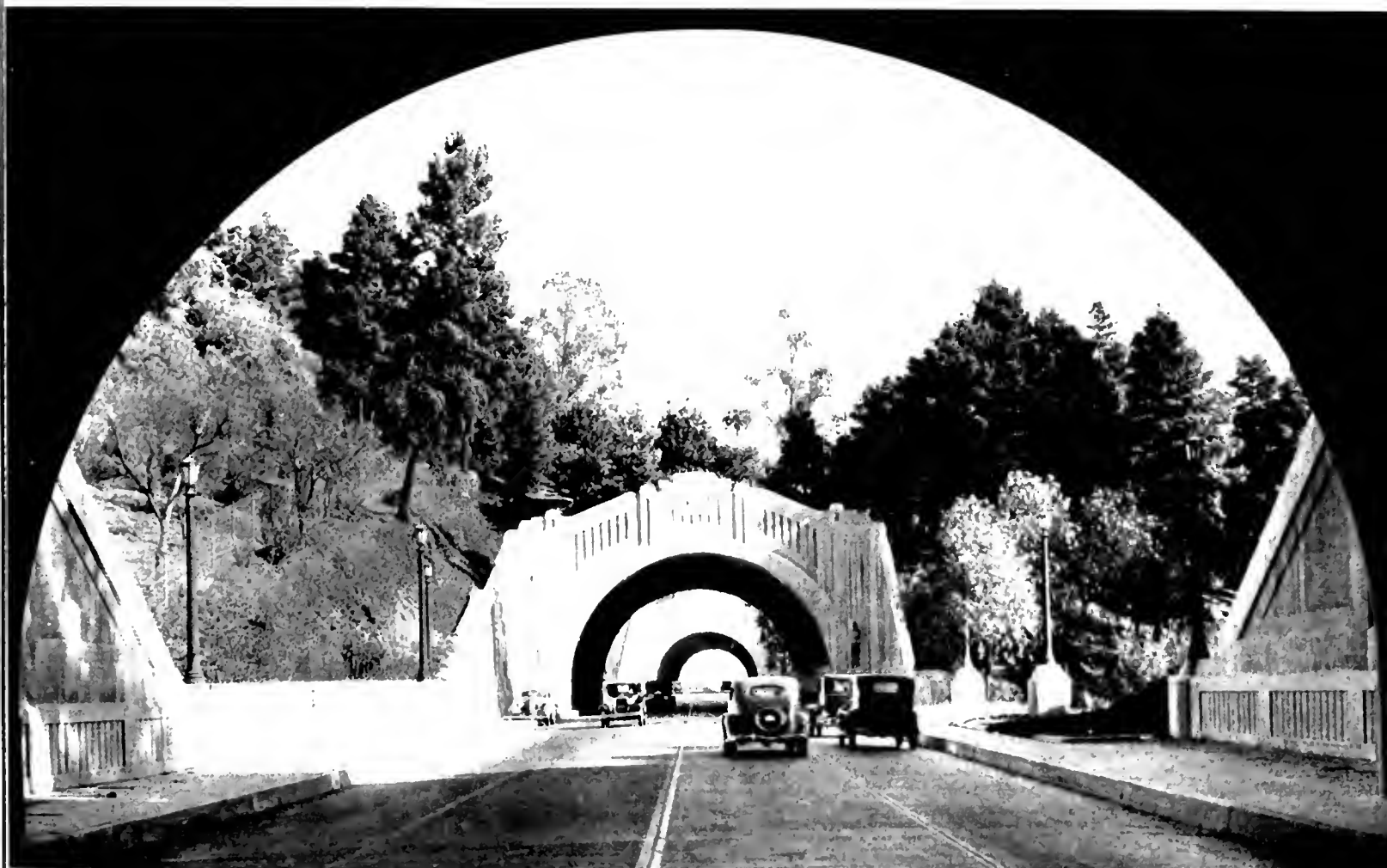
Tunnel Vista showing three completed Figueroa Street bores through park.
