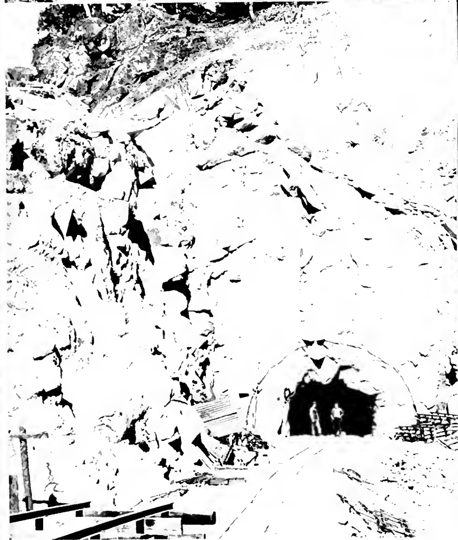
GREAT GRANITE DOMES of Feather River Canyon are being blasted and tunneled by highway engineers. The top picture shows the end of grading at Arch Rock where drilling operations begin. The upper line across the rock is a 4-inch airline for supplying the jackhammers. The other lines provide footholds for the men. Lower left photo shows 9 by 14 foot heading of tunnel No. 1. Outline for the completed tunnel is shown on face of portal. At lower right, men are loading drill holes on steep bare slope.
