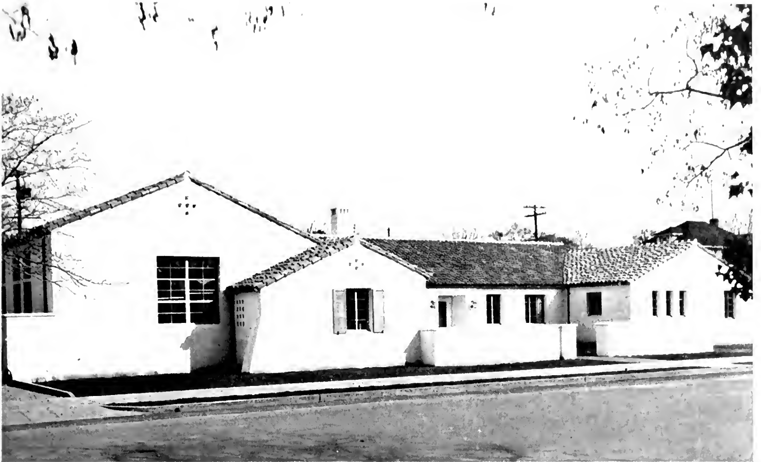
NEW DISTRICT HEADQUARTERS BUILDING in Stockton is a one story reinforced concrete structure 121 x 82 feet located at Center and Rose Streets. It has 11 office rooms in addition to a public lobby, information room, stock room and basement.
