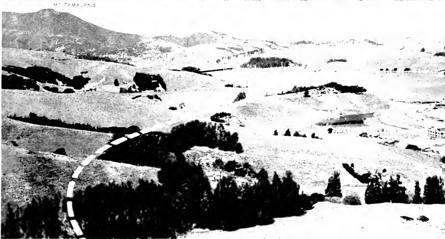
MARIN APPROACH alignment to Golden Gate Bridge through rugged Sausalito hills is shown by dotted lines. At top—Location of tunnel through high ridge. Center—General view of route from Bolinas Street. At bottom—Alignment from present State Highway at Waldo Point and Richardson Bay.
