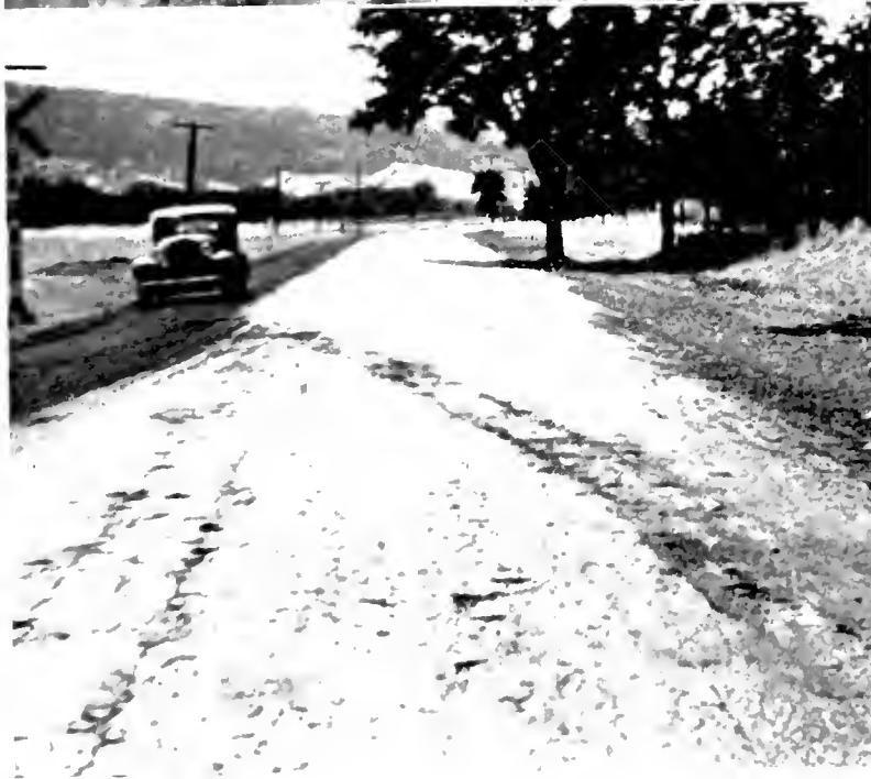
RAVAGES OF A TRACTOR. Upper left—Route 50 between Madison and Brooks, Yolo County. Caterpillar tractor and flanged heavy wheels have torn out and loosened edge of oil mixed pavement. Upper right—Route 50, between Madison and Brooks showing deep cut caused by flange of heavy wheel in bituminous macadam pavement. Lower left—Route 50, between Madison and Brooks where tractor and harvester pulled diagonally across at railroad crossing West of Capay leaving ravelled out track about 14 inches wide. Lower right—Route 50, Yolo County, armor type or bituminous pavement between Brooks and Codannassa approximately 1\frac{1}{2} inches thick where sharp flange of harvester wheel cut off edge of pavement.
