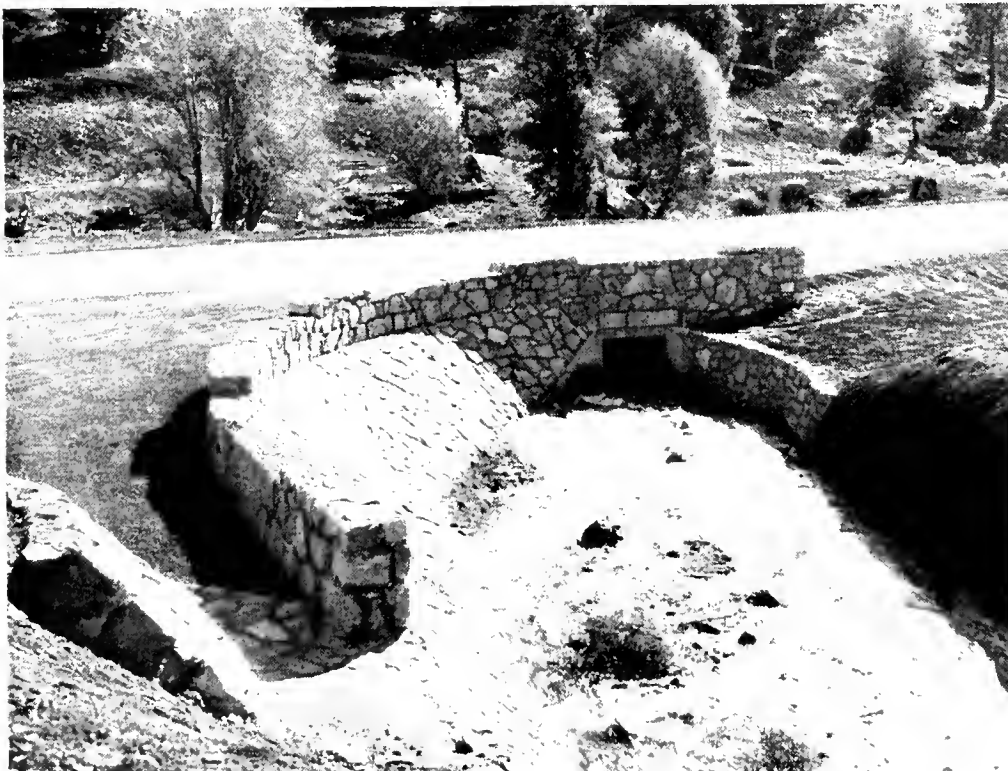
BEAUTIFICATION treatment of culvert and access to brook
