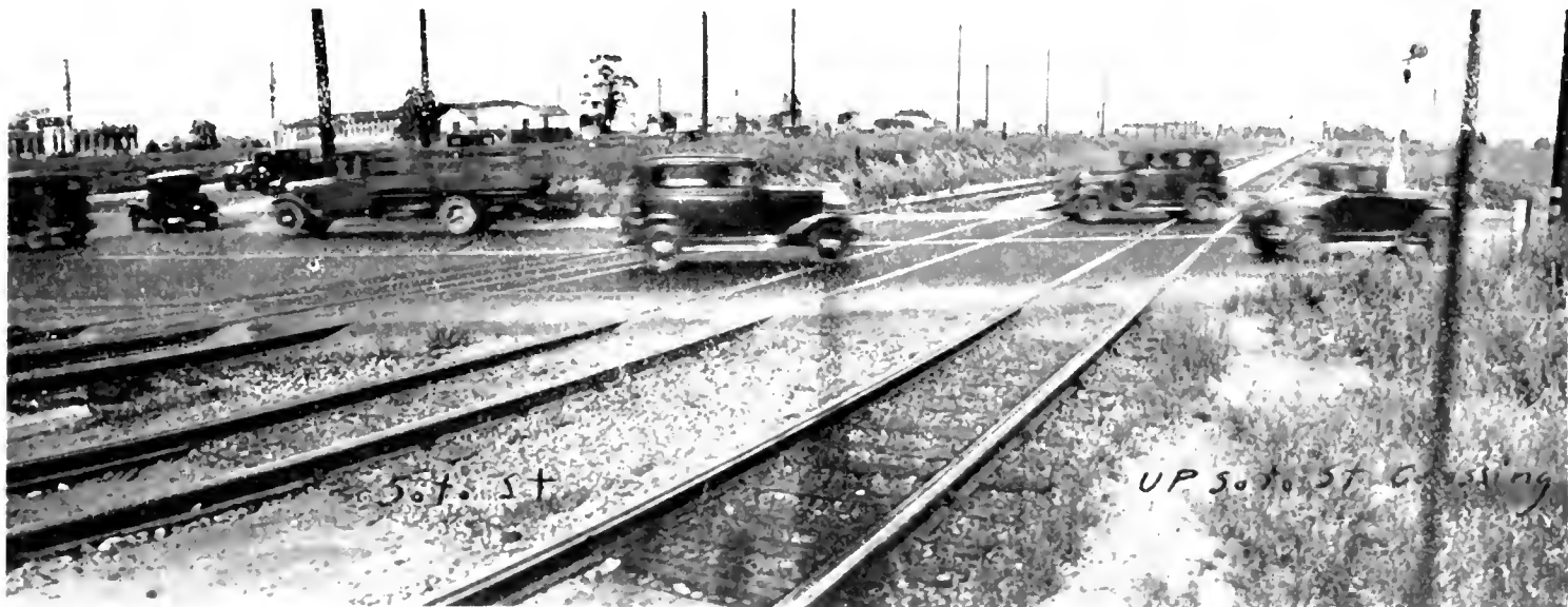
FOUR TRACK CROSSING of the Union Pacific's Main and Butte Street line on Soto Street in the city of Los Angeles. A subway will provide safety for vehicular traffic.
