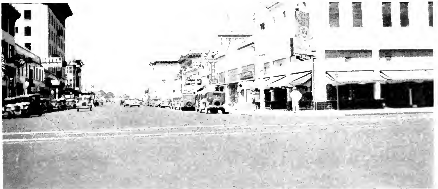
COMPLETED JOB of asphalt concrete pavement at intersection of Fresno street and Broadway.
