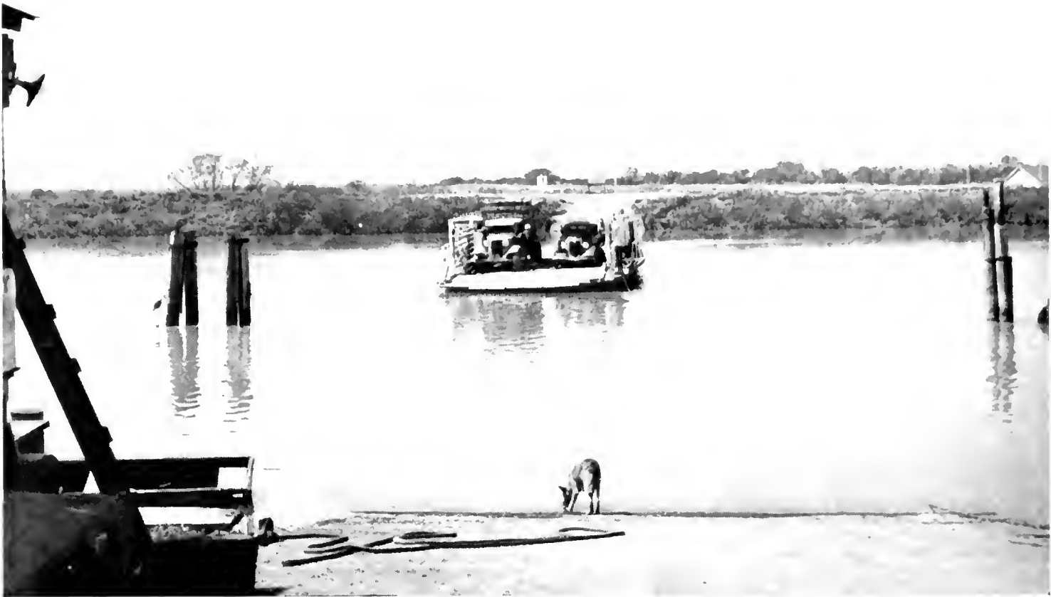
FERRYBOAT ON POTATO SLOUGH soon to be eliminated by modern drawbridge.
