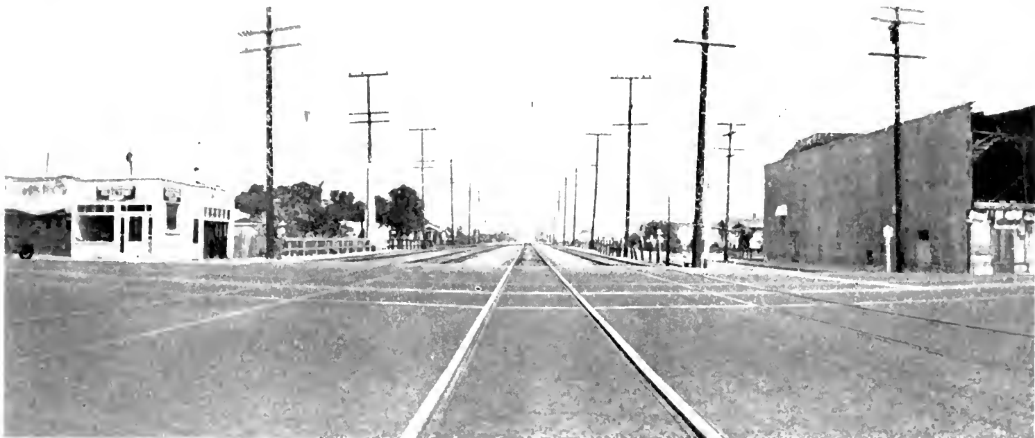
PEAK HOUR PERILS confront motorists at Graham Station on State Route 174 where Pacific Electric interurban trains cross Firestone Boulevard in Los Angeles. The danger will be eliminated by construction of a subway under the tracks.
