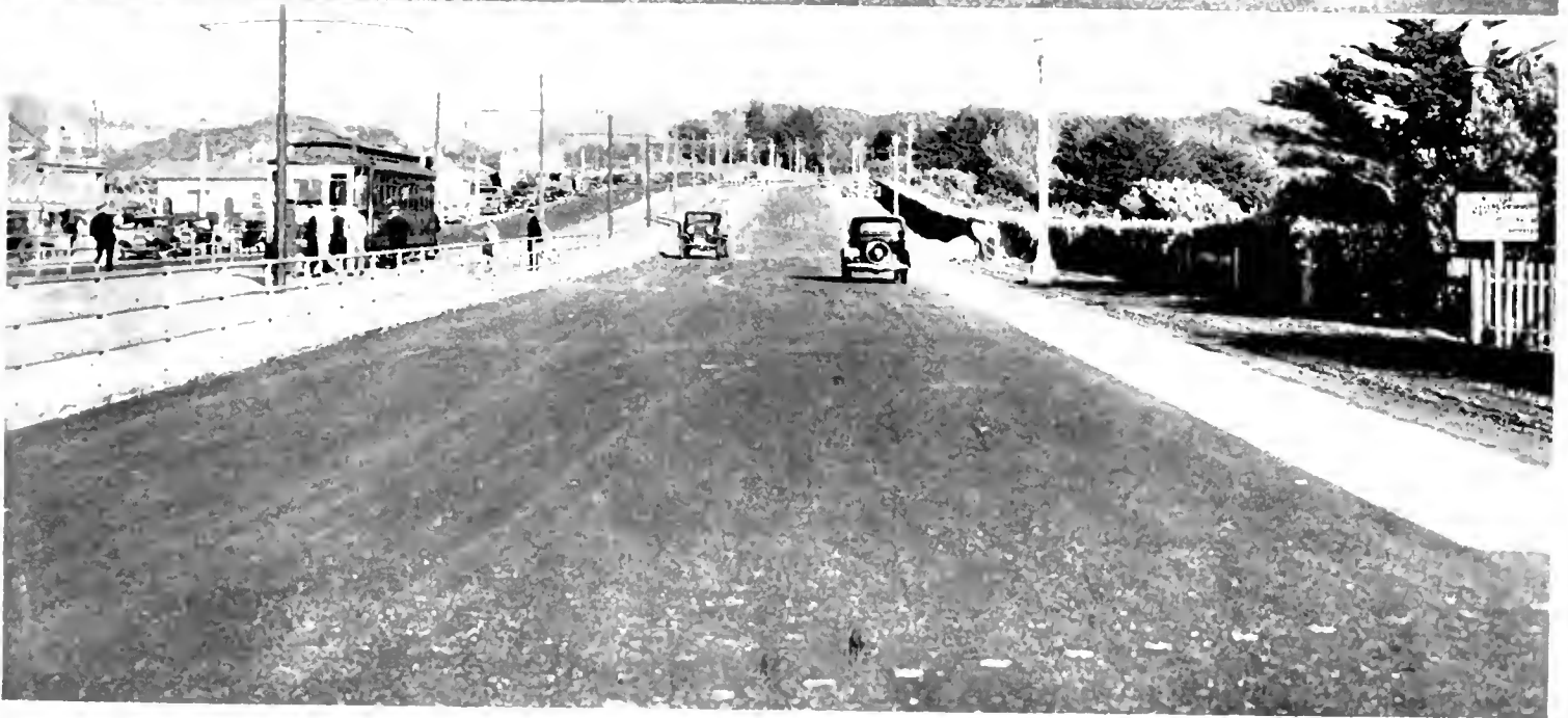
SLOAT BOULEVARD IMPROVEMENT: 1—At top, general view showing 135 foot right of way with one-way traffic on either side of trolley tracks in the center. 2—North side of highway at point opposite Fleishhacker Zoo and pool showing subway entrance to Municipal Beach. 3—South side of Sloat Boulevard Improvement at Beach Subway opposite entrance to Fleishhacker Pool.
