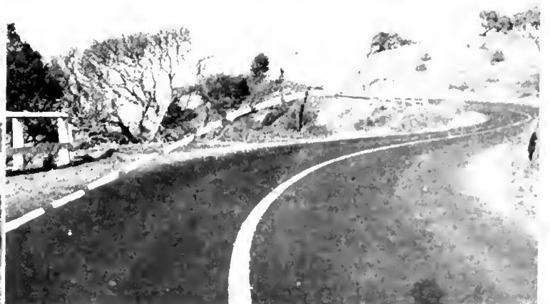
SOME 48 CURVES, mostly sharp ones, as shown in the top picture, distinguish the 3.3 miles of Pacheco Pass road from the summit easterly to the foot of the grade. New alignment indicated by dotted lines in the lower views will eliminate all short radius turns, widen the roadway and lessen grades. The historic San Luis adobe ranch house, 105 years old is shown at bottom.
