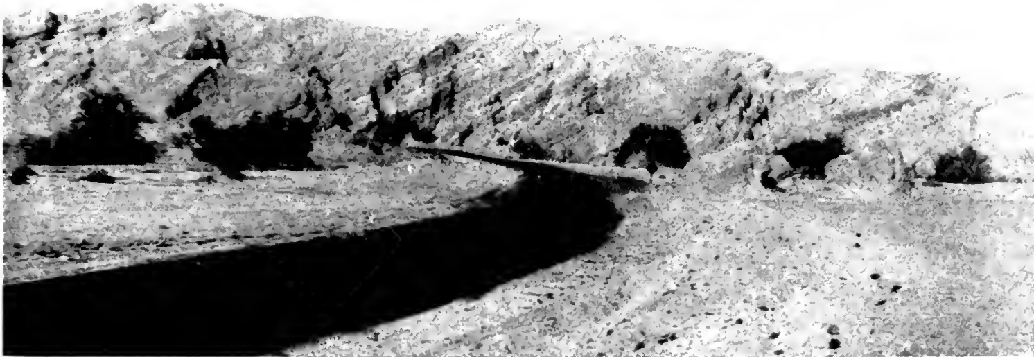
BEFORE AND AFTER THE FLOOD. The above pictures show two sections of the 7-mile stretch of highway in Box Canyon, Riverside County, that was entirely destroyed by a cloudburst storm on August 23d last and the restored highway as completely graded and surfaced on new location and better alignment and opened to traffic in 42 days.
