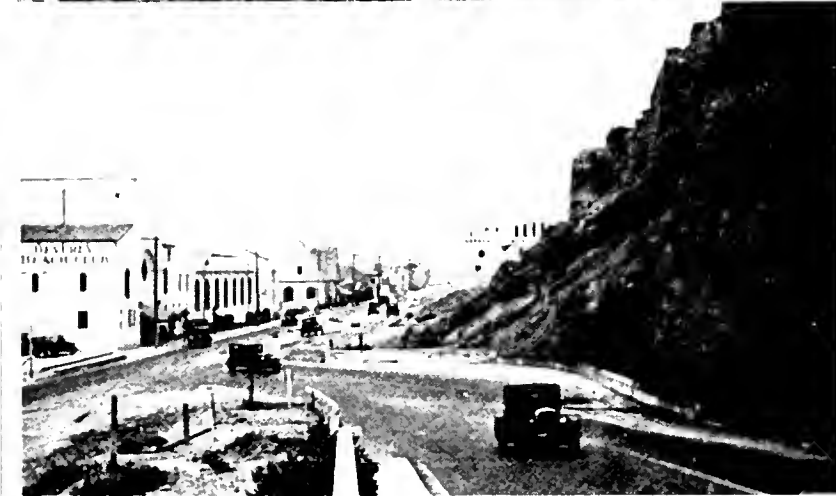
FROM BOTTLENECK TO BOULEVARD—Improved link of State Highway No. 60 at Santa Monica along the coast below the Palisades, now a fine four-lane highway is pictured at top. The old 20-foot pavement with the widening operation under way is shown in center picture, and below are “before” and “after” views of the California Avenue Incline connection.
