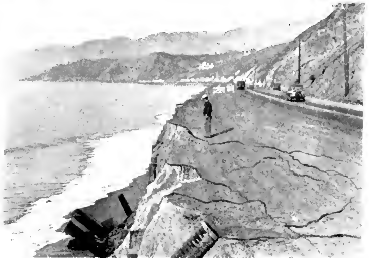
OLD OCEAN HARNESSED by groins has been toiling for State highway engineers building a fine sandy beach along the Santa Monica Coast where no beach existed. In 20 months it has made a beach a mile long and 200 feet wide as shown by shaded portions of the drawing by Artist Phil Leonard of the Los Angeles Times. It provides a public bathing beach as well as a protection to the highway. Photo shows how the waves were gouging out the highway shoulders before groins were installed.
