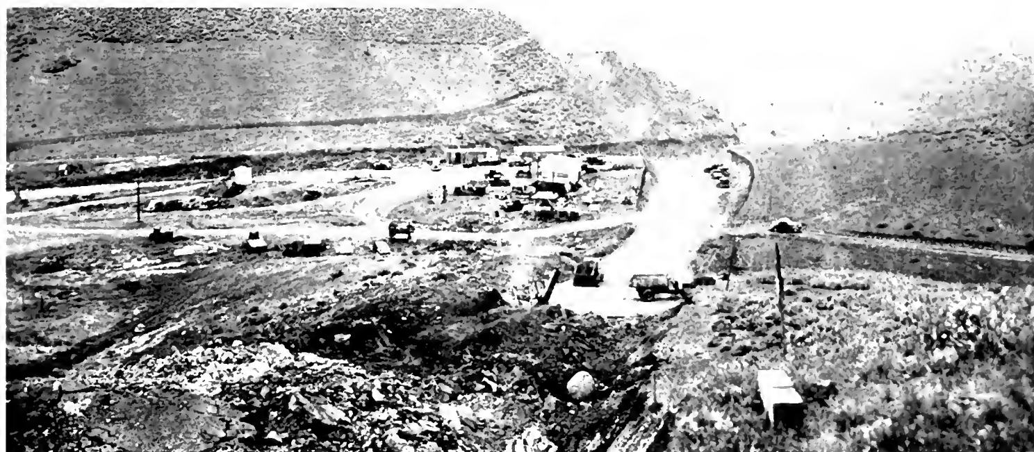
CUTS BEING OPENED UP on new line which crosses old road in center at right angles.
