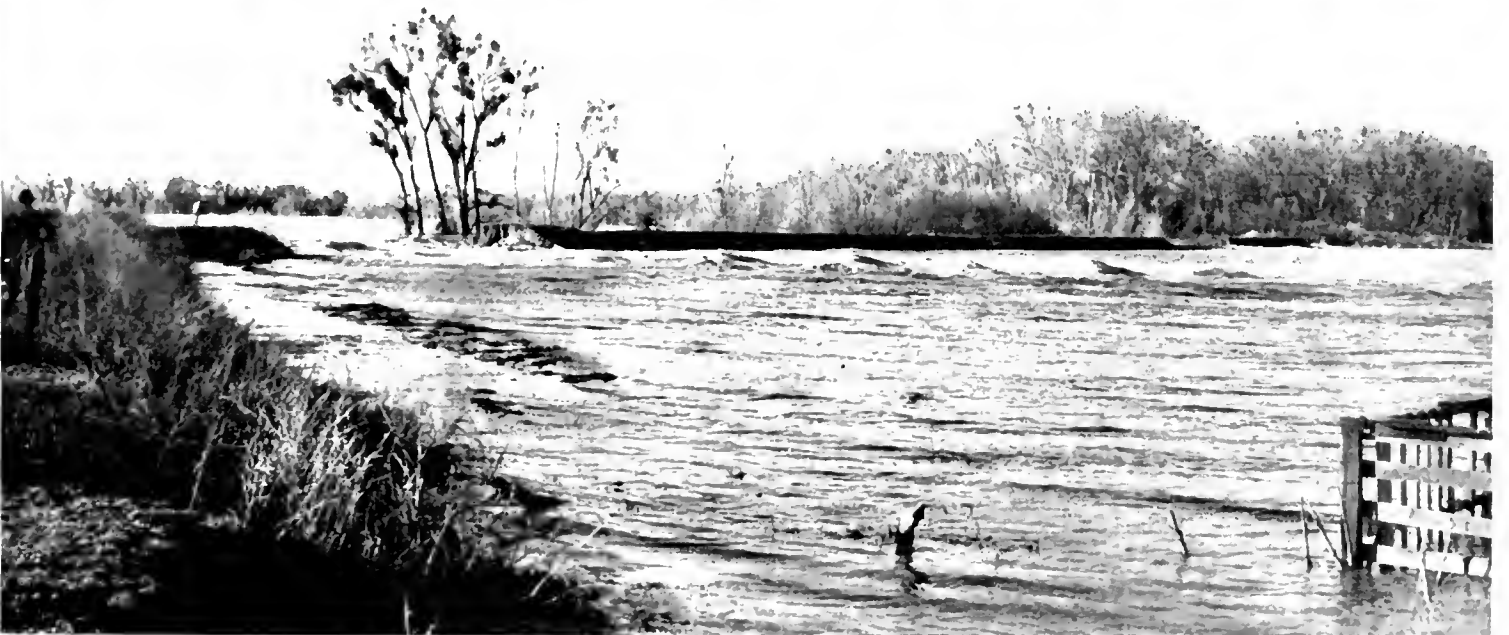
OVER THE TOP of a low levee and through a resulting breach went flood waters of the Sacramento River near Colusa in the January storm. The levee had not been completed to grade and was weakened by rodent holes. In top picture State Engineer Edward Hyatt (left) and Col. A. M. Barton, manager of State Reclamation Board are examining the break, of which different views are shown below.
