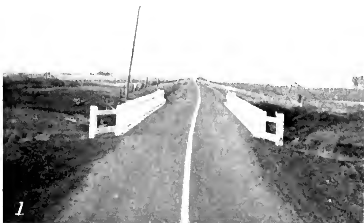
TYPICAL OF BRIDGE DETERIORATION to the danger point when taken into the secondary system was the high span across Jughandle Creek on the Mendocino shoreline coast road shown in the three top pictures. It was a combination wood and steel deck truss structure with bad approach alignment and wooden roadway shown in Nos. 4 and 5. No. 3 is a closeup of one of the lower chord joints seriously weakened by rusting of the metal. The State has made temporary repairs by adding strengthening supports. Pictures 1 and 2 show the old timber trestle on Route 101 between Dixon and the Rio Vista-Fairfield road before and after being taken over by the State.
