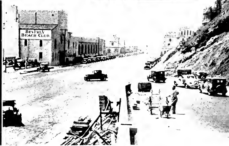
FROM BOTTLENECK TO BOULEVARD—Improved link of State Highway No. 60 at Santa Monica along the coast below the Palisades, now a fine four-lane highway is pictured at top. The old 20-foot pavement with the widening operation under way is shown in center picture, and below are “before” and “after” views of the California Avenue Incline connection.
