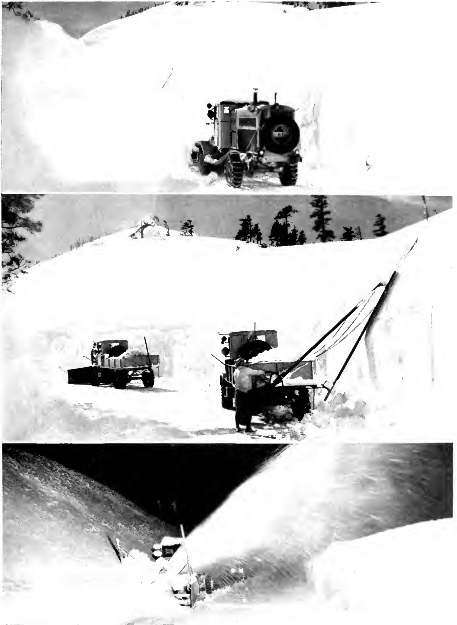
FIGHTING SNOW ON DONNER SUMMIT section of U. S. 40 kept all equipment busy day and night throughout February. At top, an auger blower type rotary plow hurling snow high over bank. Center, spud type push plow and truck with slope slice bar attachment widening roadway, and below, an auger blower working at night.
