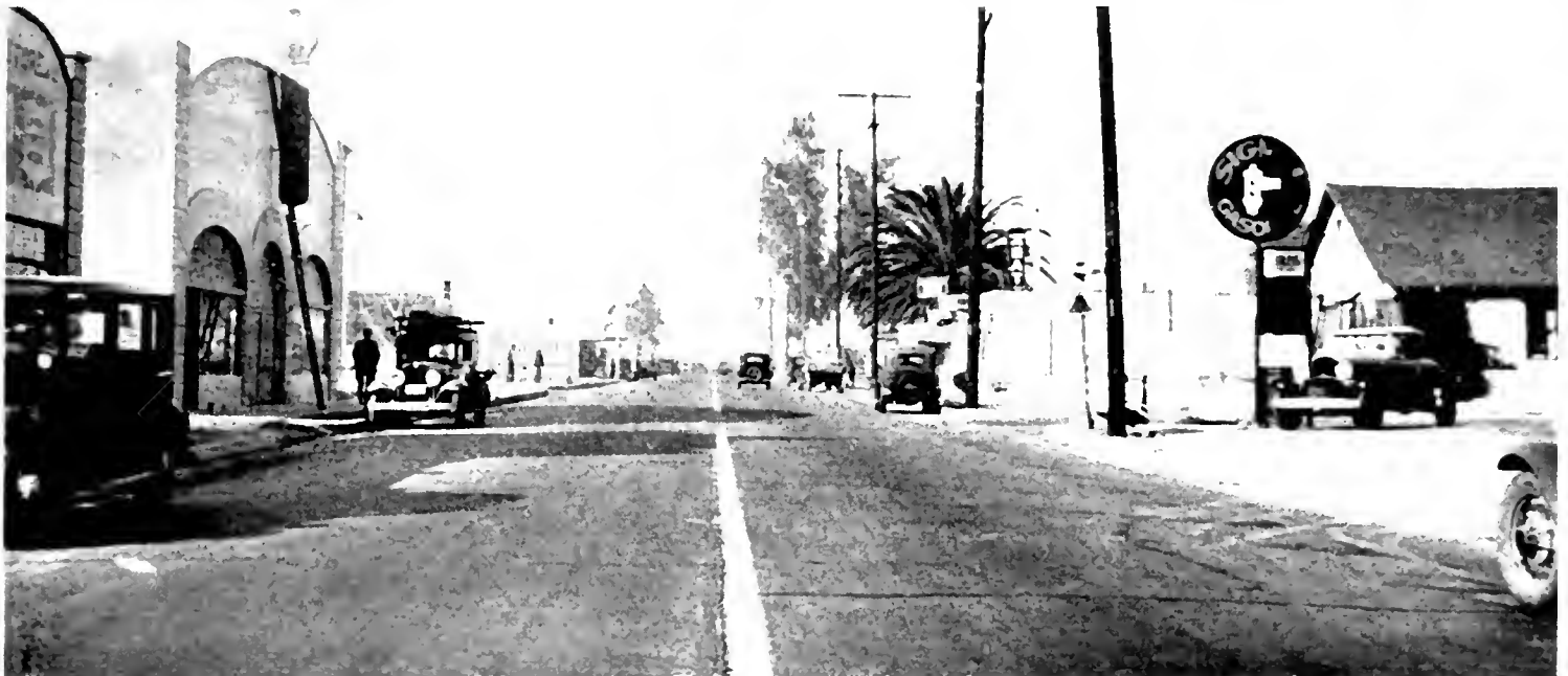
OLD BOTTLENECK CONDITION as it existed before the improvement is shown above. The old pavement was only 40 feet wide, much too narrow for the heavy traffic on this route. The section recently completed is 1.49 miles in length and has a right of way with 100 feet for the entire distance.
