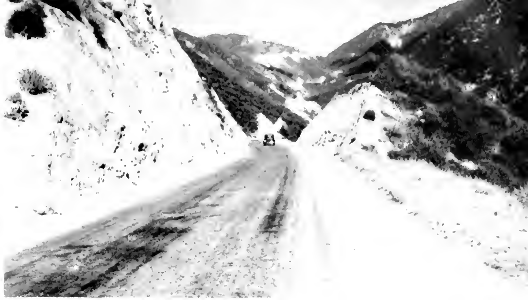
GRADING OPERATIONS call for 914,000 cubic yards of roadway excavation, 5,000,000 yards overhaul.
