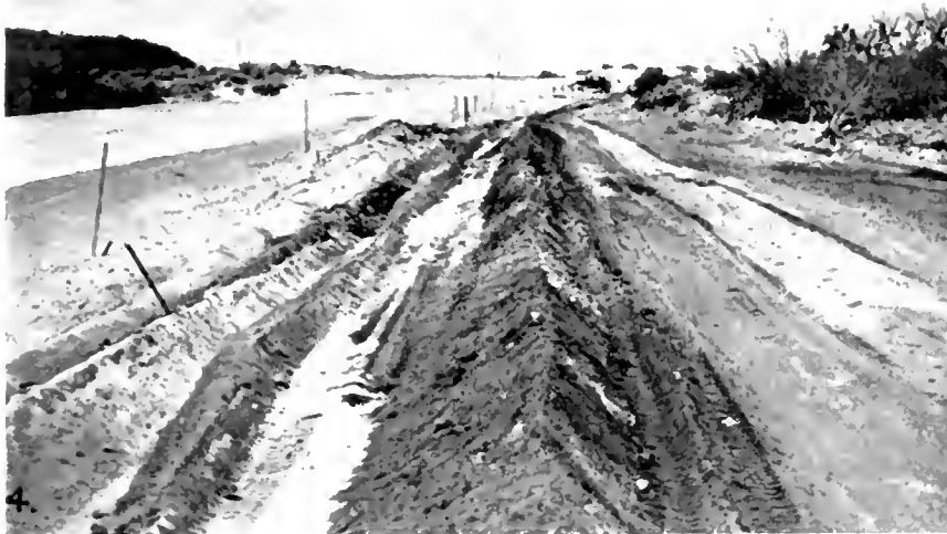
INDIO-PALM SPRINGS REALIGNMENT. 1—The San Jacinto "Angel" as seen from the main highway north of Palm Springs (Frashear Photo). 2-3—The new alignment eliminates several short, dangerous curves. 4—New grade on left composed of local, sandy soil and detour on right in course of construction. 5—Transportation conditions as they are at present in the date garden and orchard districts on this section of highway.
