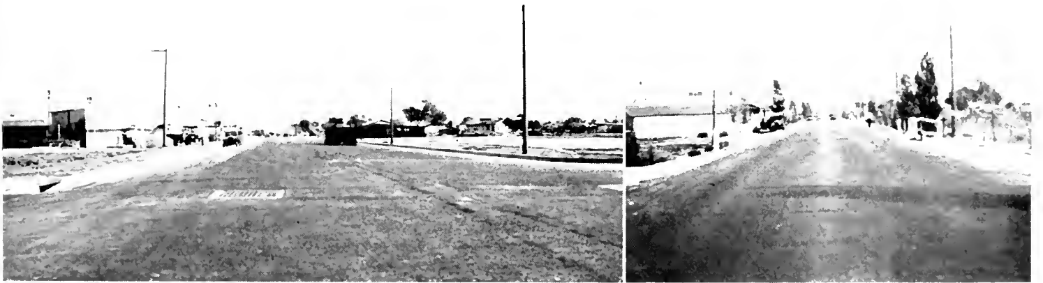
BEFORE AND AFTER views of the improved link of State highway through the city of Anaheim. At left is the newly paved and widened North Los Angeles Street, now a fine broad thoroughfare. At right is the old street narrowed by encroachments and obstructions.
