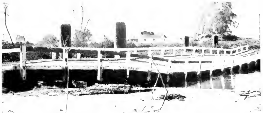
WASHED OUT DETOUR BRIDGE over Kings River east of Centerville on State Route 41.
