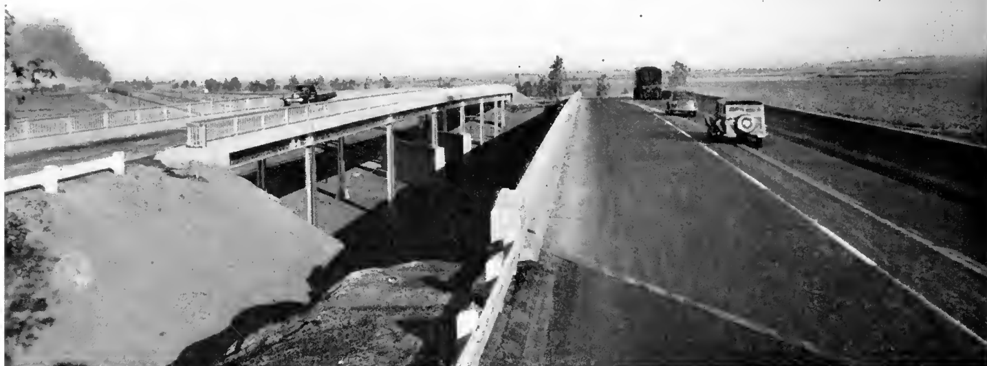
Looking northerly from south end of existing overpass at main line tracks of the Southern Pacific. New structure is on the left
