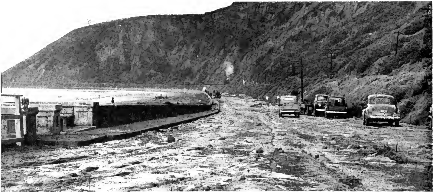
UPPER—View looking northwesterly from Seacliff, showing storm damage of October 18, 1934. LOWER—View looking northwesterly from approximately same location, taken August, 1949, showing completed four-lane divided highway
