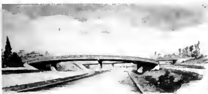
PORTAL STRUCTURE THIRD STREET SOUTHBOUND RAMP
