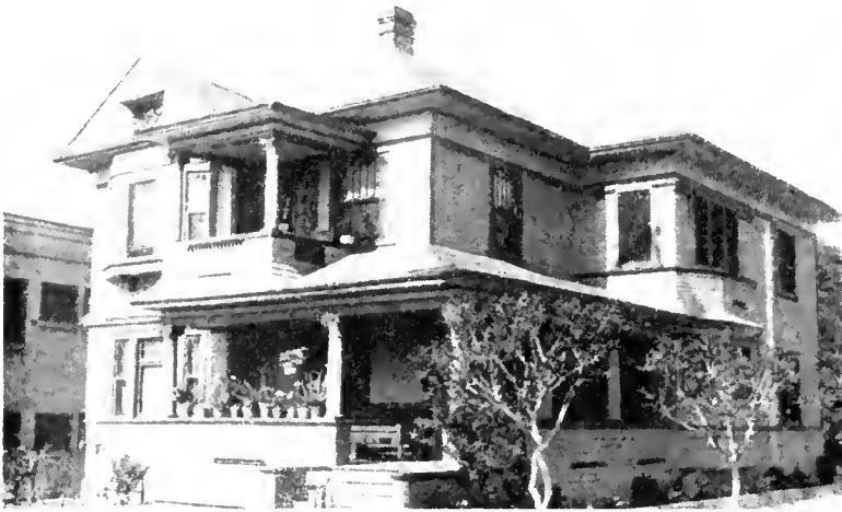
BEFORE —The old-fashioned structure pictured above was formerly located at 439 North Belmont Street. It was removed to allow construction of the Hollywood Freeway.
