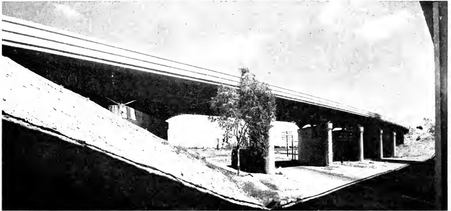
Old structure built in 1933 has solid concrete rail, curved bottom chord girders and heavy concrete piers built to skew of railroad track
