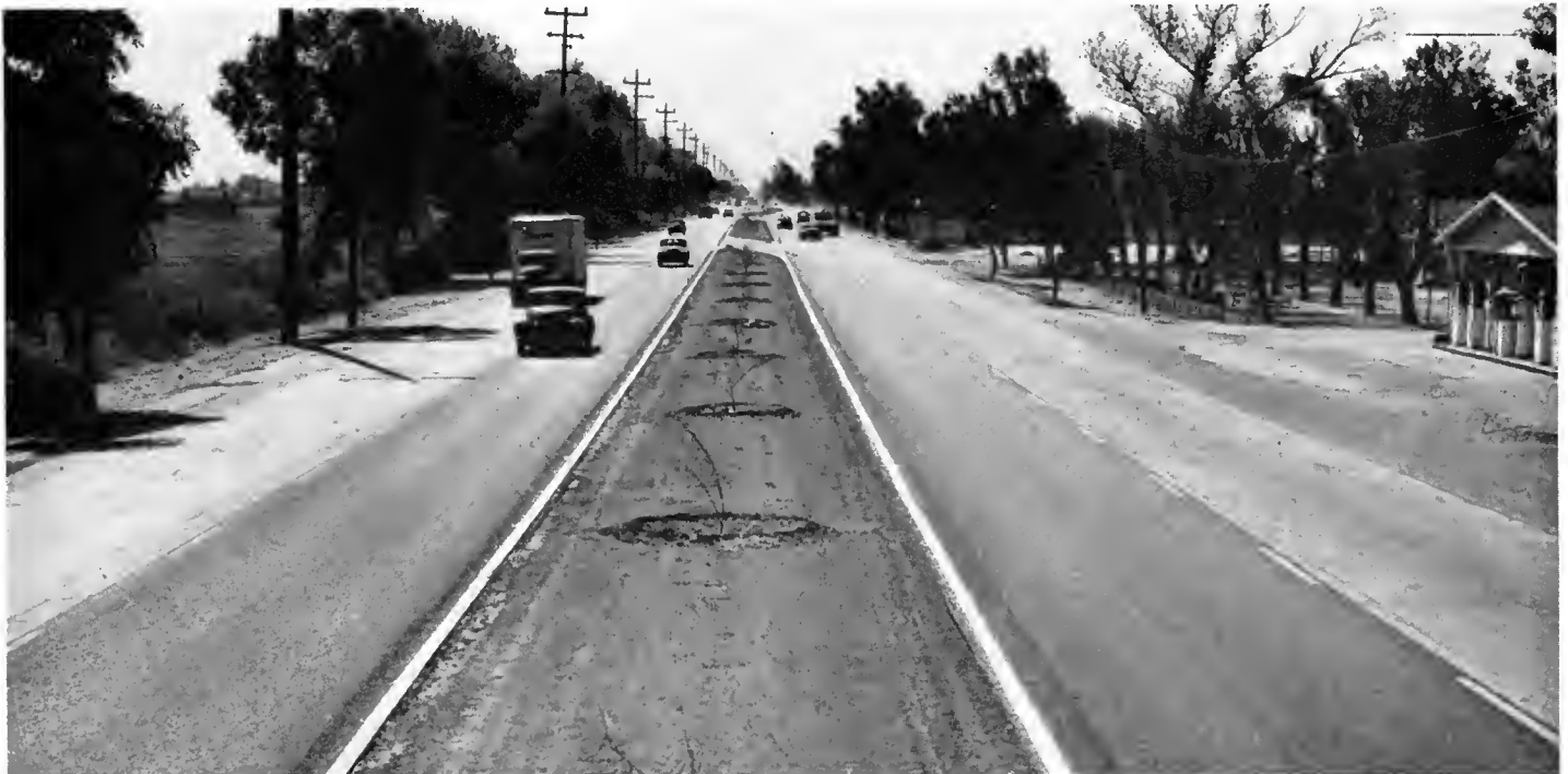
View southerly from about three miles south of Bakersfield. South Chester Avenue, chonnelized and signalized intersection in the center background
