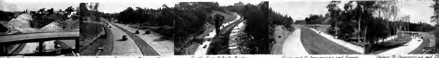
Pascoe St. Overcrossing
