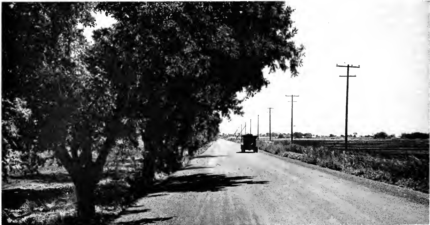
Section of new FAS Route 1156 in Yolo County looking north from State Route 99 about one-half mile east of Greendale
