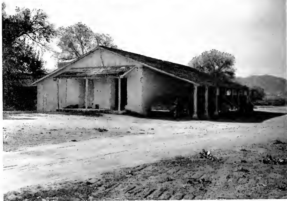
UPPER—Grading operations for relocation of U. S. 395 in the Elsinore Mountains. LOWER—Old adobe depot of Butterfield Overland Stages at Temecula, converted to grain storage warehouse
