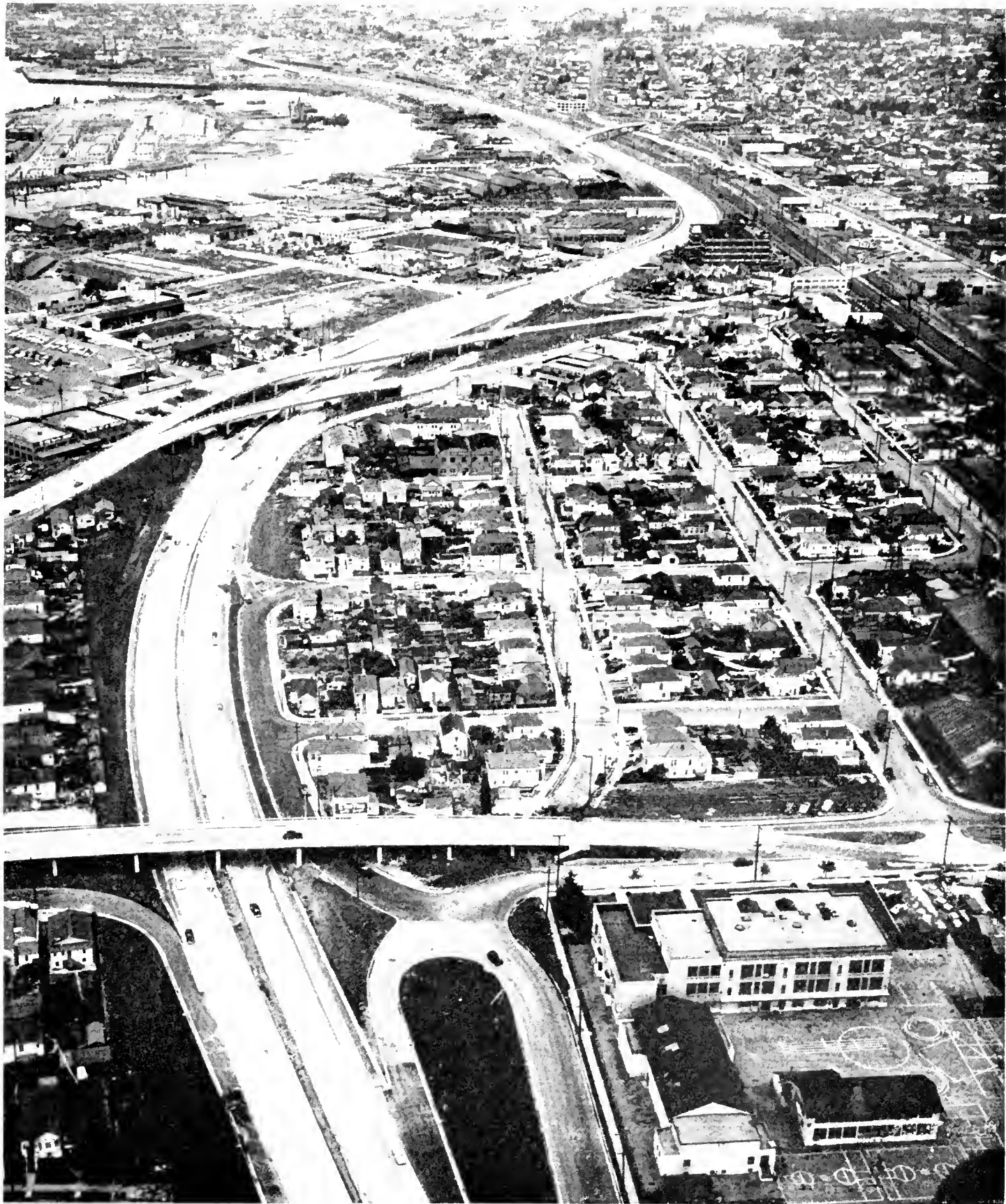
Eastshore Freeway looking north, showing 29th Avenue Overpass in foreground, 23d Avenue divided overpass in center of picture, and 19th Avenue Overhead in background
