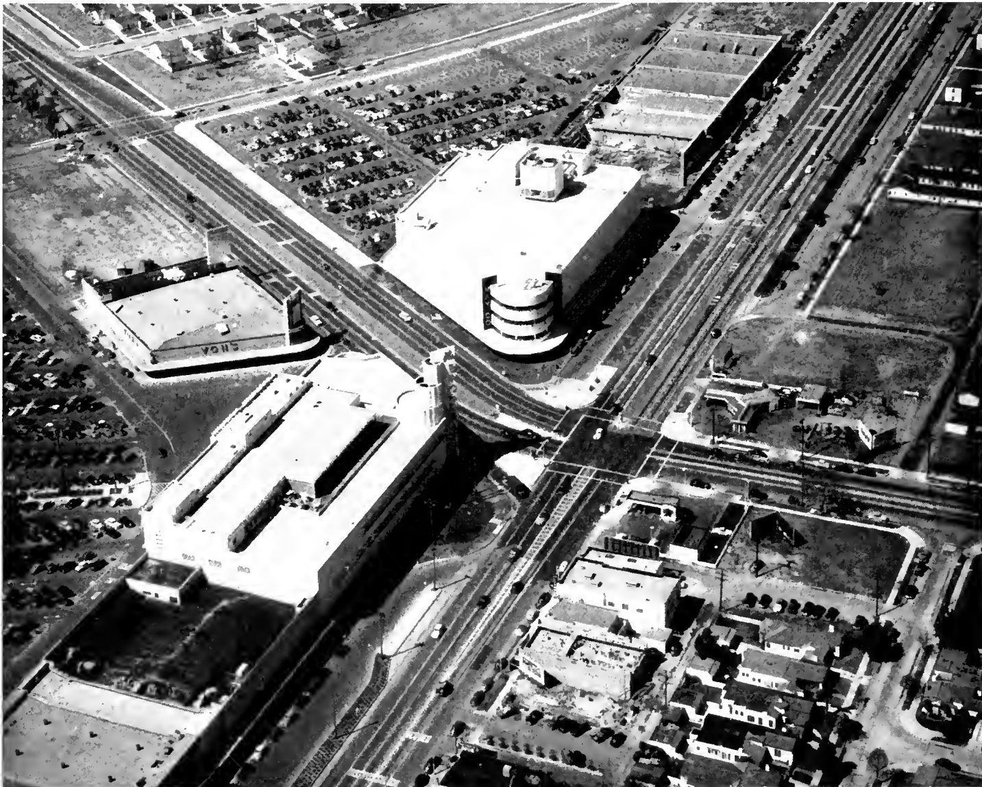
Photo C—Aerial view looking westerly showing development at intersection of Santa Barbara Avenue and Crenshaw Boulevard.—Photo by Nickerson
