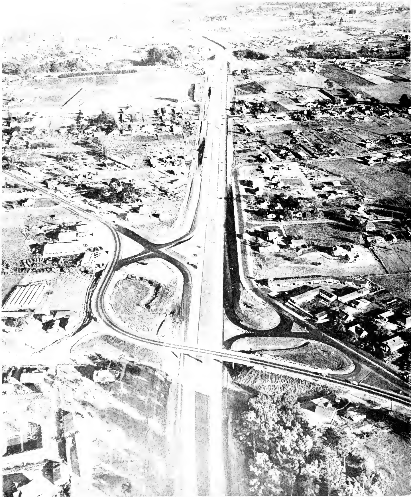
This aerial photograph shows the Soquel Road overcrossing and Paul Sweet Road interchange
