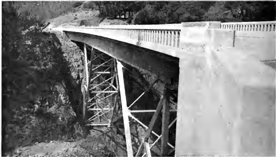
Upper—Approach to new Rock Creek Bridge, looking north. Lower—Looking north at downstream side of span
