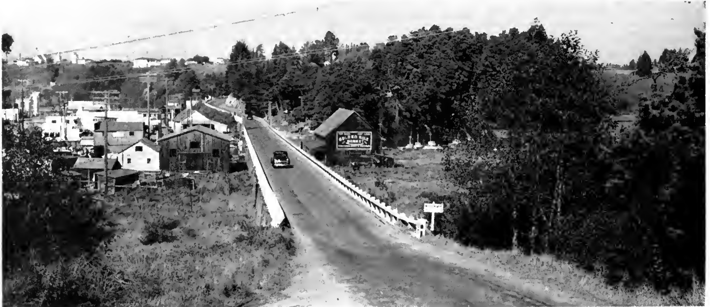
Old Noyo River Bridge which is replaced by new span
