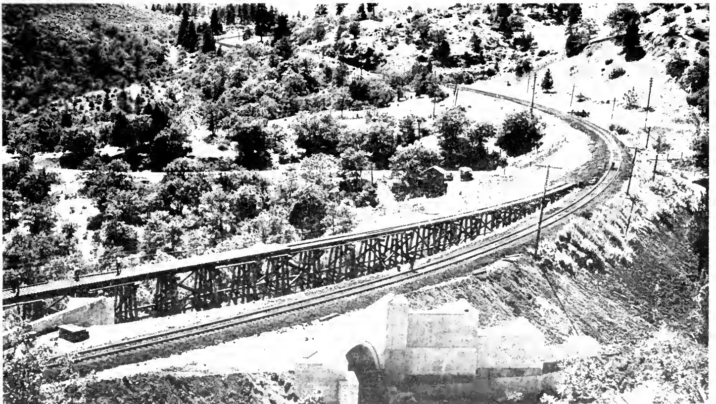
Looking westerly along the railroad track across the barrel of the Bailey Hill Underpass. The existing highway and underpass are in the background
