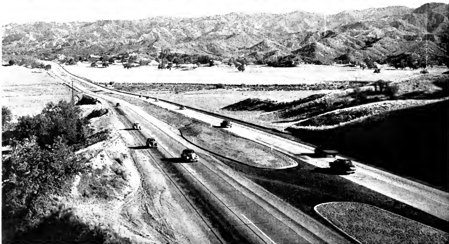
Upper—Completed construction on the Ridge Route near Pico Canyon, showing treatment to prevent haphazard crossings of central division strip between new pavement on right and old pavement on left. Lower—Completed construction on Ridge Route of Pico Canyon showing treatment of connection between new pavement on right and old pavement on left of central dividing strip
