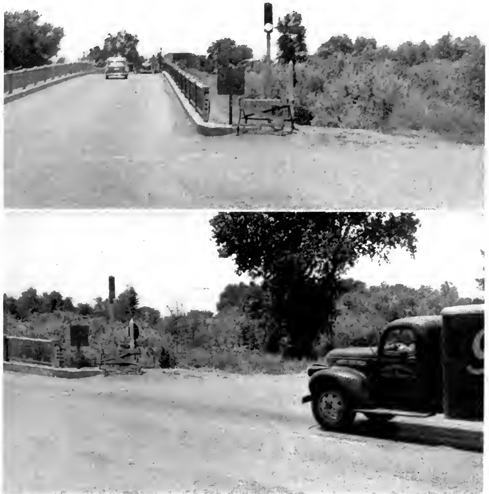
These photos show traffic signals used in one-way traffic control on Knights Landing Bridge
