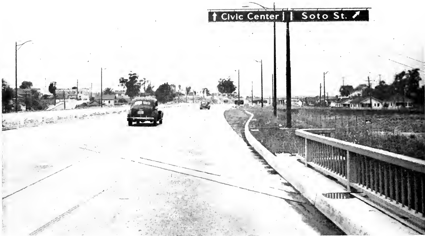
UPPER—View westerly along Santa Ana Freeway from Olympic Freeway grade separation bridge. LOWER—View easterly along the Santa Ana Freeway from near Grande Vista Street, showing Larena Street grade separation bridge
