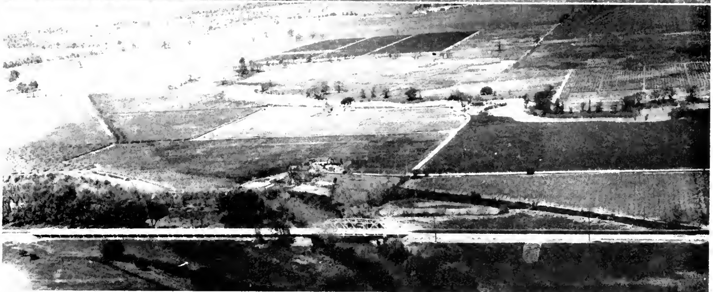
UPPER—This view looking northeast shows new bridge and portion of span across Mokelumne River
