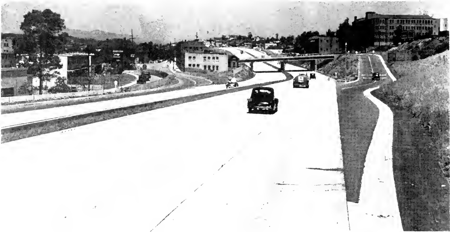
Santa Ana Freeway, looking northerly, showing Fourth Street Overpass grade separation with First Street Underpass in distance
