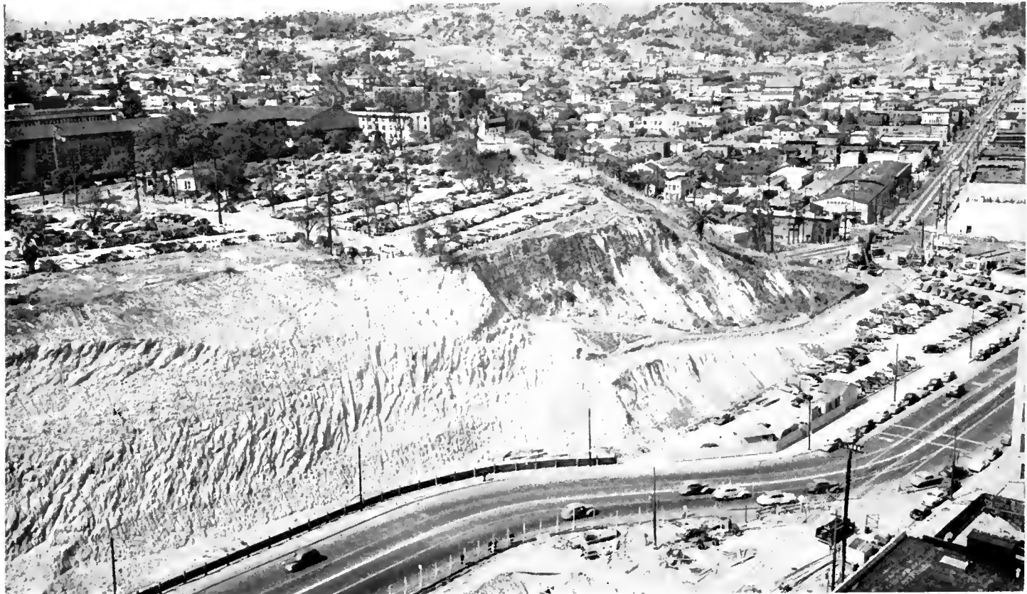
North end of Fort Moore Hill. Barricade erected by contractor along Spring Street detour to catch falling rock and dirt is shown in left foreground. Right center shows resident engineer's office, contractor's offices, construction yard and county parking ground
