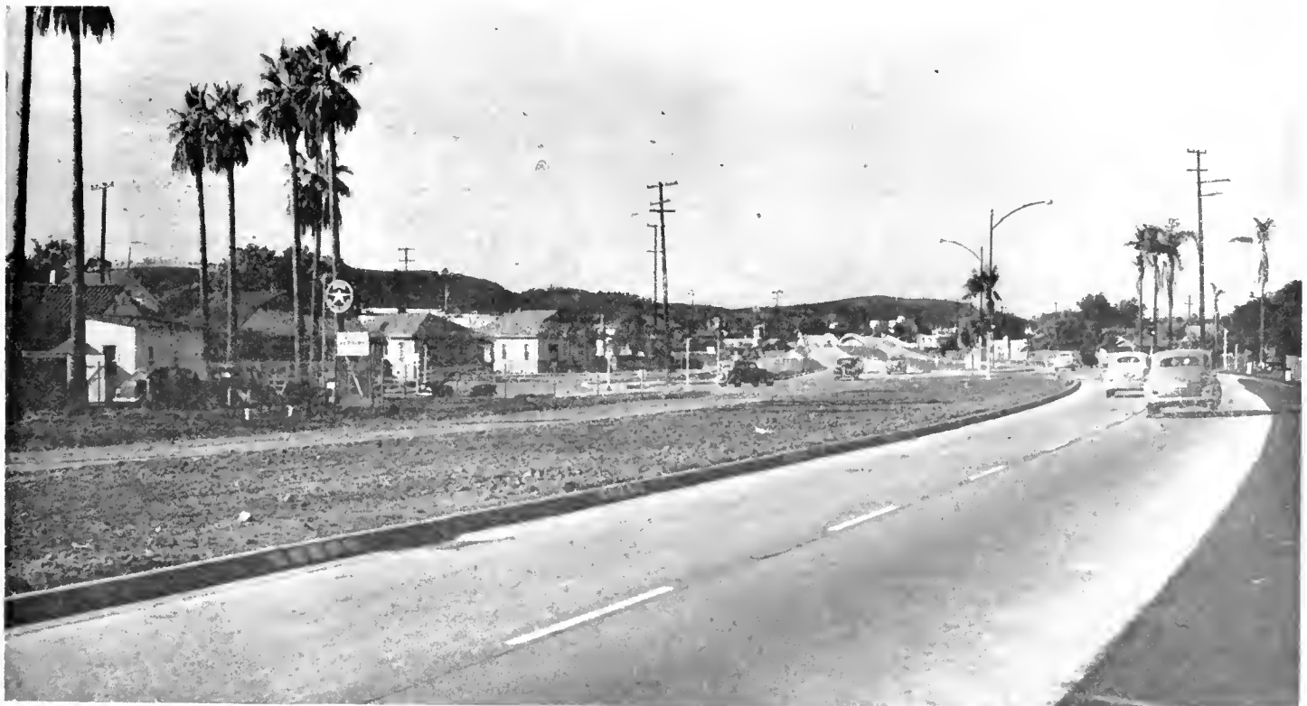
Milpos Street Intersection on easterly approach to Salsipuedes overhead structures
