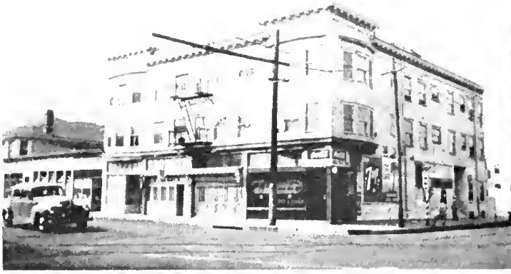
BEFORE —This three-story building with apartments above and stores below was located at 107 North Fremont Street. It was removed for the construction of the First Street bridge site on the Harbor Freeway.
