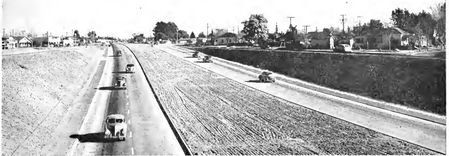
Looking southerly at California Avenue overcrossing. Wide separation between lanes allows for later construction of West Fresno Bypass
