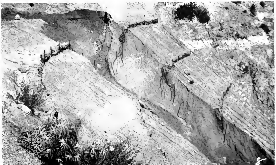
Iron pipe stakes and fencing fail to prevent slip out. Inadequate downdrains and resultant overlapping of the berm surface runoff contributed to failure. (Crest Drive, San Bernardino County)
