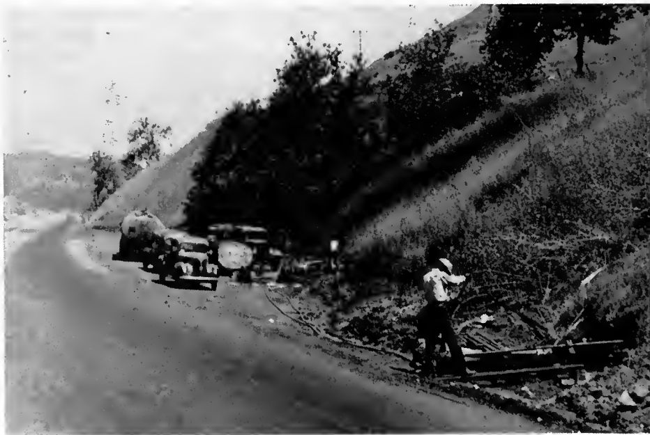
Two units drilling at Cuesta Grade
