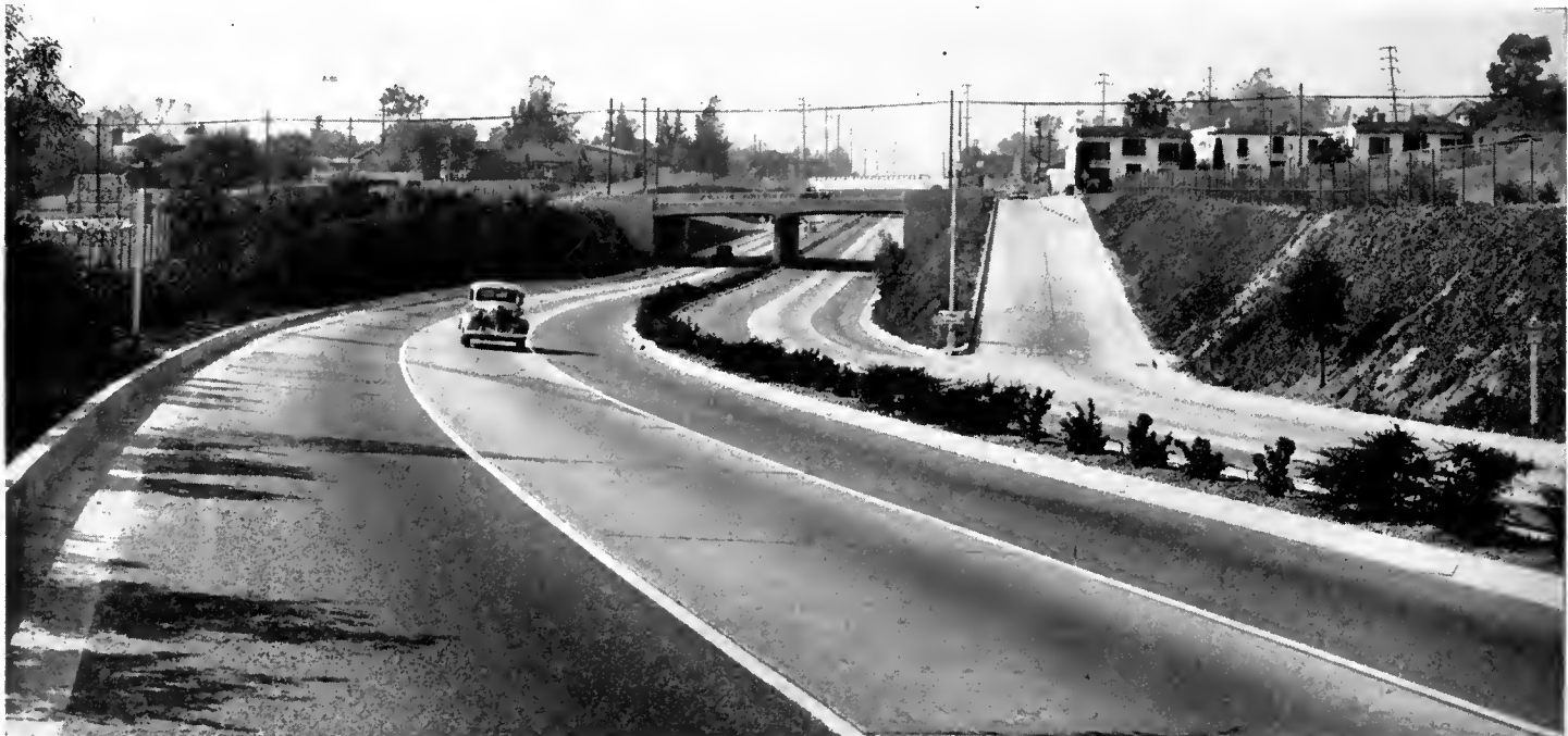
Present Fair Oaks off-ramp on Arroyo Seco Parkway where greater number of wrong-way movement accidents have originated. This structure is to be replaced by a new one, which will preclude the possibility of wrong-way use
