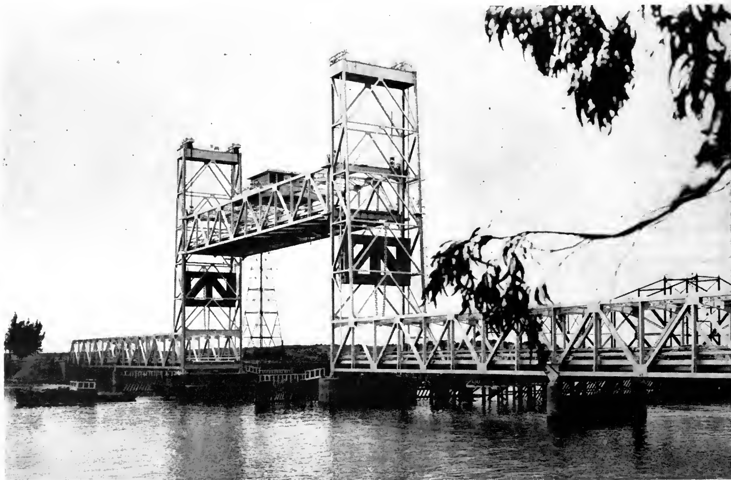
Looking northerly at downstream side of new Three Mile Slough bridge, with lift raised. The old bridge in the background will be removed by the county and re-erected at another location
