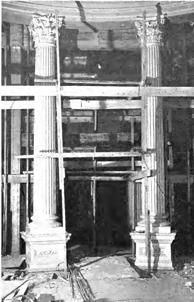
LEFT—Old cast iron columns on second floor of Capitol. New structural steel columns in the background are ready for guniting. RIGHT—Old cast iron columns on first floor at Capitol. Brick wall in background is ready for guniting
