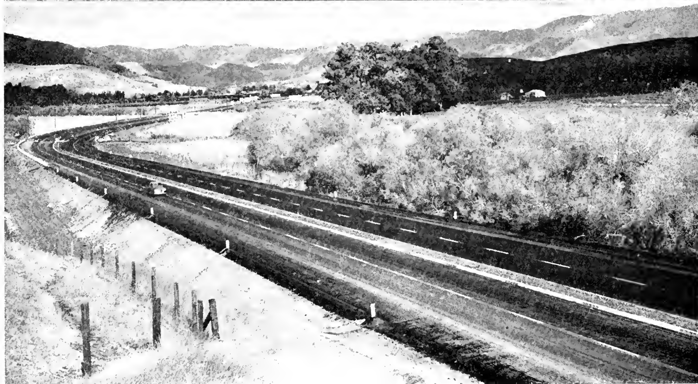
UPPER - View of new four-lane divided highway developed from old two-lane highway. LOWER - Looking north across San Luis Valley toward San Luis Obispo
