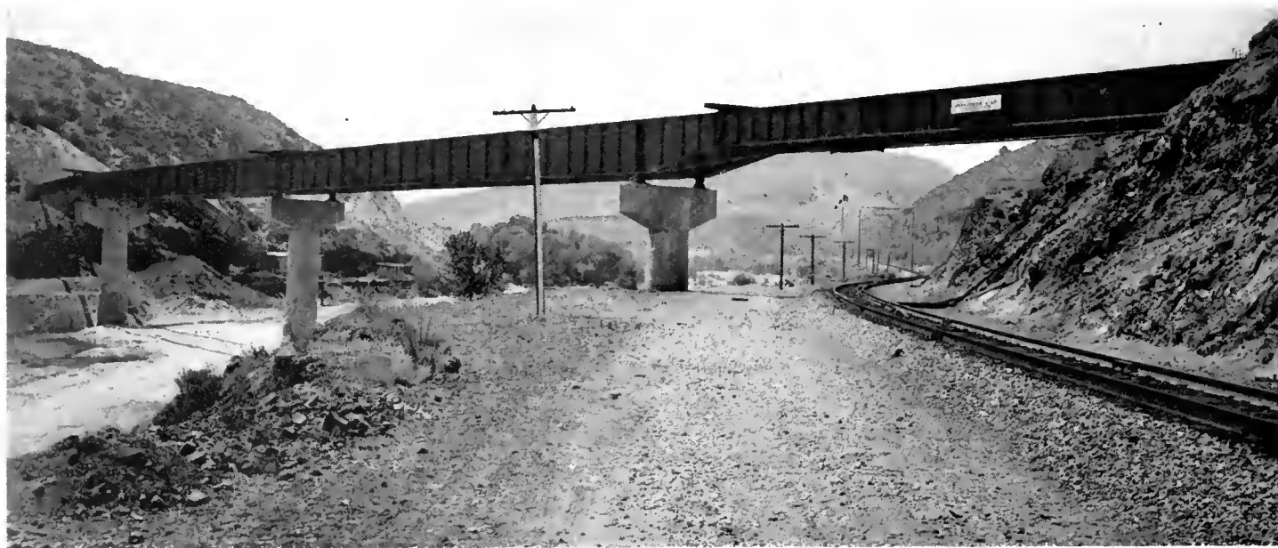
Photo of recently completed Santa Clara River bridge and overhead in Los Angeles County
