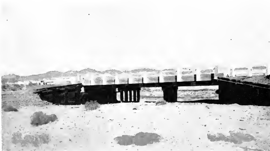
Typical desert structure after placing concrete deck and new railing
