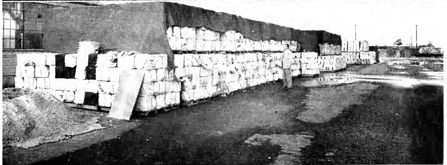
Upper—View of Sacramento warehouse showing loading dock and rail unloading facilities. Center—Las Angeles warehouse under construction showing rail facilities and portion of hard-standings. Lower—Portion of warehouse stack of survey stakes at Las Angeles. These stores protected from rains, top and bottom
