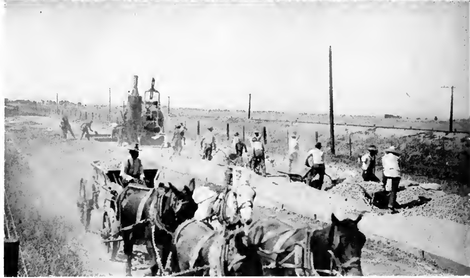
UPPER—This is U. S. 101 in Ventura County in 1916. Mr. Gibson is again stalled in the mud. LOWER—Pick and shovel crews and mule drawn equipment built highways for Mr. Gibson in 1916. This photo was taken on U. S. 99 in Butte County
