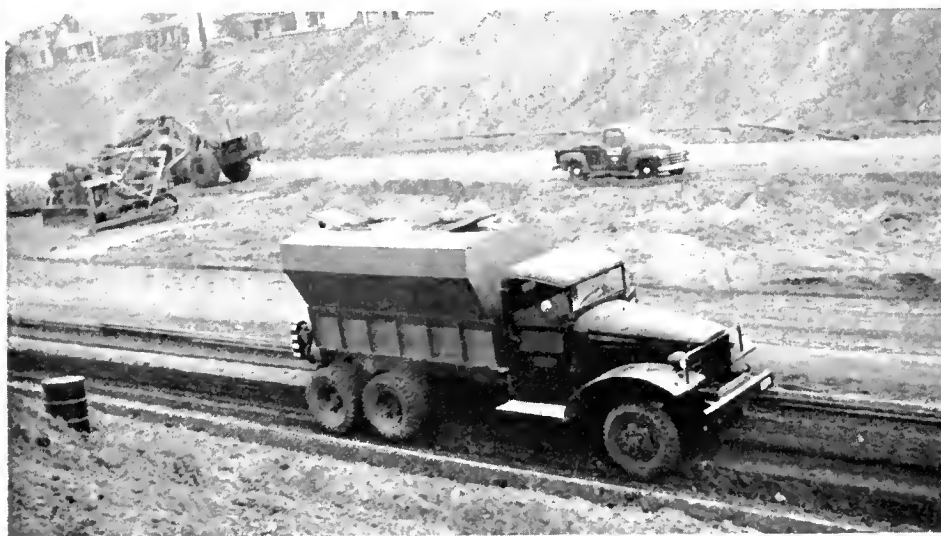
Center—Cement spreader truck in operation
