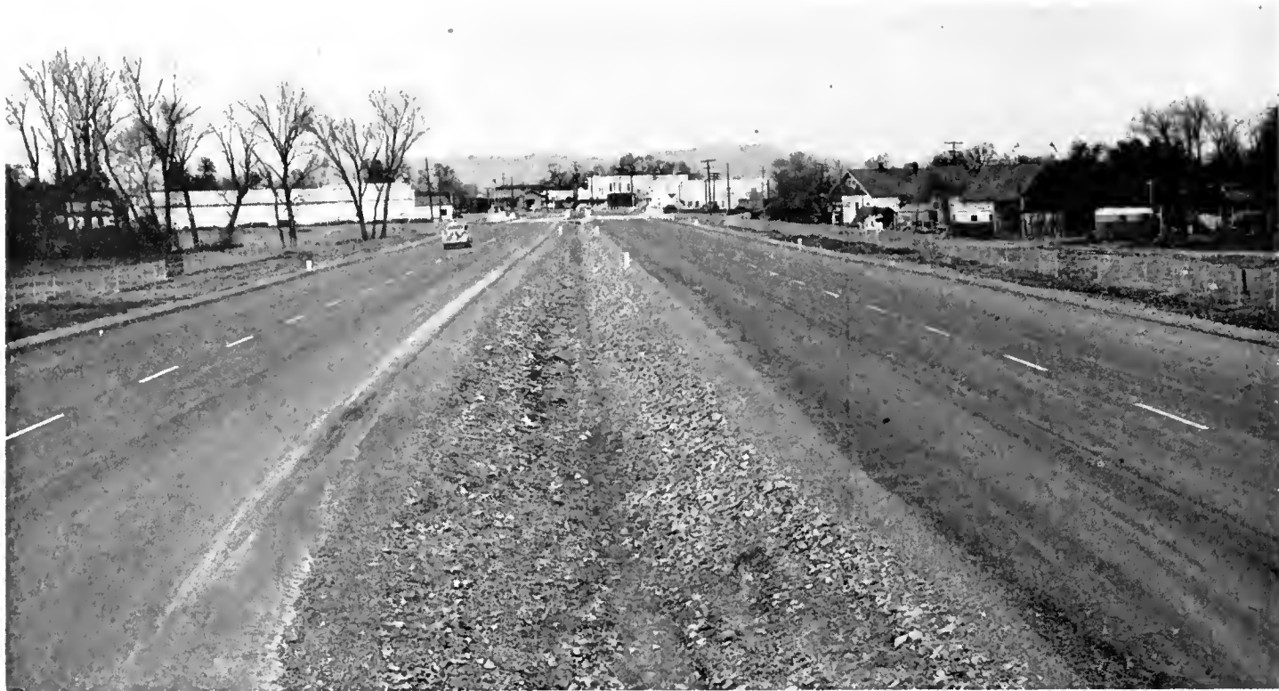
View of new highway entering Anderson. Bridges across Anderson Creek in background
