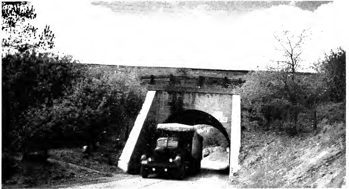
Old narrow underpass which is being replaced by the new Bailey Hill Underpass
