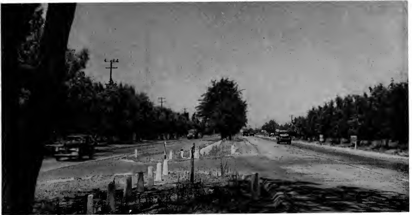
Recently completed four-lane divided highway on US 99 between Lodi and Stockton
