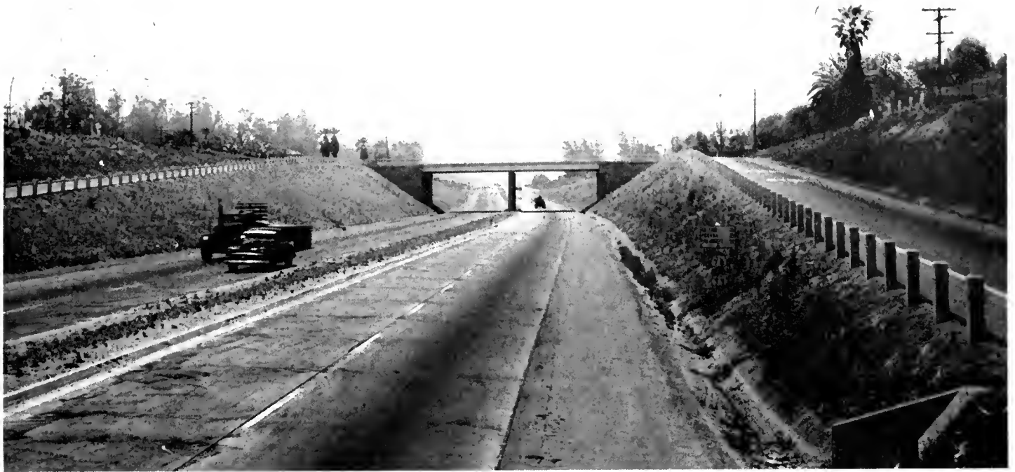
UPPER—Cedar Avenue grade separation at Blaamingtan, showing ramp connections to that community. LOWER—This is the Kaiser spur overpass. Spur railroad tracks may be seen entering underpass an left
