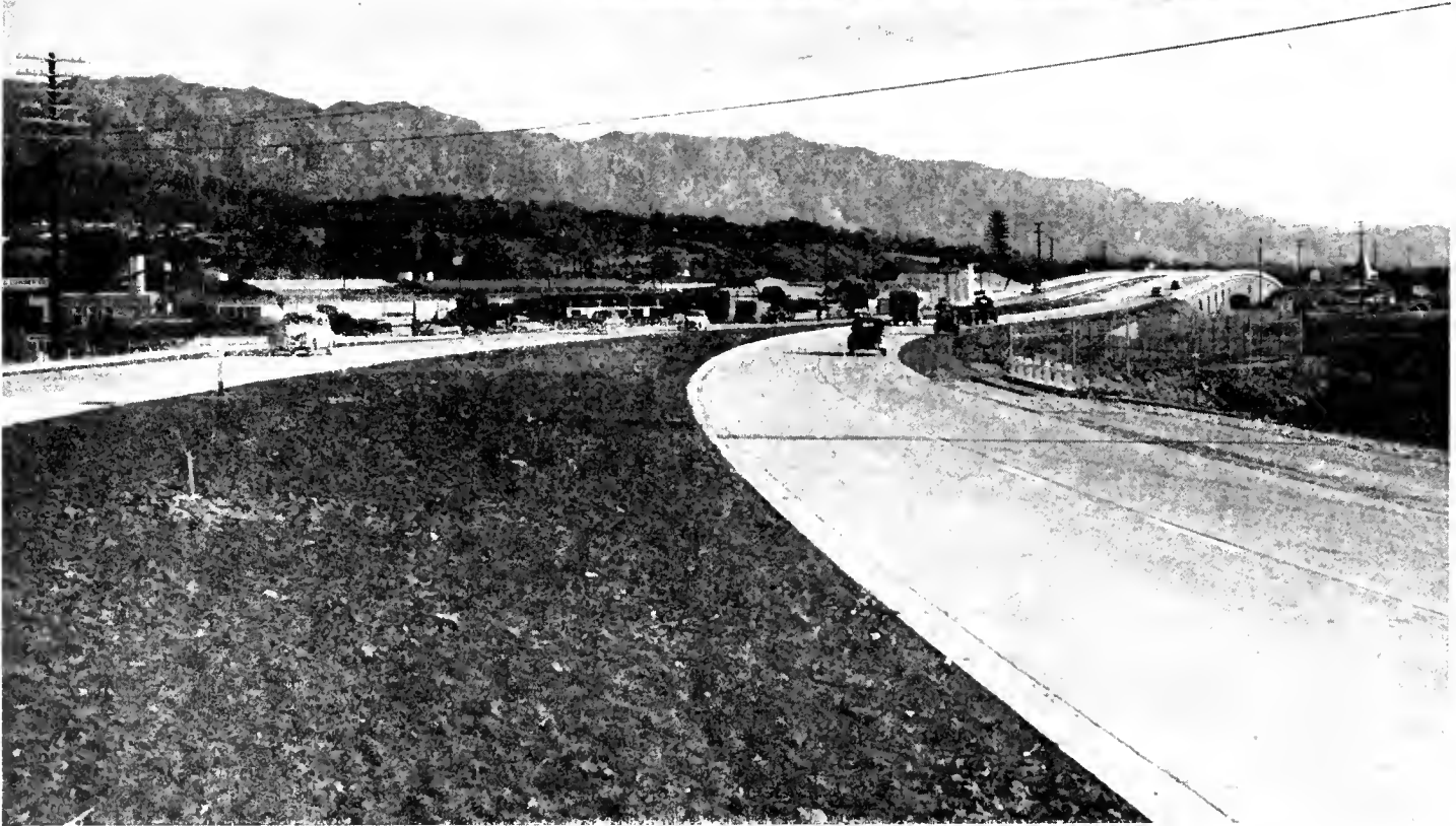
UPPER View of freeway showing Montecito Street as outer highway on southerly side. LOWER Santa Barbara Freeway looking easterly, showing Salsipuedes overhead structures. Santa Ynez Mountains in the distance
