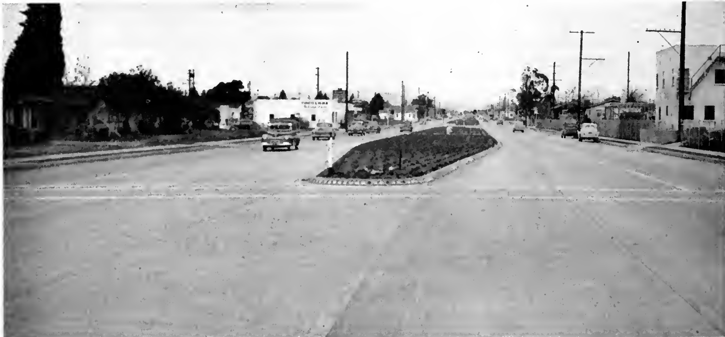
Olympic Boulevard extension looking easterly from near Lincoln Boulevard, showing newly completed divided highway construction
