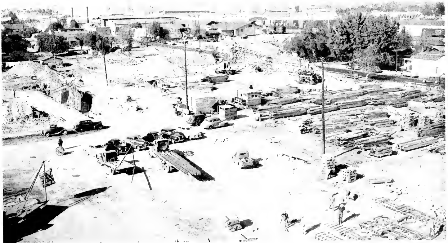
UPPER—View southerly from the church tower during the move. The old foundation with part of the cribbing used in the move is in the foreground with the cleared right of way extending beyond. Once filled with buildings, there remained only the fire station on the left with the beer wholesaler just beyond and the bar being moved when the picture was taken. LOWER—View northerly from the church tower. In the foreground workmen are laying tracks for another move. Note the retaining walls for the Monterey Street overpass that curves to the right
