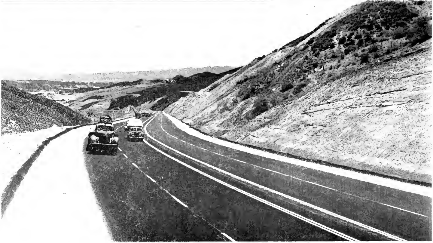
Conversion of the Ridge Route on U. S. 99 to a four-lane divided highway is under way. These photographs show completed sections of the first unit of the project north of Castaic. This route carries exceptionally heavy truck traffic
