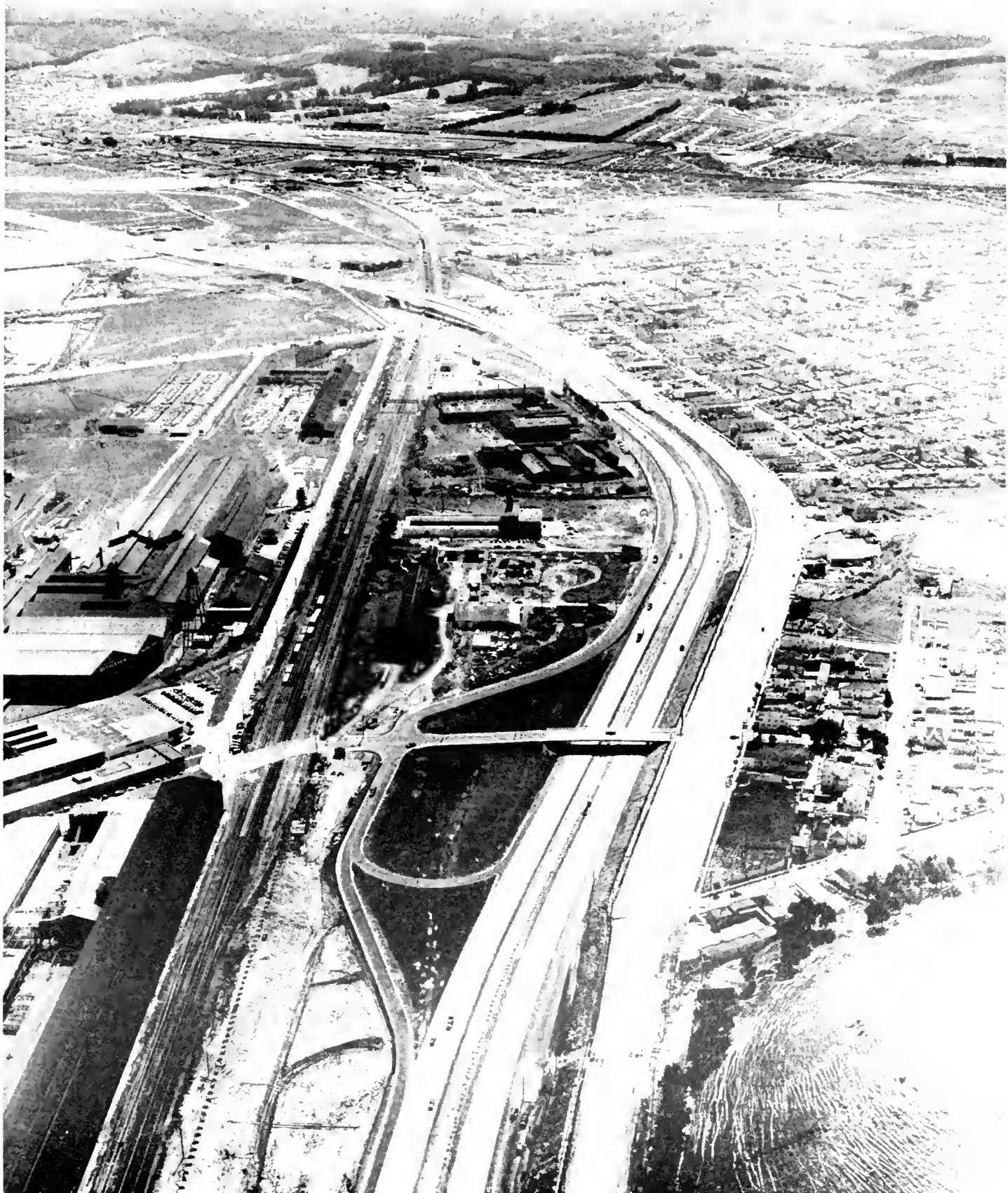
Butler Road overcrossing in South San Francisco. Pedestrian overcrossing in central section and Grand Avenue overcrossing in background
