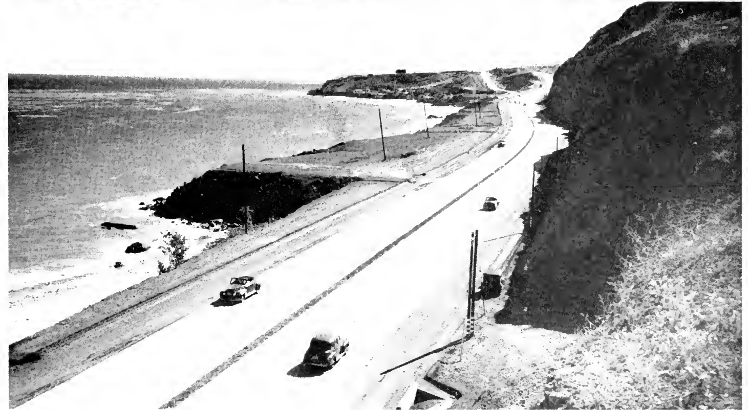
Realignment of U. S. 101 between Malibu Creek and Latigo Canyon in Los Angeles County was recently completed. These photographs show two sections of the new four-lane divided highway between these two points
