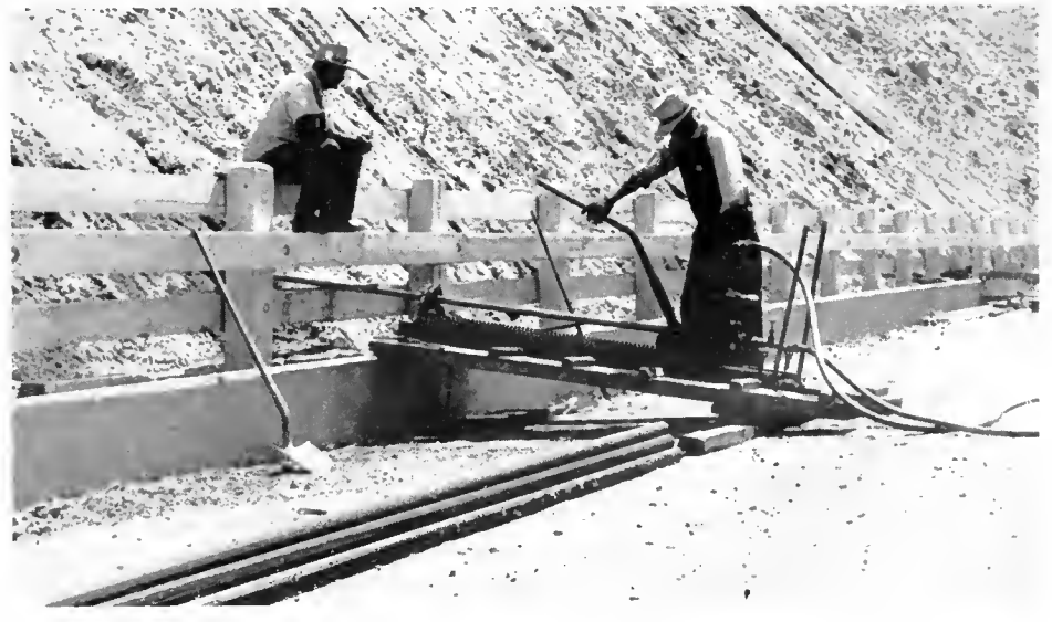
Hydrauger in drilling position at Grapevine slide
