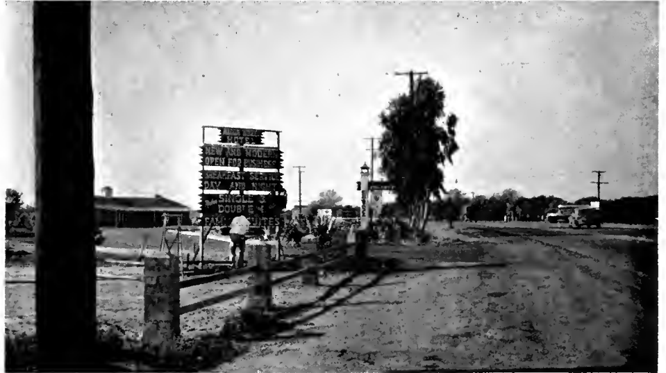
Upper—Photo taken in October, 1946. Junction Motel in background, site of Wagon Wheel improvements in center foreground. New outer highway is now constructed across the right foreground of this area. Lower—Photo taken in September, 1947, just prior to the construction of the freeway and outer highway
