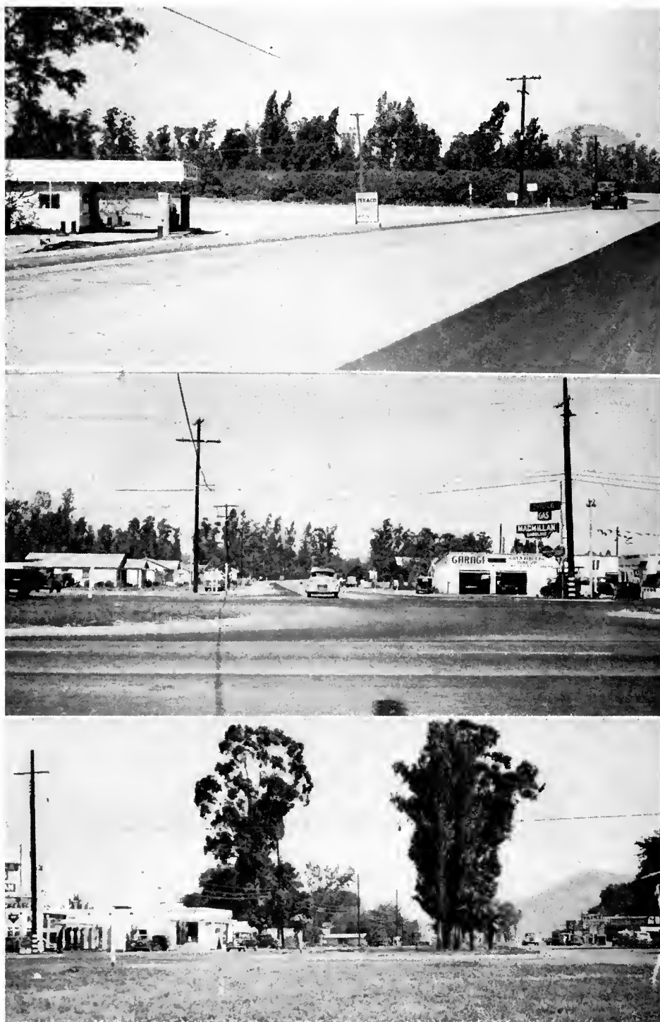
UPPER—At Fourth Street, looking northerly. Old road with 200-foot radius turning to left. CENTER—At junction in West Riverside looking northerly along the project. LOWER—At junction in West Riverside, looking west along U. S. 60 toward Riverside. Portion of Mt. Rubidoux in right background
