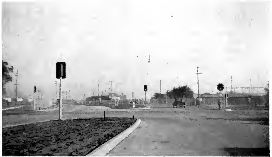
Looking westerly across 14th Street, showing left-turning lanes
