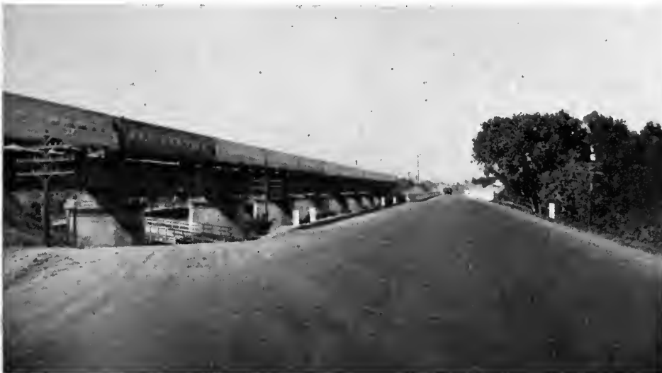
This view of new FAS highway is looking northeast
