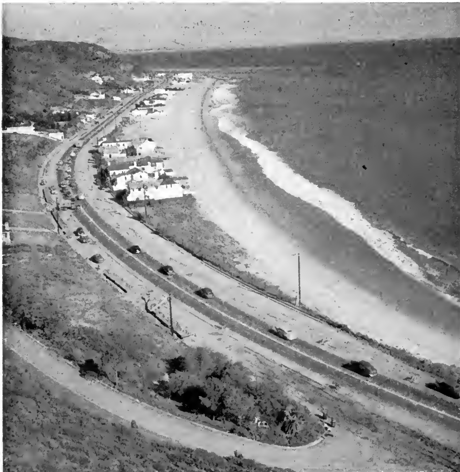
View from Carbon Point looking easterly and showing widening operations in progress
