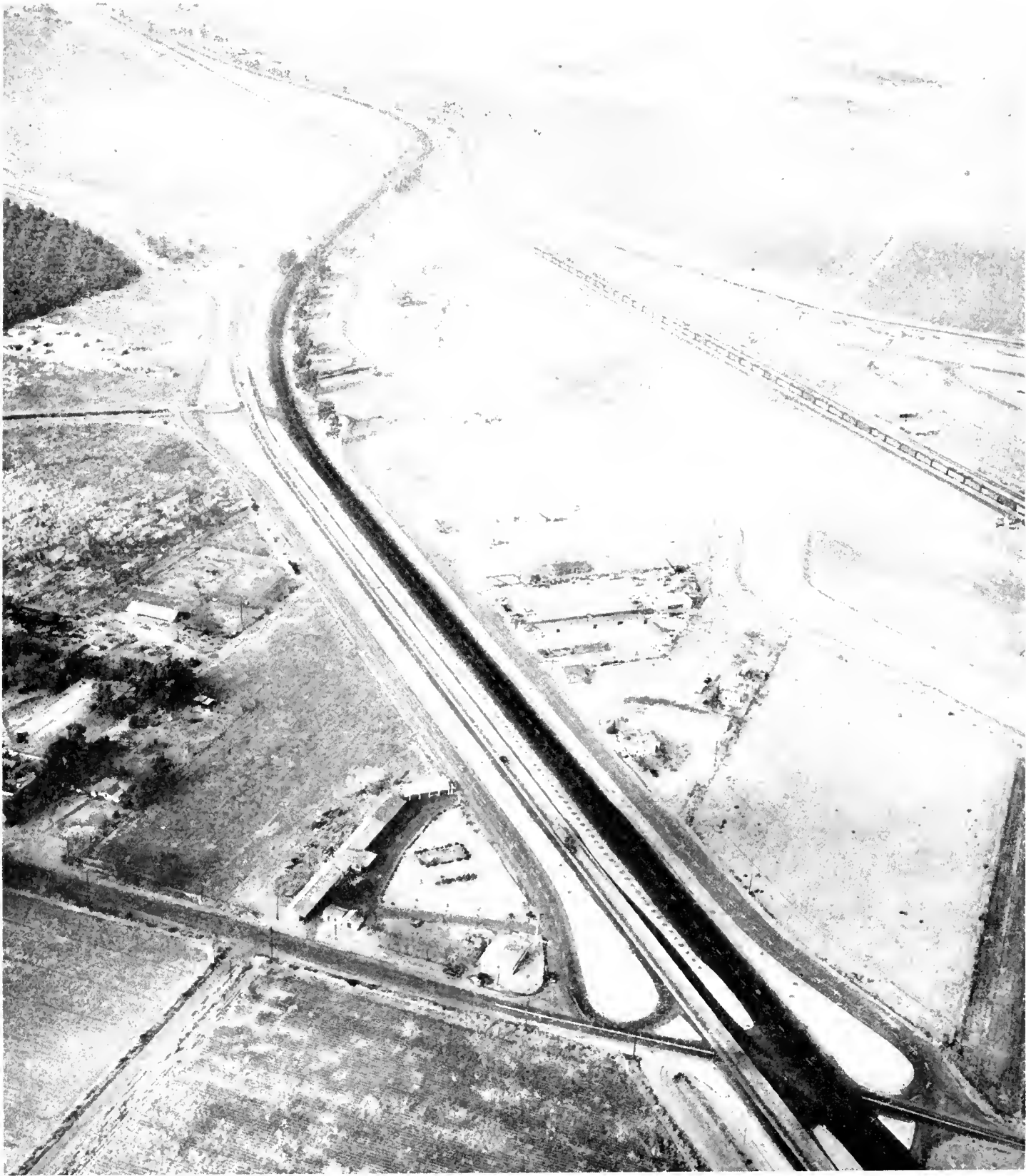
Northerly from Olive Drive. Existing highway on right used for northbound traffic and new Portland cement concrete pavement on left used for southbound traffic. Two-way outer highways border the freeway between Olive Drive and Narris Road. The Southern Pacific Overpasses appear in the background and the Standard Oil Tank Farm in the far background
