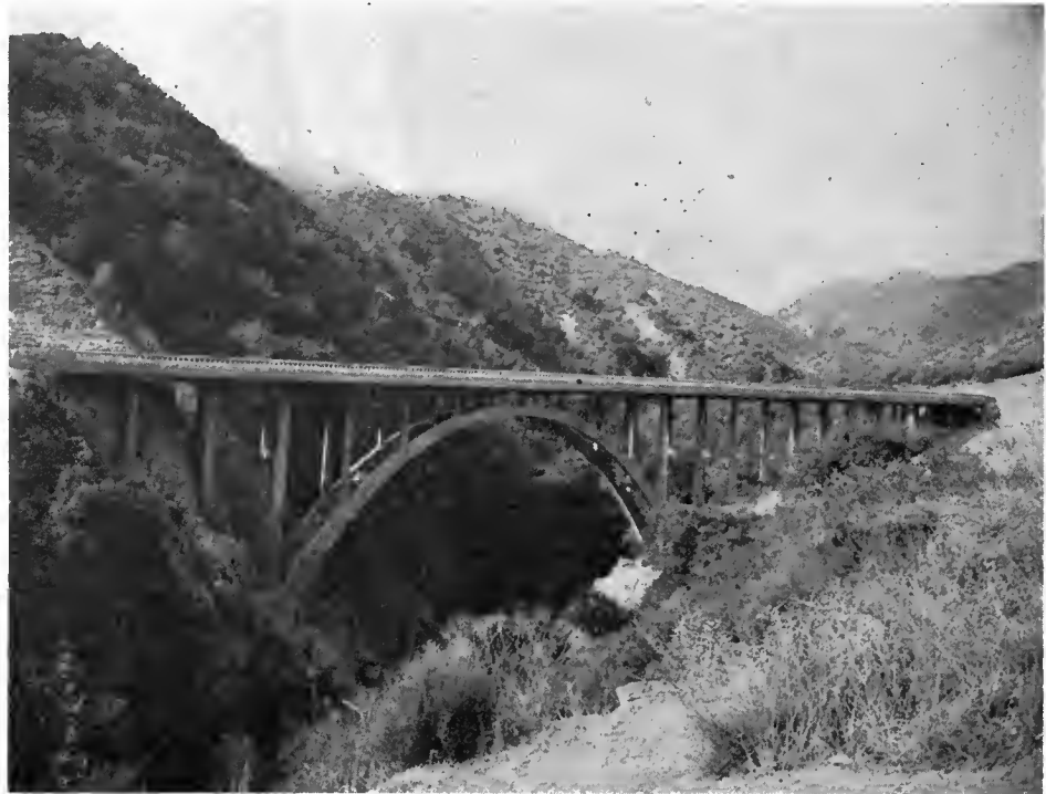
Recently completed arch bridge, which will provide a link in the new City Creek Road near San Bernardino
