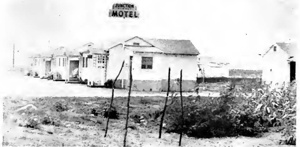
Upper—Photo taken in May, 1949. At right center is a boulevard stop for cars entering the freeway from the outer highway. Lower—Photo taken in October, 1946. Motel units shown in center of picture were moved back to make room for outer highway construction
