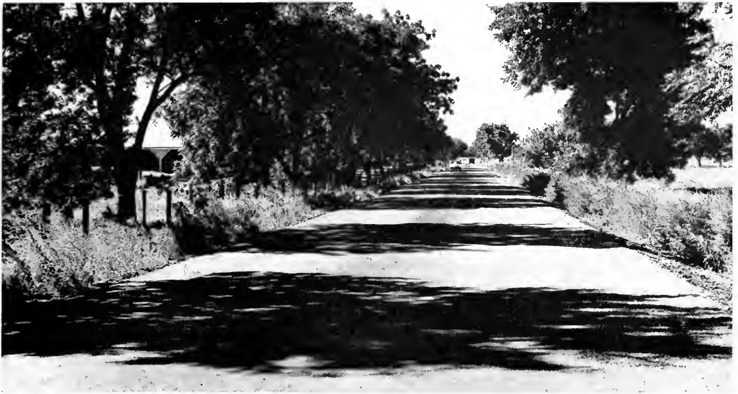
Completed section of new Yolo County highway looking west about four and one-half miles east of Greendale
