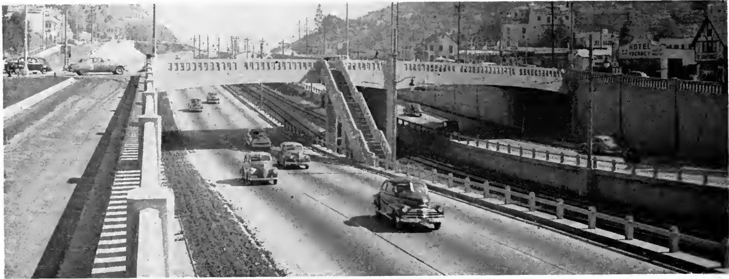
This is a closeup of the Barham Boulevard separation structure completed same years ago under a Los Angeles city contract
