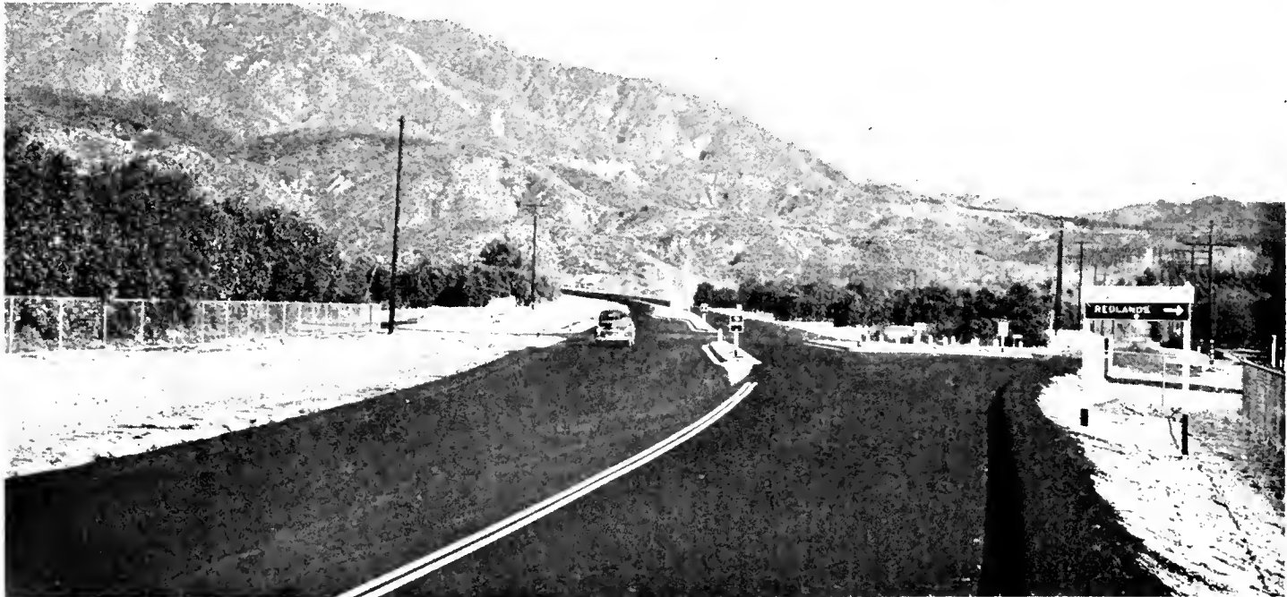
On valley floor among the orange groves. Looking East at beginning of the nearly completed First Unit. Channelized connections to Highland Avenue in foreground, leading toward San Bernardino and to Boulder Avenue at right, leading toward Redlands. New highway curving to left in background entering City Creek Canyon.
