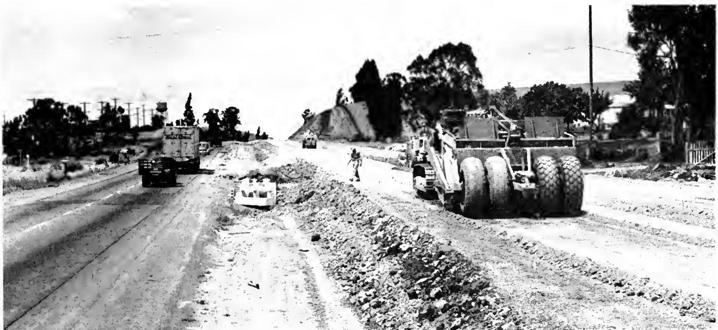
Finishing rough grade near Tennessee Street
