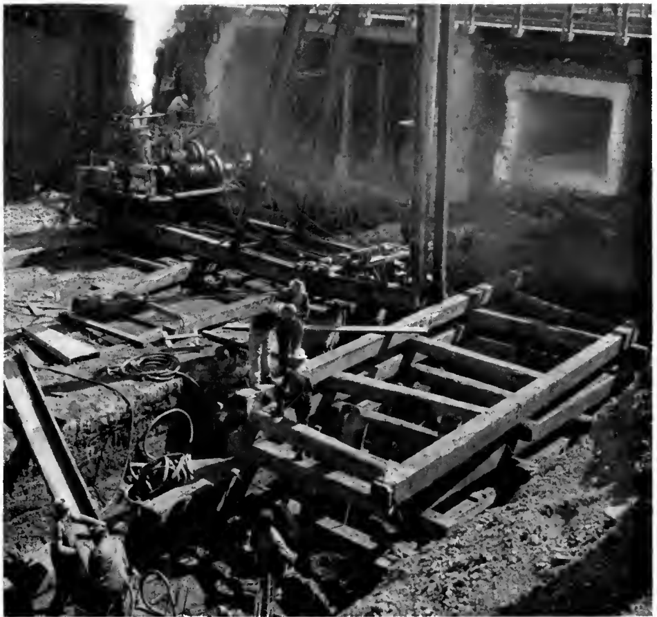
Close up of pile driving operations on 12th Street underpass project
