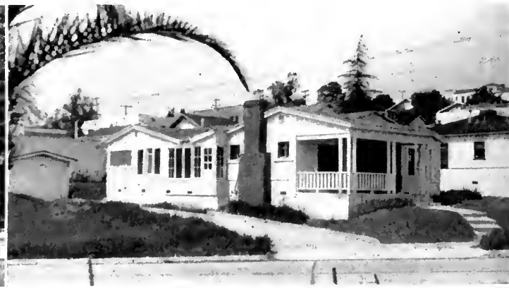
AFTER —This residence is now located at 717 Tulerasa. The eaves have been cut, the porch remodeled, and the entire building redecorated.
