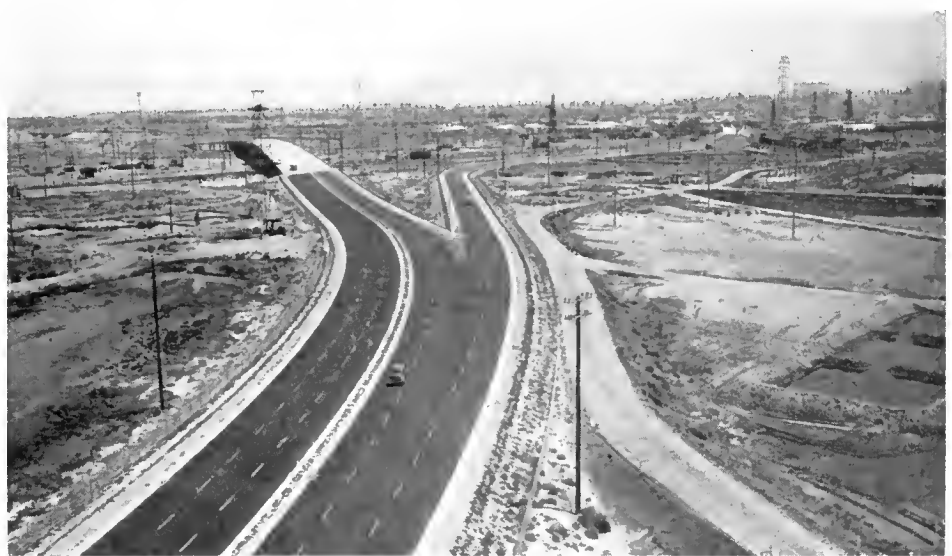
Freeway looking northeasterly toward Anaheim Street Viaduct over Union Pacific, Southern Pacific, and Pacific Electric Railroad tracks, and Anaheim and I Streets. Off ramp to Anaheim Street in Long Beach is roadway to right
