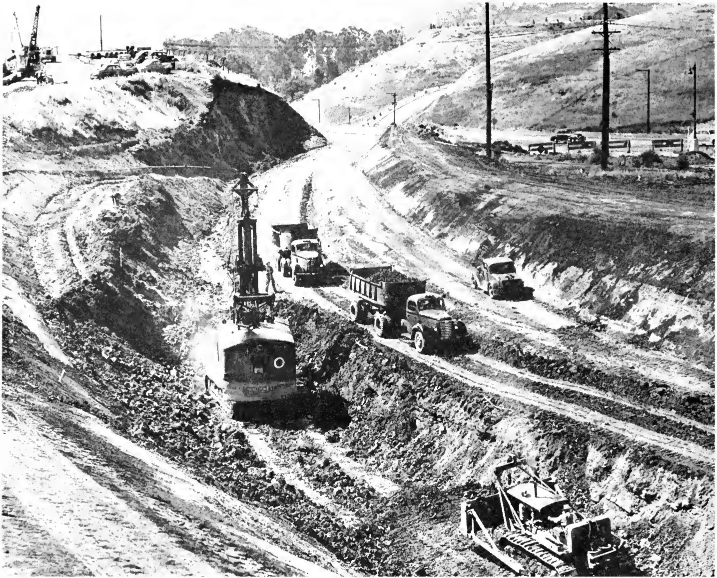
Excavating for entrance to underpass at Fourth Street
