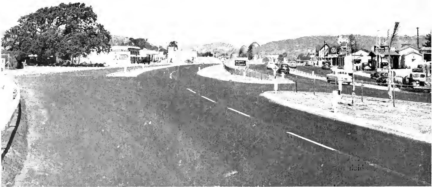
UPPER—In first block of east outer highway, Buellton, motorists have a wide choice of service stations. LOWER—Buellton today. All visible buildings except the inn proper were moved back or altered to provide this broad new boulevard
