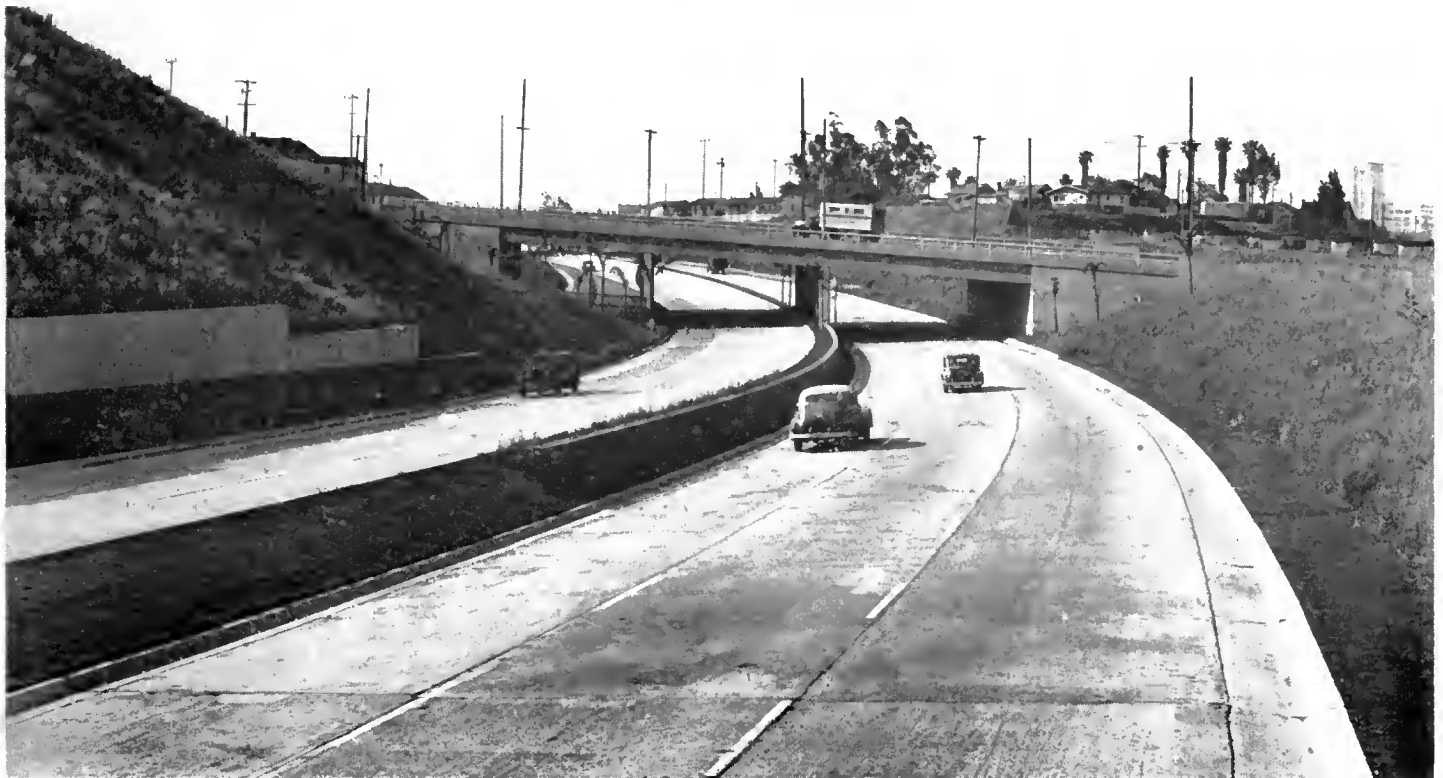
Santa Ana Freeway looking southerly to the Seventh Street grade separation
