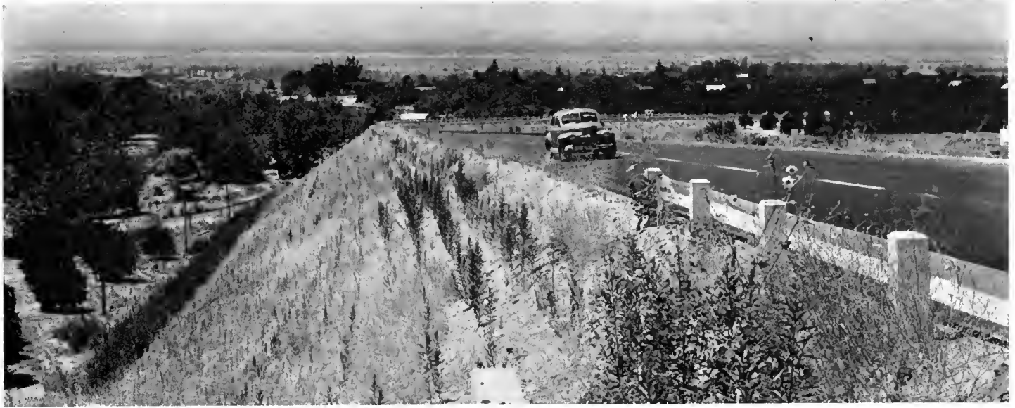
Six months after seeding, showing grain, natural growth, and Baccharis. Note heavy growth of 1½-year-old Baccharis on lower portion of fill
