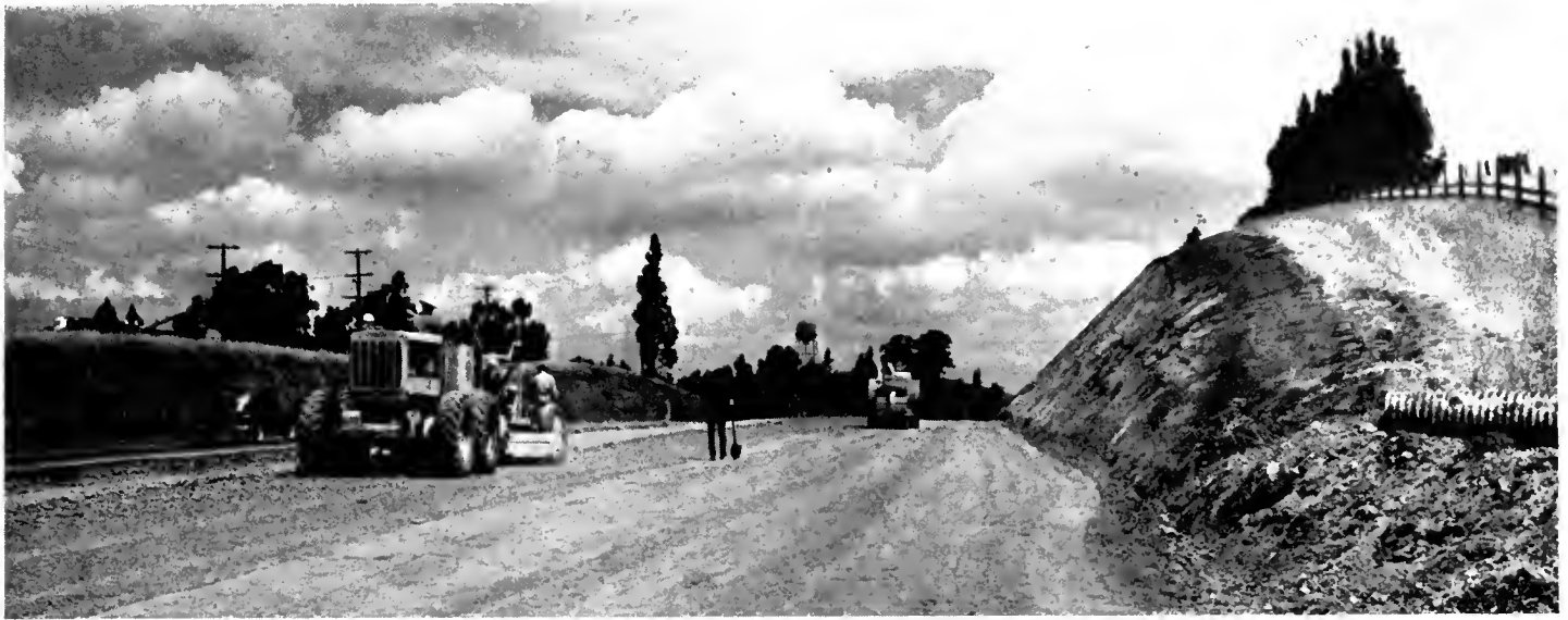
Finishing rough grade near Fleming Avenue
