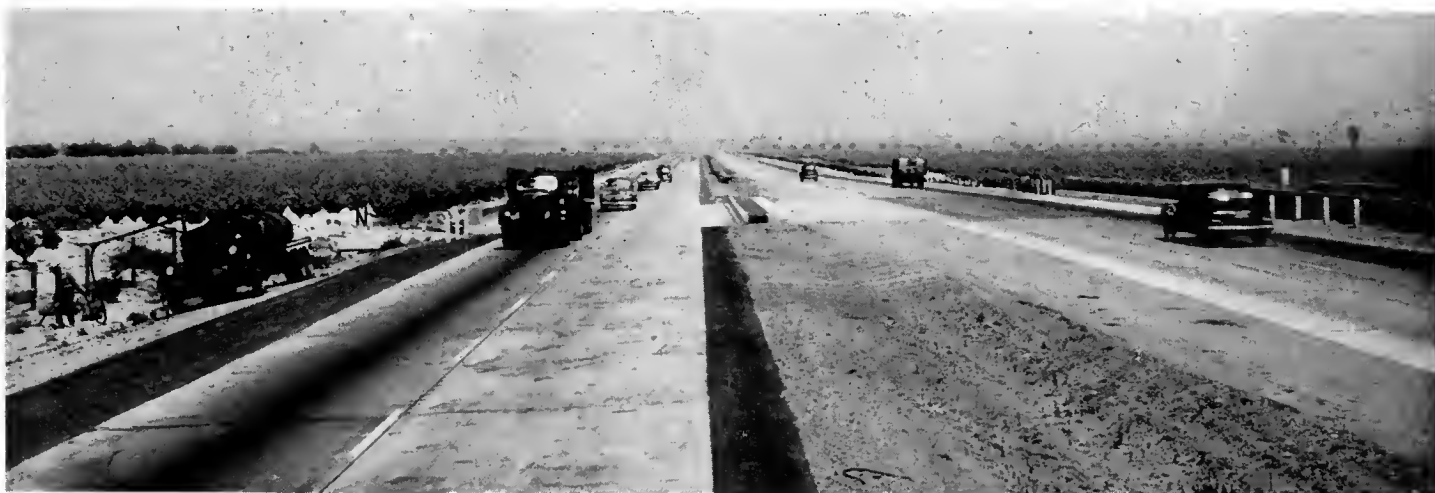
West of Etiwanda Avenue, showing heavy mixed truck and passenger traffic on new freeway. Pavement on right is former three-lane pavement now used for east bound traffic
