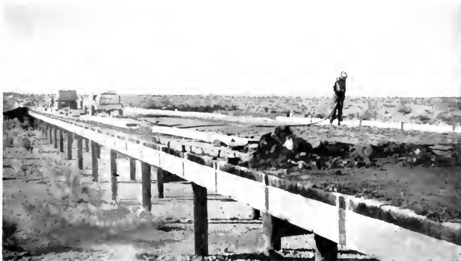
Removing surfacing from desert bridge preparatory to redecking
