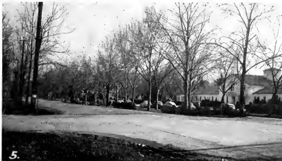
Parking along the outer highway leaves the main center roadway clear for through traffic
