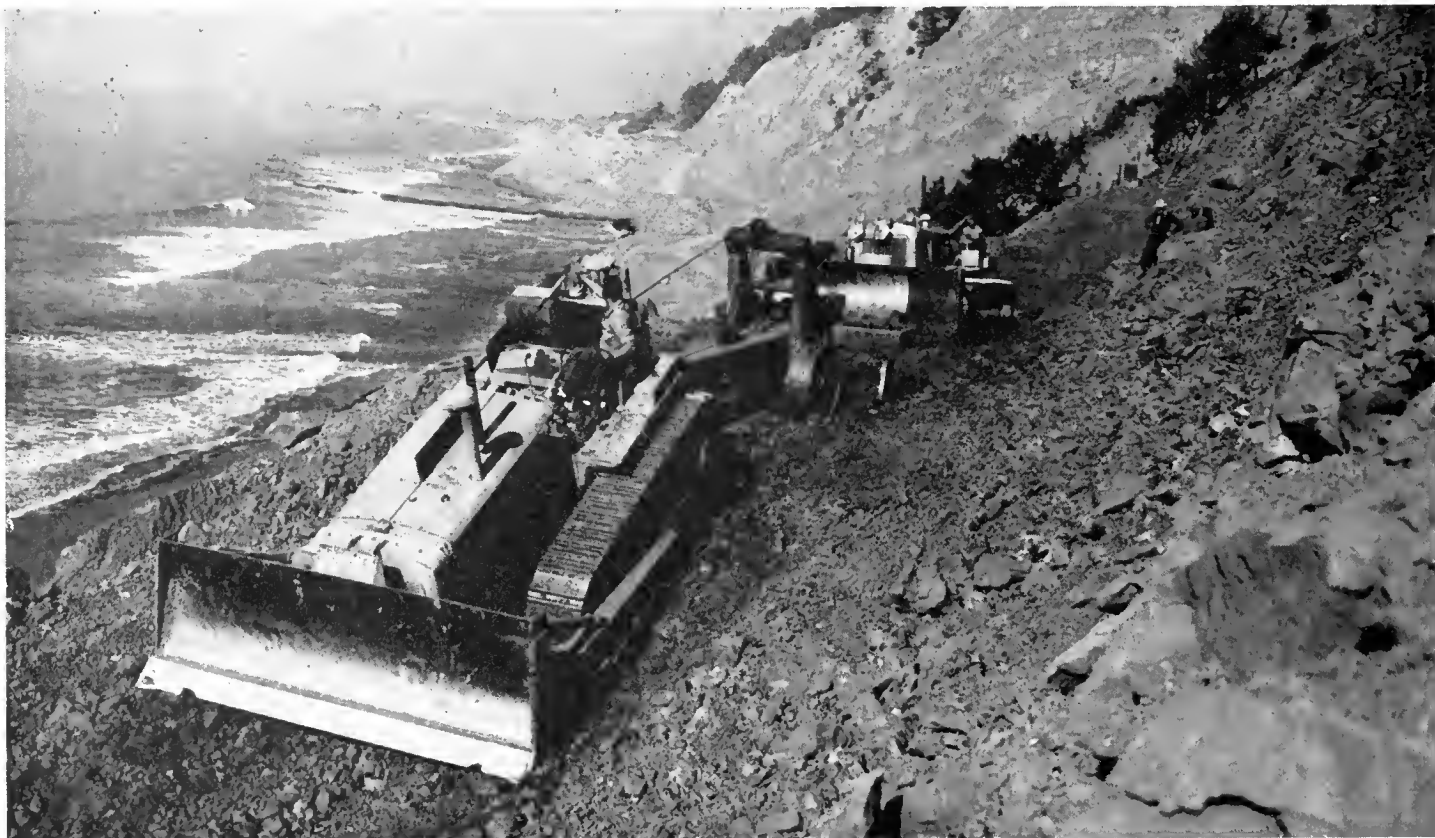
Bulldozer crews on the Waddell Bluffs job did not have an easy task
