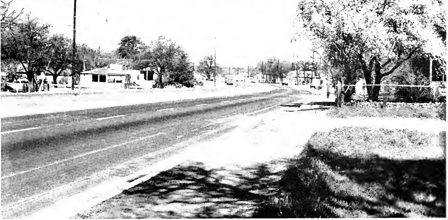
Upper—Aerial view showing old, winding road on left and new highway on right on top of Cottonwood Hill. Lower—Four-lane divided highway into Cottonwood
