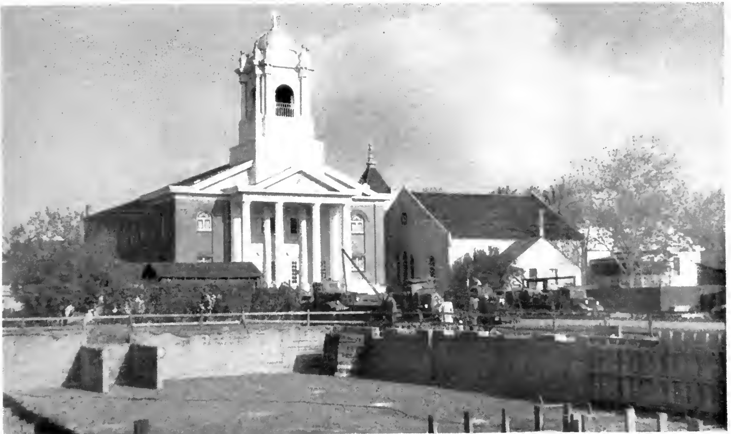
View of church being towed longitudinally along city streets with the newly constructed base and concrete foundation in the foreground
