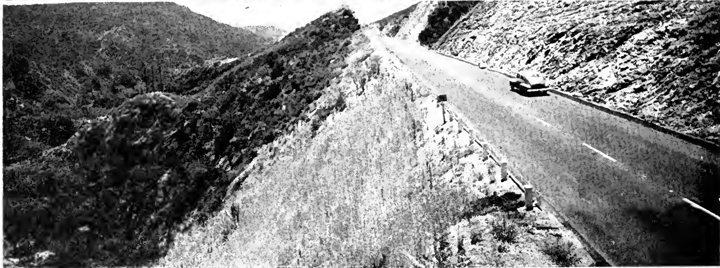
Upper - Grain and Baccharis six months after planting. Center - Vegetative erosion protection 1 1/2 years after planting. Embankment is 130 feet high. Lower - Vegetative erosion protection, five months old
