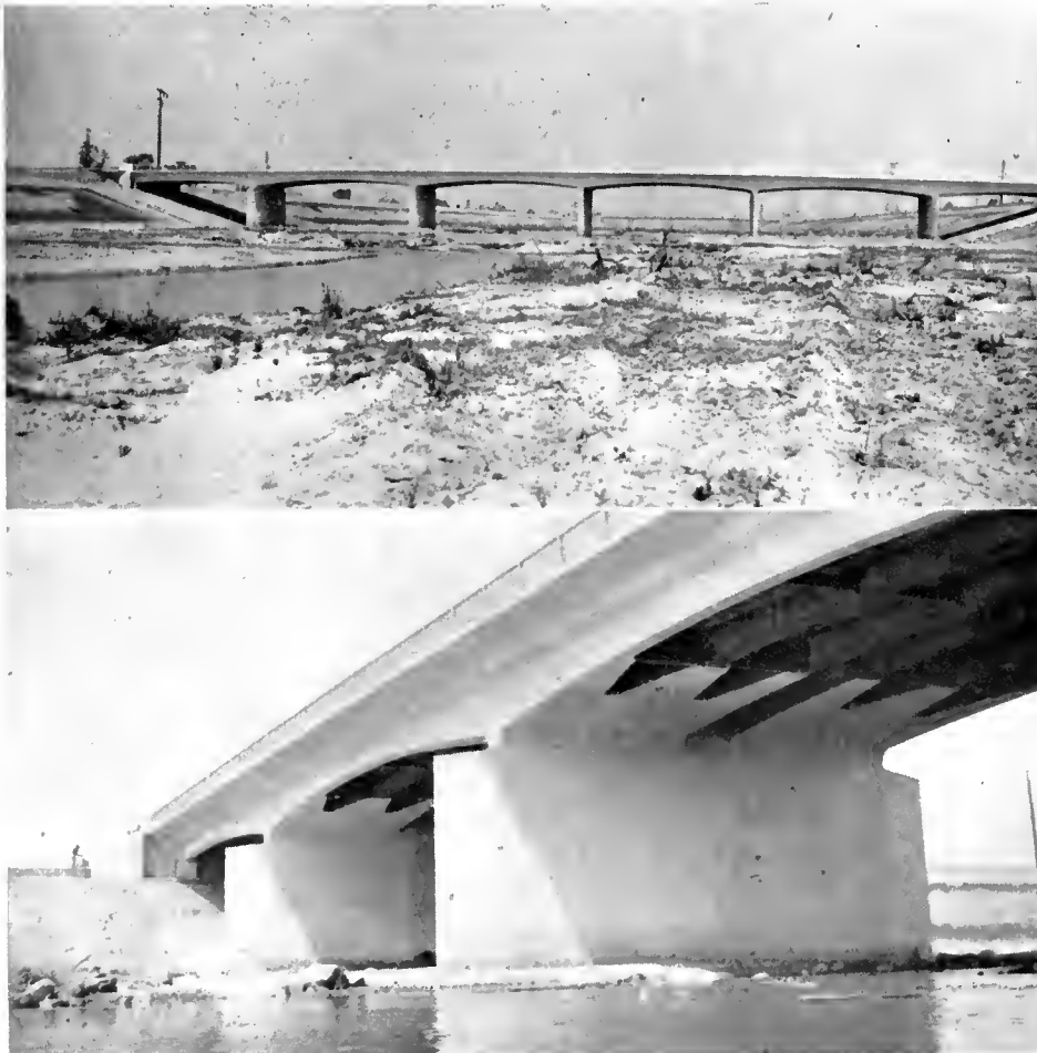
Two views of Florence Avenue bridge across Los Angeles River constructed with FAS funds
