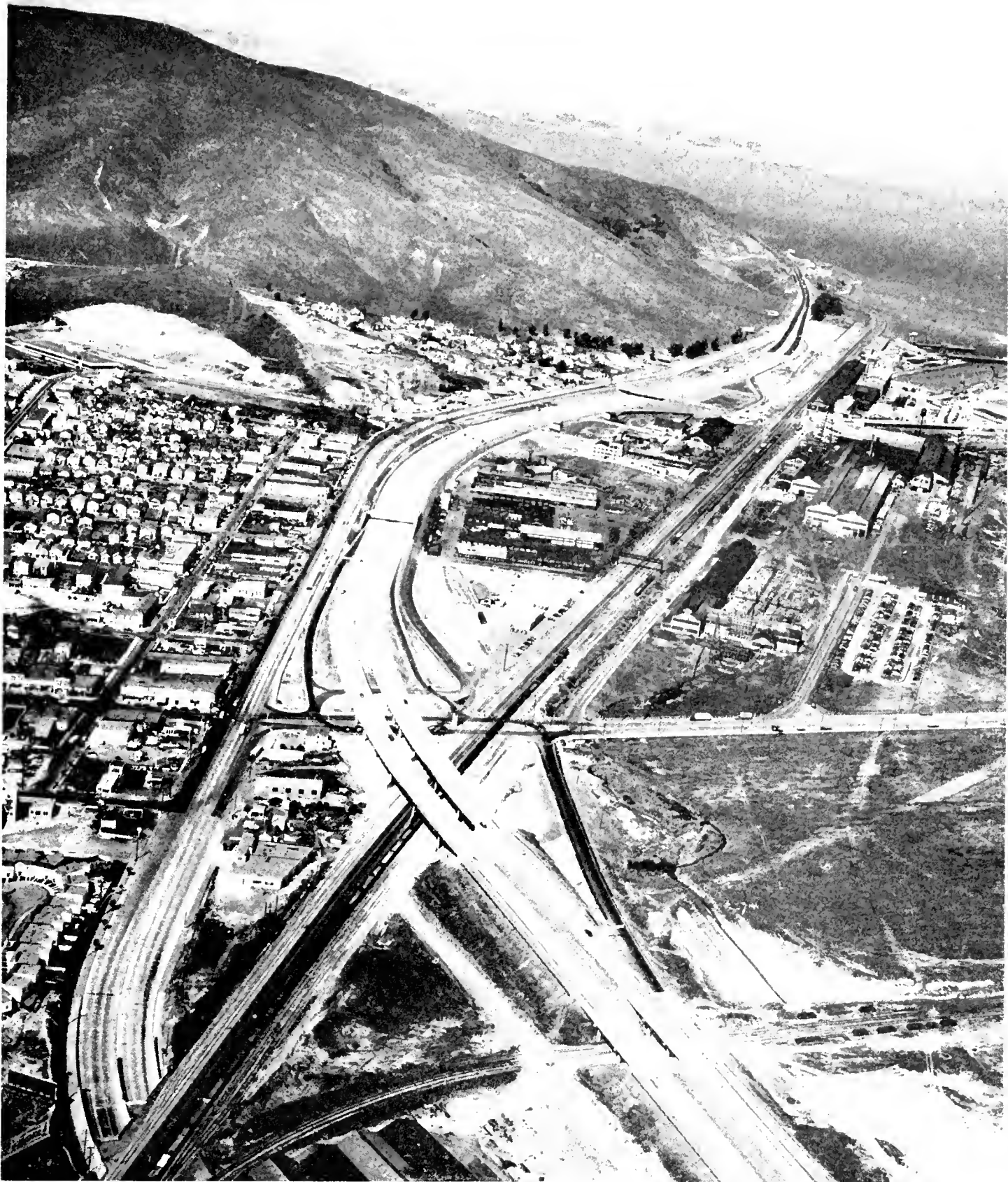
Looking north on the new Bayshore Freeway toward Sierra Point, Hunter's Point in distance
