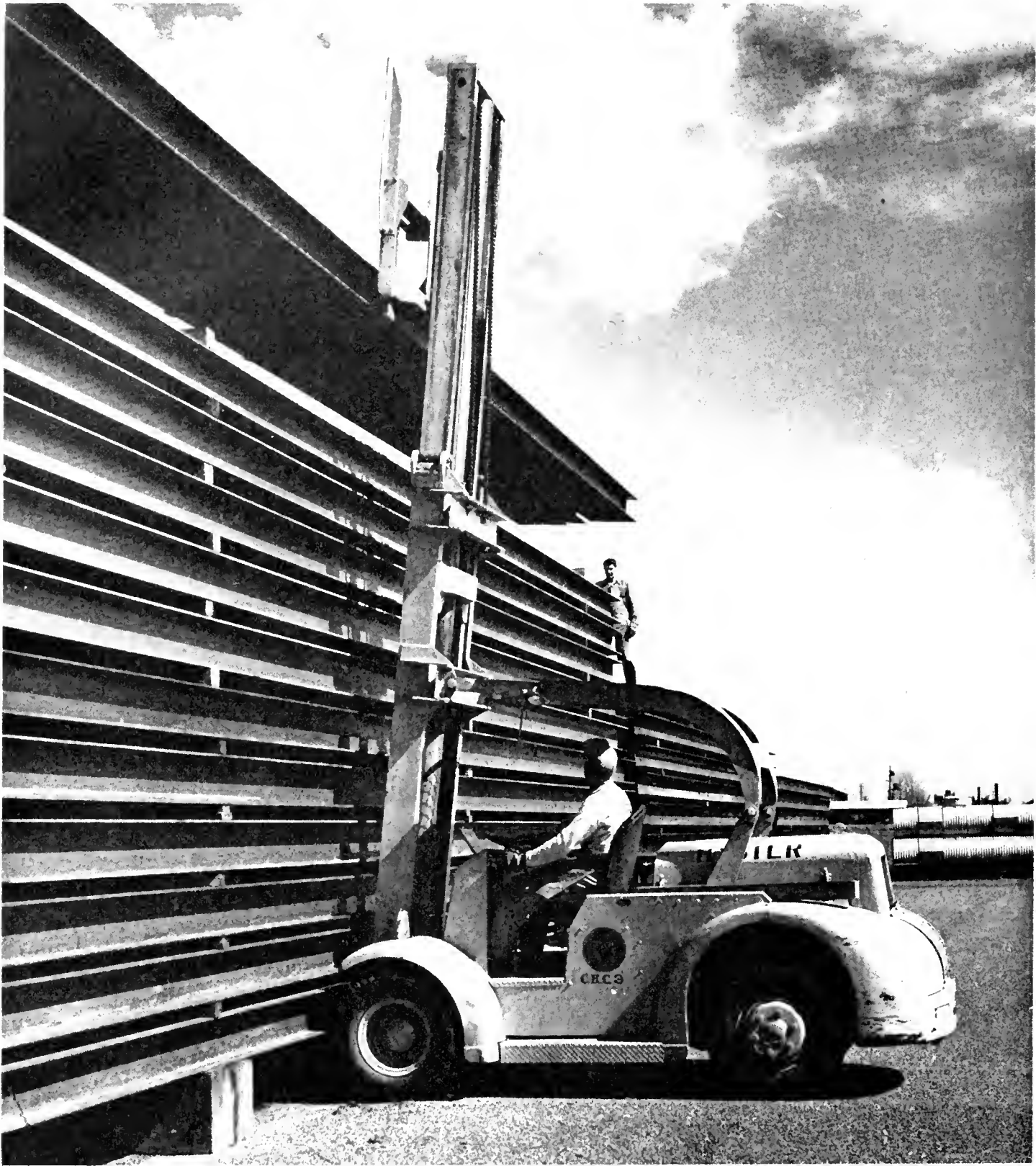
Lift truck stacking H piling at Sacramento warehouse. Contractor may borrow required piling from Stote and save weeks or possibly months awaiting shipment
