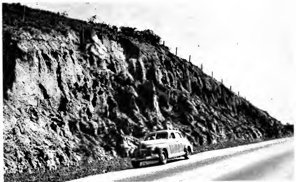
Highly erasive soil near Salinas. Note loss of soil above fence line. Slaughtered material bladed off traveled way must be hauled away by truck
