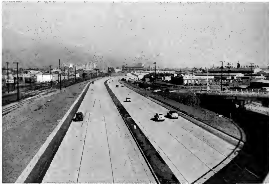
Completed section of Eastshore Freeway opened to traffic on July 22d
