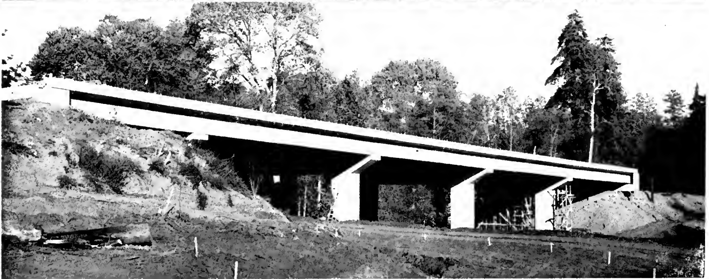
UPPER—Soquel Road Overcrossing, looking west. LoFonda Avenue Overcrossing in background. CENTER—North Aptos Underpass, under tracks of the Santa Cruz-Watsonville branch of the Southern Pacific Railroad. LOWER—Aptos Creek Bridge and Spreckels Drive Undercrossing
