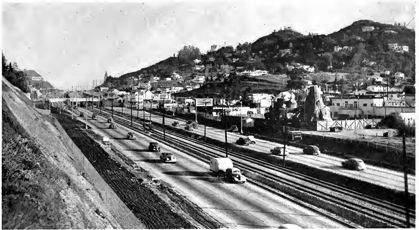
Looking southeasterly along completed freeway showing Barham Boulevard grade separation overcrossing
