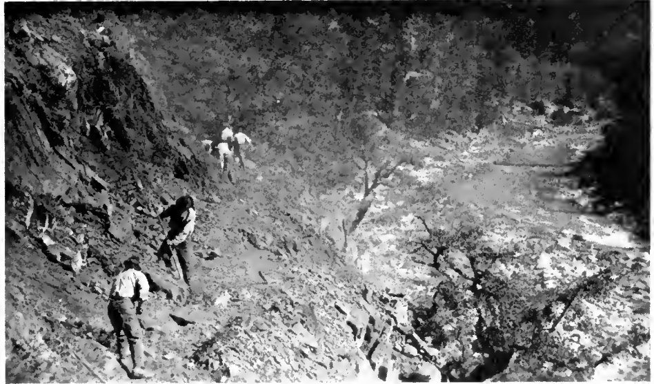
Early day methods of building highways with prison labor. UPPER—Finishing roadway with horses and carts along Klomoth River, Siskiyou County, 1920. CENTER—Excavation with teams and slip scrapers in Mendocino County, 1916. LOWER—Pioneering trail on North Fork of Yubo River, Sierrro County, 1916
