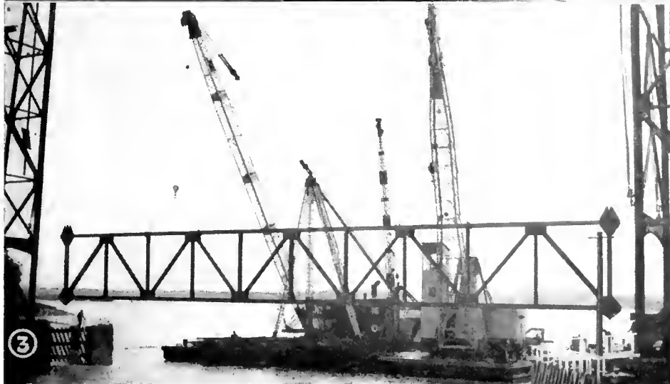
1—Picking up one-half of lift truss prior to carrying it around by barge and putting it in place. 2—Barge transporting one lift span truss to its position in the channel. 3—Placing truss in place in channel between lift towers
