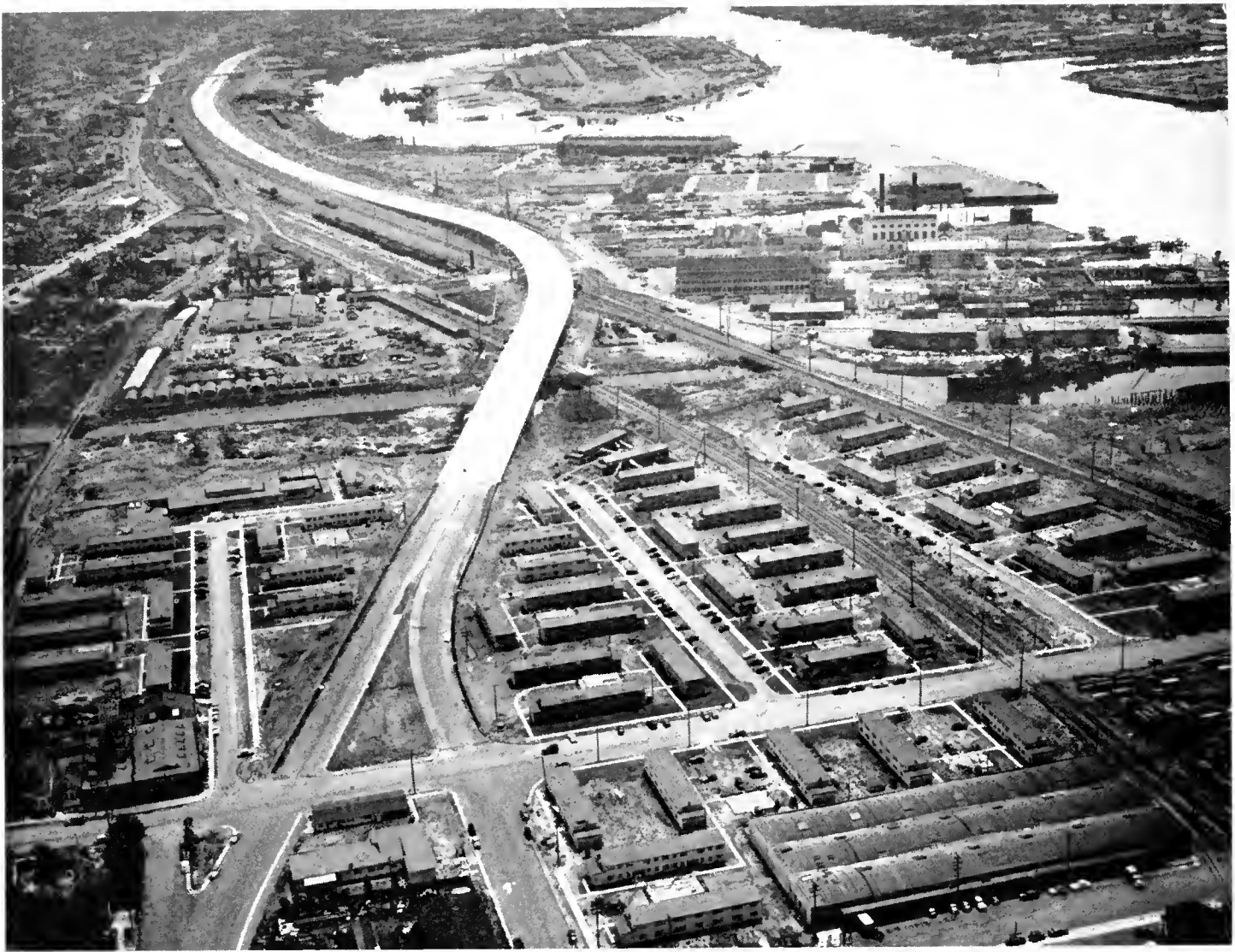
Eastshore Freeway, looking south from temporary connection to Oakland city street system at Fallon Street. In center is 5th Street structure over Western and Southern Pacific Railroads and Lake Merritt Canal in center
