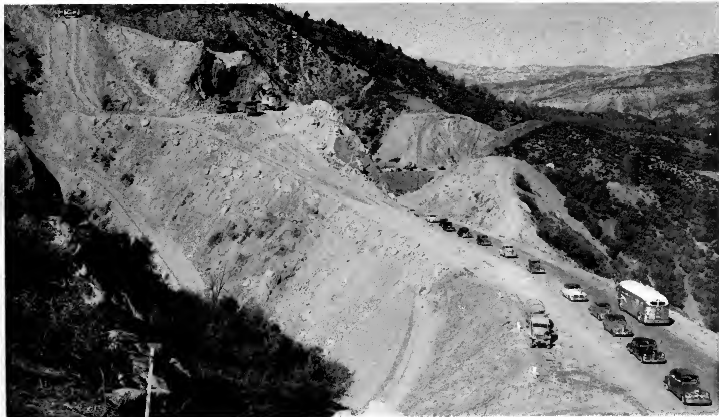
Controlled traffic using Ridge Route while heavy grading is in progress
