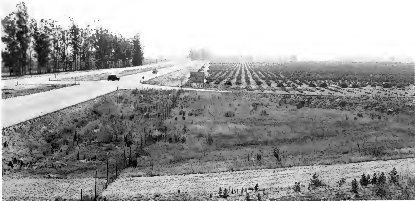
Looking westerly showing vineyard adjacent to north right of way line, right of way fence, and area used for private hauling road
