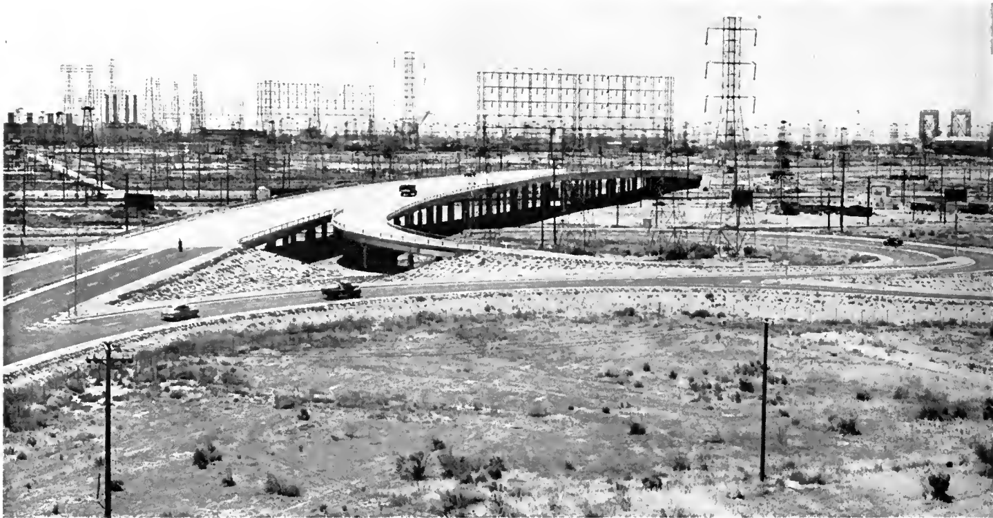
Looking south toward Anaheim Street Viaduct showing off and on connections to freeway
