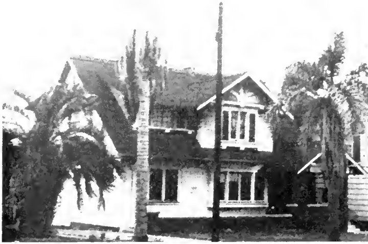
BEFORE —This typical old, two-story building was located at 1422 Bellevue in the right of way of the Hollywood Freeway.
