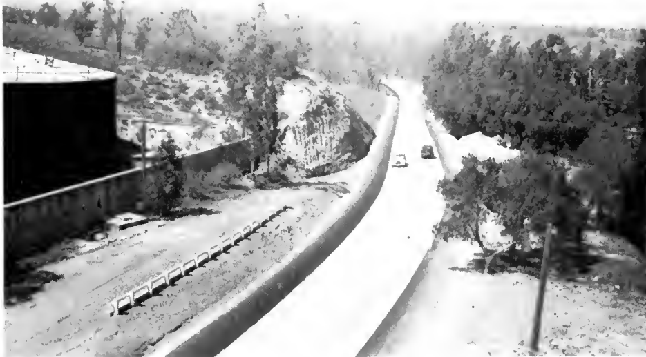
On Crestmore Road, looking northerly toward spur track crossing. Old reverse curves on left and behind tree on right
