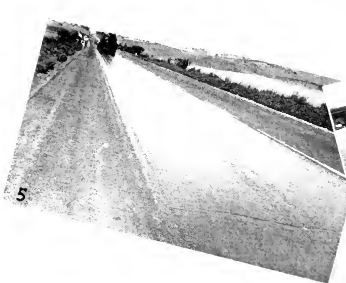
1—A tray representing one square yard placed on pavement to determine uniformity of distribution of screening spreader. 2—A newly completed seal coat. 3—Screenings being applied to the surface with a mechanical spreader. 4—Distributor truck starting spread of asphalt. 5—Freshly applied asphalt immediately following passage of distributor. 6—Screenings being rolled with a tandem roller
