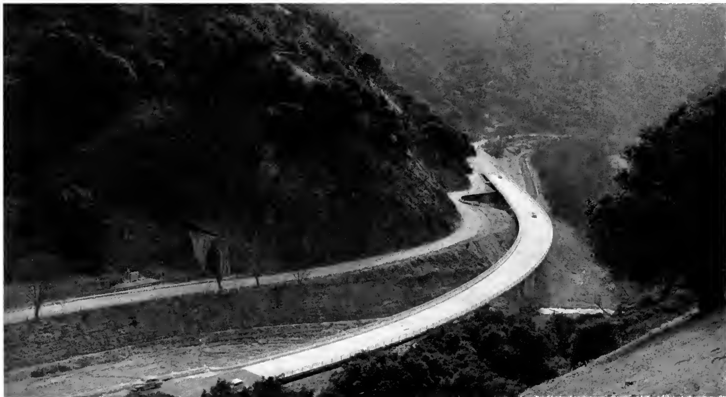
This is the new $450,000 Alameda Creek Bridge and overhead four miles east of Niles in Alameda County
