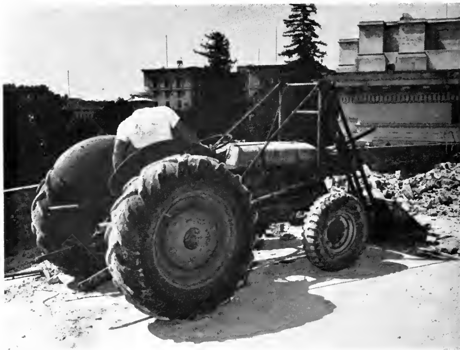
Tractor operating on fourth floor of Capitol during demolition operations
