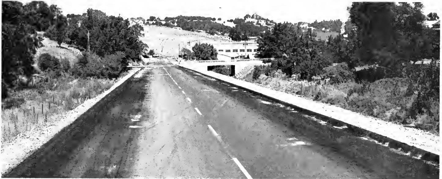
The new bridge in the background is at the junction of the Carson Pass Highway and the Mother Lode Highway on the new alignment
