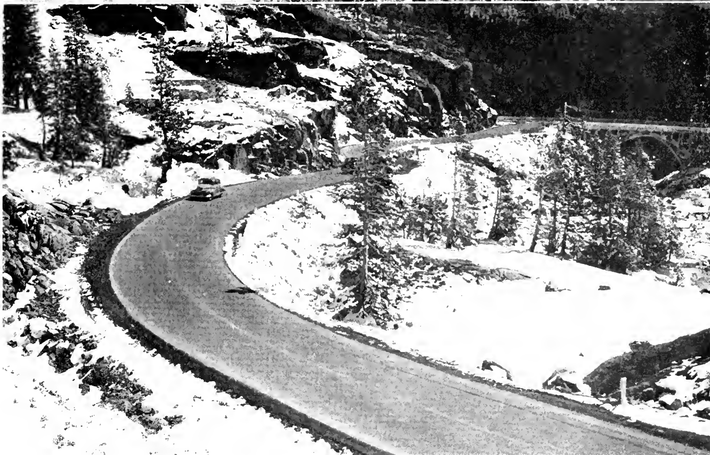
UPPER—View of Flycasters Curve, looking east, which is to be widened. LOWER Curves will be eliminated on this section of U. S. 40, looking east near Donner Summit, with Donner Summit Bridge in background
