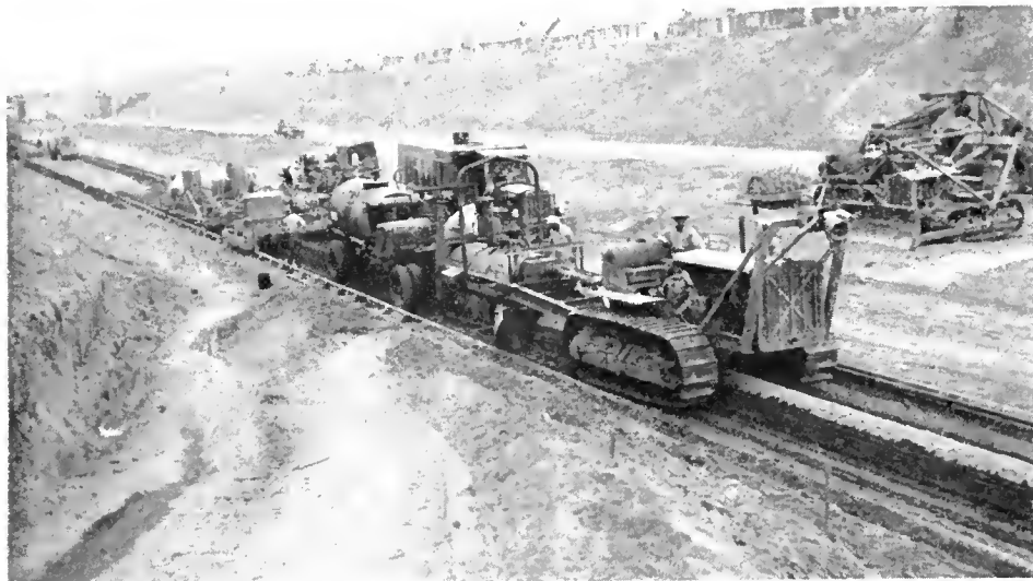
Upper—Mixing and spreading cement treated base
