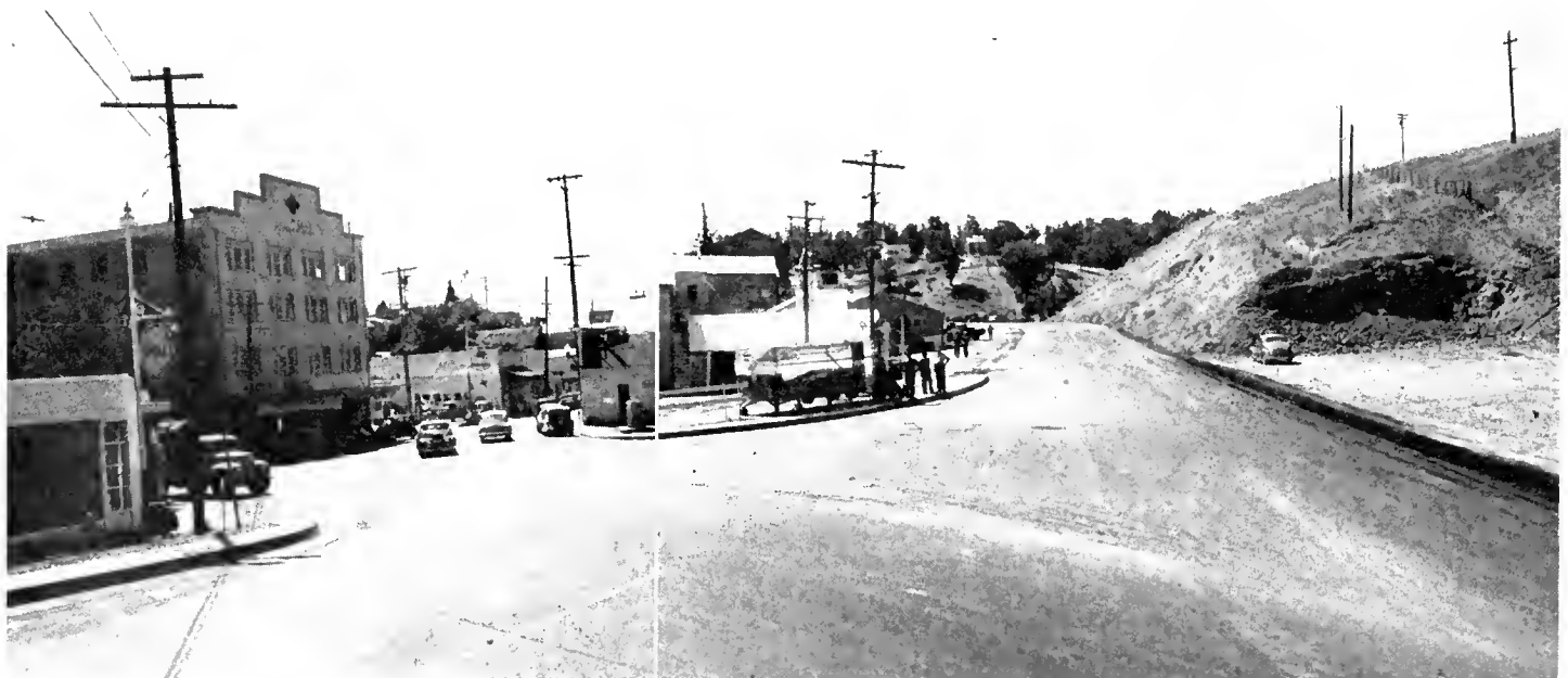
This photograph shows the existing entrance into Jackson on the left and the new alignment on the right
