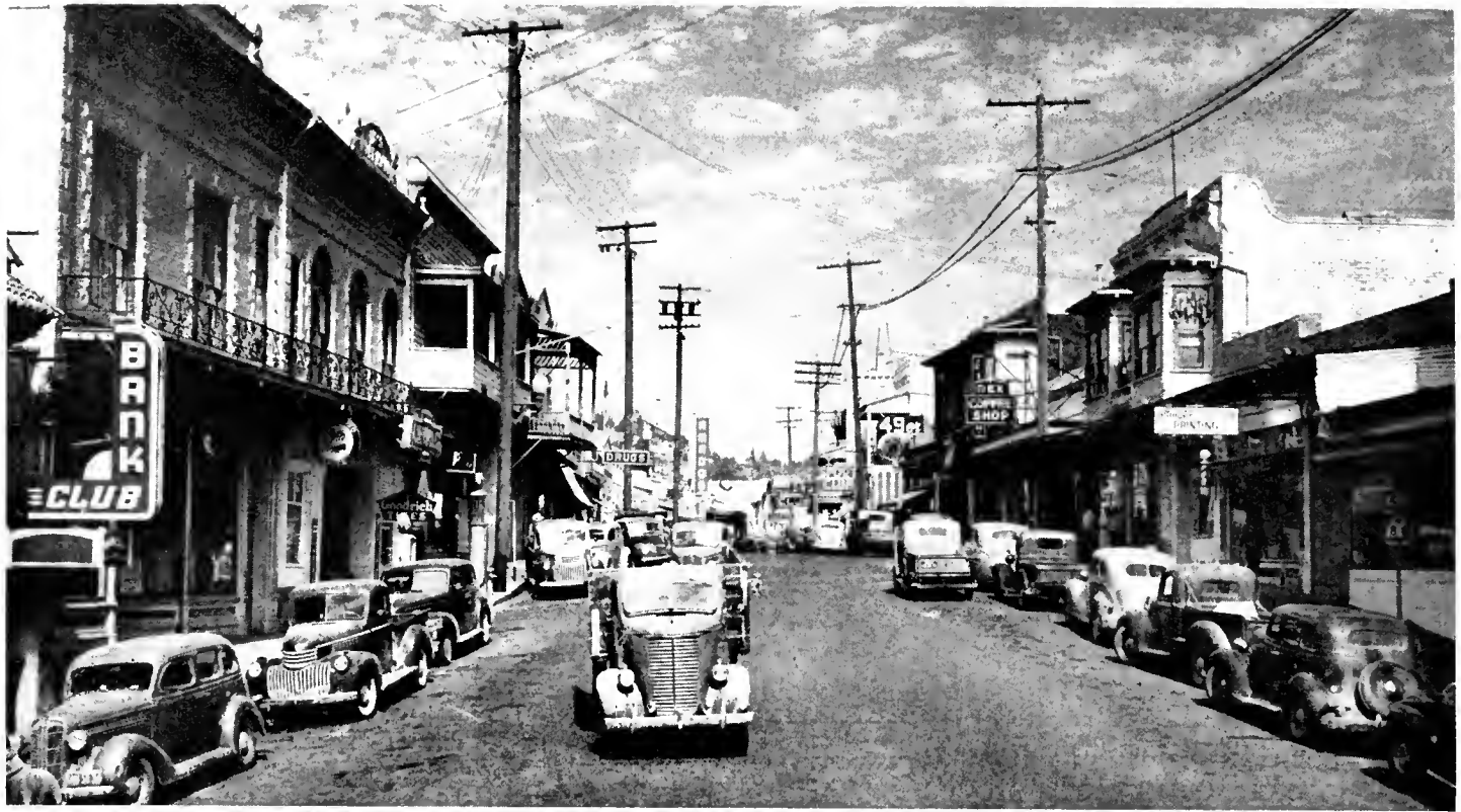
This congested route through Jackson was the only one available until new highway was built
