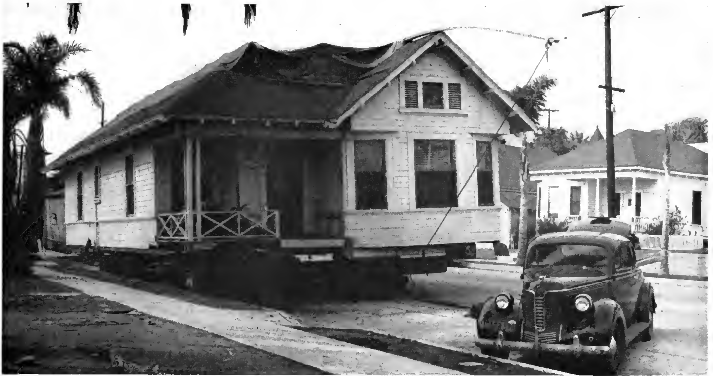
This five-room frame dwelling has just left the old location at 1456 Bellview Avenue, within the limits of the Hollywood Freeway right of way, and will soon be completely rehabilitated, modernized, and again in occupancy by a family. This procedure minimizes the affect of freeway construction on the housing shortage in the metropolitan areas
