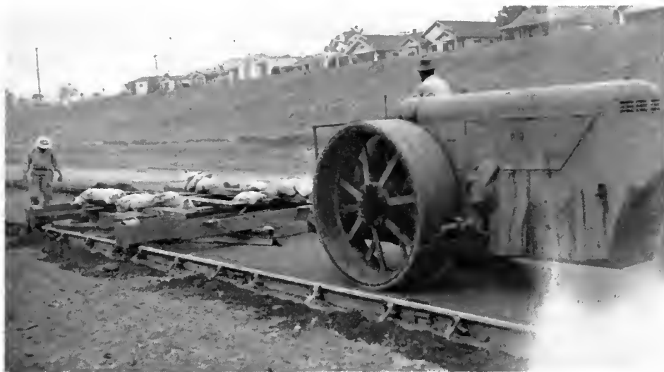
Cutting subgrade to finish grade
