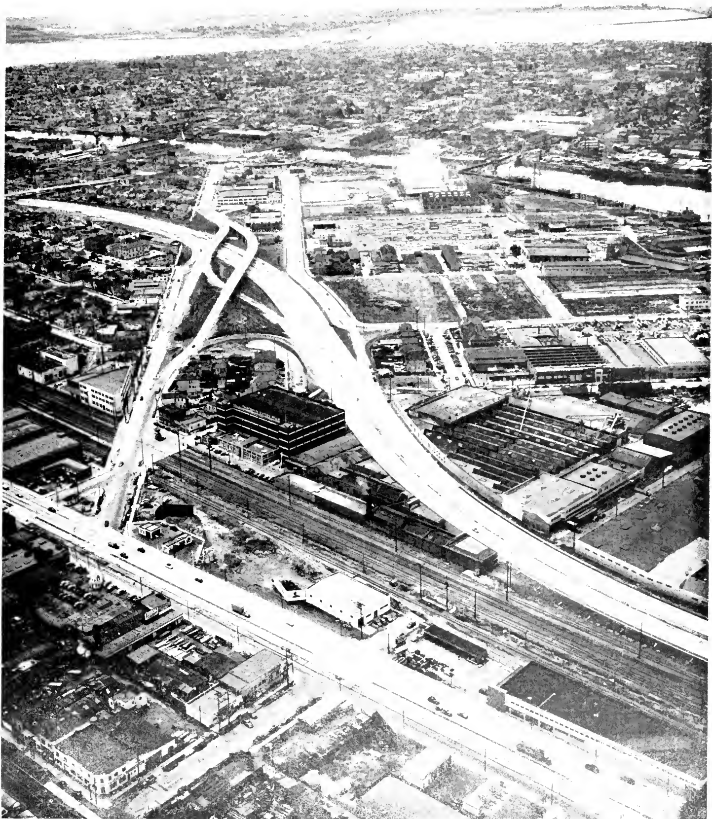
Aerial View of Eastshore Freeway Looking south, showing 23rd Avenue Overhead and Kennedy Street approach
