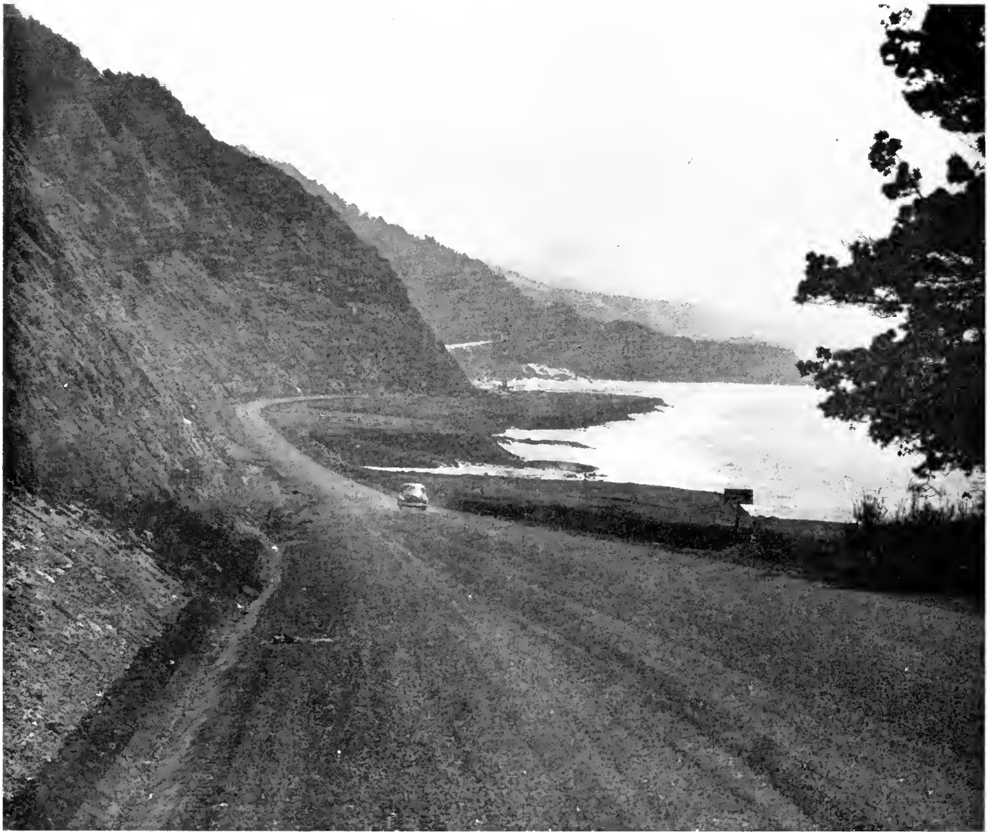
When this picture of the new Waddell Bluffs Highway was taken, paving and striping were about to begin
