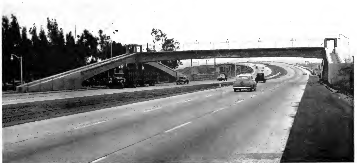
Pedestrian overpass in South San Francisco, showing 120-foot clear span across new Bayshore Freeway
