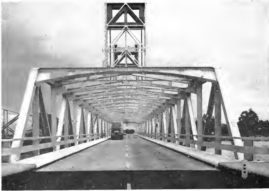
Looking southerly along bridge. The new bridge roadway is 26 feet in width with two 3-foot 6-inch sidewalks
