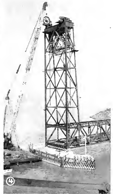
4—Erecting 10-foot diameter sheave on top of tower
