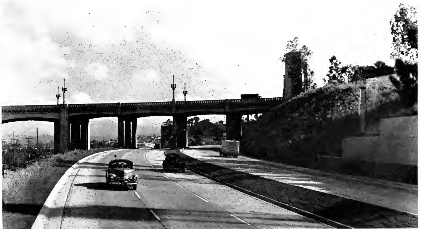
Santa Ana Freeway looking northerly, showing the Sixth Street Viaduct
