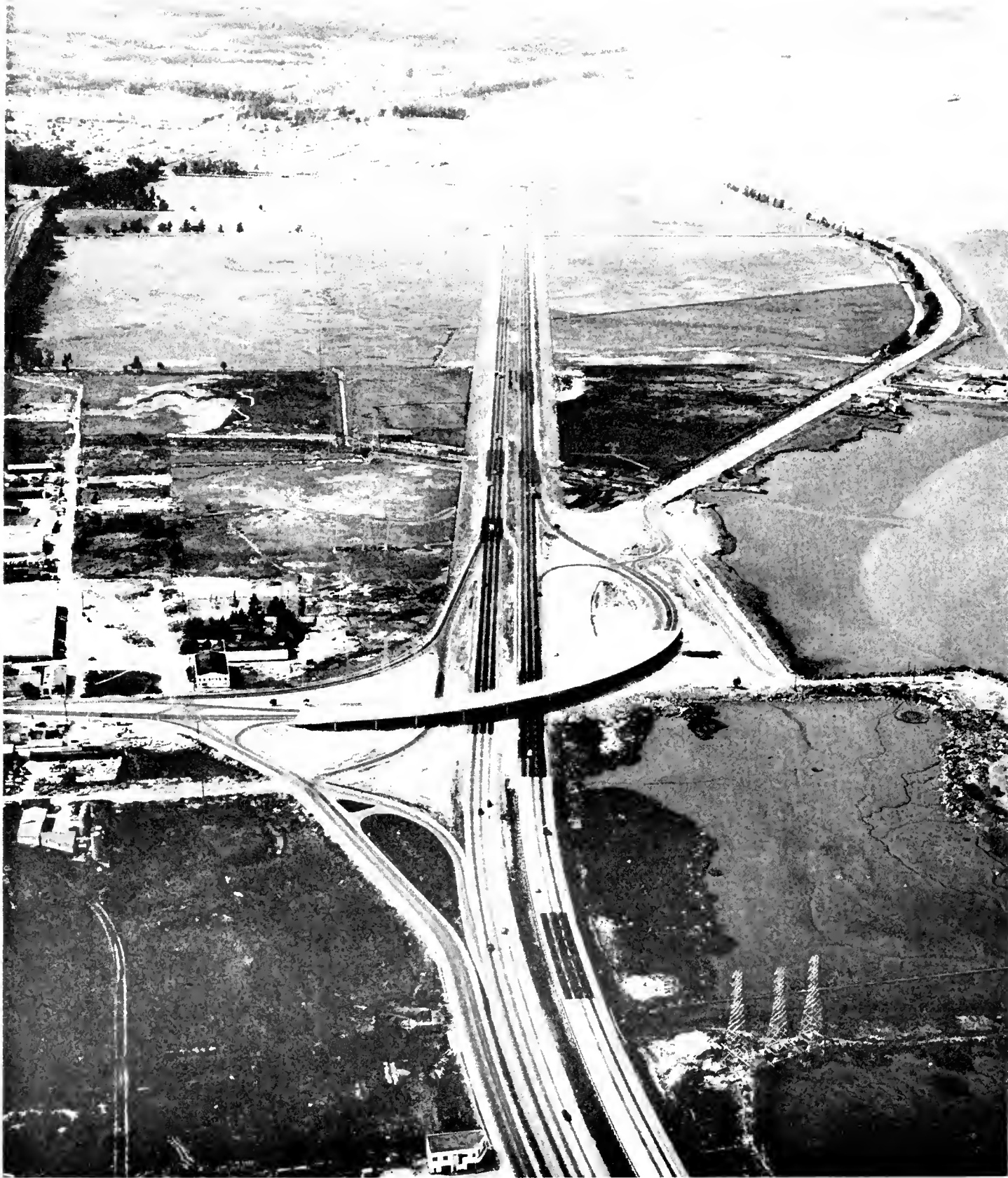
Broadway overcrossing in Burlingame looking north. Old Bayshore Highway is on right
