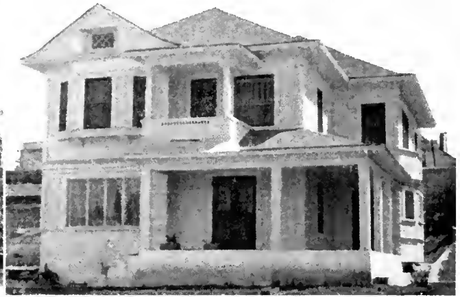
AFTER —This building is now located at 226 North Westlake in Los Angeles. A slight change in the porch and the new paint job give the residence a much more pleasing look.
