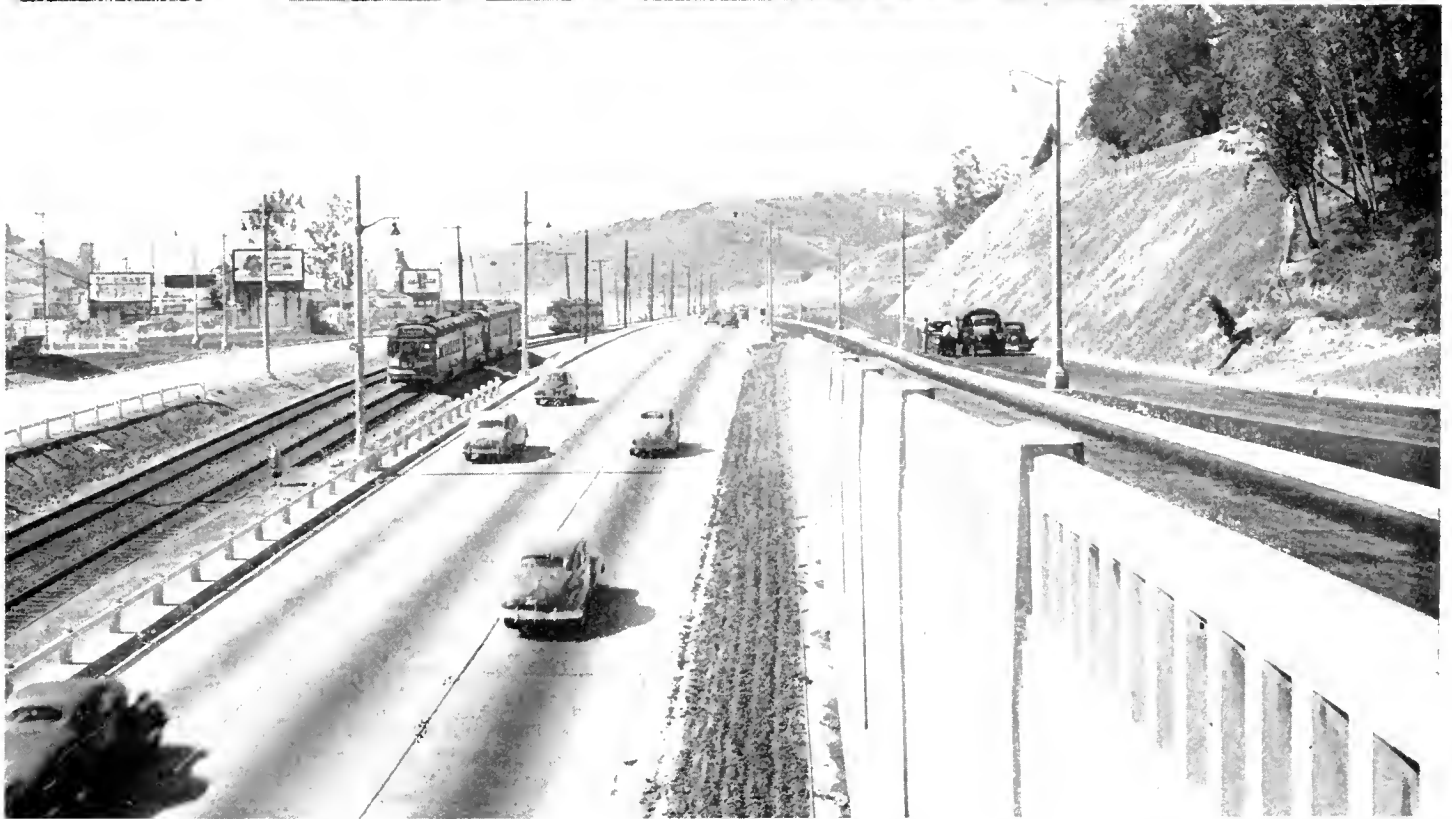
Upper—Completed freeway looking northeasterly from Barham Boulevard and showing fence constructed to protect pedestrians. Lower—Looking northwesterly from Barham Boulevard showing completed freeway with provision in the center for rail rapid transit
