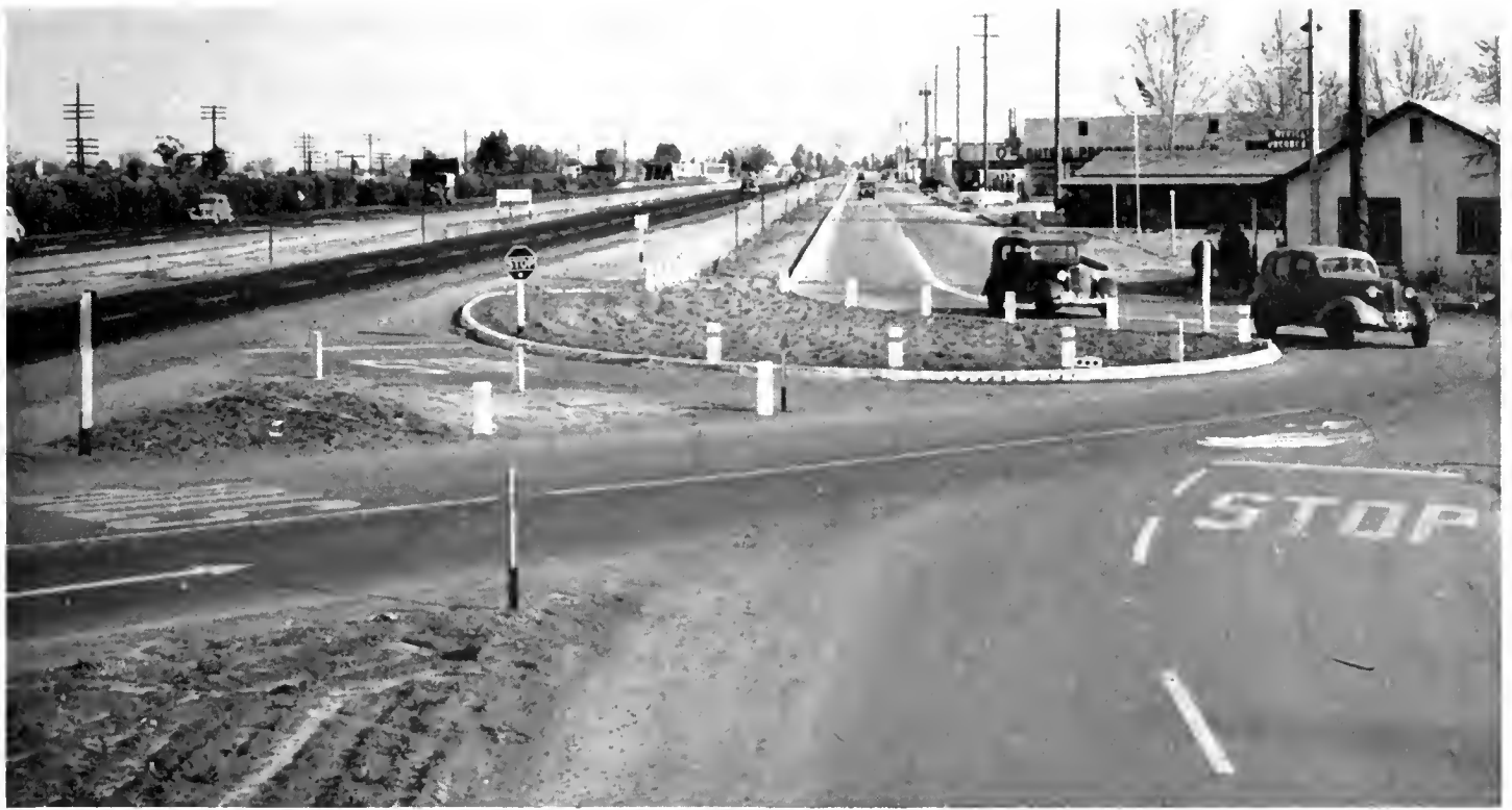
Photo E —Typical outer highway installation adjacent to multiple-lane limited freeway improvement on U. S. 99 at Malaga, a short distance south of Fresno
