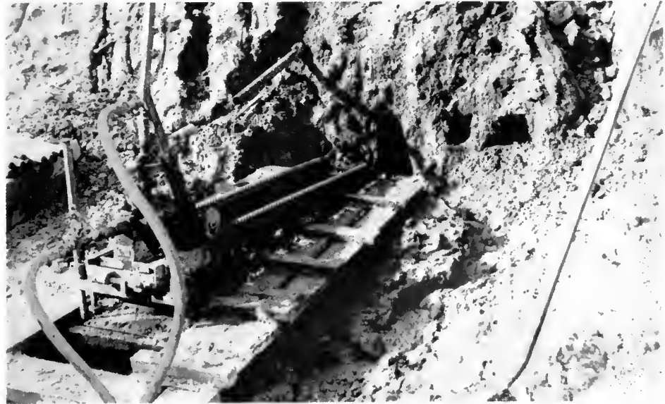
Drilling slide at Camp Cajon with hydrauger
