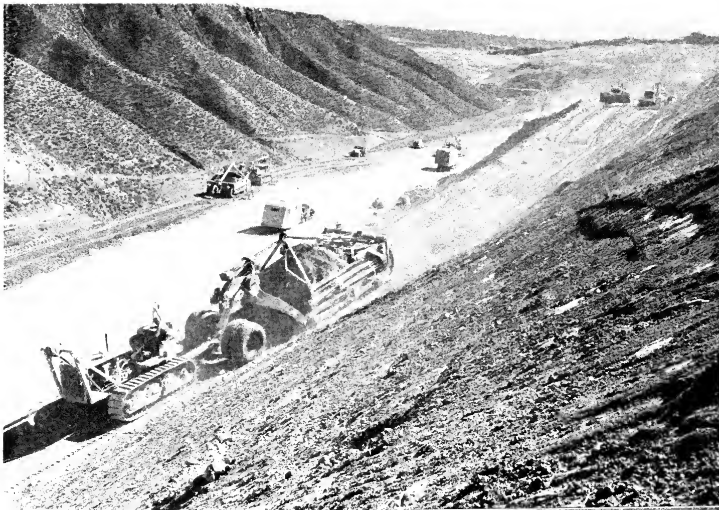
Two views of heavy excavation cut operations on new Ridge Route Highway
