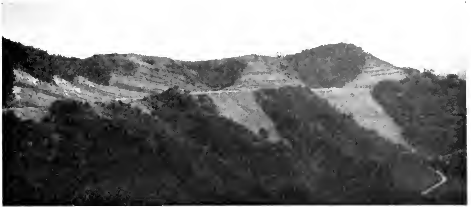
Extensive cut and fill area exposed to erosive forces by construction of this high-standard mountain road. Compare with old road at lower right. (Near San Marcos Pass above Santa Barbara)
