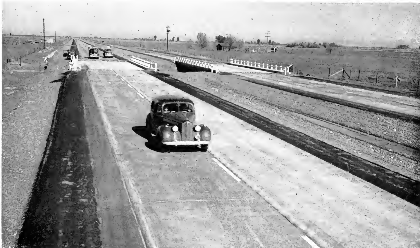
This photograph was taken north of Midway looking toward Dixon and shows bridge units which converted this section of US 40 into a four-lane divided highway
