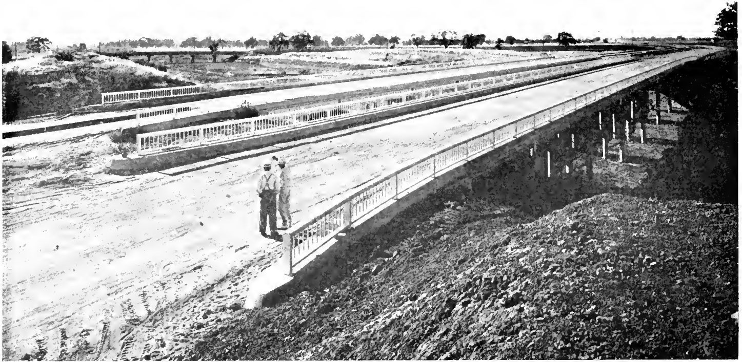
Looking north across diverting canal bridges. Lackeford Road Bridge on left
