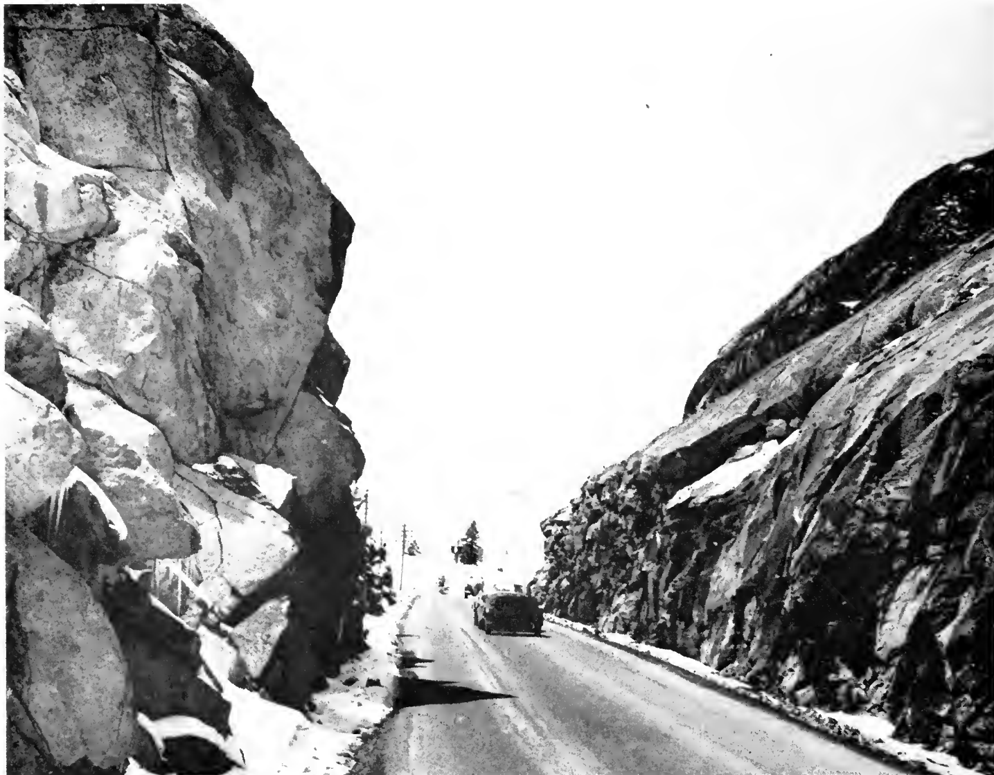
Looking west of rock cut to be widened at Donner Summit
