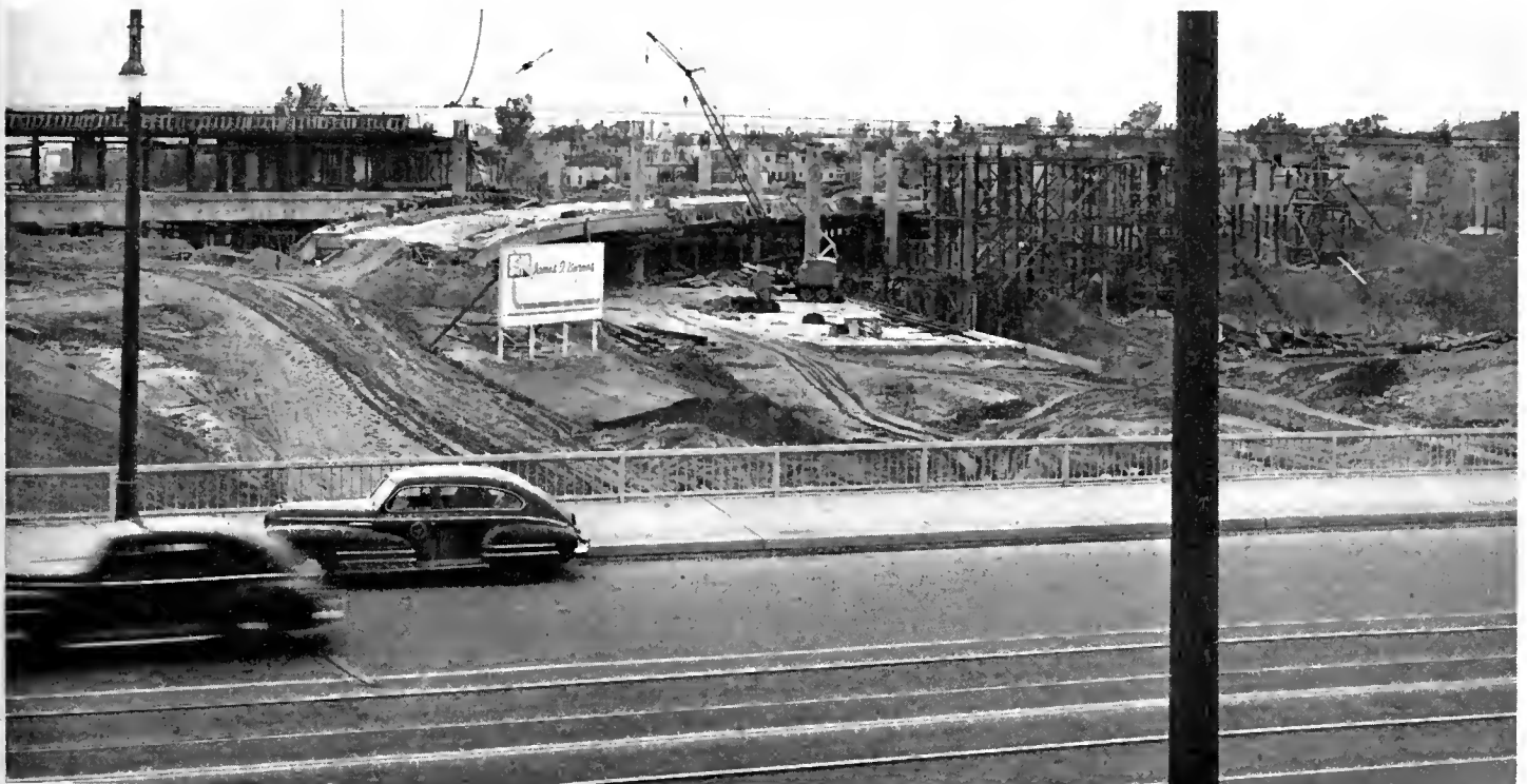
Four-Level structure looking south from the completed Sunset Boulevard Bridge over the Arroyo Seco Parkway
