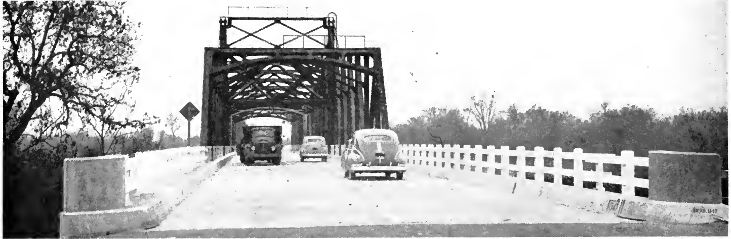
Traffic begins using newly dedicated Butte City Bridge
