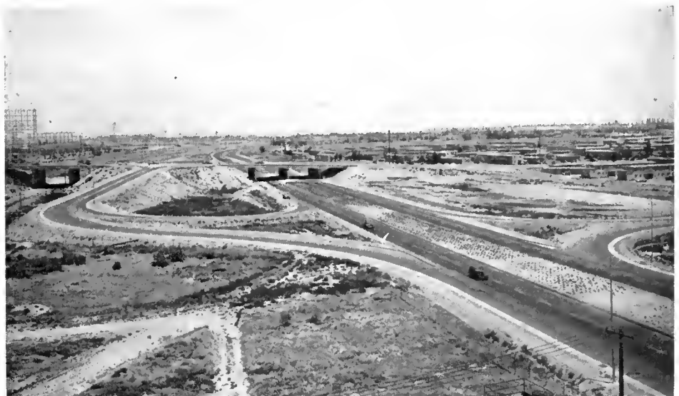
Looking north toward Pacific Coast Highway (US 101 Alt) grade separation over freeway, with Claverdale connections in foreground
