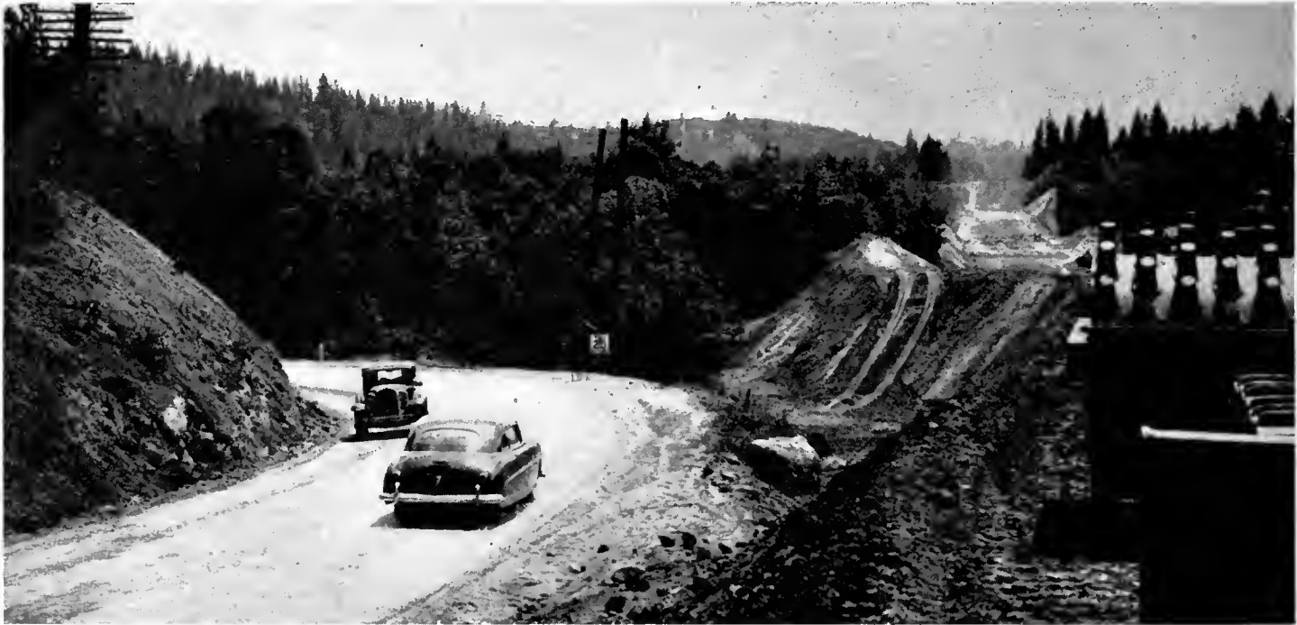
Beginning of construction of new four-lane divided highway on U. S. 40 between Applegate and Auburn in Placer County. Existing highway on left, grading for new location on right, looking west from Applegate
