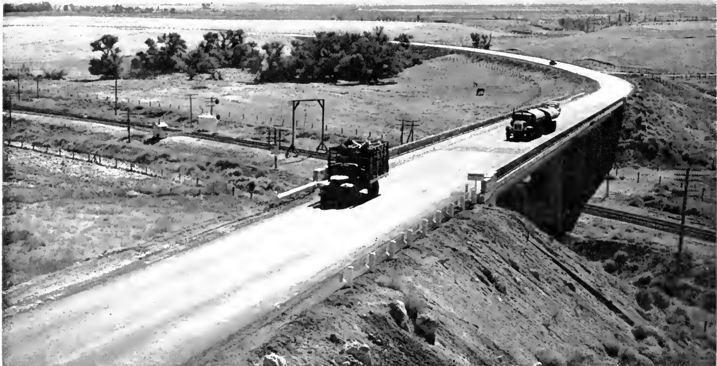
This view shows new Keene-Tehachapi highway crassing Tehachapi Overhead
