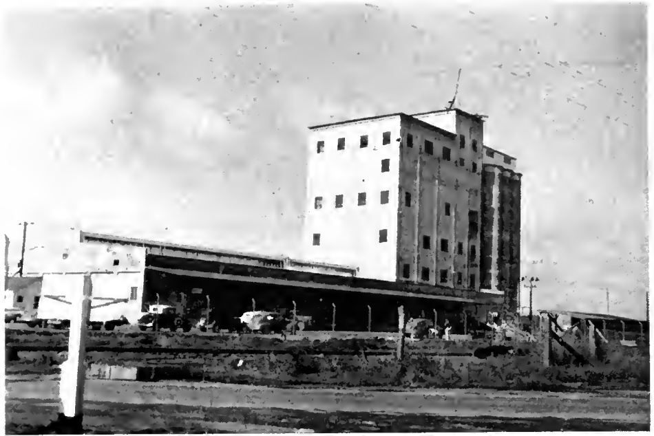
Large concrete office and warehouse structure of the San Joaquin Valley Poultry Producers' Association was constructed upon one of the parcels investigated subsequent to development of the freeway
