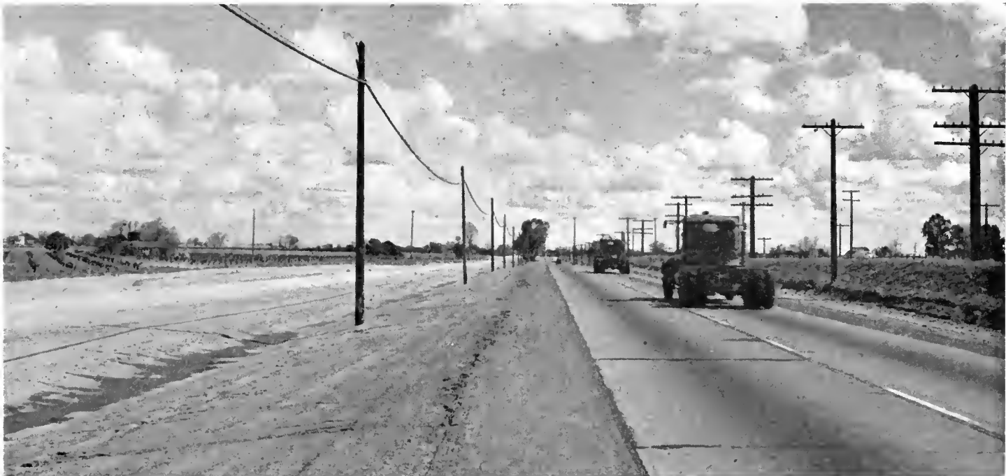
Looking toward Livingston from south city limits showing new four-lane divided highway
