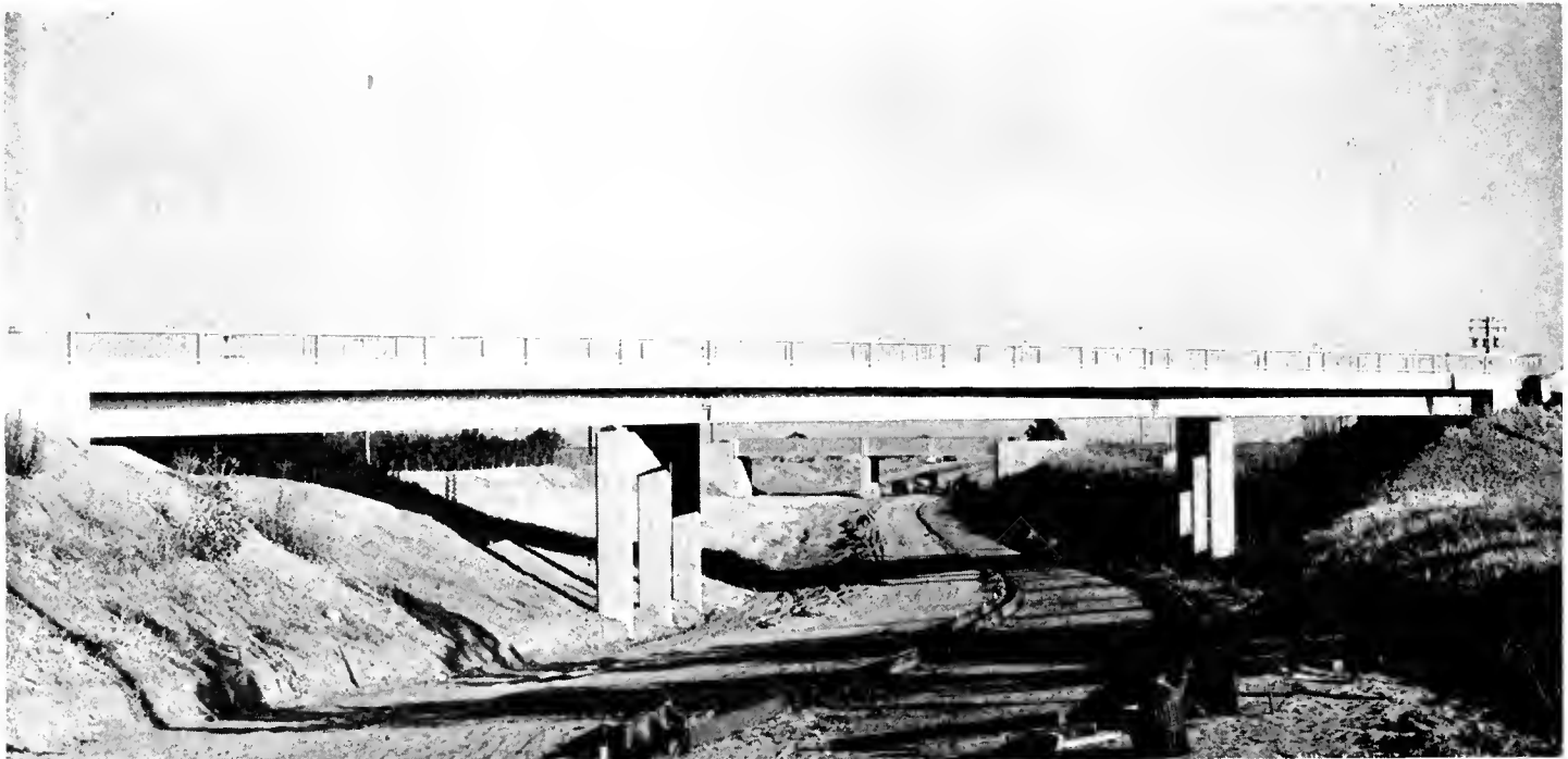
Looking south from separation of Wilson Way. Central Cali'arnia Traction Company railroad underpass in background
