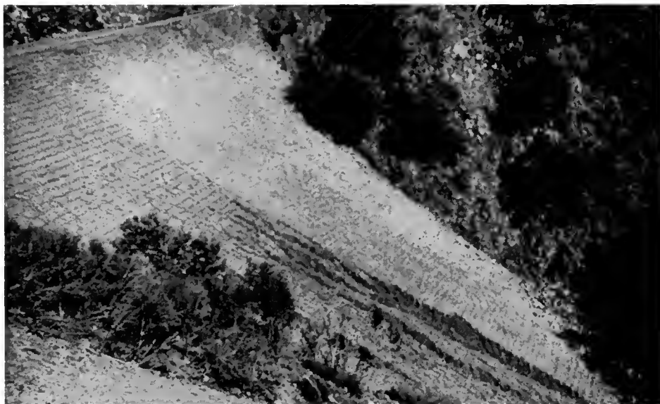
An early experiment in wattle spacing. Wattles widely spaced on left half of slope, closely spaced on right half. (Angeles Crest Highway, Los Angeles County)
