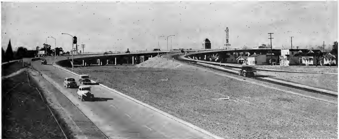
Looking from west end of California Avenue overcrossing. California Avenue off-ramp at left and on-ramp at right. Future West Fresno Bypass will pass under first and third span of structure at left center
