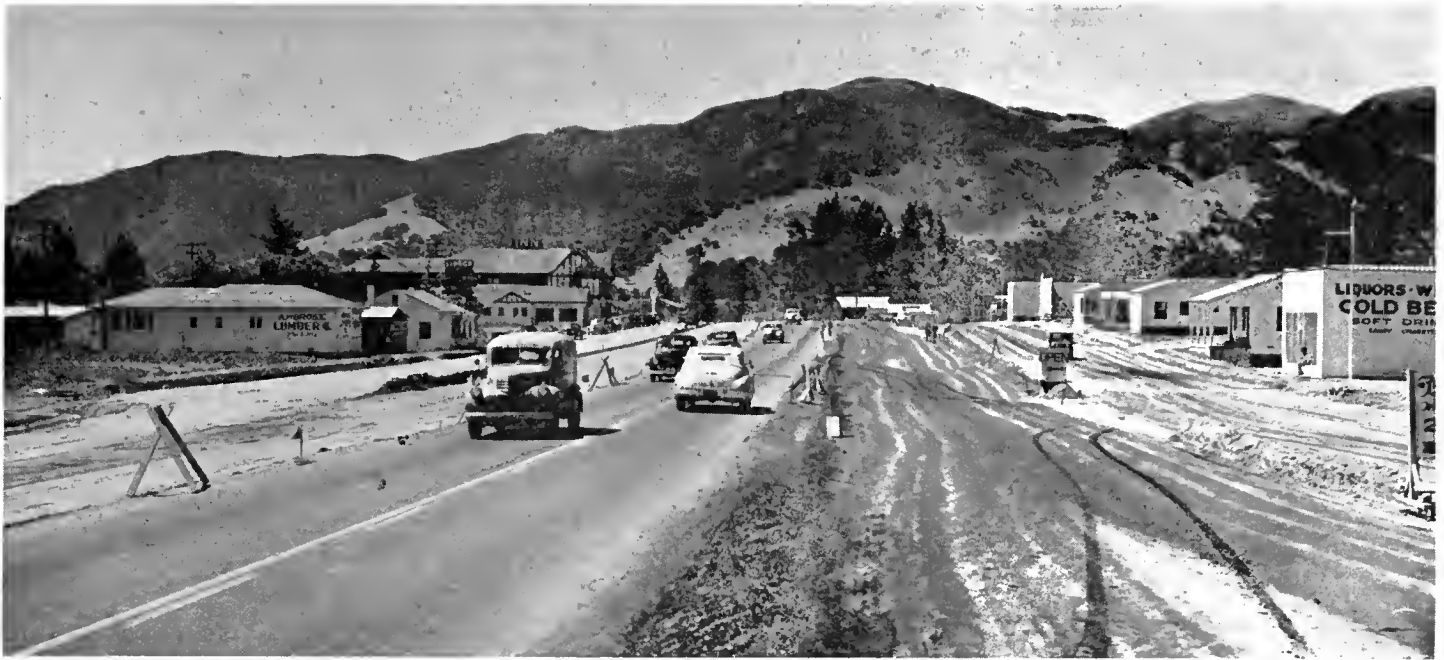
This view is looking southerly through Buellton, showing relocated buildings
