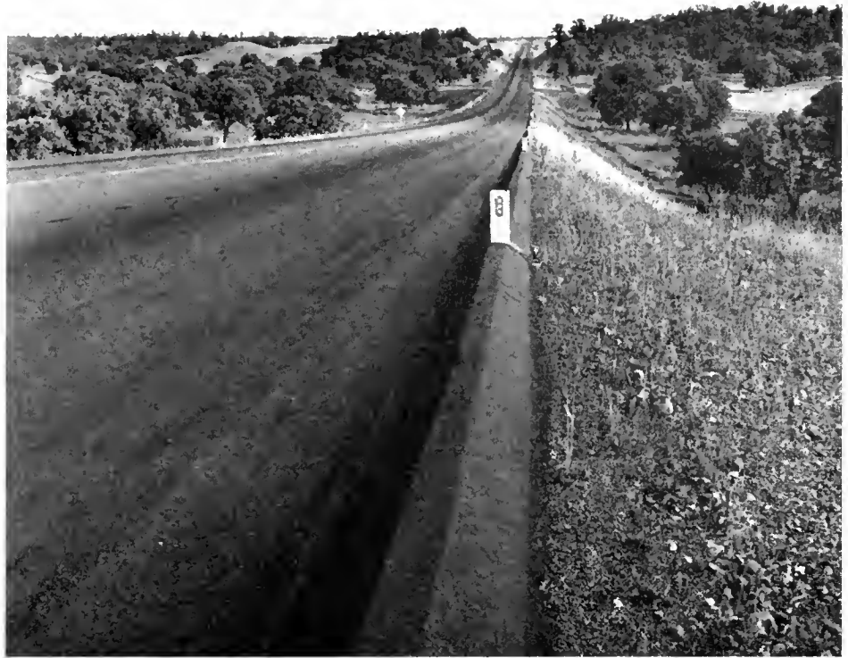
Four lanes tapering to two with machine-shaped and finished drainage dike and reflectorized guide posts
