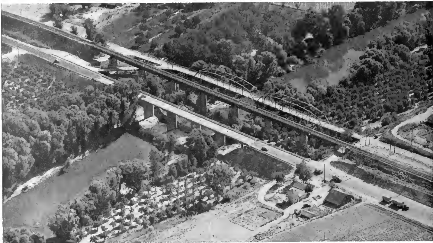
New bridge in foreground replaces 38-year-old structure across Tuolumne River, one mile south of Empire in Stanislaus County
