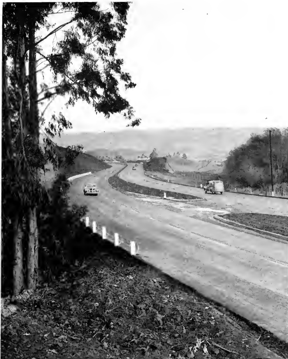
Freeway relocation of U. S. 101 south of San Luis Obispo looking north toward Santa Lucia Range
