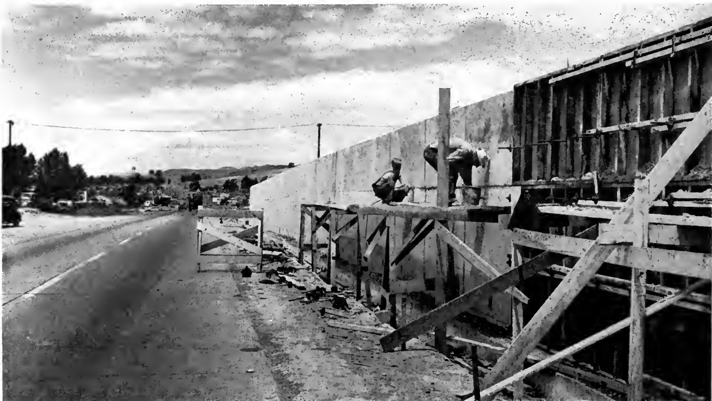
Constructing retaining wall between main highway, U. S. 40, and outer highway
