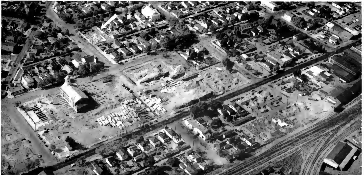
The church move from the air. Note the church on rails. The old foundation with part of the cribbing in left foreground; the new foundation being readied on the next street above as indicated by arrow
