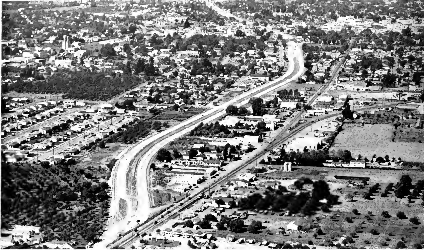
Aerial photo looking north from intersection of new freeway and existing highway south of Santa Rosa. This was taken in October, 1948, when grading was completed and paving started north of Santa Rosa Creek only, and clearly shows the new freeway in comparison to the old route through town
