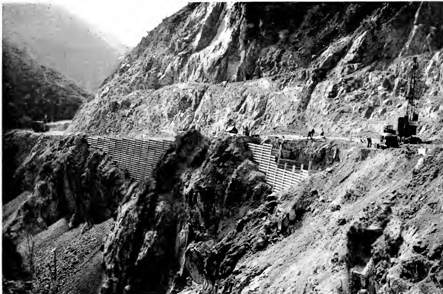
On a precipitous rock slope above the bed of City Creek on the First Unit are these two bin-type retaining walls. The one on left is completed, the one on right under construction. Remains of old road appear above
