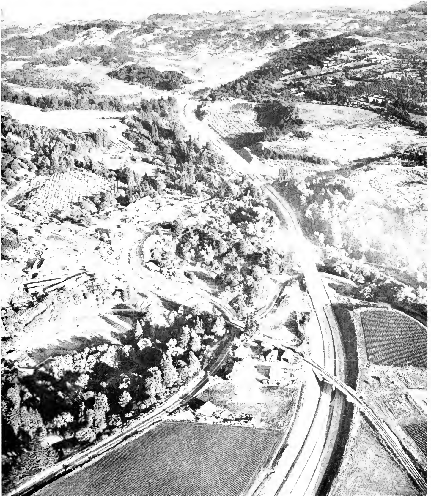
Aptos Creek Bridge looking toward South Aptos Railroad Underpass with North Aptos Underpass in the foreground. Town of Aptos in left center
