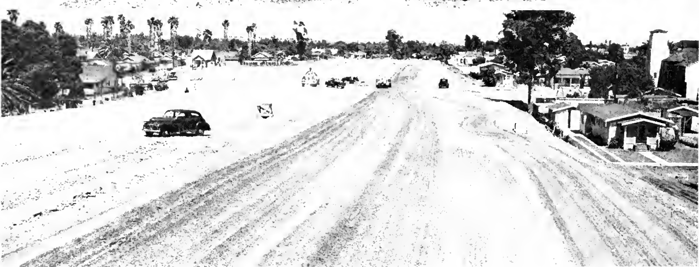
Upper—View looking west of Indiono Street grade separation, showing earth-moving and compacting equipment at work. Center—View looking east from Euclid Avenue grade separation, showing construction work in progress. Completed Larena Street grade separation in background. Lower—Looking east from Indiono Street grade separation showing Eastman Avenue, the easterly terminus of the contract in the background. Grading is complete and roadway ready for subgrade and paving operations
