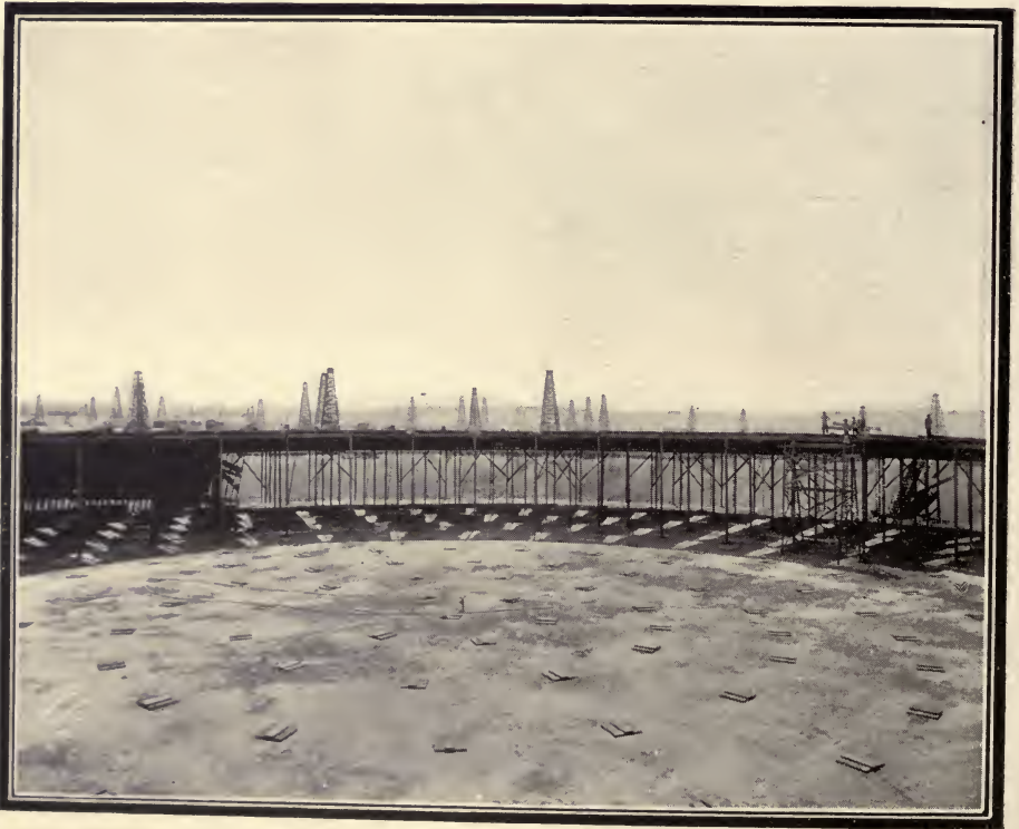
Interior of an Oil Reservoir (Under Construction)
