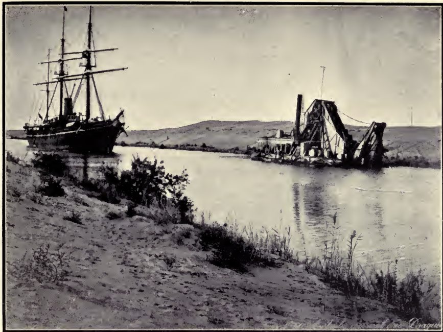
One of the dredgers at work.
