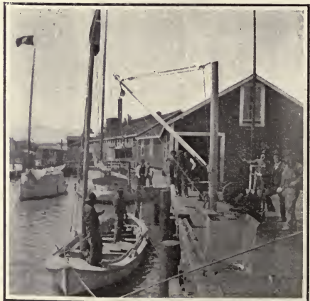
Hoisting fish. Superintendent Croxon at hoist.
