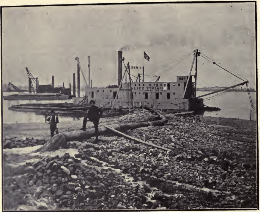
Dredging Gravel and Cobblestone.
