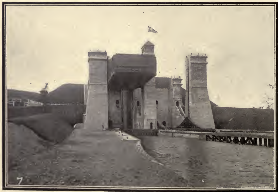
The locks at Peterborough, Ont., showing one Hydraulic lift down and the other up
