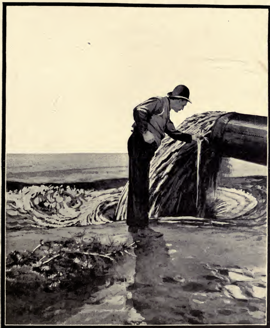
Capt. Alex. Watt, Part Owner and Manager, examining character of spoil.
