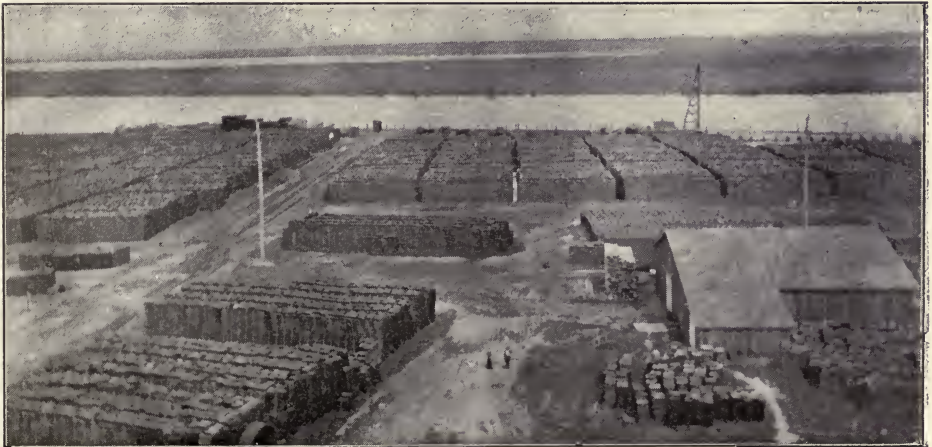
Shingle Yard at Los Medanos
