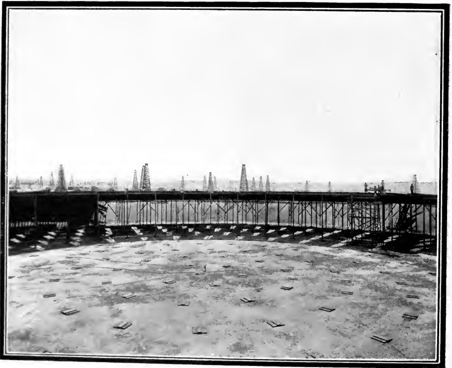
Interior of an Oil Reservoir (Under Construction)
