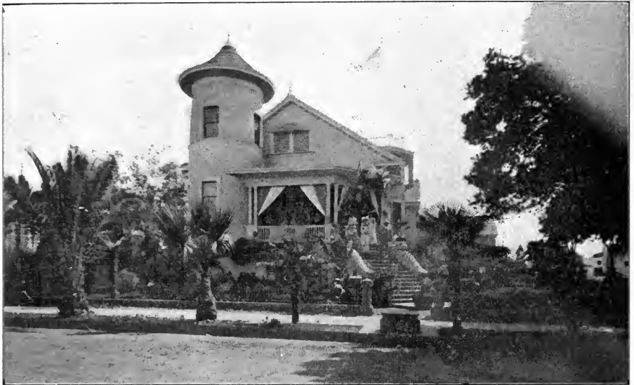
Residence of Dr. Chas. W. Decker, Palo Alto
