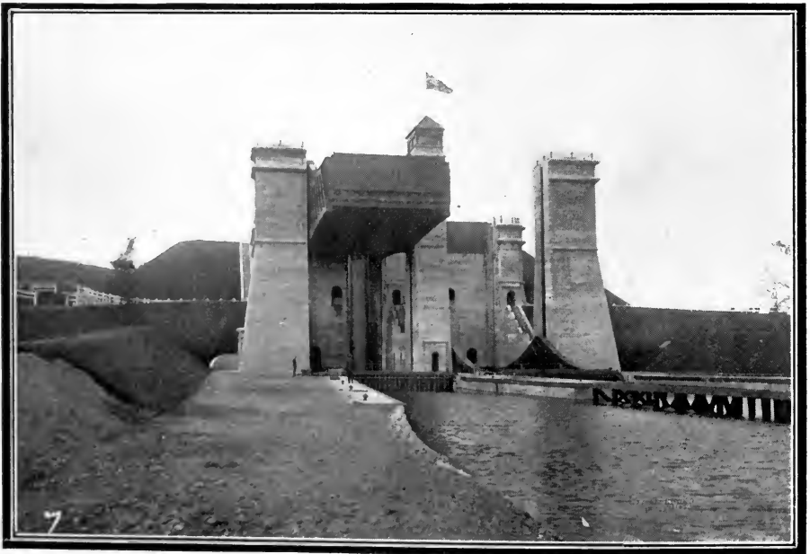
The locks at Peterborough, Ont., showing one Hydraulic lift down and the other up
