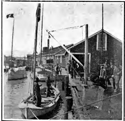
Hoisting fish. Superintendent Croxon at hoist.
