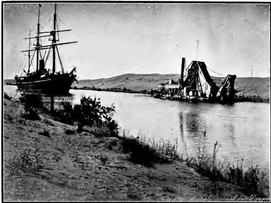
One of the dredgers at work.
