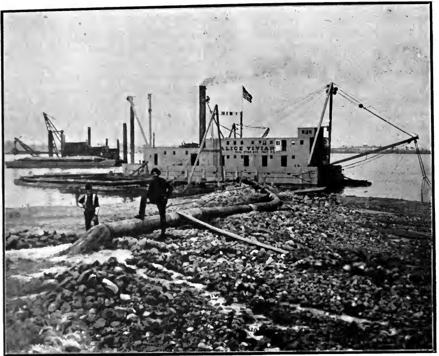
Dredging Gravel and Cobblestone.
