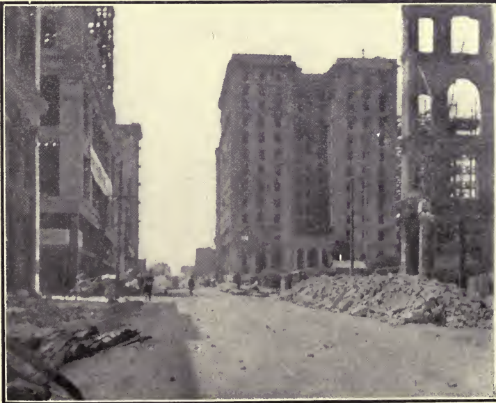
View of St. Francis Hotel. This building was gutted by fire. The building was not so badly injured but that it will be repaired.
