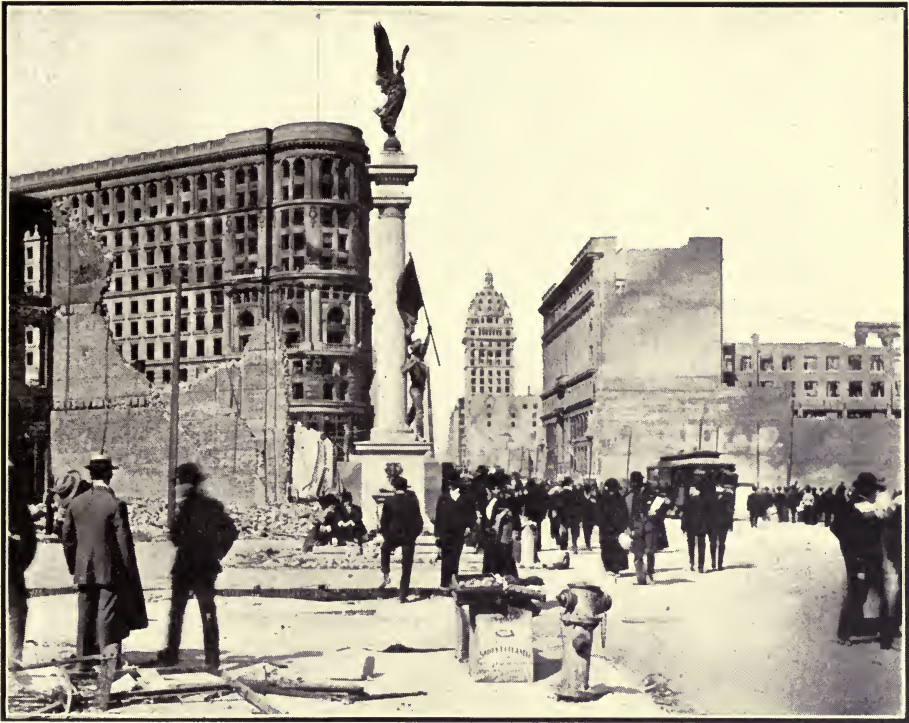
Looking east down Market street, showing James Flood building, Native Sons' monument, Claus Spreckels' building, and Emporium. All but the last are not seriously injured.
