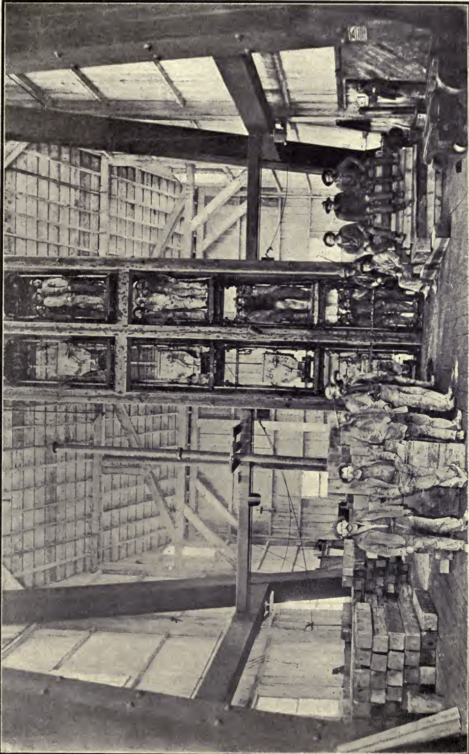
Four-deck cage, Anaconda mine, showing miners going "on shift," and empty ore cars.
