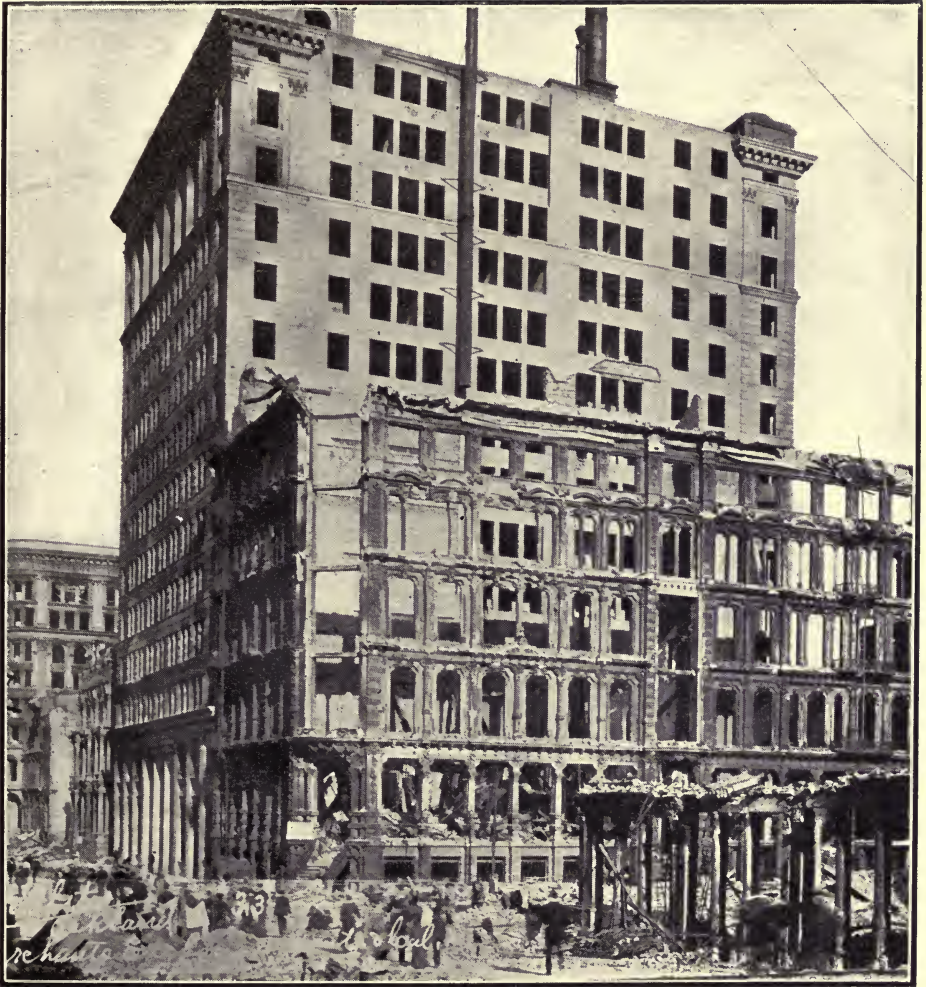
Merchant's Exchange Building on California street, San Francisco, after the earthquake and fire. In the foreground is the California Safe Deposit Building, completely ruined by the fire. In background is the Mutual Life Insurance Company's building on Sansome and California Streets.
