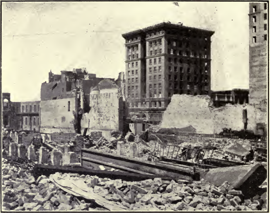
Front of the Kohl building. This building is but slightly injured by fire, and is now occupied by tenants. Fire raged all around it.
