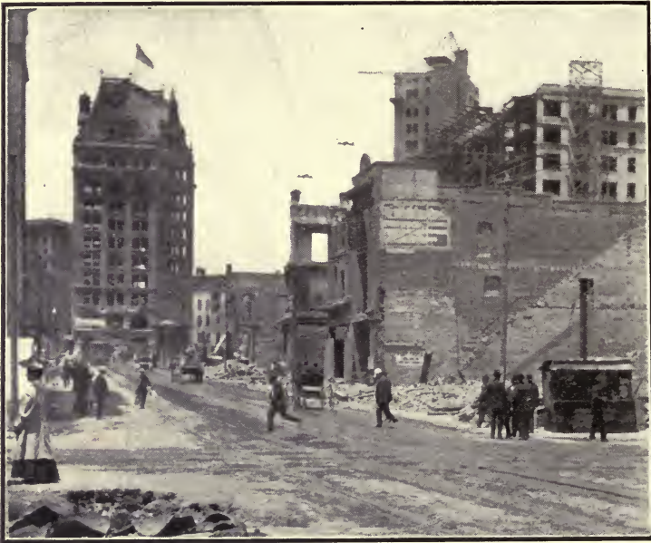
Mutual Savings Bank, taken from Third street. A steel structure with gray sandstone facing that stood the fire in fine shape. New buildings rising on the right of picture, the highest of these being the new Chronicle building.
