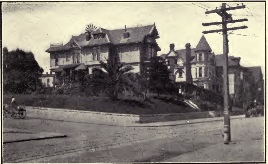
Residences on Pacific avenue. This picture shows how little damage was done by the earthquake. Chimneys are still standing and concrete garden walls are uninjured.
