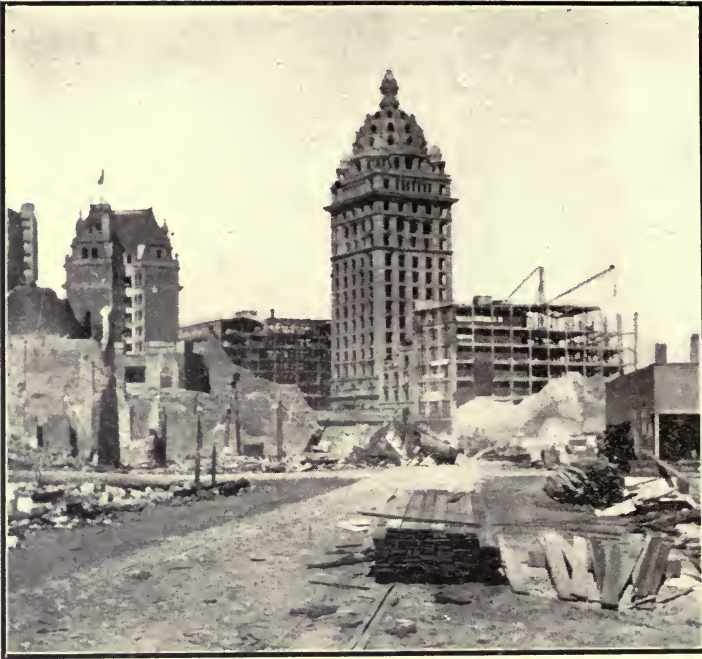
View of Call building, looking from Geary street. Building operations are going on in all directions.
