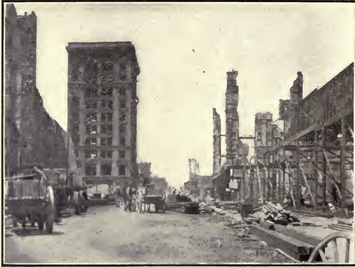
View of Shreve Building, looking down Grant avenue.
