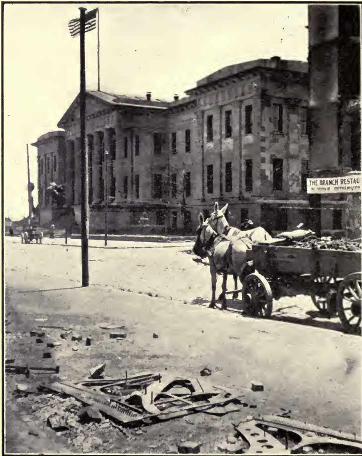
The U. S. Mint, which is unhurt by fire or 'quake. This is an example of a well-built edifice. All of the Government buildings in San Francisco were saved, not because of an especial effort to do so, but because of superiority in construction.
