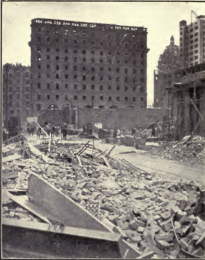
Crocker building, from Montgomery street. A granite, steel, brick and terra cotta building; will be re-occupied after repairs. On the right may be seen the Call and the new Chronicle buildings.
