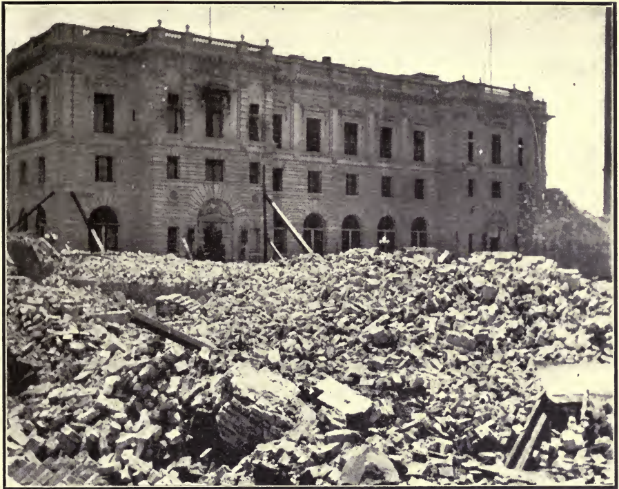
View of Post-office, looking from Market street. The building in the foreground, was shattered by dynamite to save the Post-office, and the damage on the Government building was by earthquake and dynamite only.
