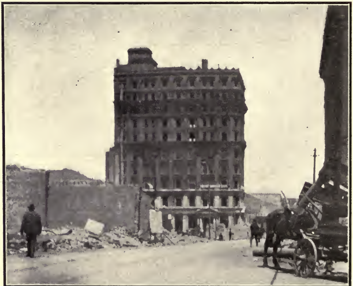
Union Trust Building, Montgomery and Market, looking down Post street. Fire raged all around this modern steel, brick and terra cotta building, but without inflicting serious injury to tenants' belongings. The wall on the left is what is left of the Masonic Temple.
