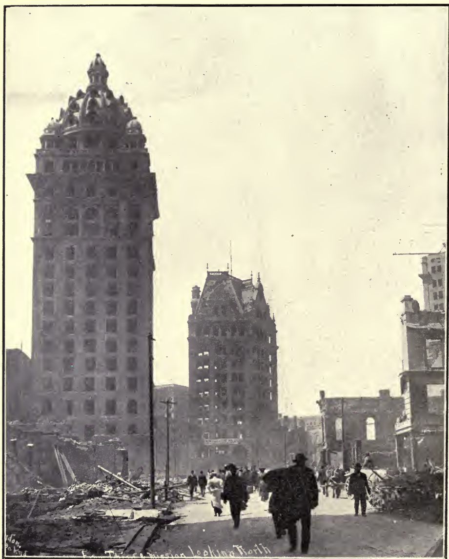
Looking N. W. from Third and Mission streets, San Francisco. Claus Spreckels and Mutual Savings Bank Buildings of steel, concrete and granite, gutted internally, but sound structurally.
