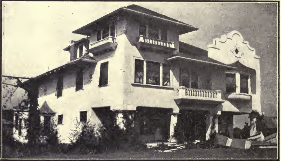
“The Chi Psi Lodge had skated off its foundations.”
