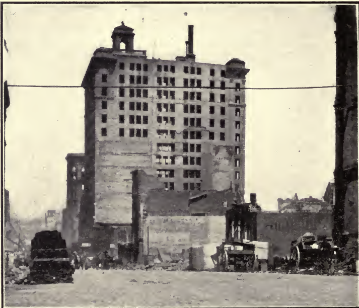
The Merchants' Exchange, partially occupied and being remodeled.
