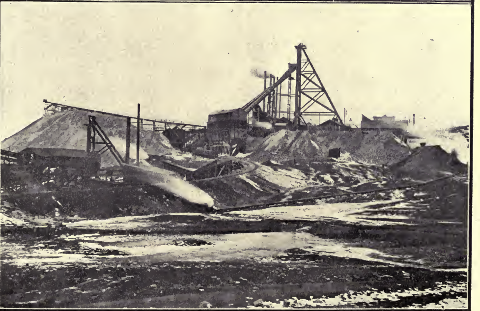
1. Bell and Diamond mines. 2. Cora mine, showing hoist and dumps.
