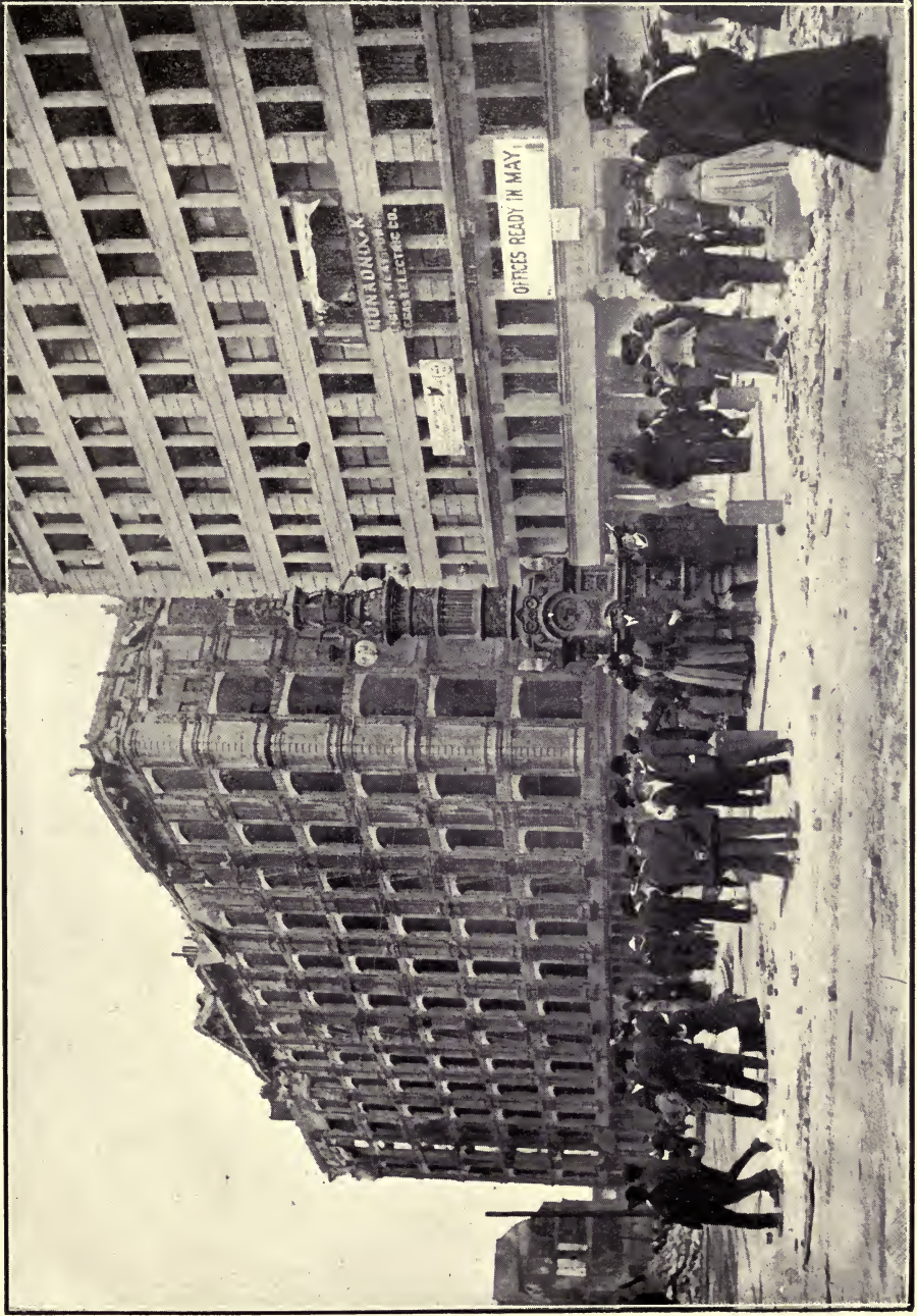
The Palace Hotel, San Francisco, for many years the largest in the world, gutted by the flames. Next to it the Monadnock, a modern steel and concrete structure, not greatly damaged.
