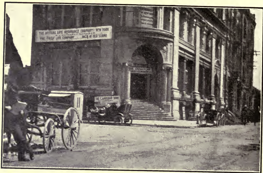
Canadian Bank of Commerce, occupying the ground floor of the Mutual Life Insurance Co. building on Sansome and California. Although gutted by fire, the construction of this building was so perfect that it will soon be in perfect condition. It is now occupied by the Mutual Life and Canadian Bank of Commerce.
