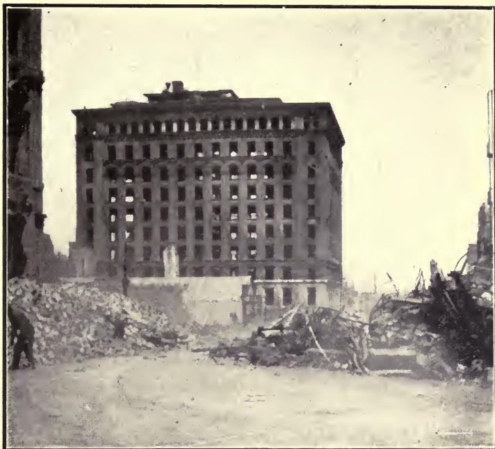
Mills building, looking down Bush street. Brick and steel structure which was injured by fire, property of D. O. Mills.
