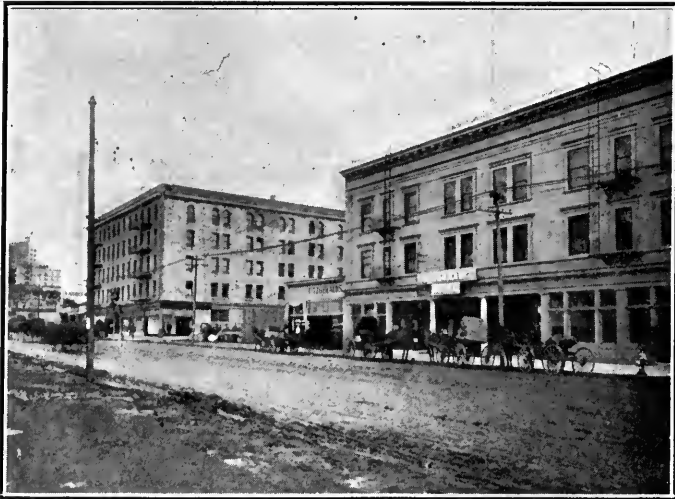
A section of Third, between Howard and Folsom Sts., San Francisco.
