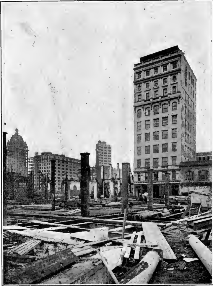
North side of Mission street, near Second. South side is now in course of construction. Atlas building completed.
