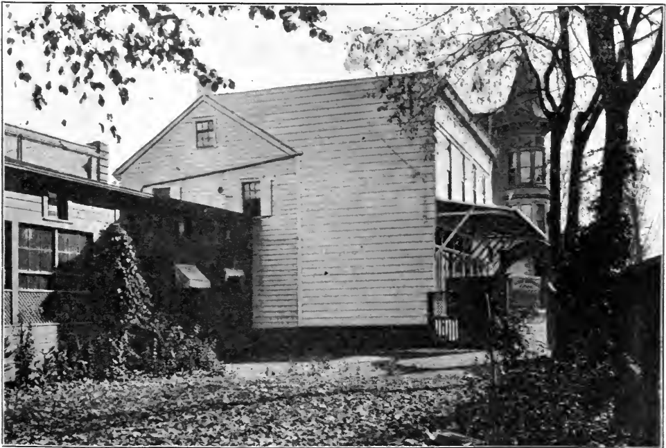
Frederickburg Resort, north side, showing original structure. Entire front has been added later. E. P. Carey, Photo.
