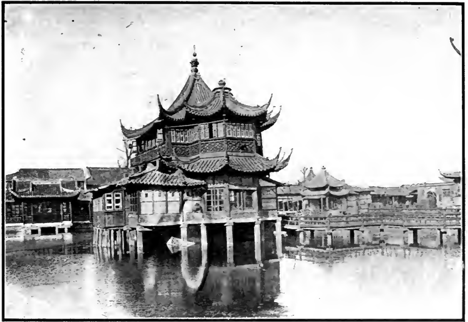
The Willow Pattern Tea House from the north side.
