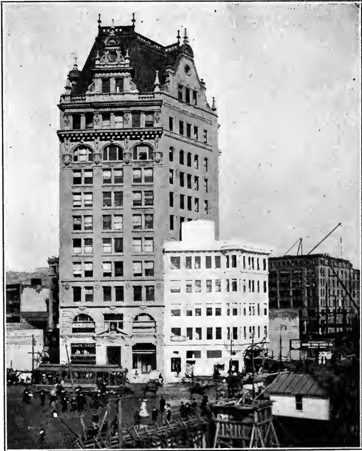
Mutual Savings Bank Building. The five story building adjoining was the first reinforced concrete structure finished since the fire.
