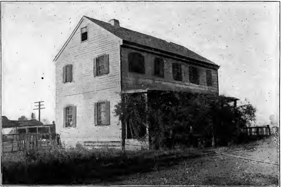
The Watkins house. Shows much neglect in recent years.
