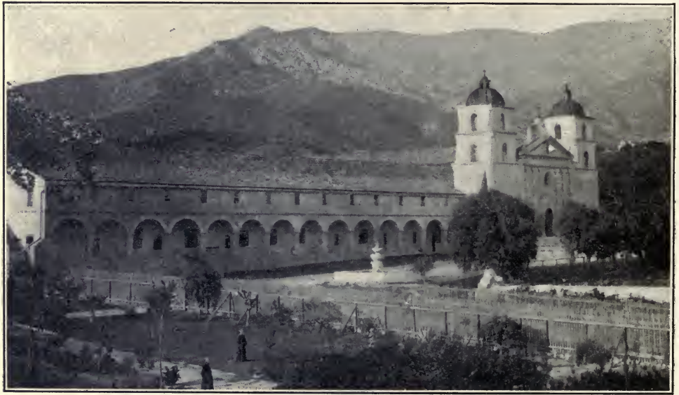
THE MISSION BUILDING AS IT STANDS TO-DAY.
