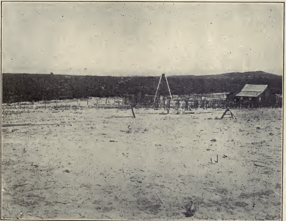
DERRICK AND BUILDINGS ON OIL GROUND, NEAR DEL MONTE HEIGHTS.
