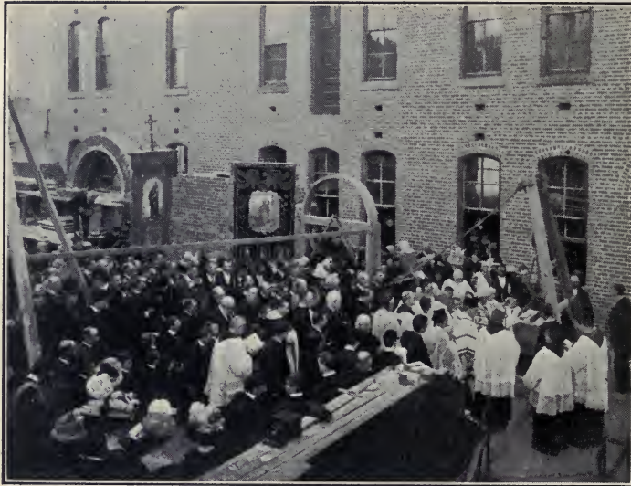
LAYING THE CORNER STONE OF ST. BONIFACE CHURCH
