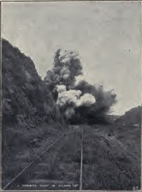
BLASTING WITH DYNAMITE IN CULEBRA CUT.
