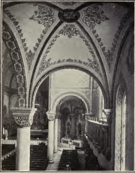
ST. BONIFACE'S CHURCH, GOLDEN GATE AVENUE. FRANCISCAN. BURNED AND NOW BEING REBUILT.
