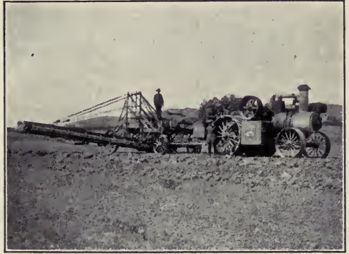
STREET GRADING OUTFIT IN OPERATION AT NEWARK
