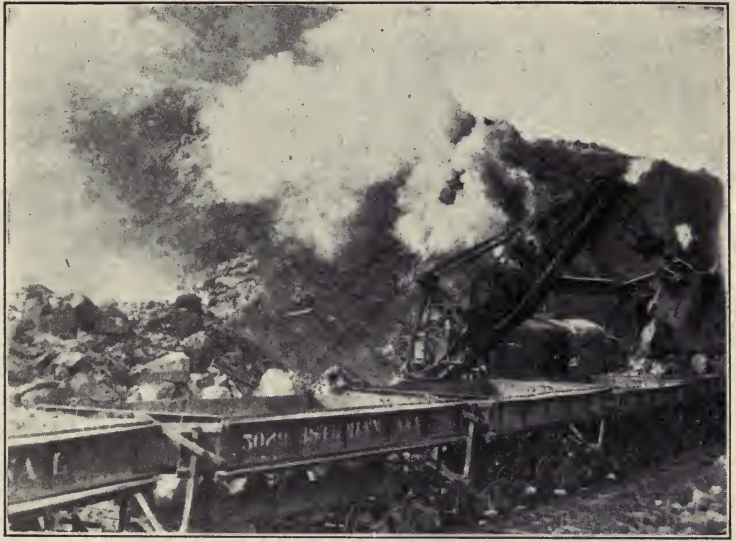
BUCKET DREDGERS IN ACTION AT PANAMA.
