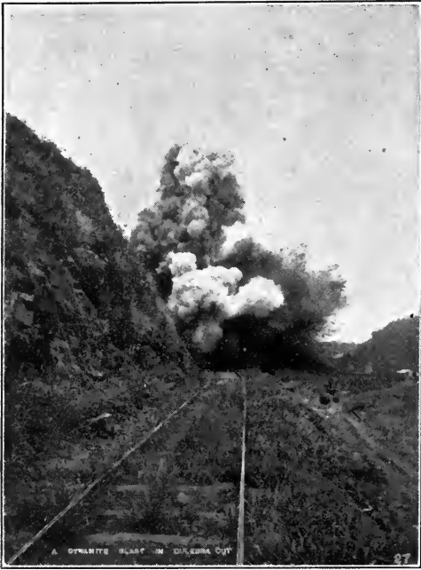
BLASTING WITH DYNAMITE IN CULEBRA CUT.
