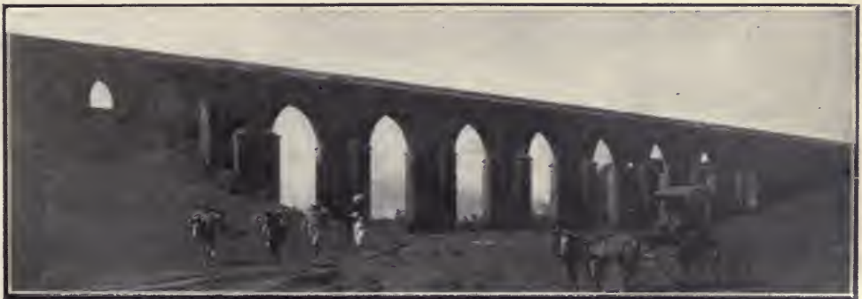
A MAGNIFICENT ENGINEERING WORK. AQUEDUCT ARCH, GUATEMALA.
