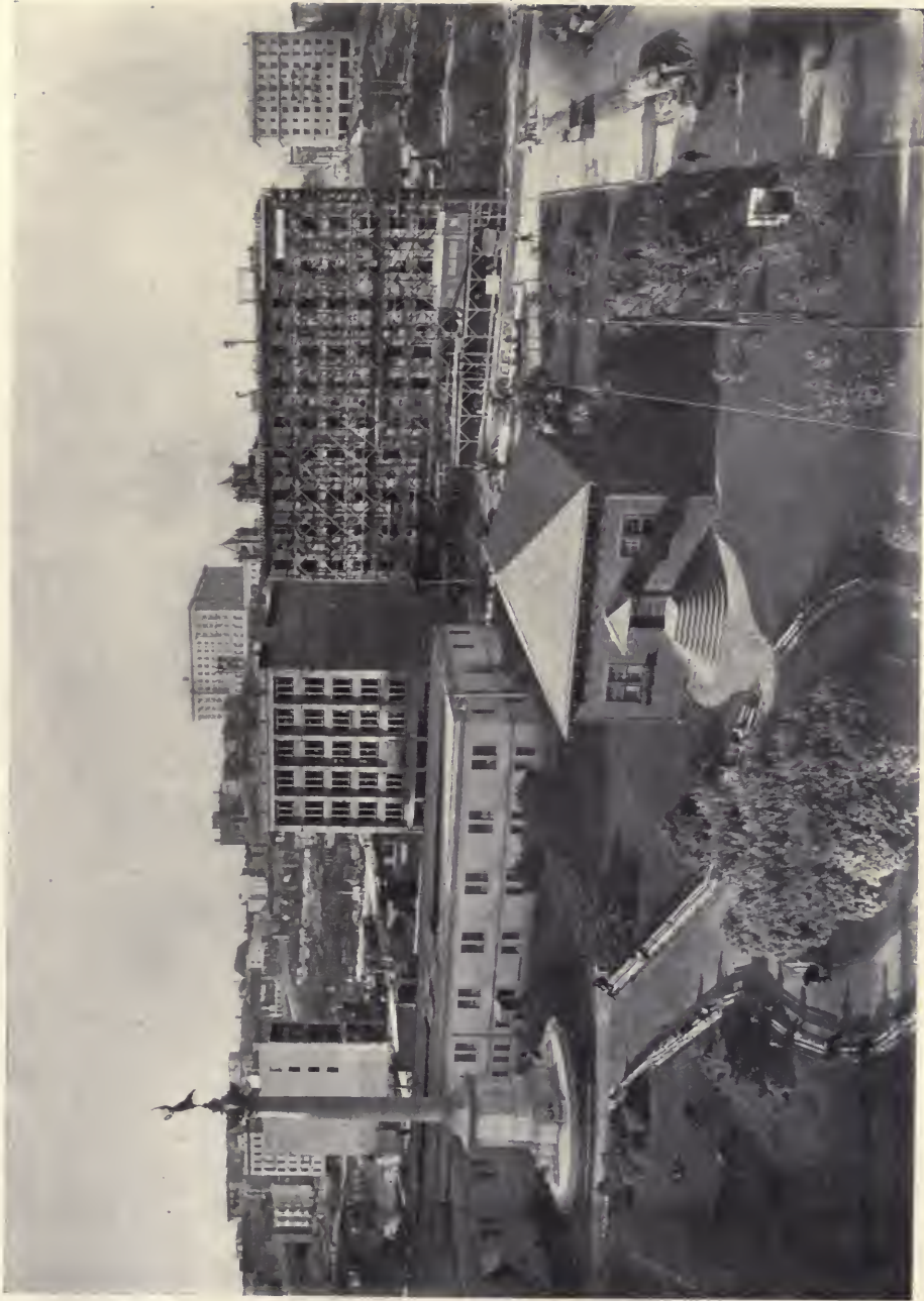
THE BUSIEST CITY IN THE WORLD. —During the time the St. Francis Hotel was being re-constructed, the Little St. Francis was erected on Union Square, alongside the Dewey Monument. The hotel was completed a few weeks ago, and this temporary structure removed.
