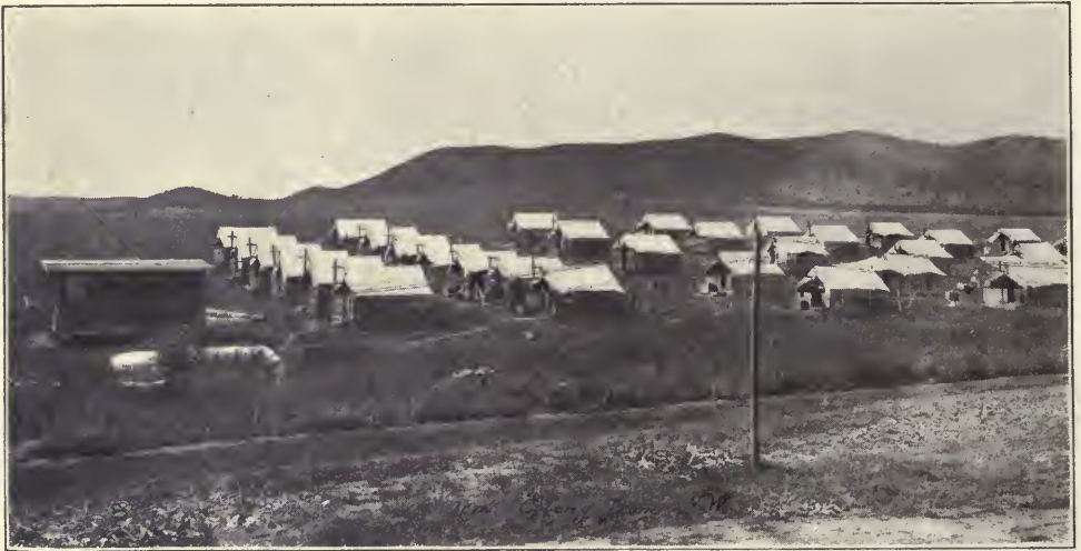
THE TENT SANATORIUM, FORT STANTON, NEW MEXICO.
