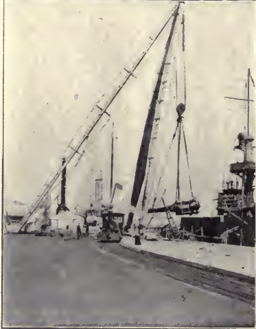
U. S. S. BENNINGTON IN DRY-DOCK. LIFTING 12-INCH GUNS FROM MONITOR WYOMING.
