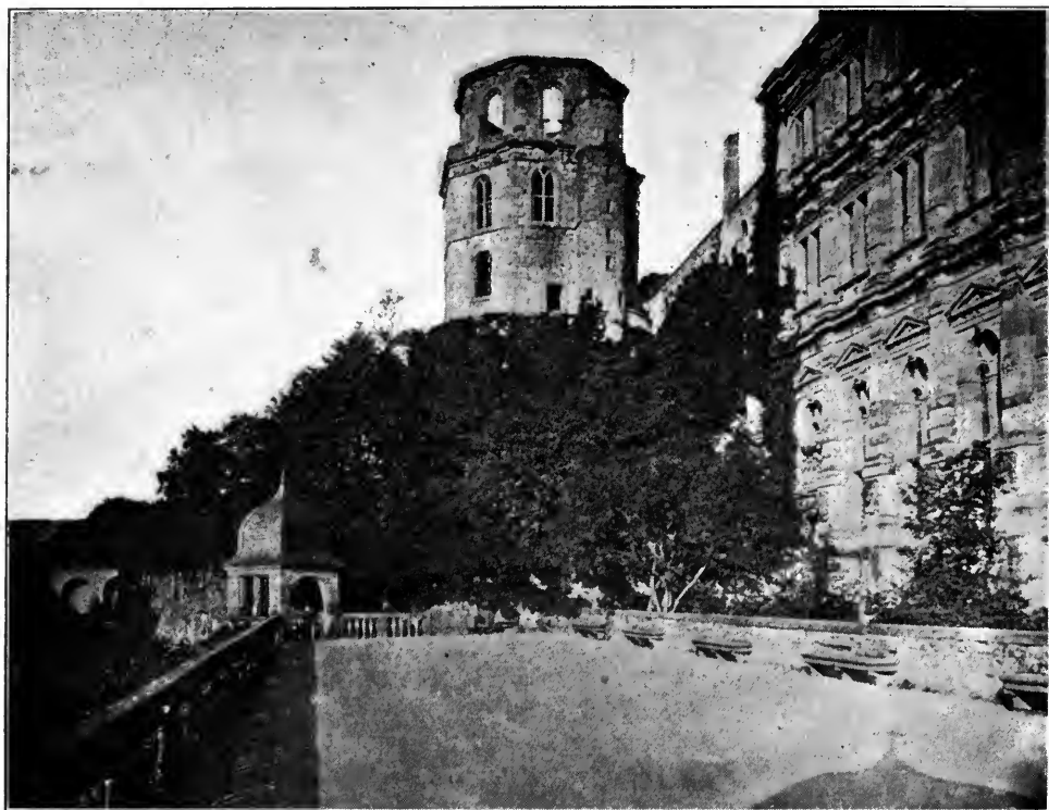
THROUGH GERMANY AND A VISIT TO HISTORIC HEIDELBERG.
