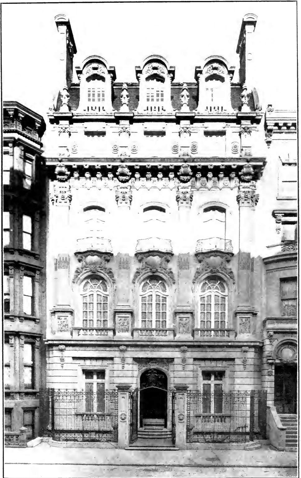
E. H. HARRIMAN'S NEW CITY HOME, 11 EAST SIXTY-SECOND STREET, NEW YORK CITY.
