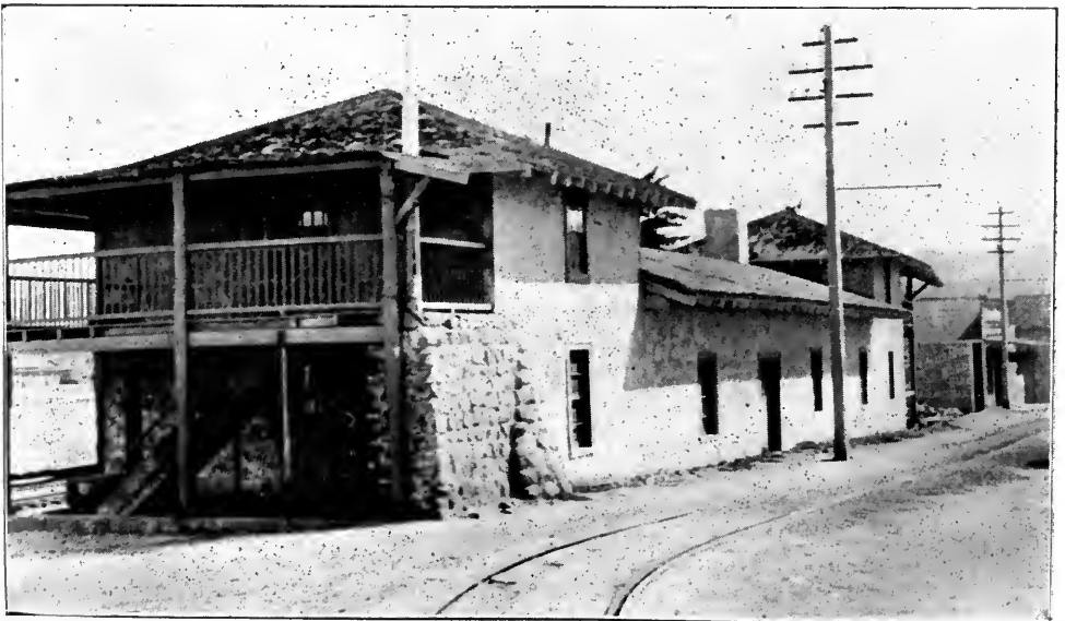
MONTEREY CUSTOMS HOUSE AFTER RESTORATION.
