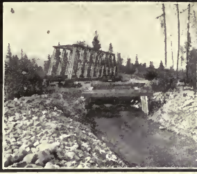
Head gate on Ward Ditch.
