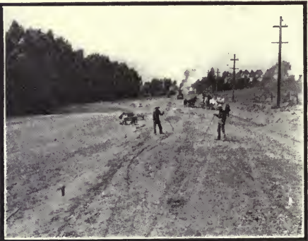
SURFACING THE BOULEVARD.
