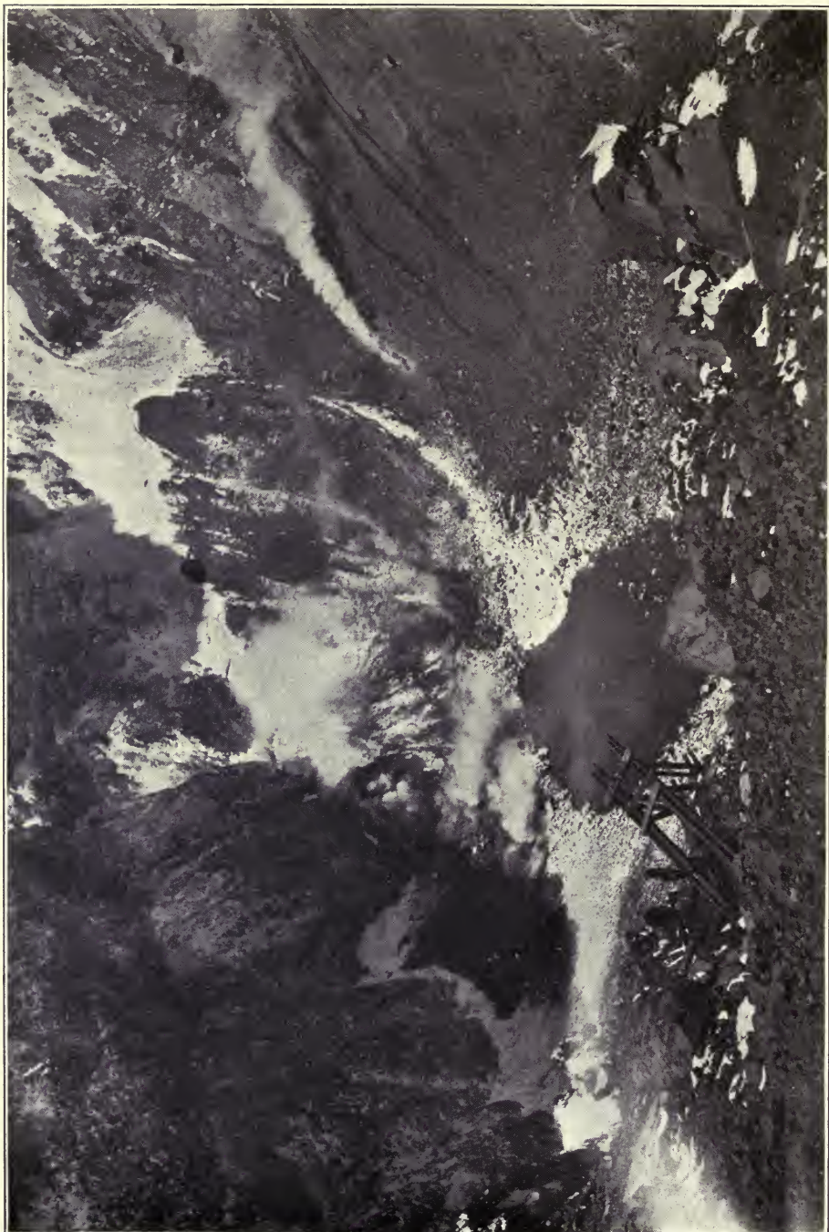
MARVELOUS MEXICO—The crater of Popocotapi. This interesting picture shows a derrick over a two hundred foot precipice. Here men are let down to mine sulphur and the product is hauled upward by means of the same gear. Photo. Sumner W. Matteson.
