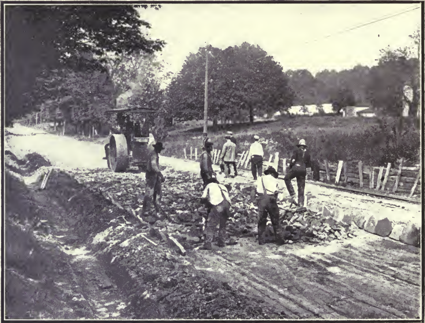
CLEVELAND TO PAYNESVILLE ROAD, BUILT BY THE AUTOMOBILE CLUB. SHOWING THE THOROUGH MANNER IN WHICH THE ROAD WAS LAID.
