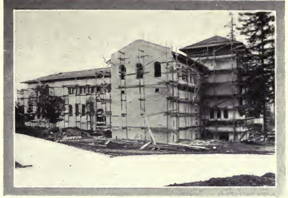
AN EXHIBITION BUILDING STILL IN COURSE OF CONSTRUCTION.
