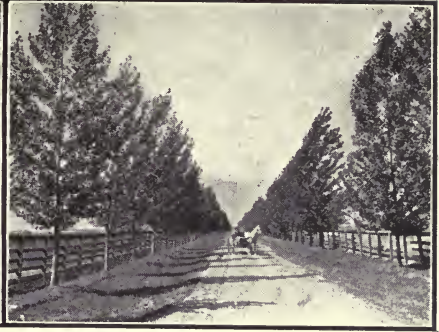
There are miles of these drives in the Bitter Root Valley. The county spends thousands every year in keeping them in shape.
