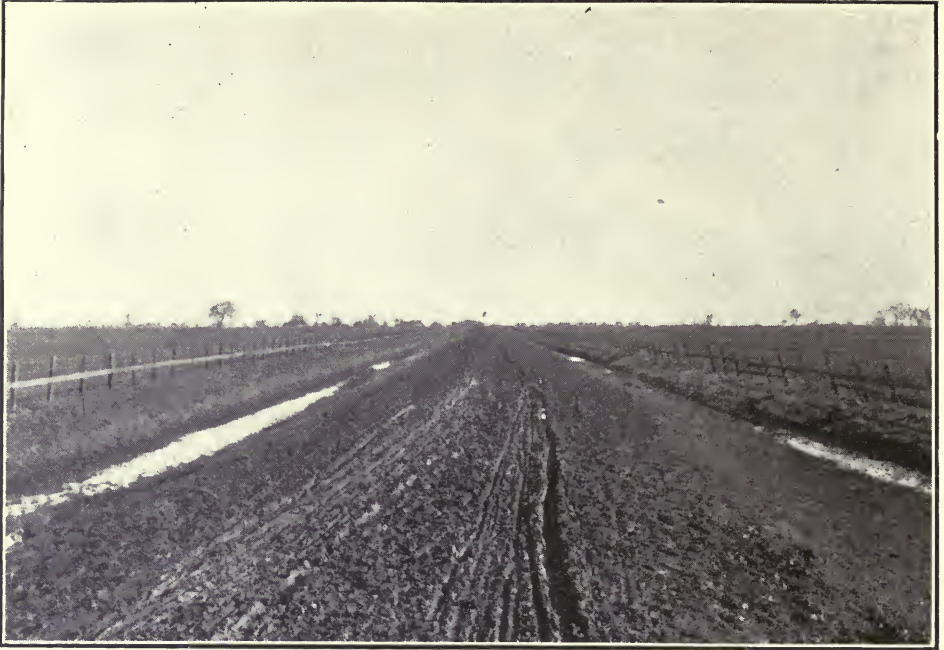
PORTION OF MARIPOSA ROAD NEAR STOCKTON BEFORE BEING IMPROVED.
