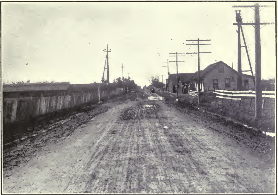
“OBJECT LESSON” ROAD NEAR STOCKTON, WHERE IT MERGES INTO A CITY STREET
