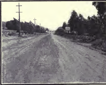
THE FINISHED ROADWAY.
